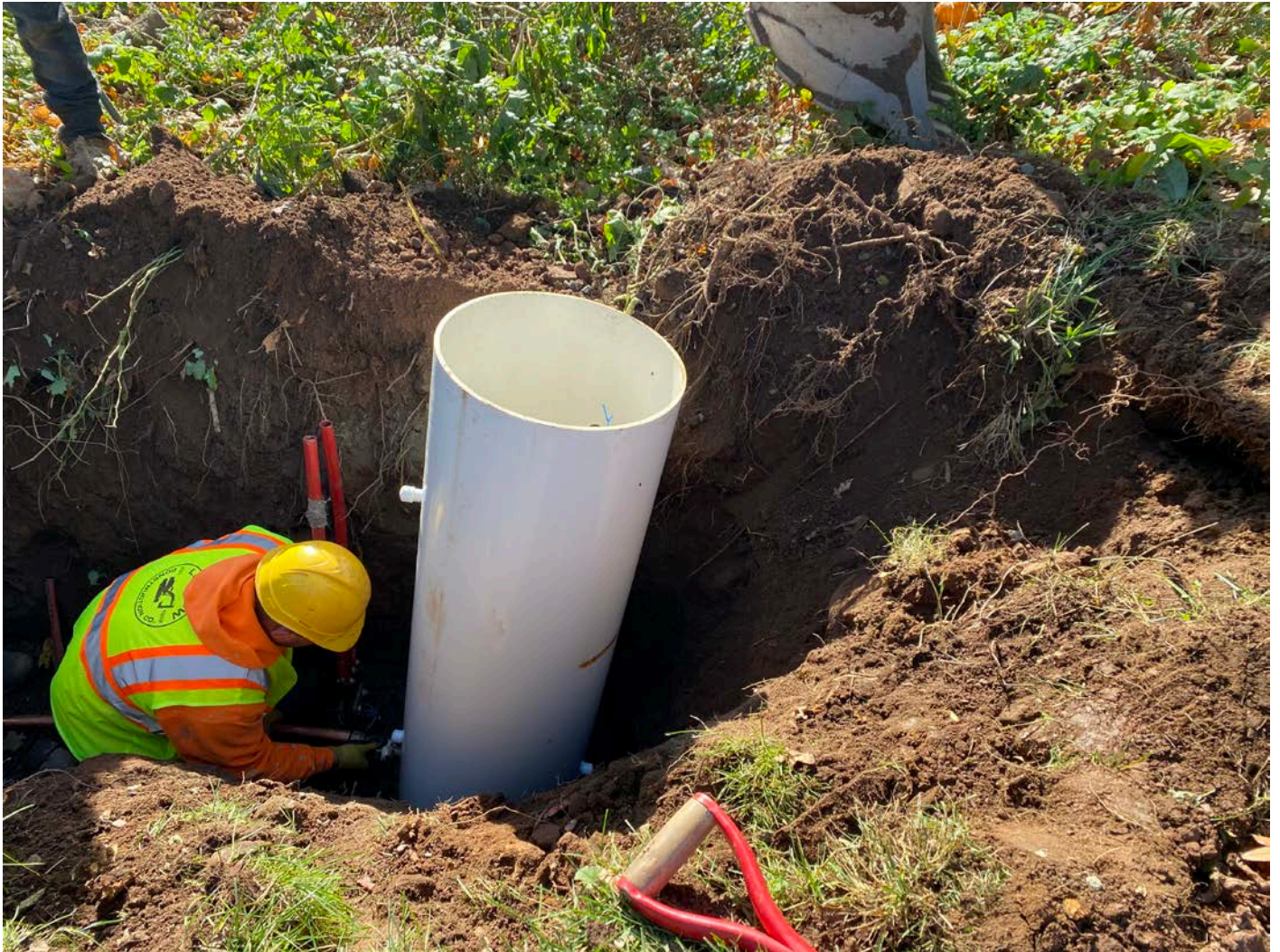
Picture 3: Ludlow installs the meter pit for the installation of a 1.5” copper water service line for the 228R Maple Ave residence. Looking south.
