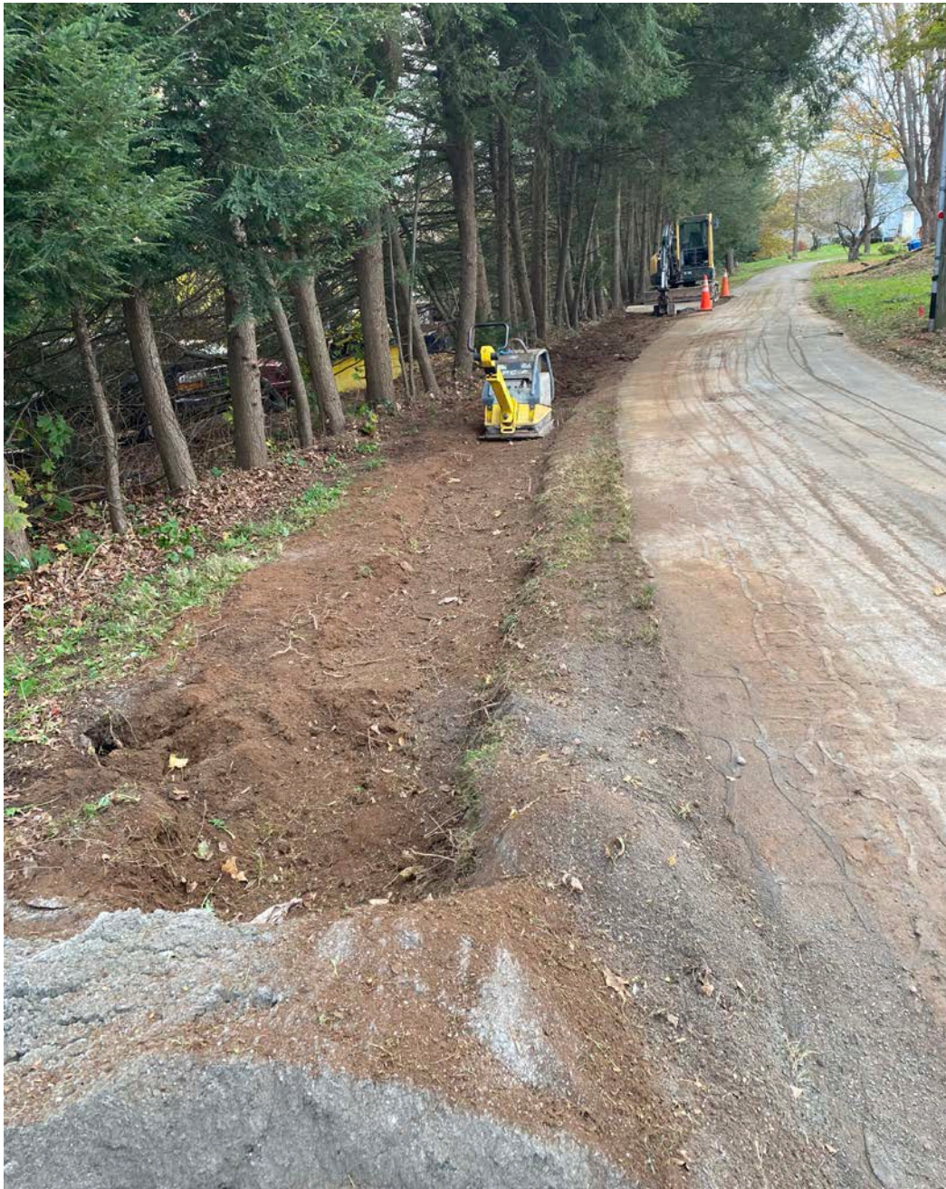
Picture 10: Ludlow compacts the backfill in the trench of the 1.5” copper water service line to 212R Maple Ave. residence looking west.
