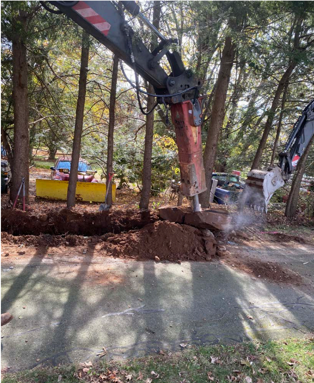
Picture 8: Ludlow uses the jack hammer to break a small section of rock in the trench. Looking south.
