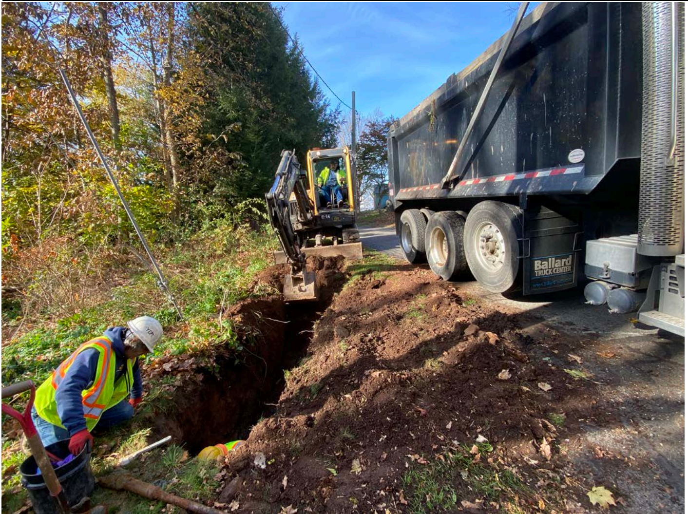
Picture 2: Ludlow excavating the trench for the installation of a meter pit just south of the driveway of the 228R Maple Ave residence. Looking west.
