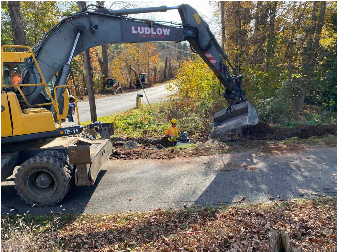
Picture 7: Ludlow places sand around the area with the meter pit at the 228R Maple Ave residence. Looking south.
