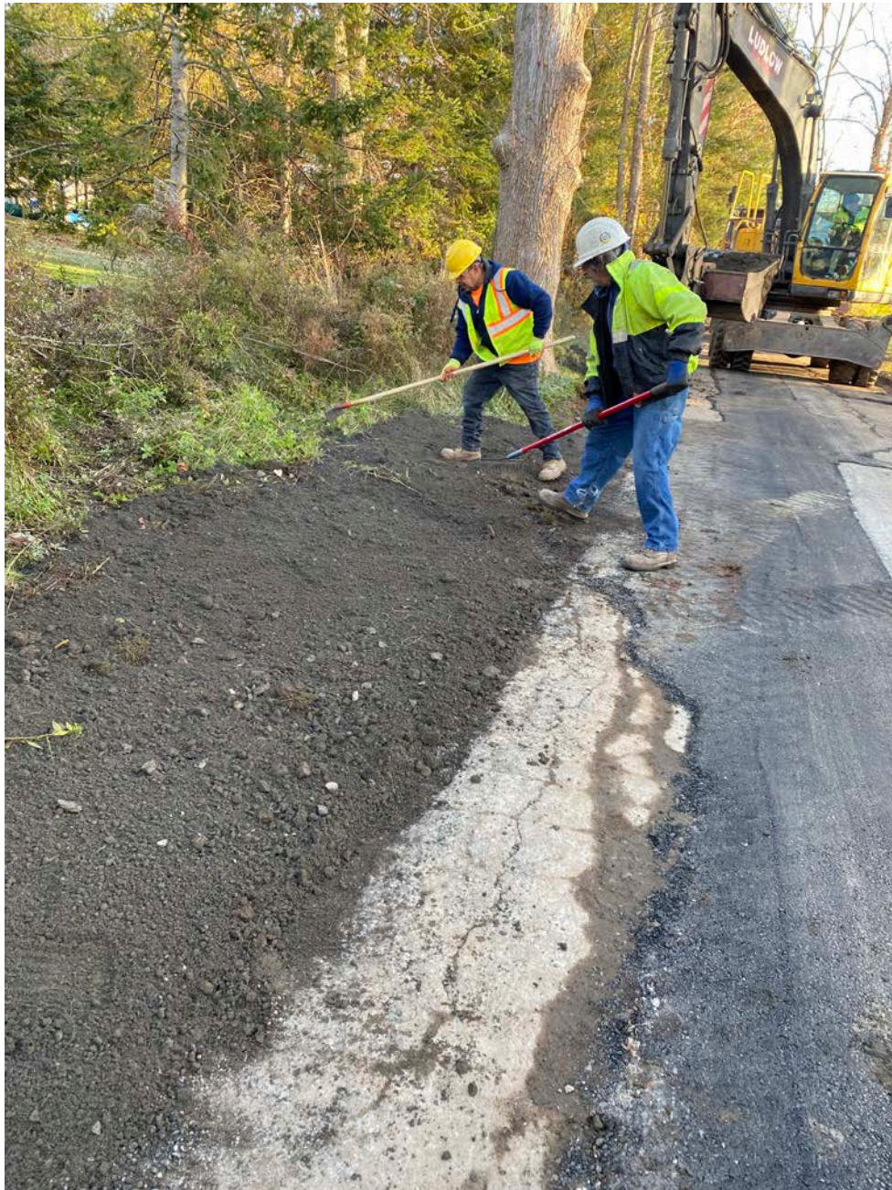
Picture 1: Ludlow loaming and seeding the disturbed area surrounding the driveway of the 212R Maple Ave residence. Looking West.
