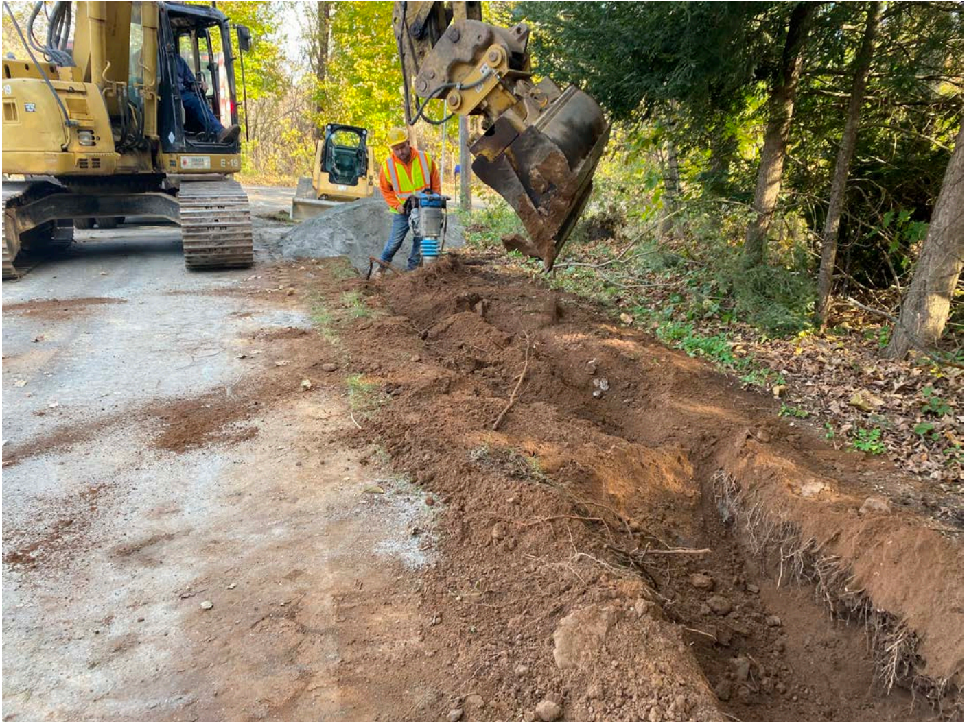
Picture 9: Ludlow backfills the trench of the 1.5” copper water service line to 228R Maple Ave. residence with native fill. Looking east.
