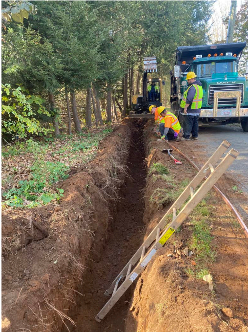
Picture 5: Ludlow excavates a trench at the 228R Maple Ave property for the placement of a 1.5” copper service line. Looking west.
