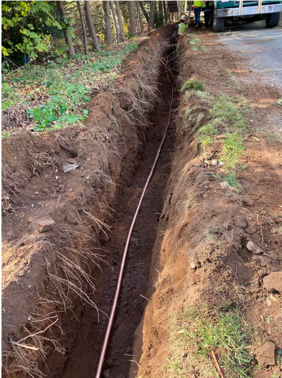
Picture 6: Ludlow placing a segment of the 1.5” copper service line in the trench for the 228R Maple Ave. residence property in Durham. Looking west.
