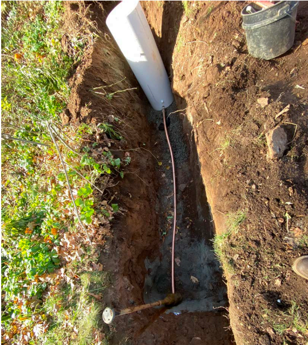
Picture 4: Ludlow connects the new meter pit to the curb stop at the 228R Maple Ave residence. Looking west.
