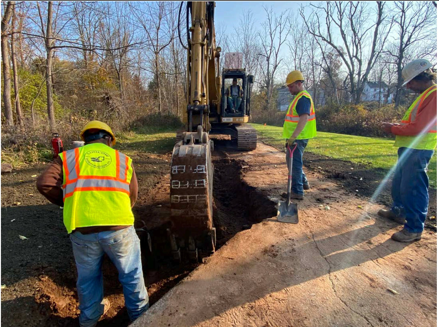
Picture 3: Ludlow excavates a depth of 1' in the original trench down the driveway of the 212R Maple Ave residence. Looking East.
