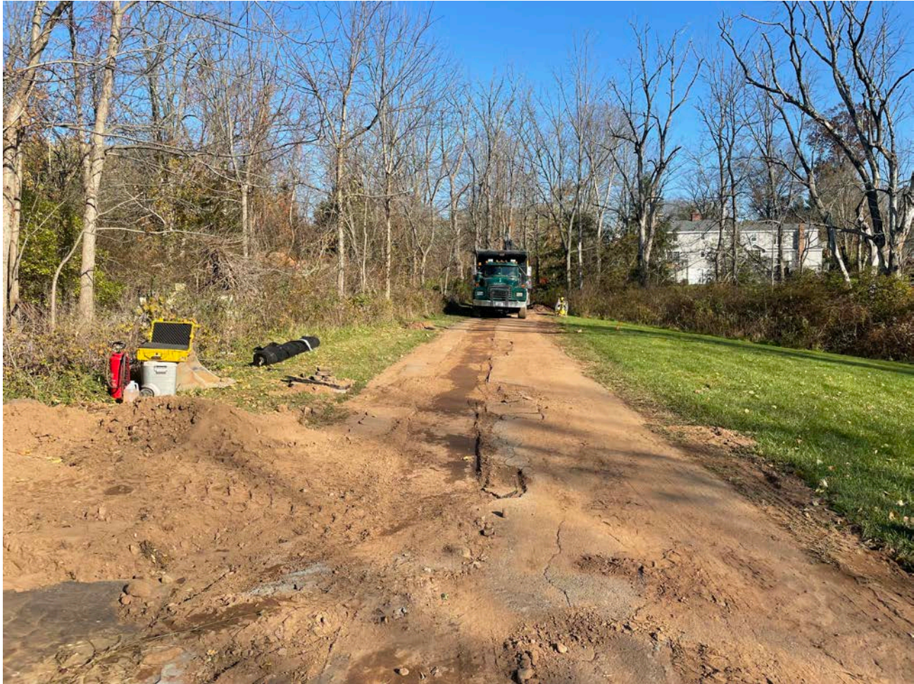
Picture 7: View of the progress at the end of the day at the 212R Maple Avenue property where Ludlow installed a 1.5" copper water service line. View to the east.
