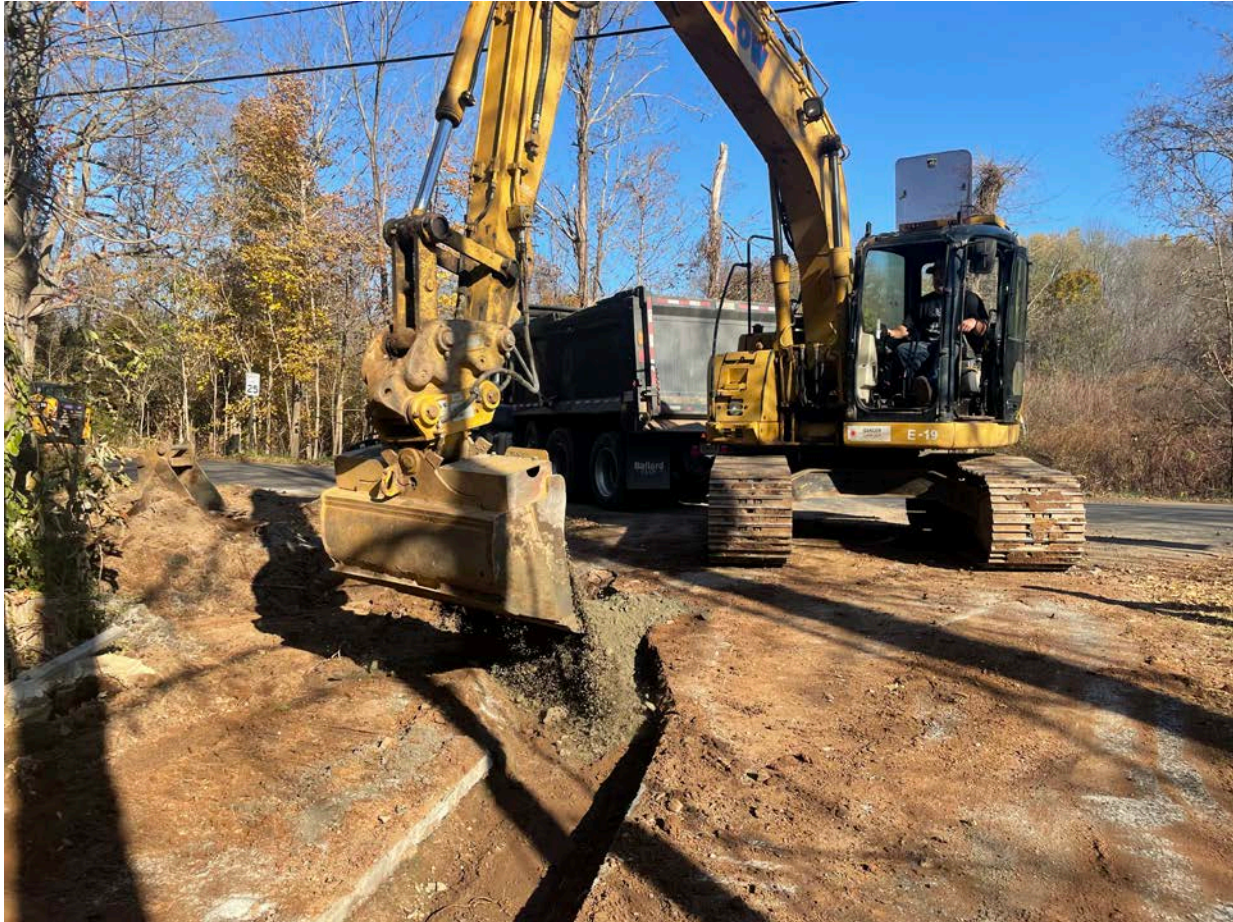
Picture 6: Ludlow placing an 18' layer of 1.25"-minus gravel in the trench that was excavated for the installation of a 1.5" copper water service line at the 212R Maple Avenue property. View to the east.
