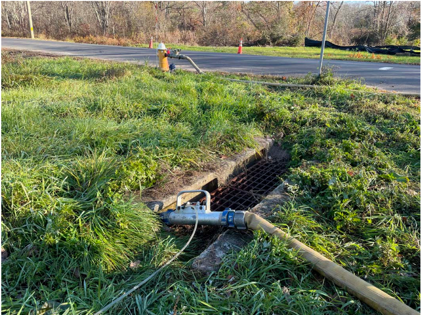
Picture 2: JMS in the process of introducing calcium thiosulphate into the chlorinated water that is being purged from the Pickett Lane and Maiden Lane water lines. The water is being discharged into a catch basin located on the northwest corner of the intersection of Brick Lane and Maiden Lane. View to the northeast.
