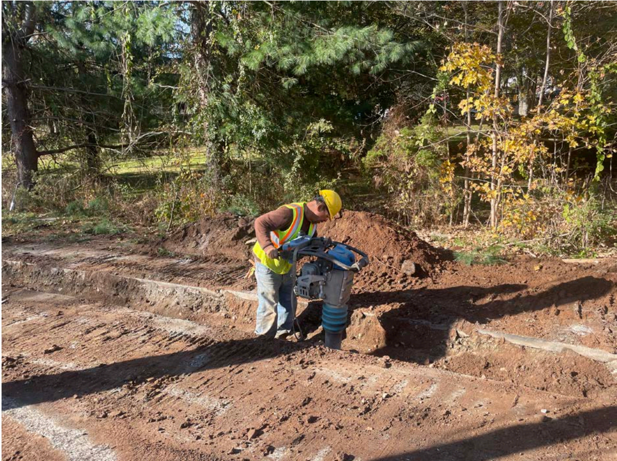
Picture 5: Ludlow compacting native fill that was placed in 1' lifts over the sand and caution tape that was placed over the 1.5" copper water service line Ludlow installed at the 212R Maple Avenue property. View to the northwest.
