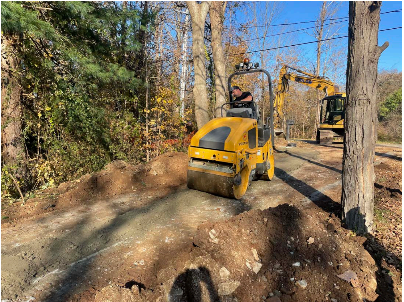
Picture 8: Ludlow compacting 1.25"-minus gravel in the trench that was excavated for the installation of a 1.5" copper water service line at the 212R Maple Avenue property. View to the east.
