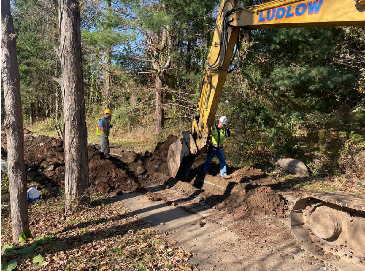
Picture 4: Ludlow excavating a trench on the driveway of the 212R Maple Avenue property for the installation of a 1.5" copper water service line. View to the west.
