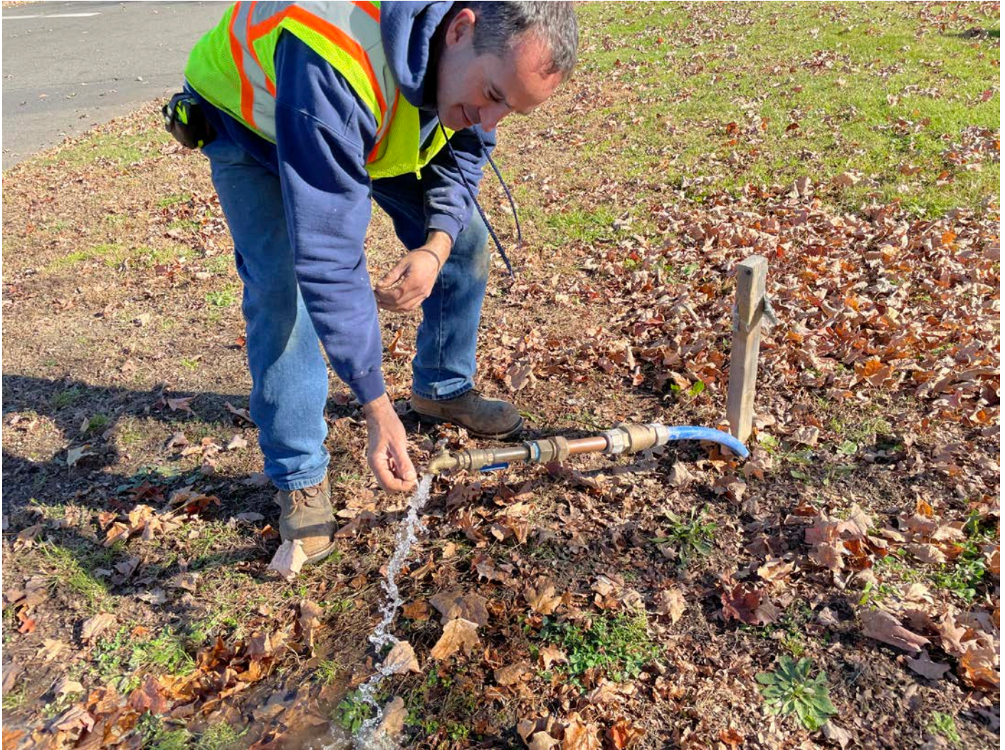
Picture 10: Ludlow testing the concentration of chlorine in the Pickett Lane waterline at Station ~525+28 as JMS is introducing sodium hypochlorite from an upstream point on the water line.
