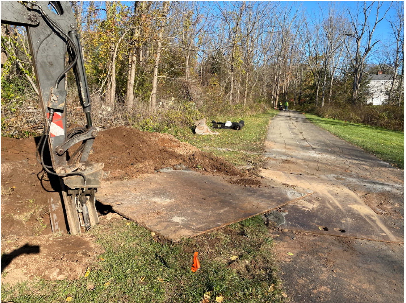
Picture 10: Ludlow places a plate over the section of open trench where the construction for the connection of the 1.5" copper water service line to 212R Maple Ave will resume on Monday. Looking East.
