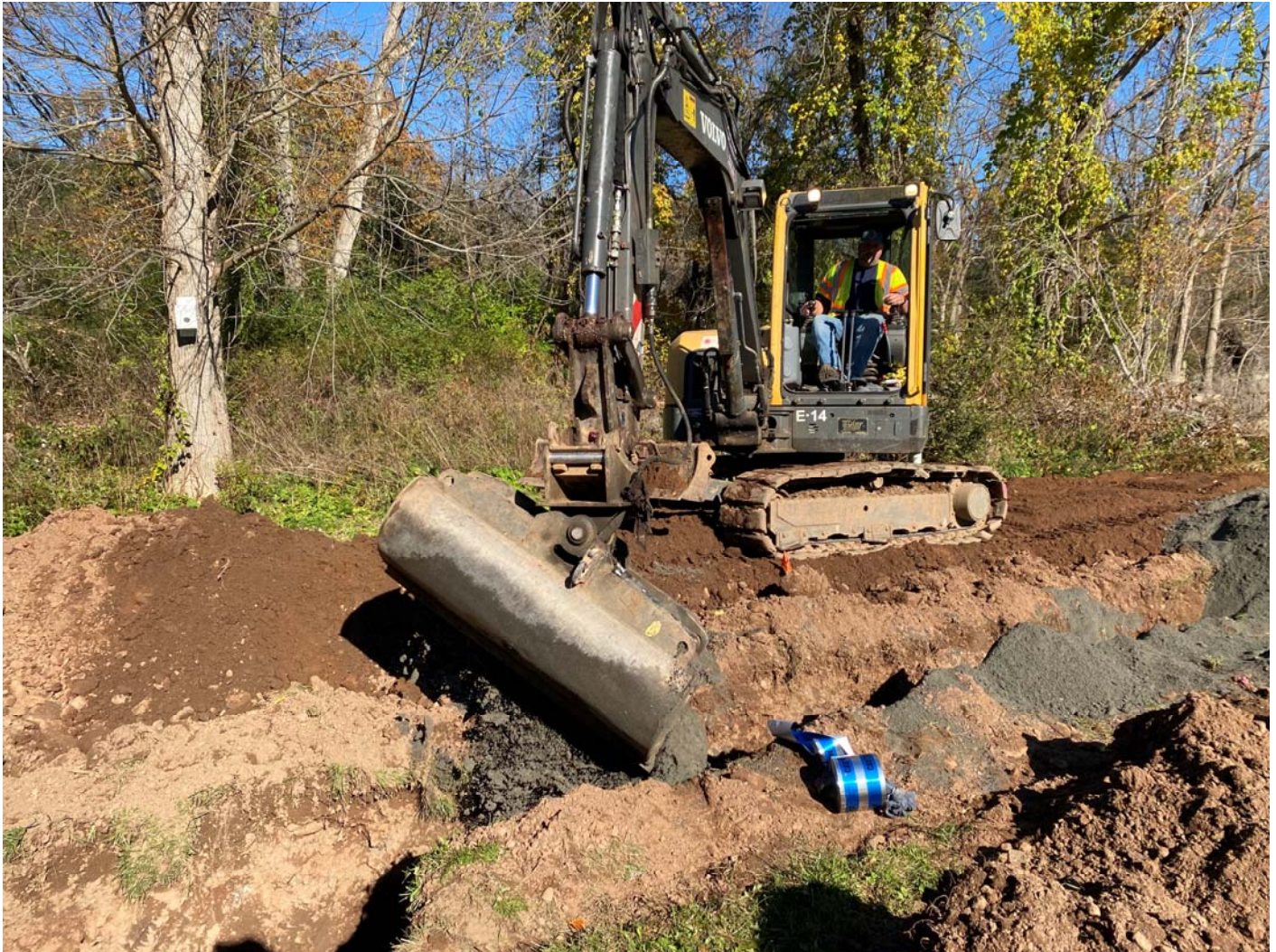
Picture 8: Ludlow backfills the trench of the 1.5” copper water service line to 212R Maple Ave residence with native fill. Looking North.
