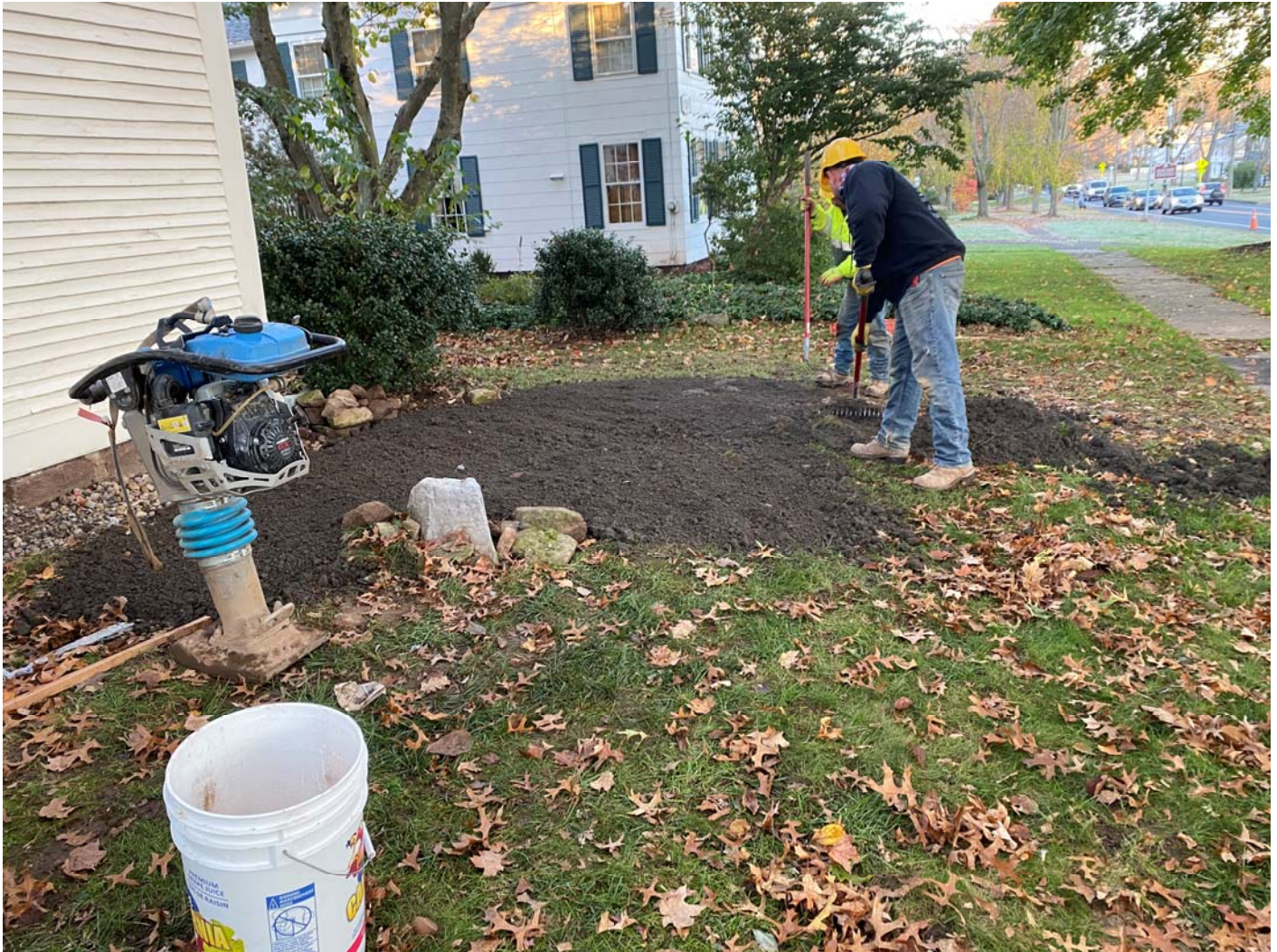
Picture 2: Ludlow grades and loams the disturbed area of the 248 Main Street residence. Looking North.
