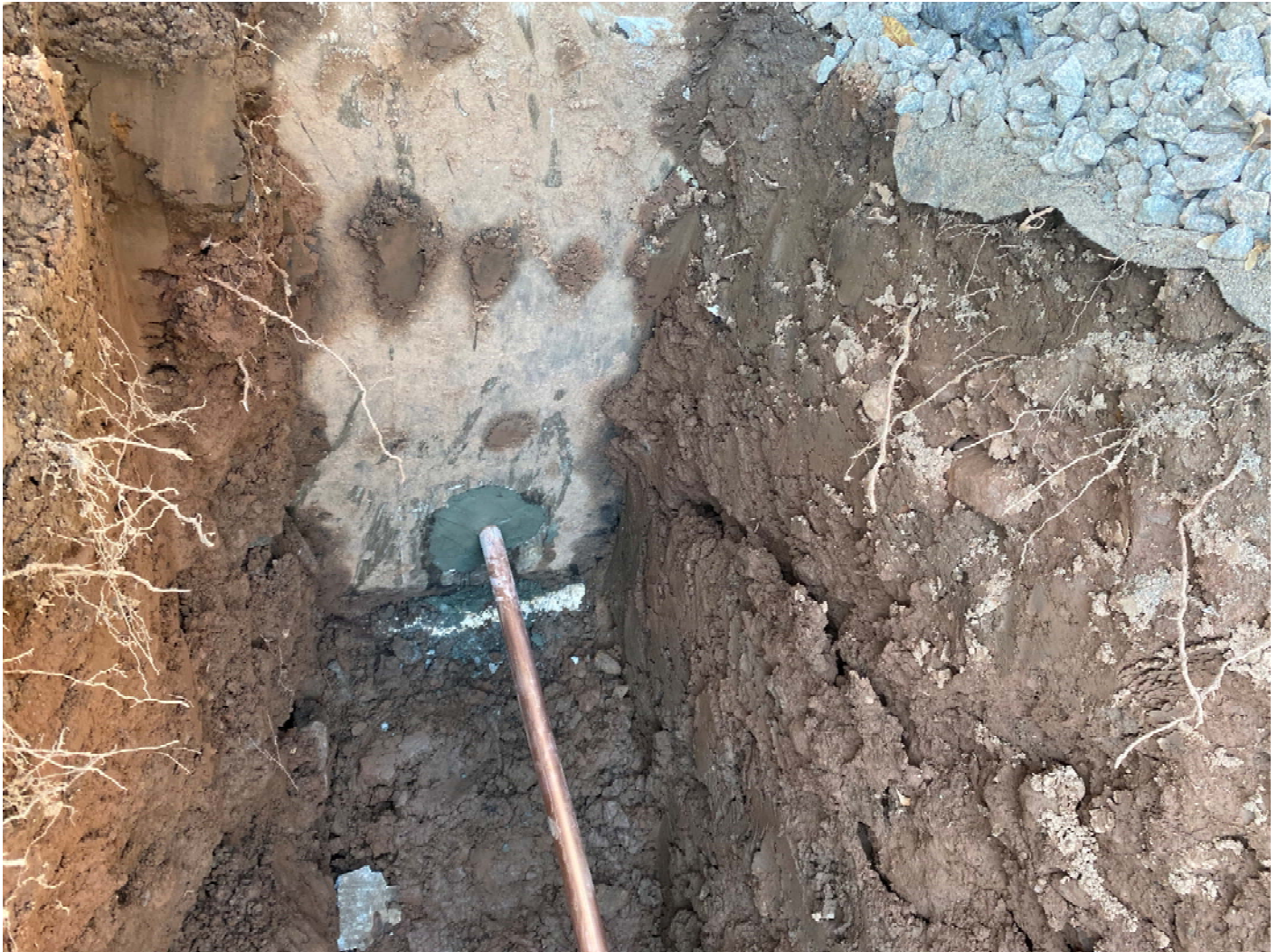
Picture 6: Ludlow inserts the 1.5” copper service line through the foundation of the Northeast corner of the 212R Maple Ave residence. Looking West.
