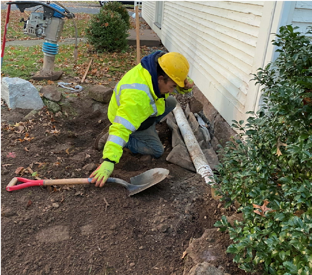
Picture 1: Ludlow restoring the previously sealed area around the connection to the 248 Main Street residence. Looking South.
