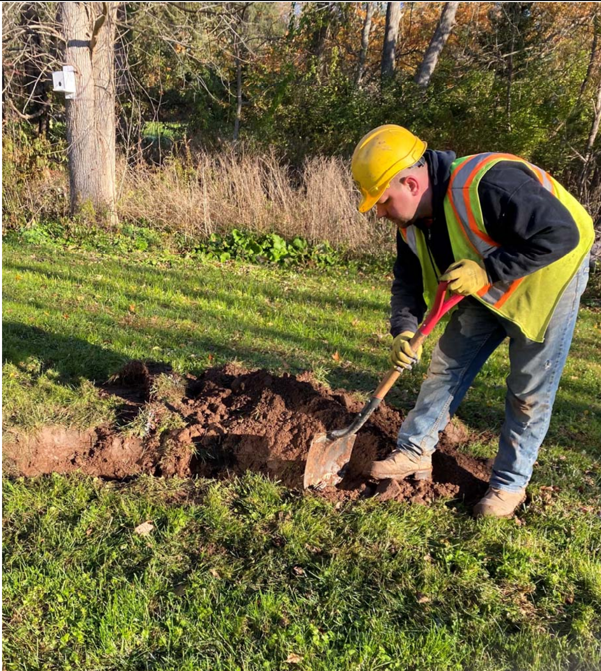
Picture 3: Ludlow hand digs to locate an existing electric utility line at the 212R Maple Ave residence. Looking North.
