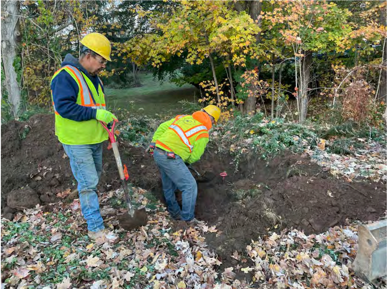
Picture 1: Ludlow preparing to remove the curb stop for the 212R Maple Avenue property, to be reinstalled later today south of this location. View to the west.
