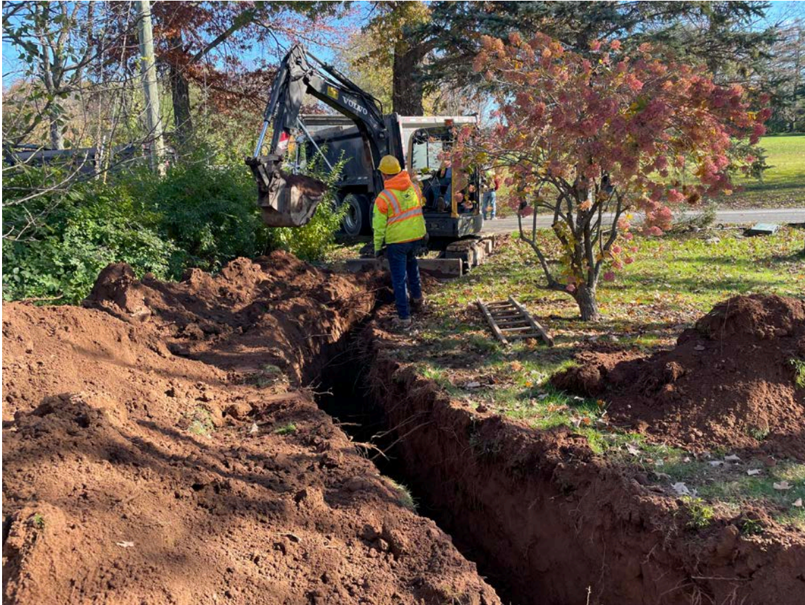
Picture 3: Ludlow excavating a trench at the 200 Maple Avenue residence for the installation of a 1" copper water service line. View to the east.
