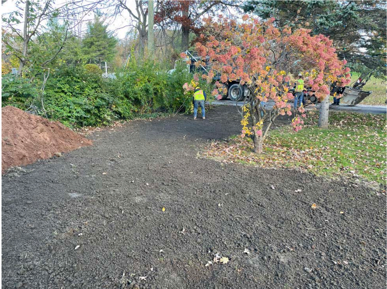
Picture 6: Ludlow raking out loam at the 200 Maple Avenue residence after the installation of a 1" copper water service line. View to the east.
