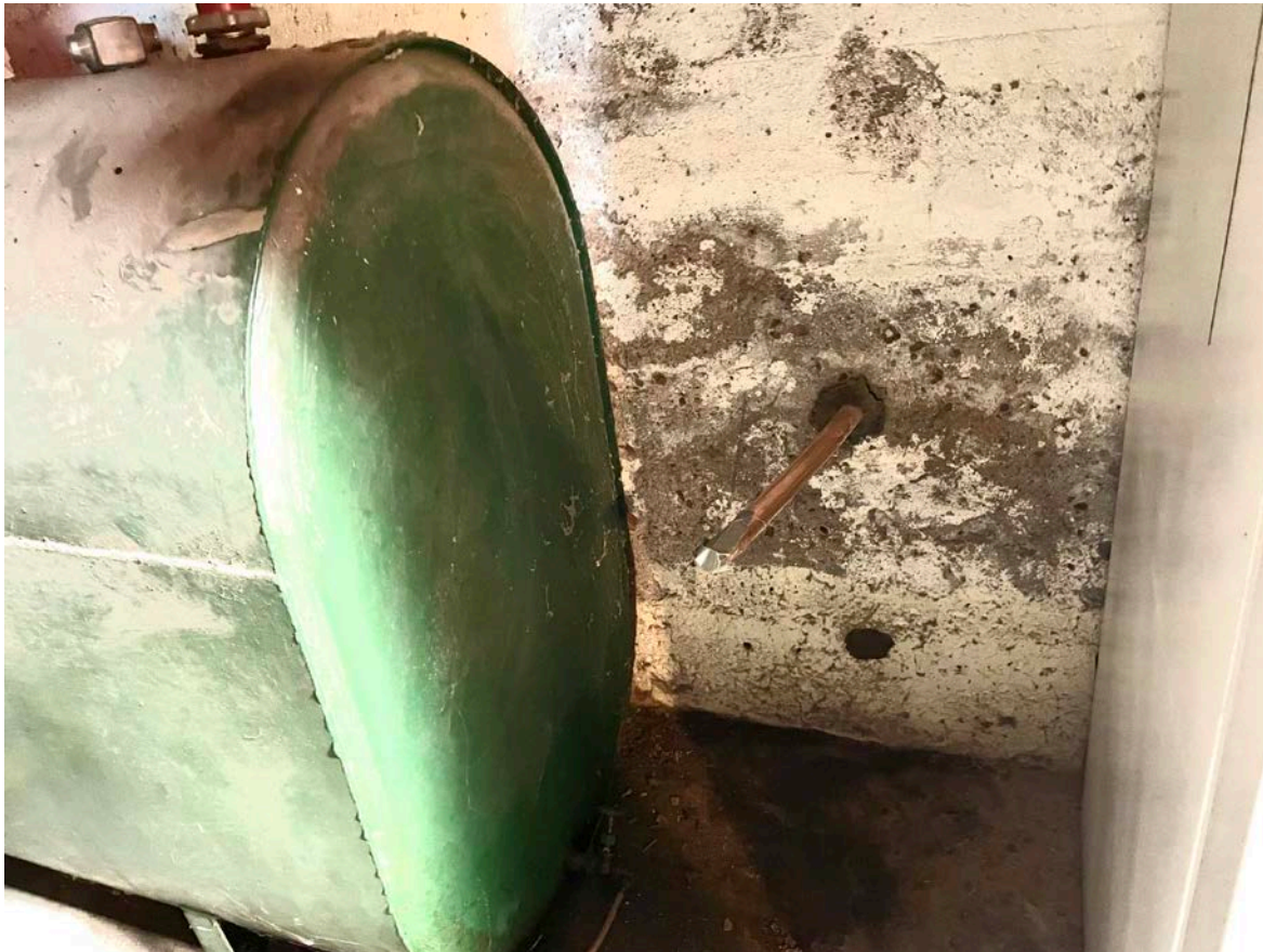
Picture 7: Copper pipe penetrating the eastern wall of the 200 Maple Avenue foundation. View to the east.
