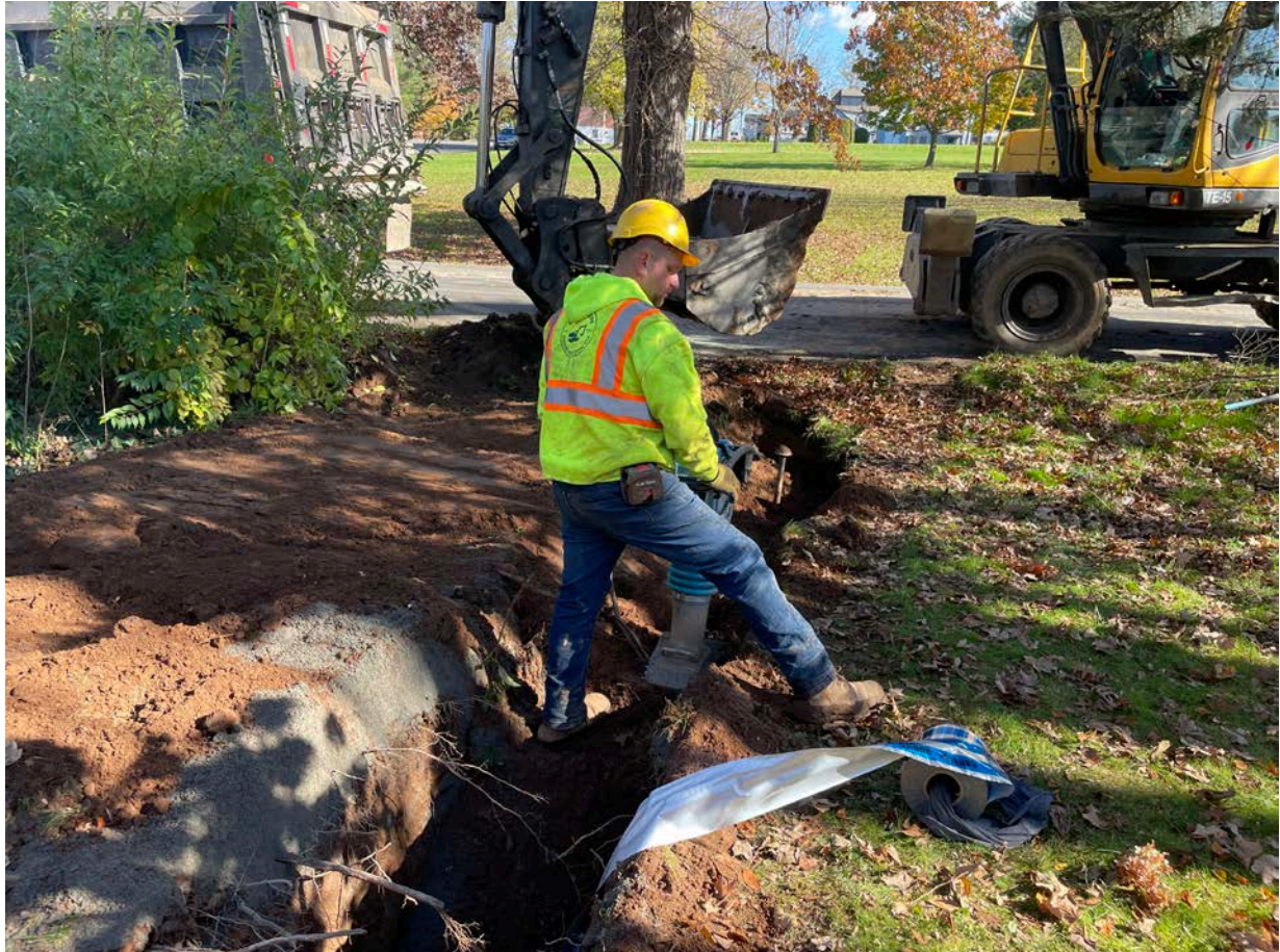
Picture 4: Ludlow compacting fill in the trench they excavated at the 200 Maple Avenue residence during the installation of a 1" copper water service line. View to the east.
