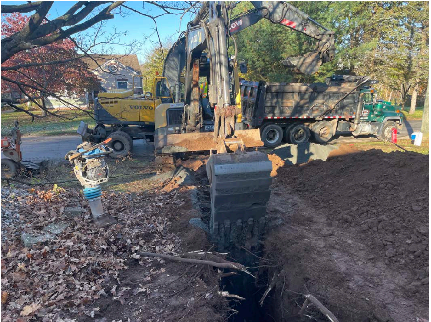
Picture 2: Trench that Ludlow is excavating at the 187 Maple Avenue residence for the installation of a 1” copper water service line. View to the northwest.
