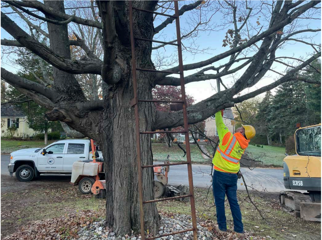
Picture 1: Ludlow is using a chainsaw to trim some branches off a tree that's in the path of the 1" copper water service line they installed at the 187 Maple Avenue residence today. View to the west.
