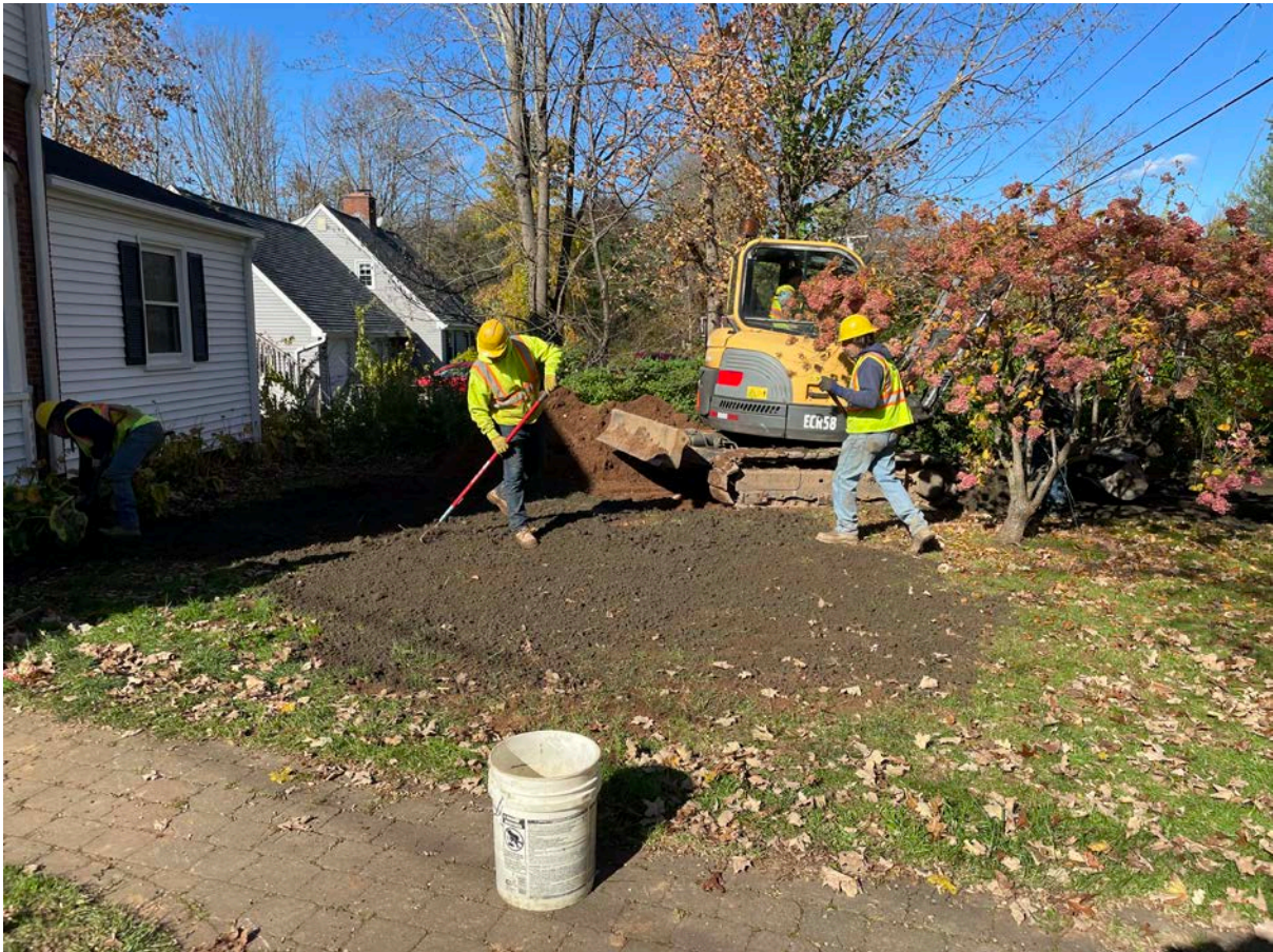
Picture 5: Ludlow placing and raking out loam at the 200 Maple Avenue residence after the installation of a 1" copper water service line. View to the north.
