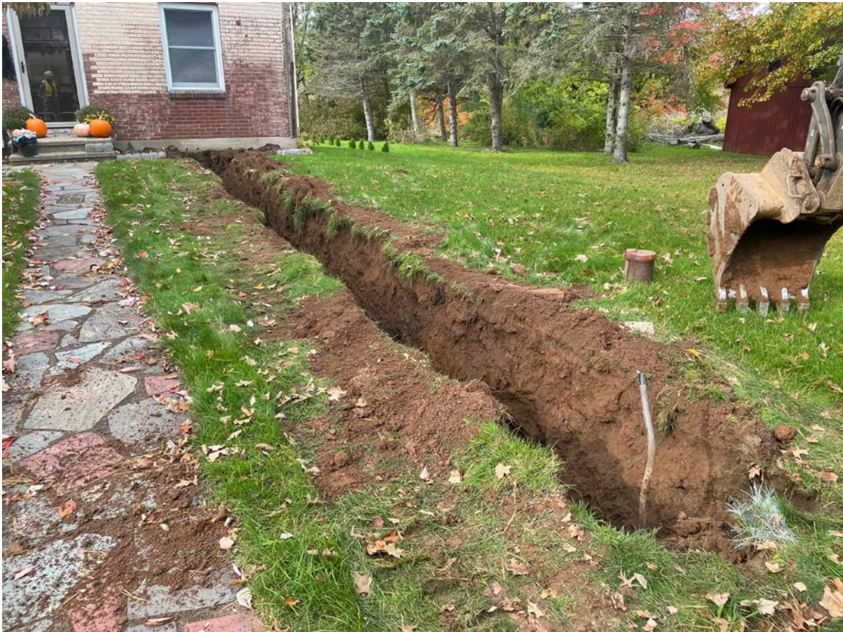
Picture 5: Trench that Ludlow has excavated at the 188 Maple Avenue residence for the installation of a 1" copper water service line. View to the west.
