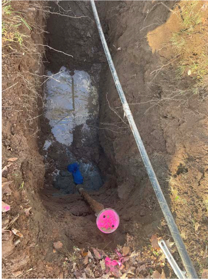
Picture 3: Water observed pooling at the east end of the trench that Ludlow has excavated at the 184 Maple Avenue residence for the installation of a 1" copper water service line.
