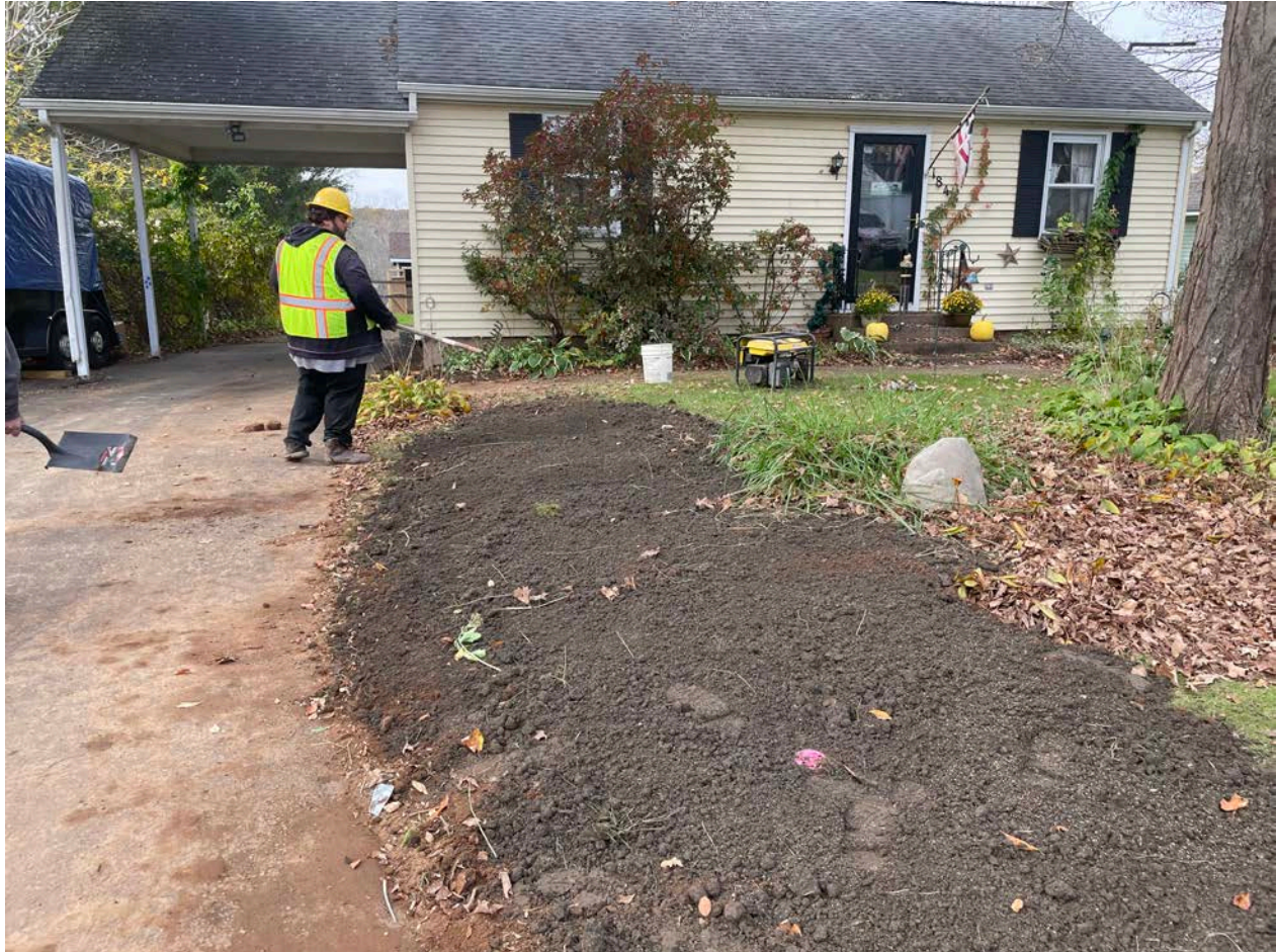
Picture 6: Ludlow raking out loam that they placed on the portions of the 184 Maple Avenue property that were disturbed during the installation of a 1" copper water service line. View to the west.
