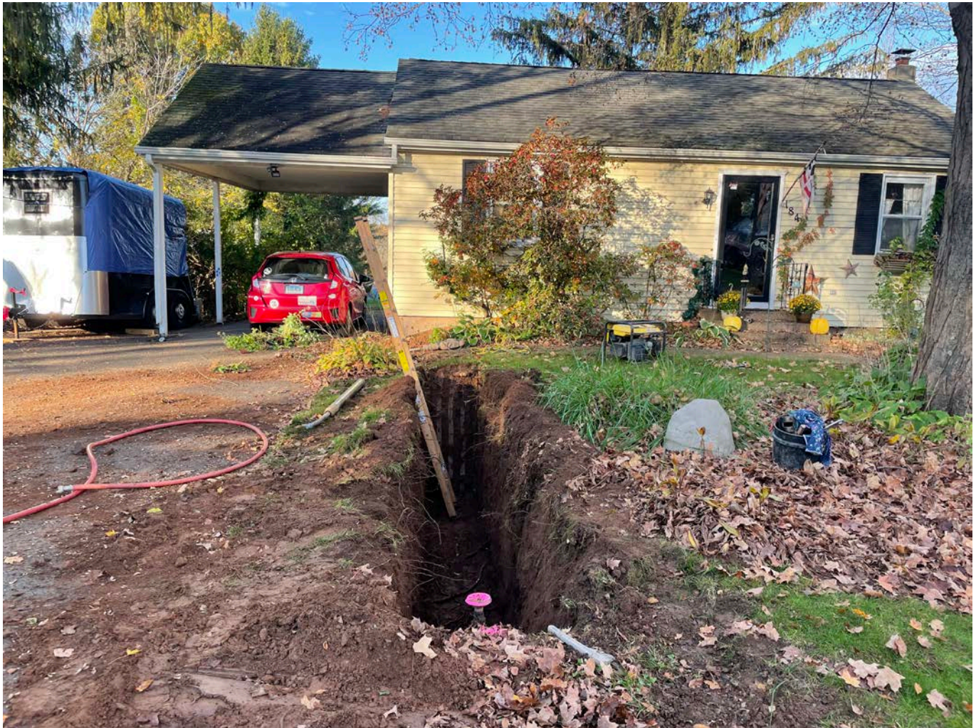
Picture 2: Trench that Ludlow has excavated at the 184 Maple Avenue residence for the installation of a 1" copper water service line. View to the west.
