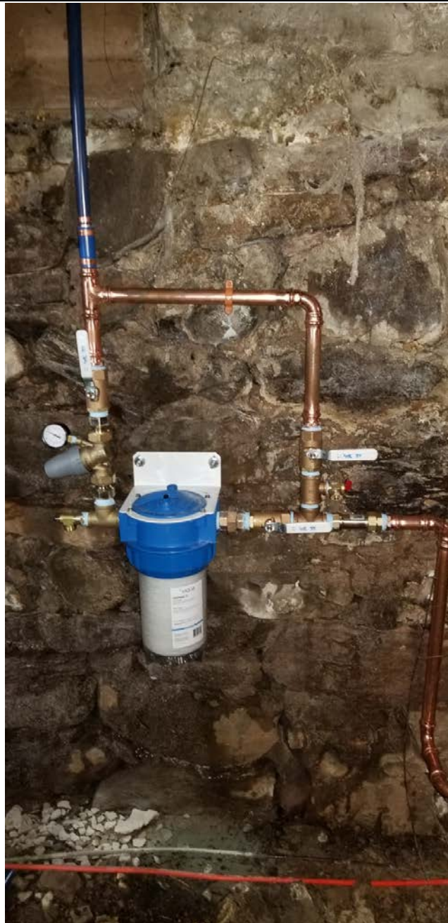
Picture 8: Final water service components that Fazzino Plumbing installed at the 208 Main Street, Durham, residence.
