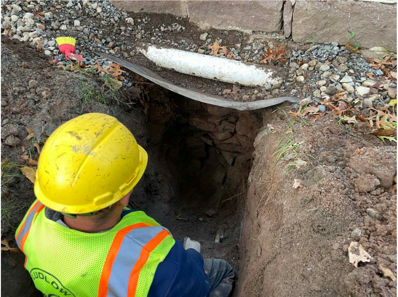
Picture 1: Ludlow placing non-shrink grout on a section of the eastern foundation of the 248 Main Street residence. View to the west.
