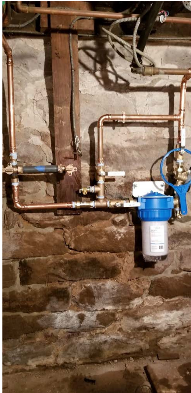
Picture 7: Final water service components that Fazzino Plumbing installed at the 110 Maple Avenue, Durham, residence.
