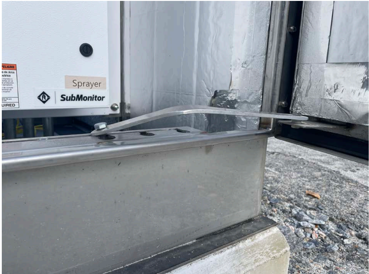
Picture 4: Bent support arm on one of the south-facing doors of the electrical cabinet located north of the altitude vault at the water tank work zone. View to the northeast.
