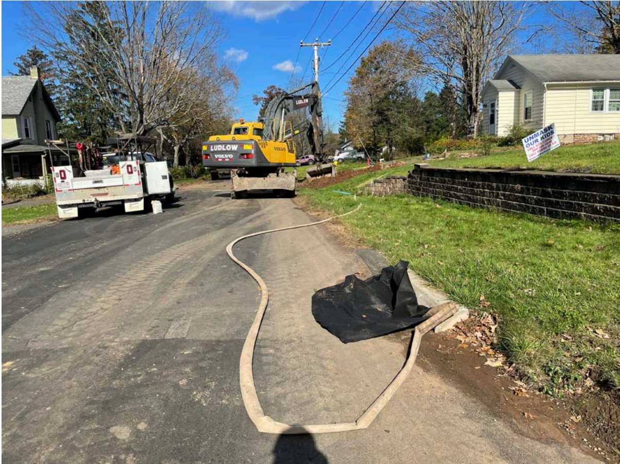
Picture 5: Ludlow set up to pump water out of the trench they excavated at the 175 Maple Avenue property for the installation of a 1" copper water service line. View to the north.
