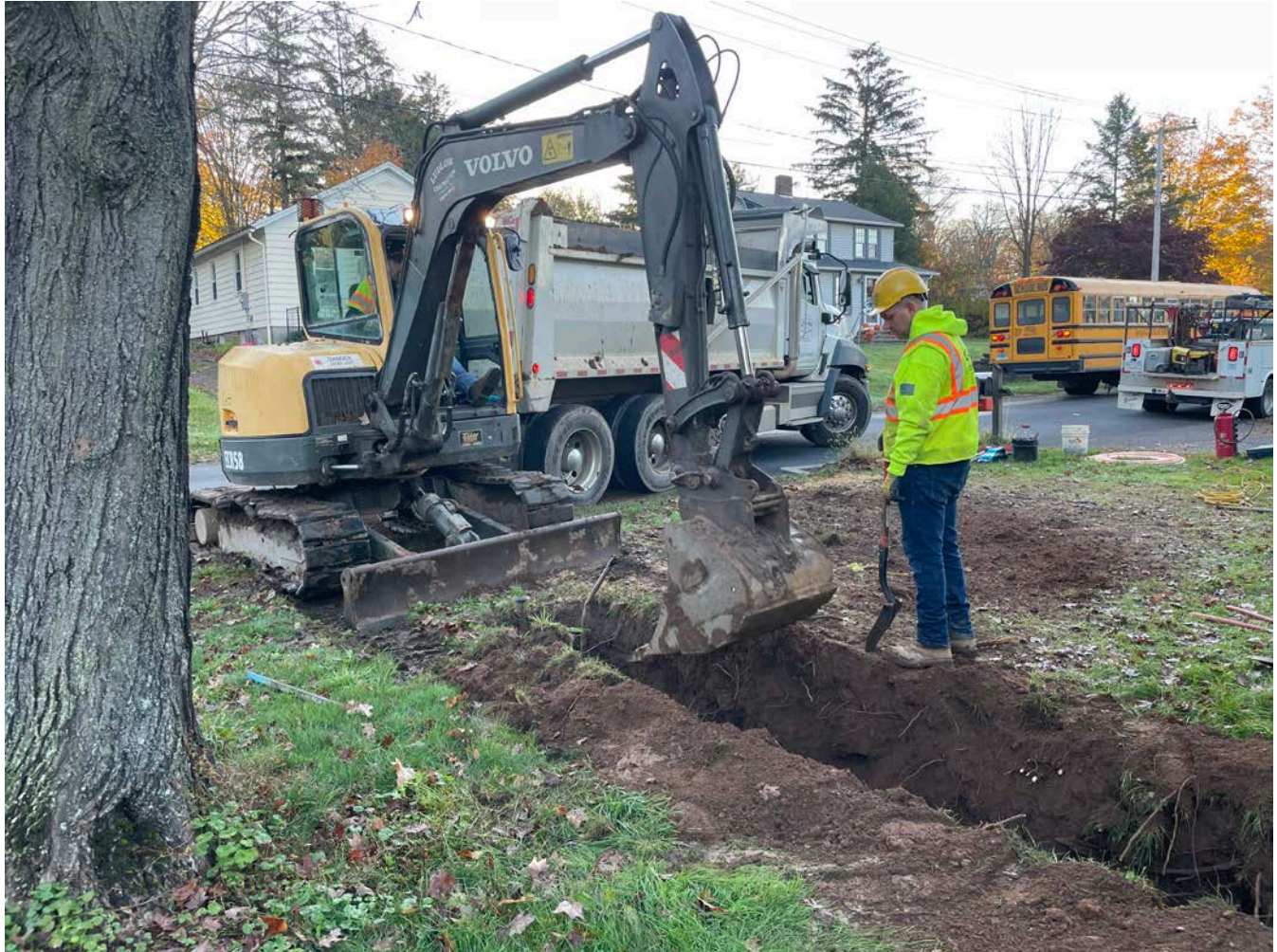
Picture 1: Ludlow excavating on the east side of the 176 Maple Avenue, Durham, residence for the installation of a 1" copper water service line. View to the southeast.
