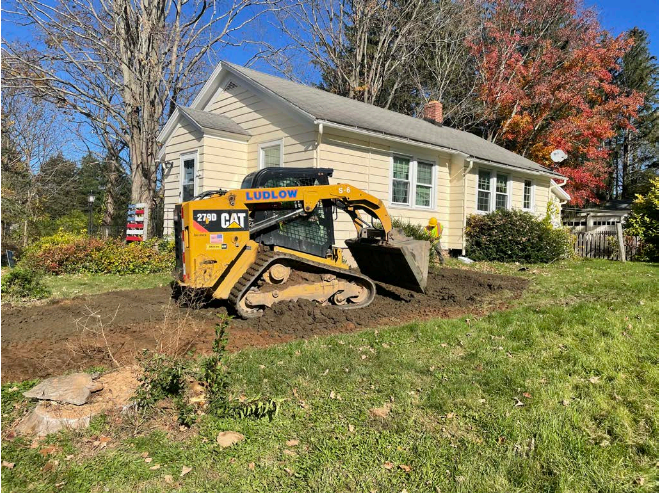
Picture 7: Ludlow grading loam as they restore the portions of the lawn at the 175 Maple Avenue residence that were disturbed during the installation of a 1" copper water service line. View to the northeast.
