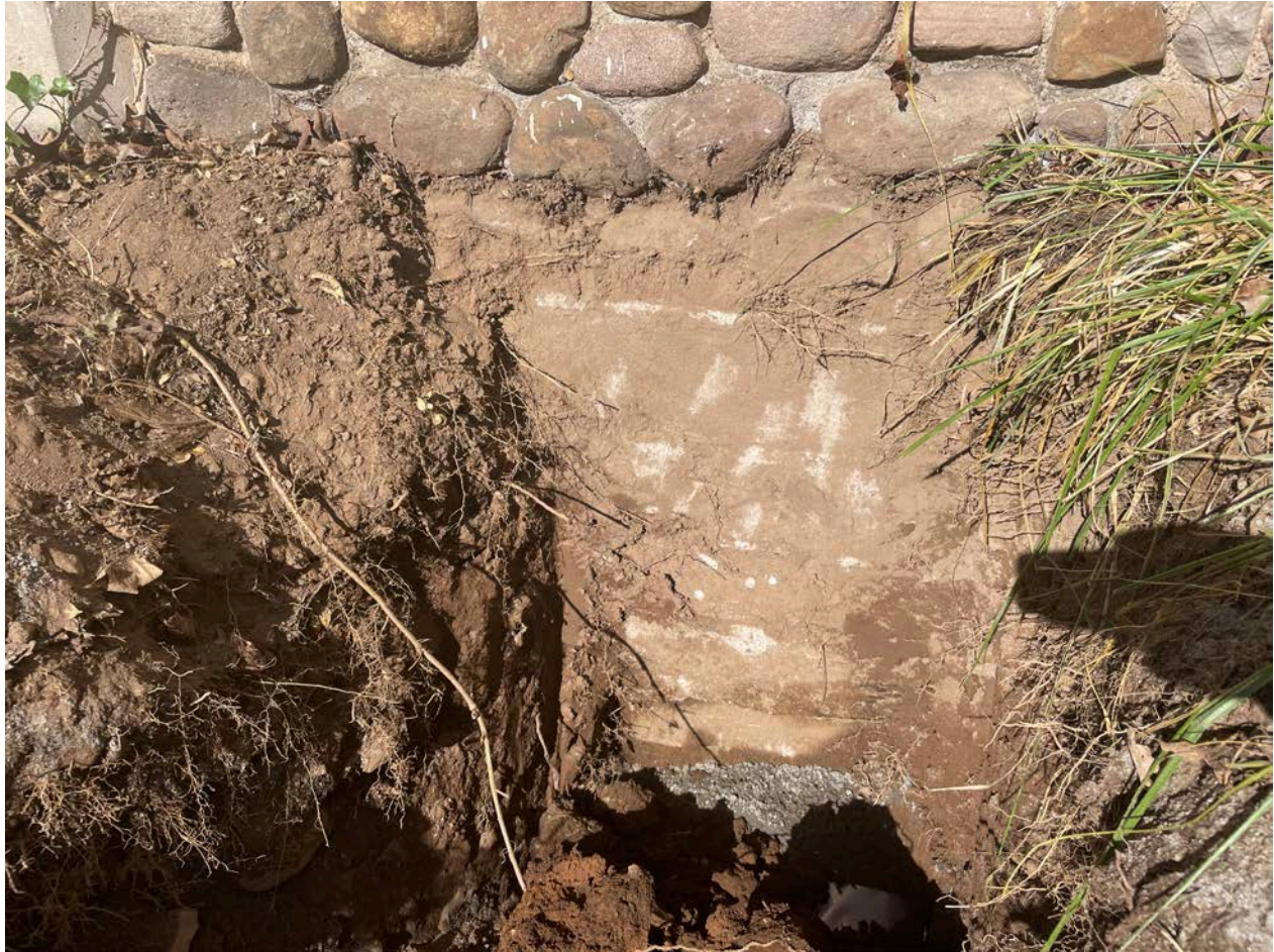
Picture 6: Concrete foundation on the south side of the 175 Maple Avenue residence that Ludlow has daylighted during the installation of a 1" copper water service line. View to the north.
