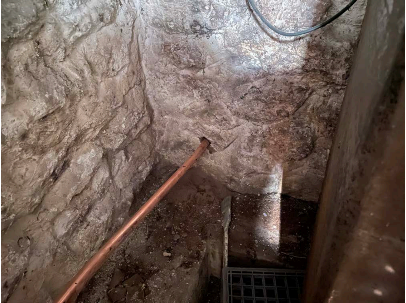
Picture 3: 1" copper water service line that Ludlow installed through the eastern foundation of the 176 Maple Avenue, Durham, residence. View to the northeast.
