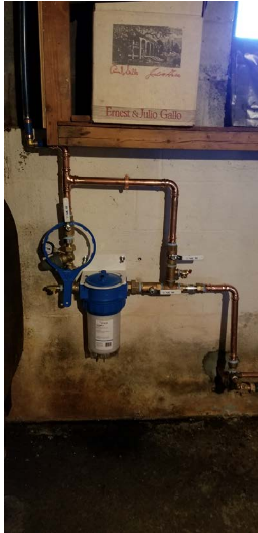
Picture 10: Final water service components that Fazzino Plumbing installed at the 202 Main Street, Durham, residence.
