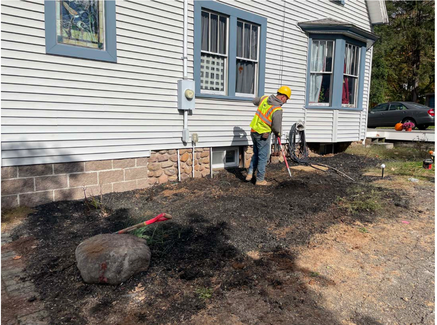
Picture 13: Ludlow raking out loam on a section of the garden on the south side of the 173 Maple Avenue residence that was disturbed by the installation of a 1" copper water service line. View to the east.
