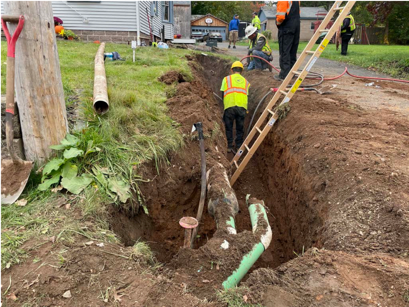
Picture 7: View of the trench that Ludlow is excavating on the north side of the driveway for the 173 Maple Avenue residence. View to the east.
