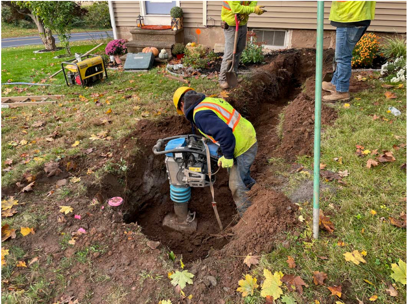
Picture 2: Ludlow compacting fill that was placed over caution tape and sand that was placed over the 1" copper water service line they installed on the east side of the 158 Maple Avenue residence. View to the southwest.
