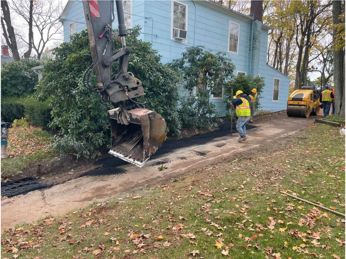
Picture 7: Ludlow placing asphalt on the trench footprint on the driveway of the 208 Main Street, Durham, property. View to the southwest.
