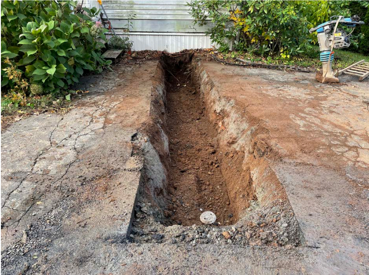
Picture 5: Trench that Ludlow excavated on the east side of the 162 Maple Avenue residence, prior to the placement and compaction of 1.25"-minus gravel. View to the west.
