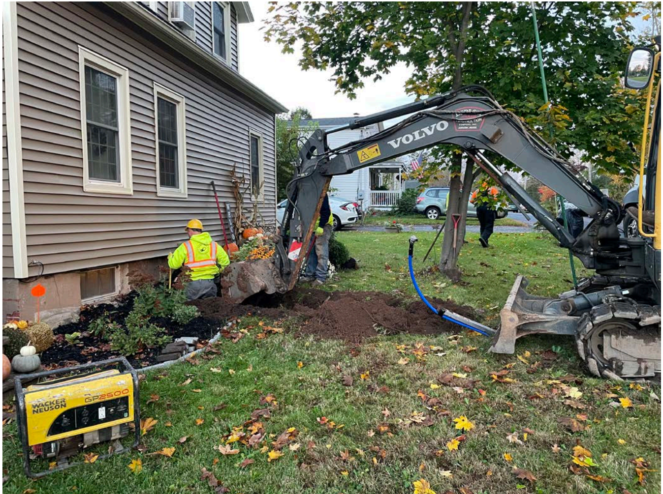
Picture 1: Ludlow excavating on the east side of the 158 Maple Avenue, Durham, residence for the installation of a 1" copper water service line. View to the north.
