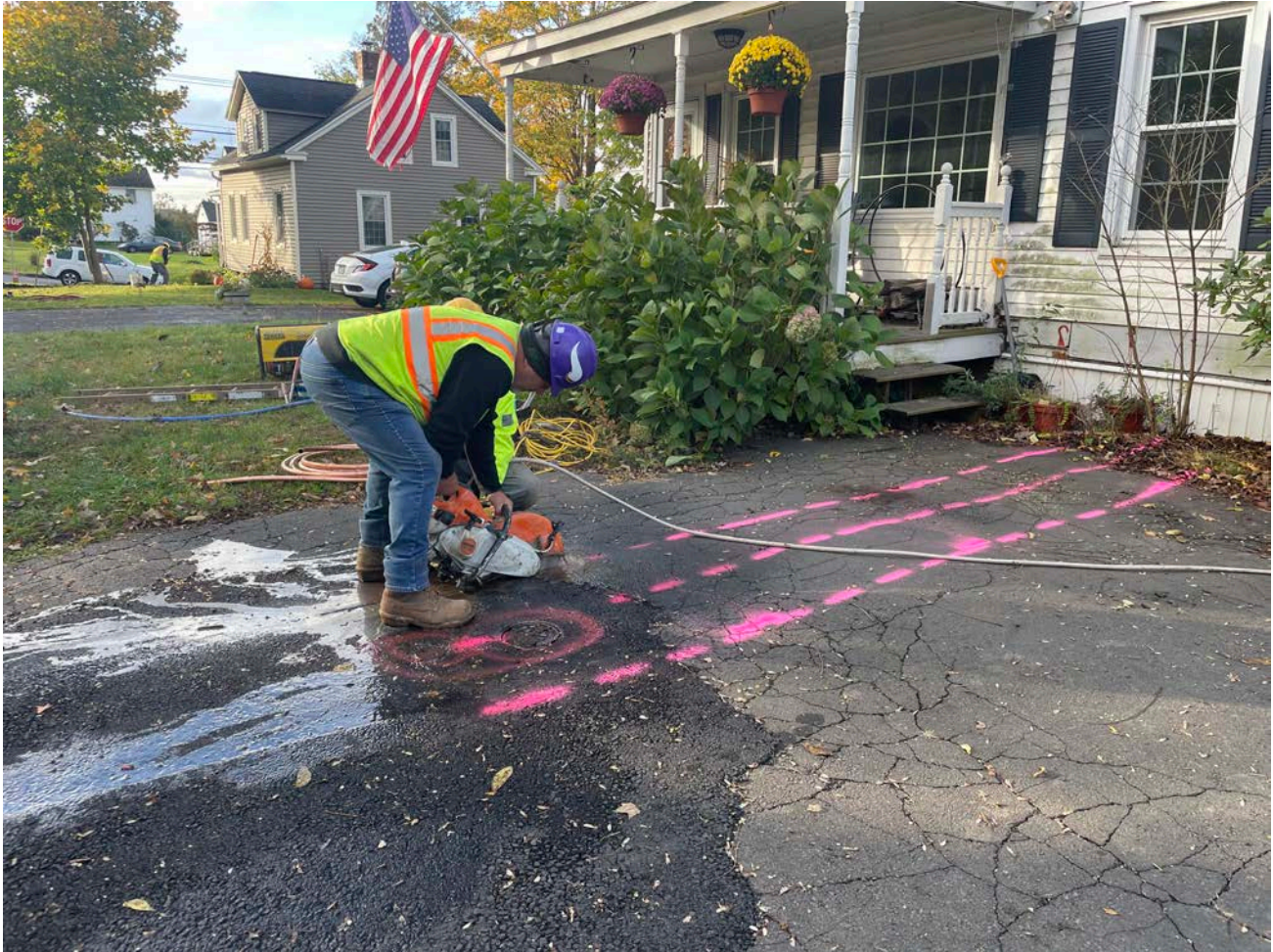
Picture 3: Ludlow saw cutting a footprint for the trench they will excavate on the asphalt driveway of the 162 Maple Avenue, Durham, residence for the installation of a 1" copper water service line. View to the southwest.
