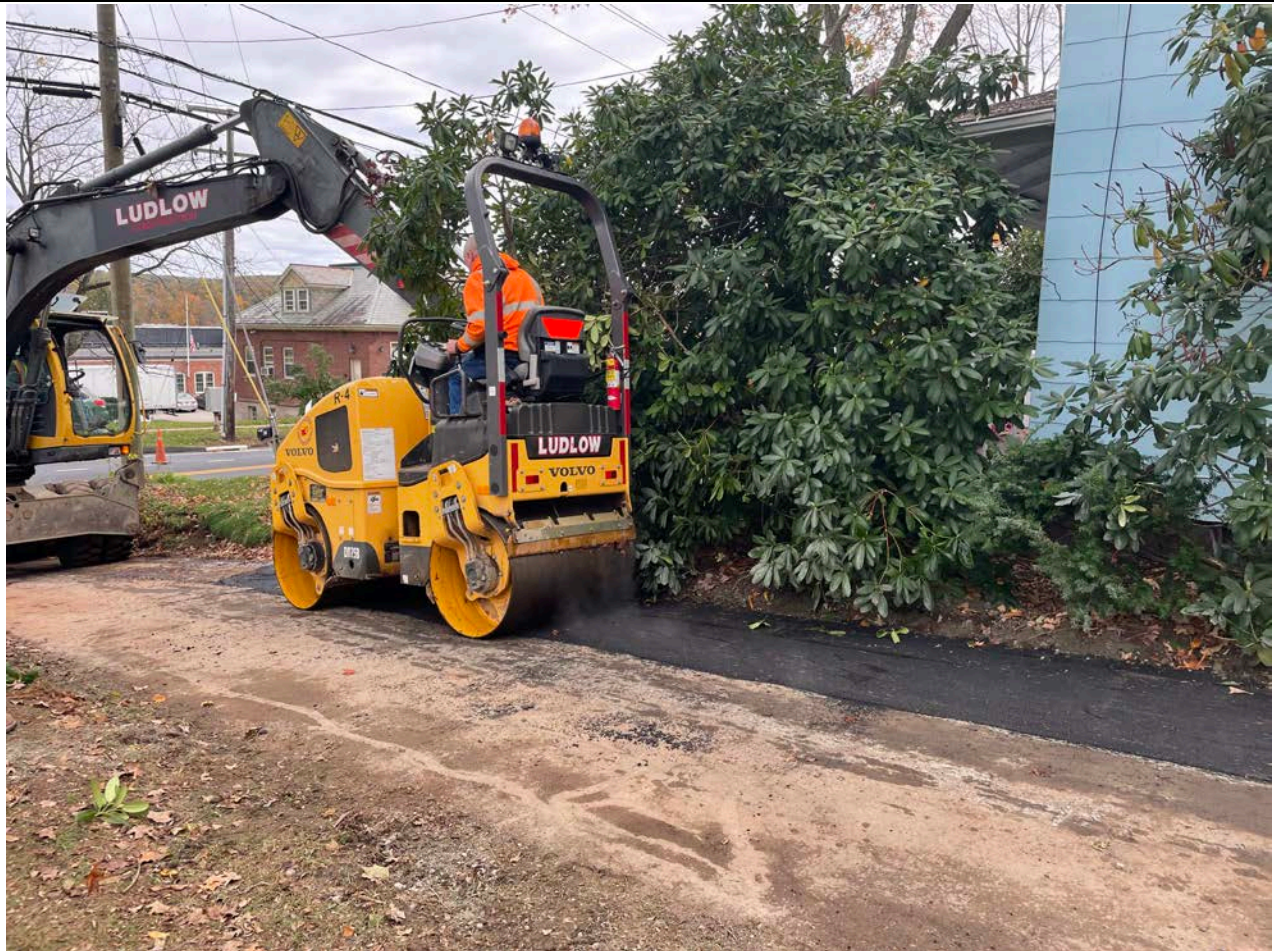
Picture 8: Ludlow compacting asphalt that they just placed on the trench footprint on the driveway of the 208 Main Street, Durham, property. View to the southeast.
