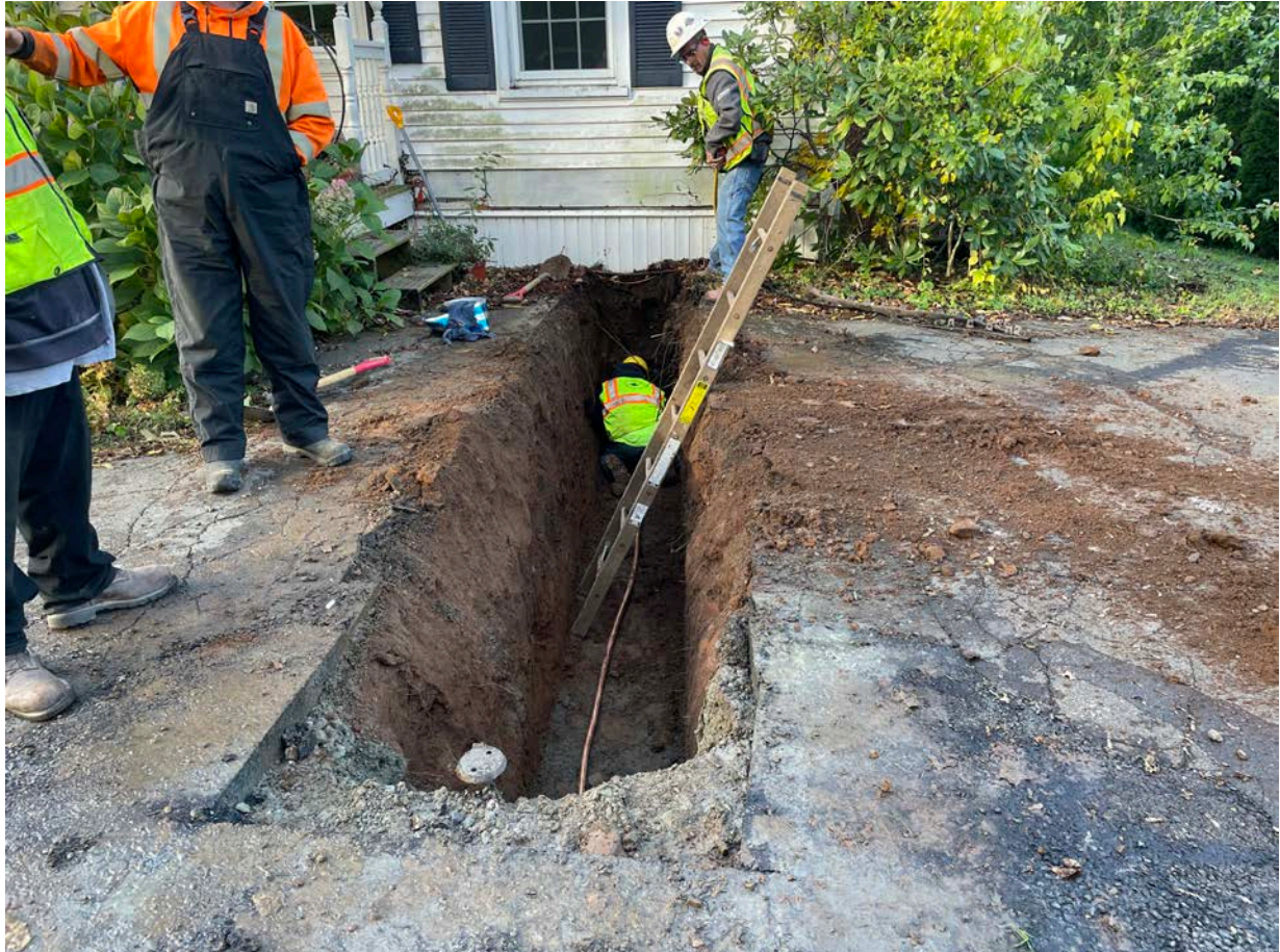
Picture 4: Ludlow placing a 1" copper water service line in the trench they excavated on the east side of the 162 Maple Avenue residence. View to the west.
