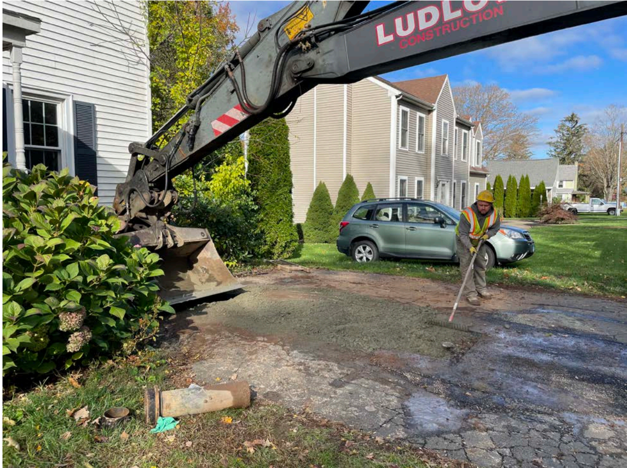
Picture 6: Ludlow grading 1.25"-minus gravel in the trench that Ludlow excavated on the east side of the 162 Maple Avenue residence. View to the north.
