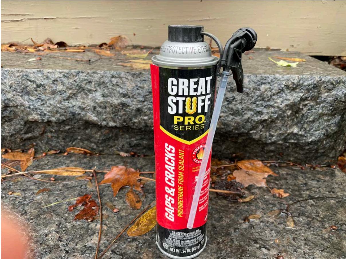
Picture 5: Polyurethane foam sealant that Ludlow used as a seal between the 4" PVC sewer pipe and the 1" copper water service line they are installing on the east side of the 202 Main Street residence.
