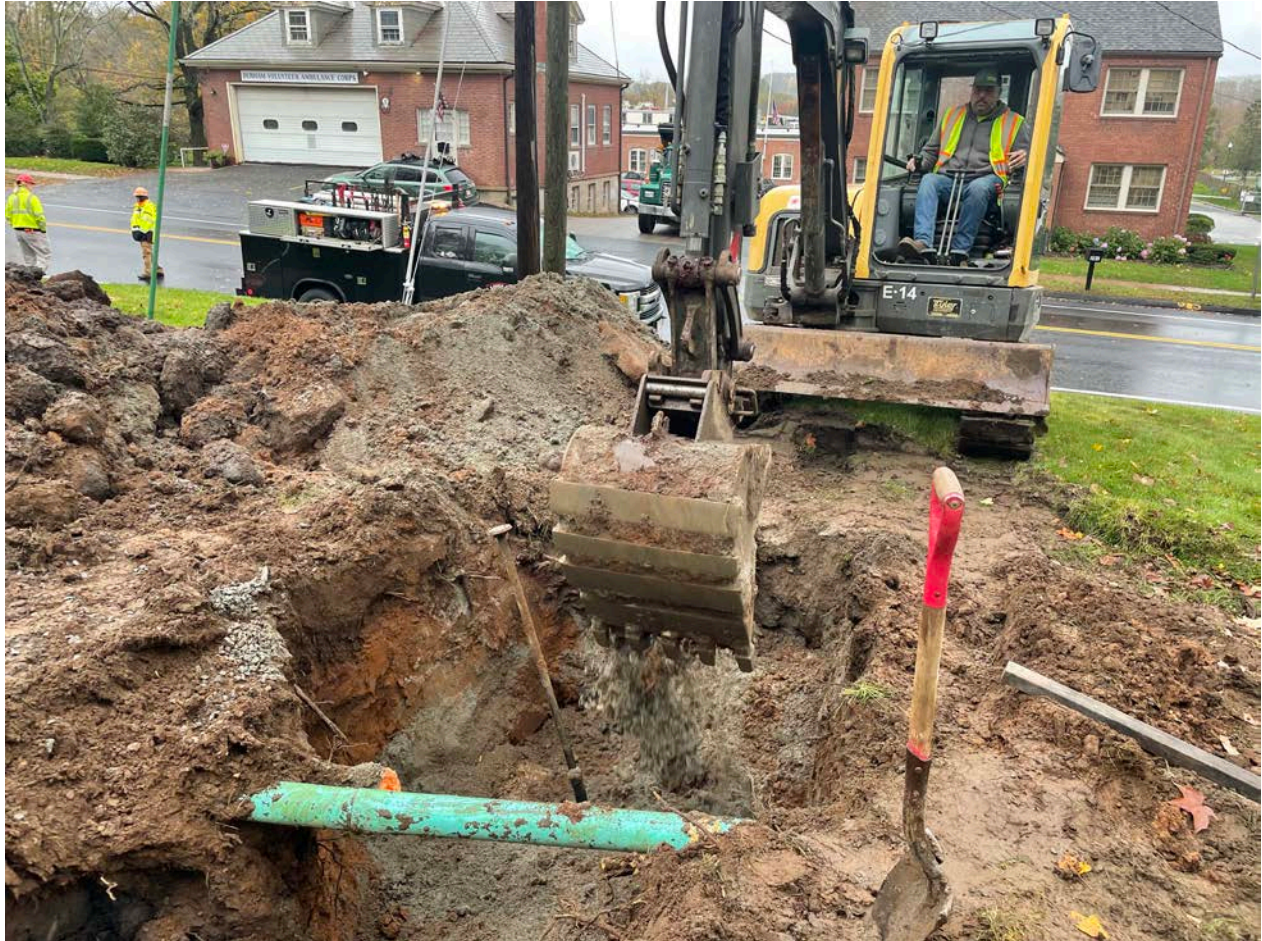
Picture 6: Ludlow placing sand over the 4" PVC sewer pipe that was placed as a sleeve over the 1" copper water service line they installed on the east side of the 202 Main Street residence. View to the west.
