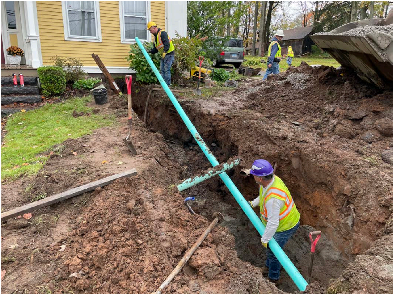
Picture 2: Ludlow placing 4" PVC sewer pipe over the 1" copper water service line they are installing on the east side of the 202 Main Street residence. View to the west.
