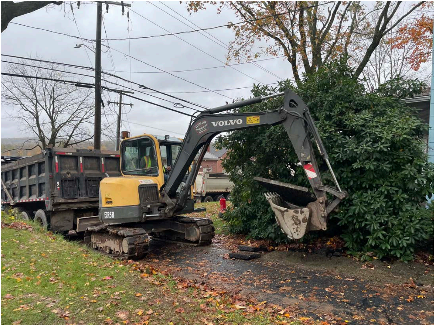
Picture 9: Ludlow removing asphalt from the driveway of the 208 Main Street residence as part of the installation of a 1" copper water service line. View to the southeast.
