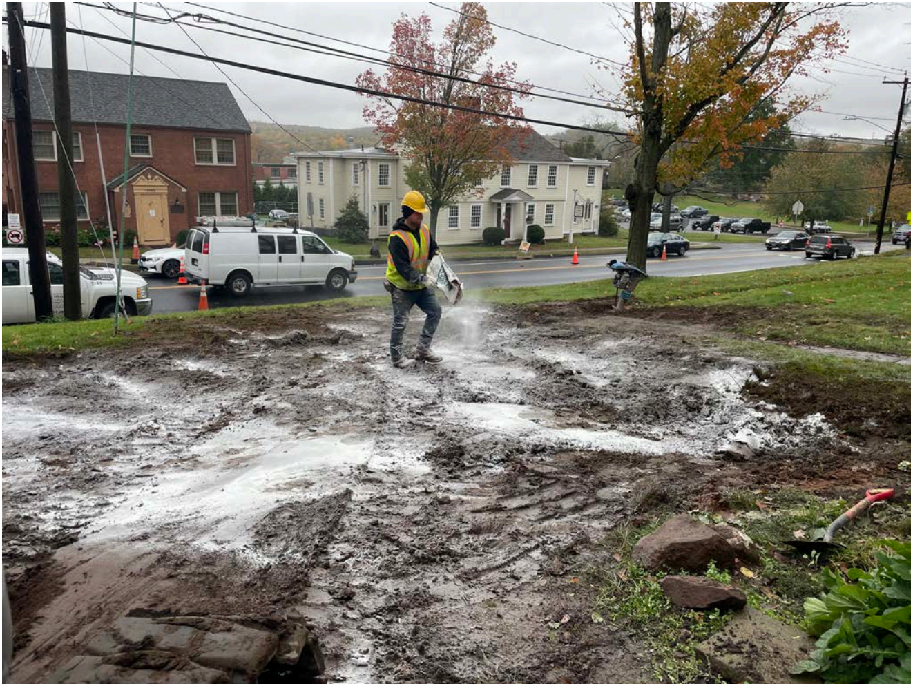
Picture 7: Ludlow is spreading lime on top of the fill they used to backfill the trench and to repair the sections of the lawn that were disturbed during the installation of a 1" copper water service line at the 202 Main Street property. View to the southeast.
