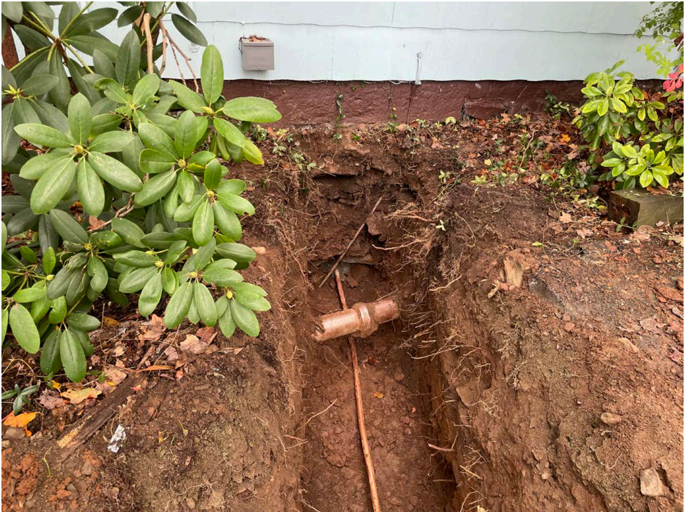
Picture 10: 1" copper water service line that Ludlow has inserted through the northern foundation of the 208 Main Street residence. View to the south.
