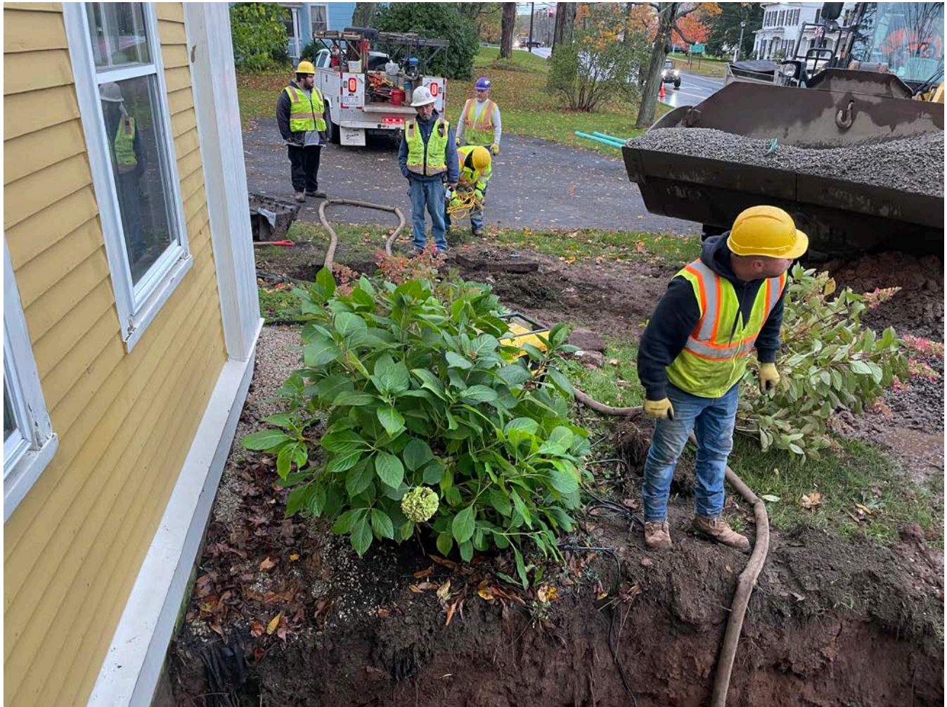
Picture 1: Ludlow pumping water from the excavation they made on the east side of the 202 Main Street, Durham, residence into the septic tank located on the northeast corner of the house. View to the north.
