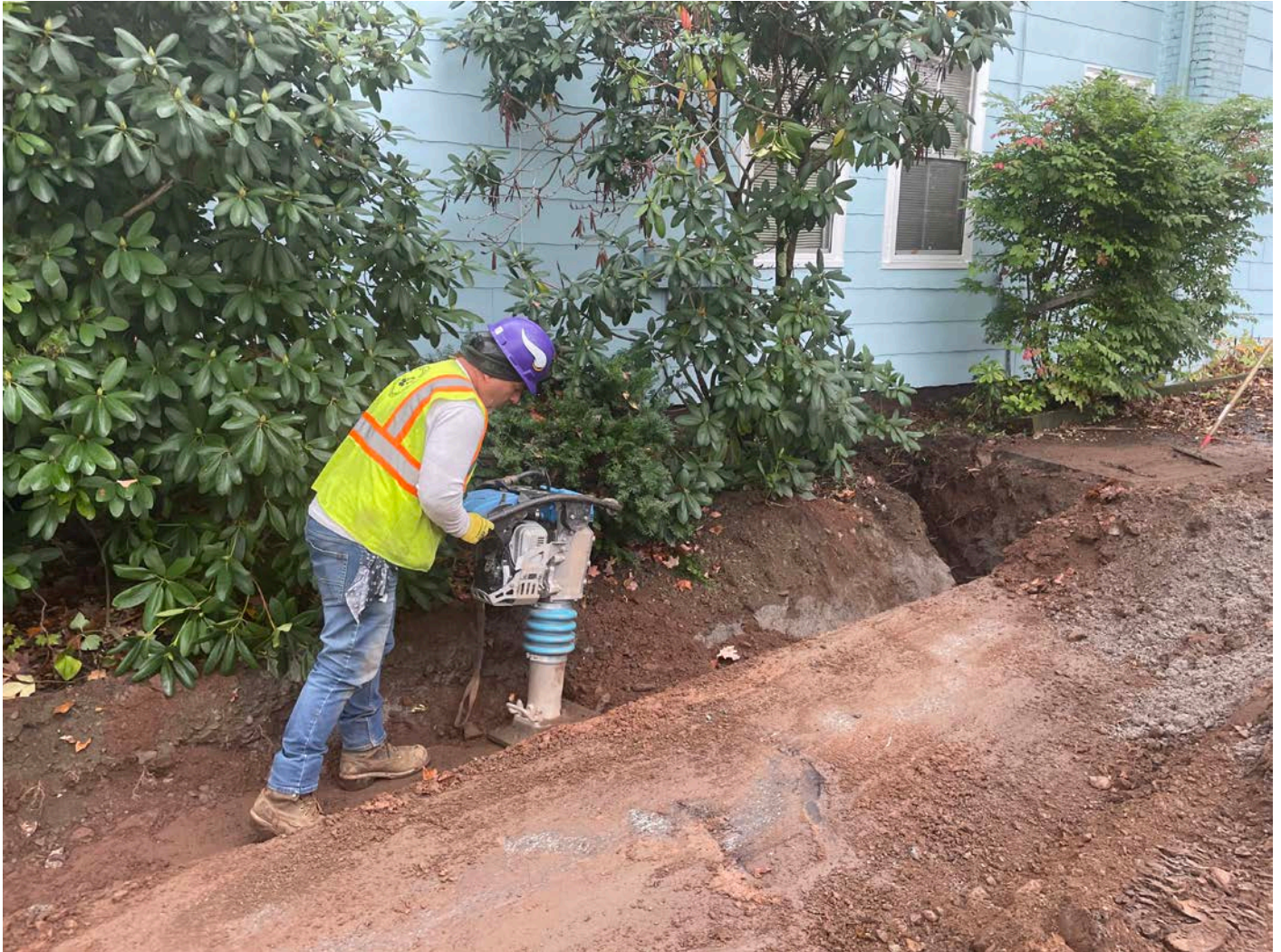
Picture 11: Ludlow compacting fill over sand and caution tape that was placed over the 1" copper water service line they installed at the 208 Main Street residence. View to the southwest.
