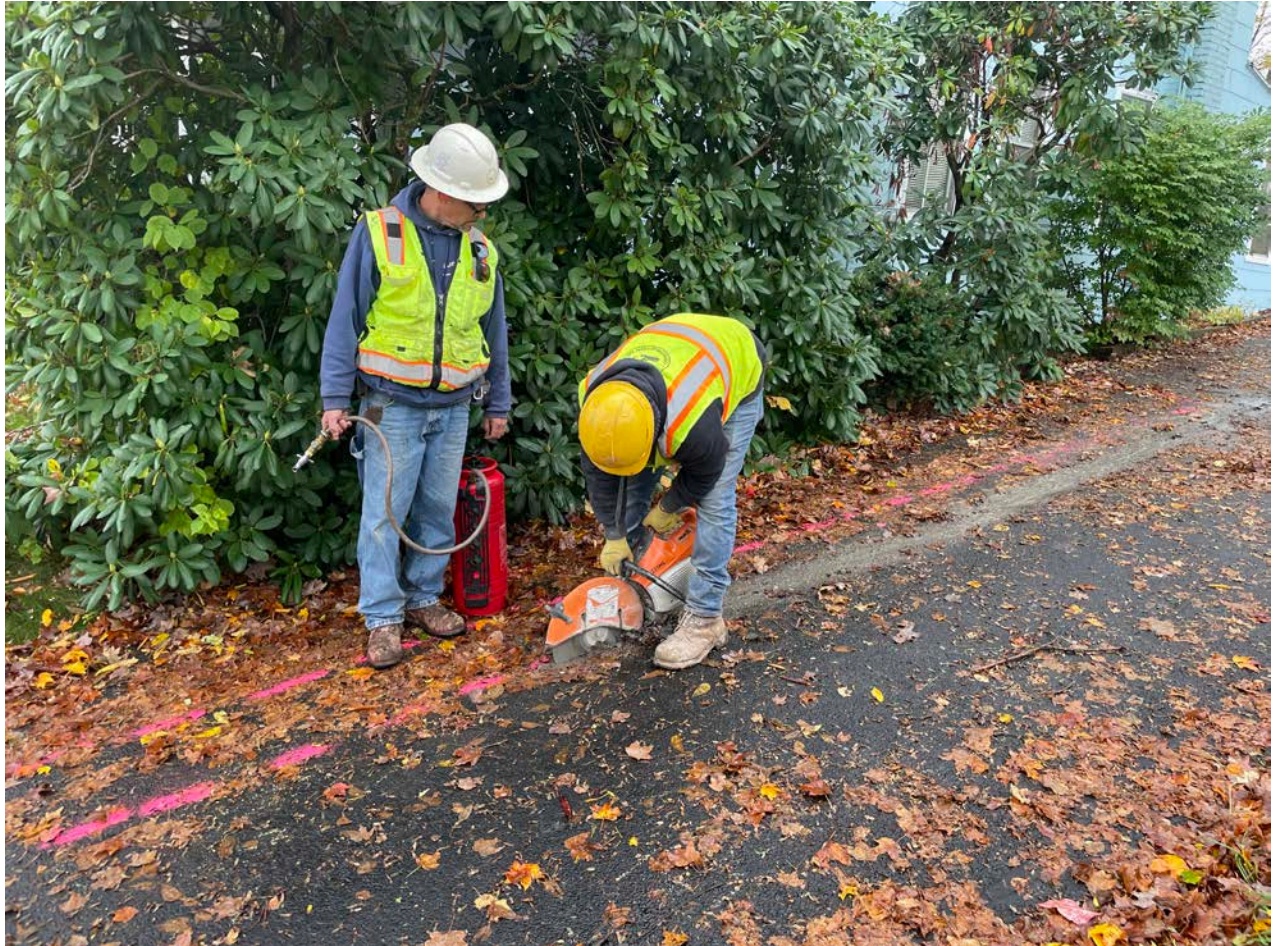
Picture 8: Ludlow saw cutting a footprint for the trench they will excavate on the asphalt driveway of the 208 Main street residence for the installation of a 1" copper water service line. View to the southwest.
