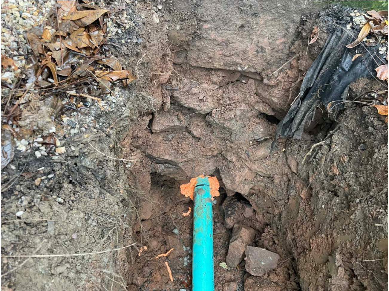
Picture 3: 4" PVC sewer pipe that Ludlow placed over the 1" copper water service line they are installing on the east side of the 202 Main Street residence. Ludlow has placed polyurethane foam sealant between the 4" PVC and the 1" copper line. View to the west.
