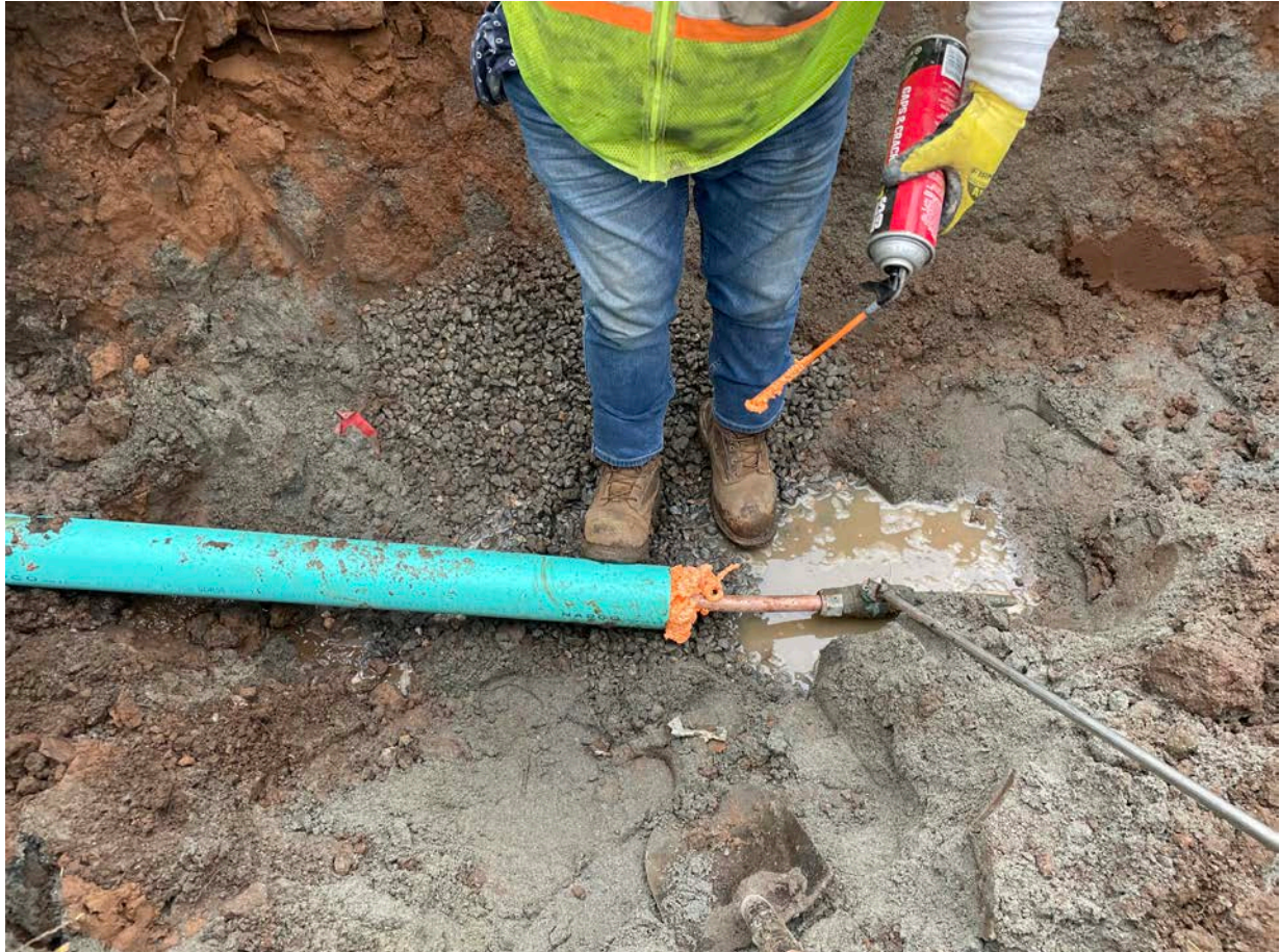
Picture 4: Ludlow has just placed polyurethane foam sealant between the 4" PVC and the 1" copper water service line they are installing on the east side of the 202 Main Street residence. View is of the east side of the 1" copper water line where it connects to the curb stop for the 202 Main Street property. View to the north.
