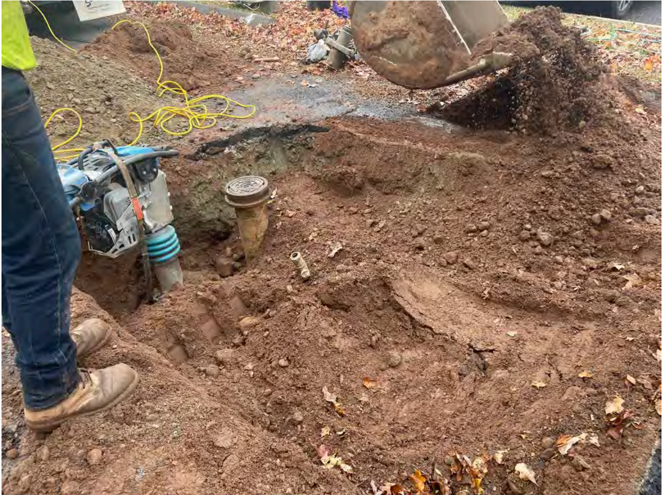
Picture 7: Ludlow backfilling over the corp stop that Ludlow just installed at Station 503+91. The road box for the valve stem located at Station 503+93 can be seen ~1' to the northwest of the 1" copper line that Ludlow installed up to surface grade that they attached to the corp stop at 503+91. View to the northwest.
