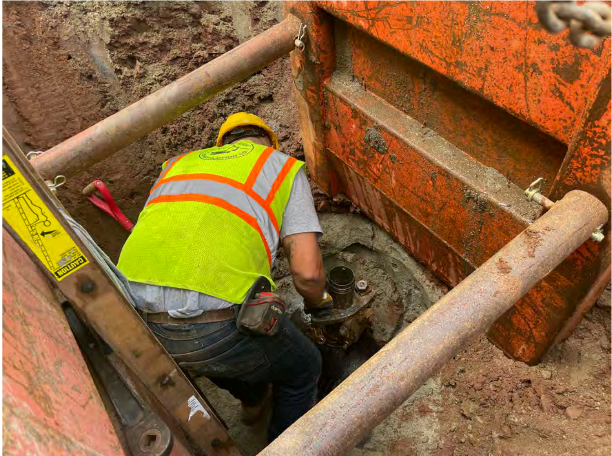
Picture 6: Ludlow removing tapping mechanism after having tapped the 12" DIP water line at Station 503+91 on Pickett Lane. View to the northwest.
