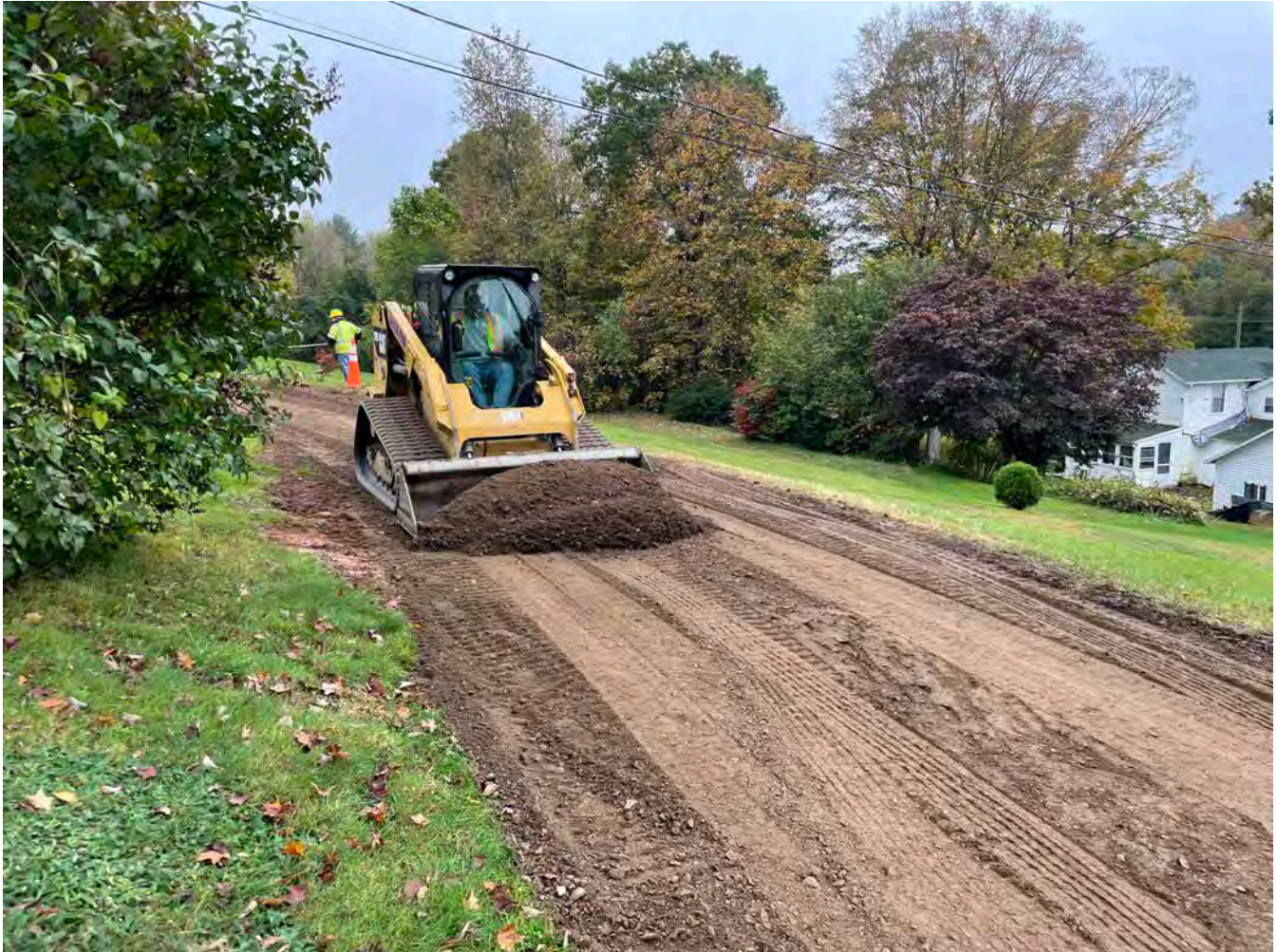
Picture 1: Ludlow grading gravel that was replaced on the driveway of the 175 Main Street, Durham, property. View to the southwest.
