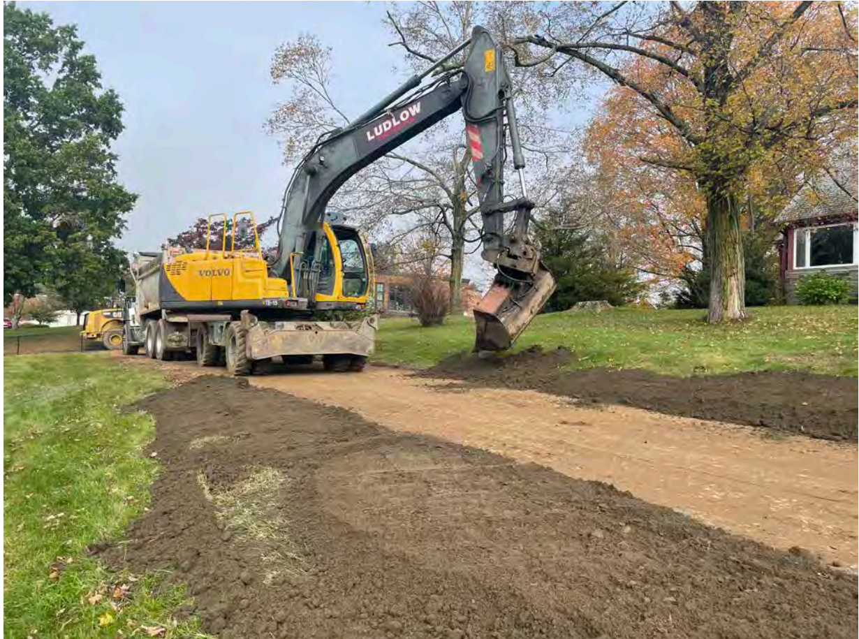
Picture 4: Ludlow placing loam along the edges of the driveway at the 175 Main Street property. View to the north.
