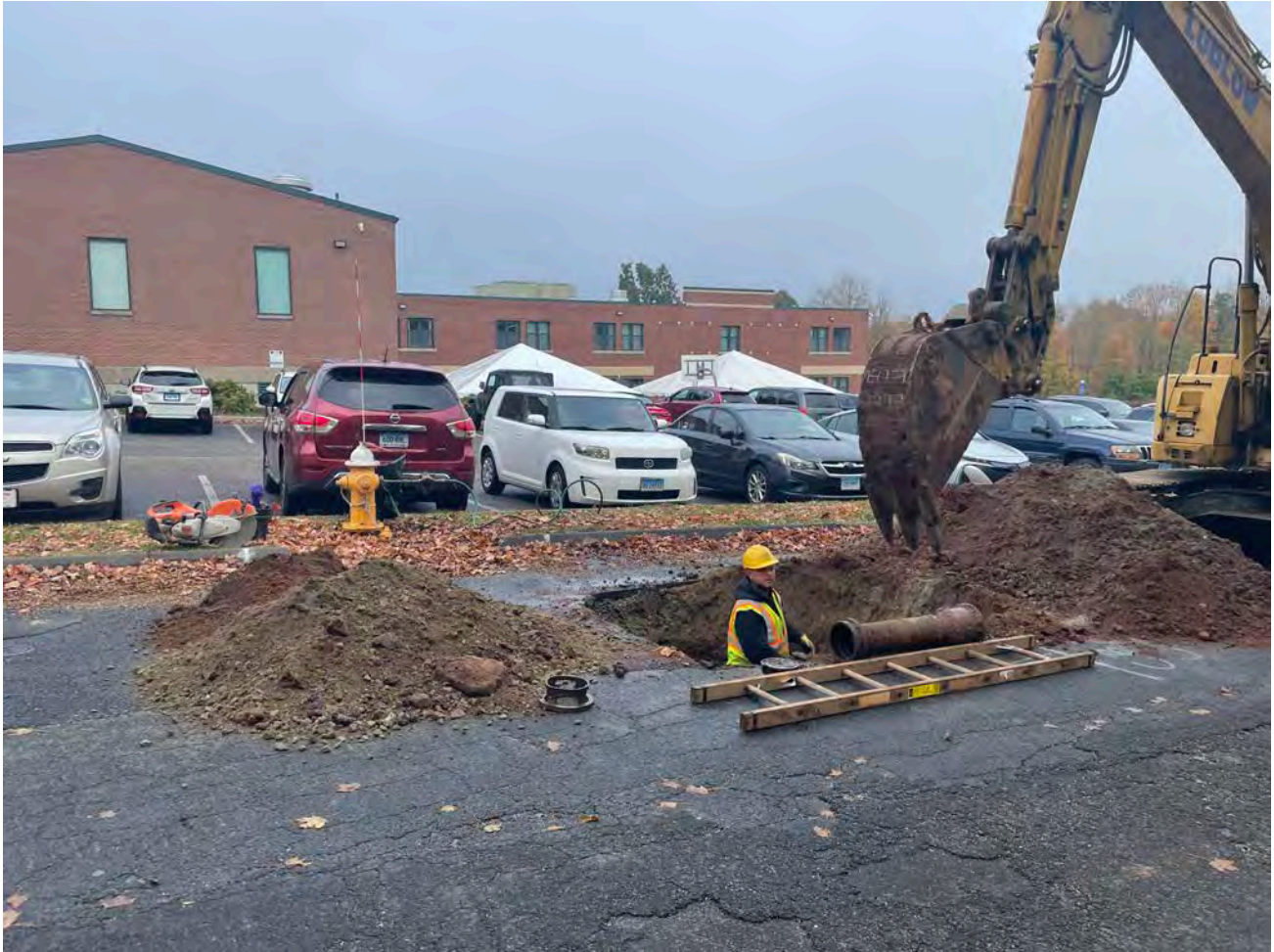
Picture 3: Ludlow excavating at Station 503+91 on Pickett Lane to install a chlorinator/dechlorinator injection port on the 12" DIP water line they installed last year. View to the northeast.
