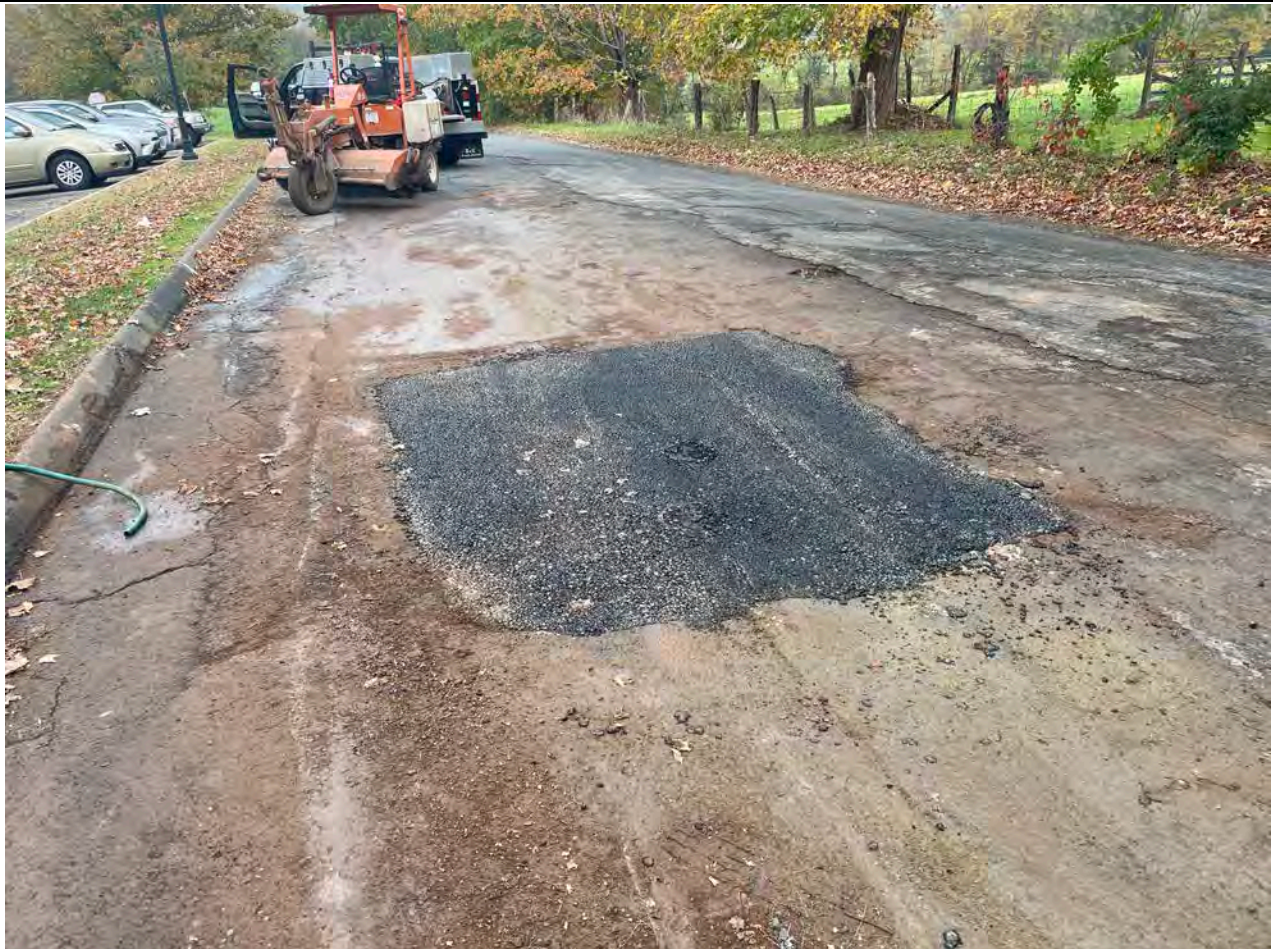
Picture 8: Asphalt patch that Ludlow placed over the backfilled excavation at Station 503+91 on Pickett Lane, Durham. View to the east.
