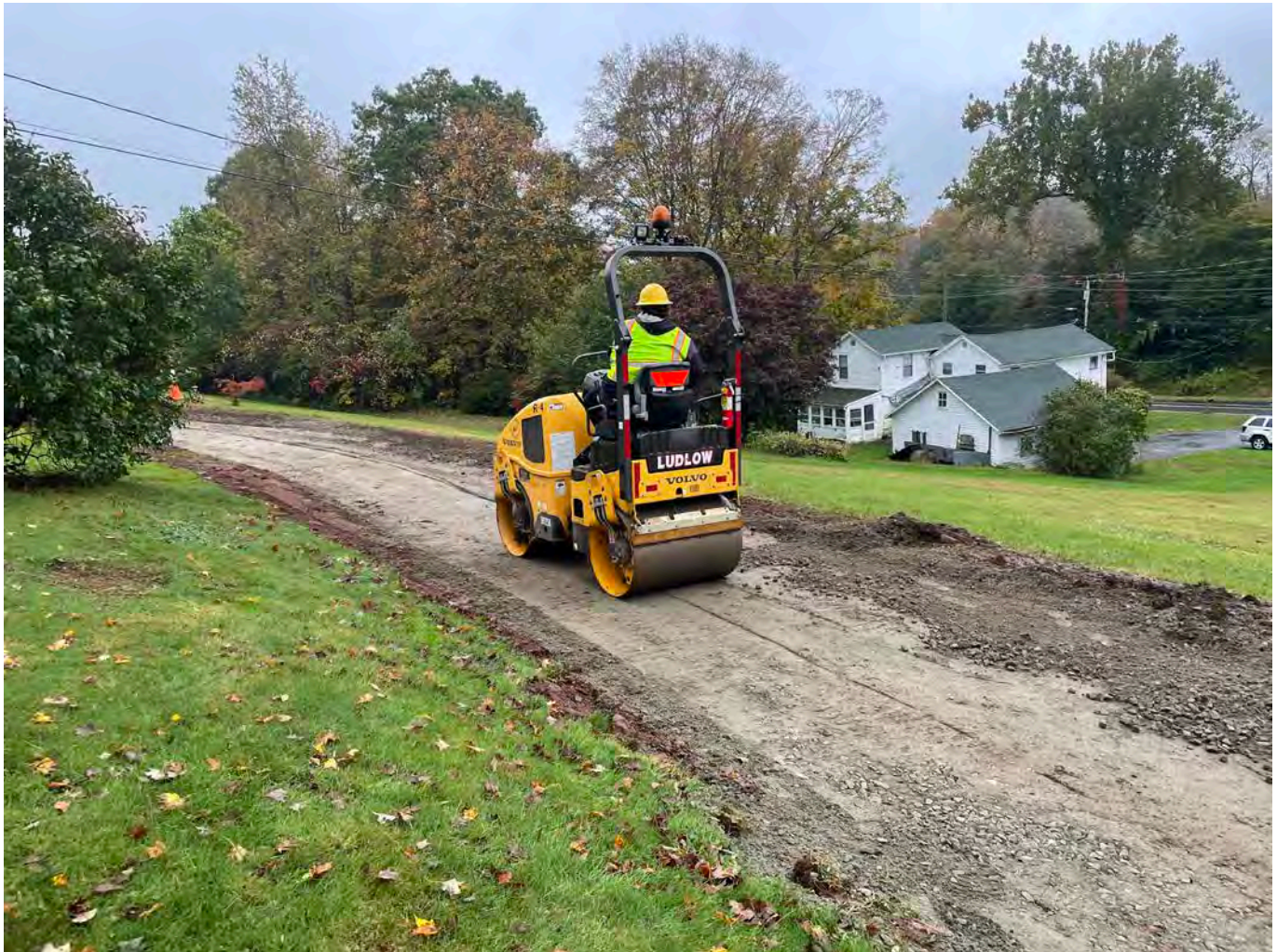
Picture 2: Ludlow compacting gravel that was replaced on the driveway of the 175 Main Street, Durham, property. View to the southwest.
