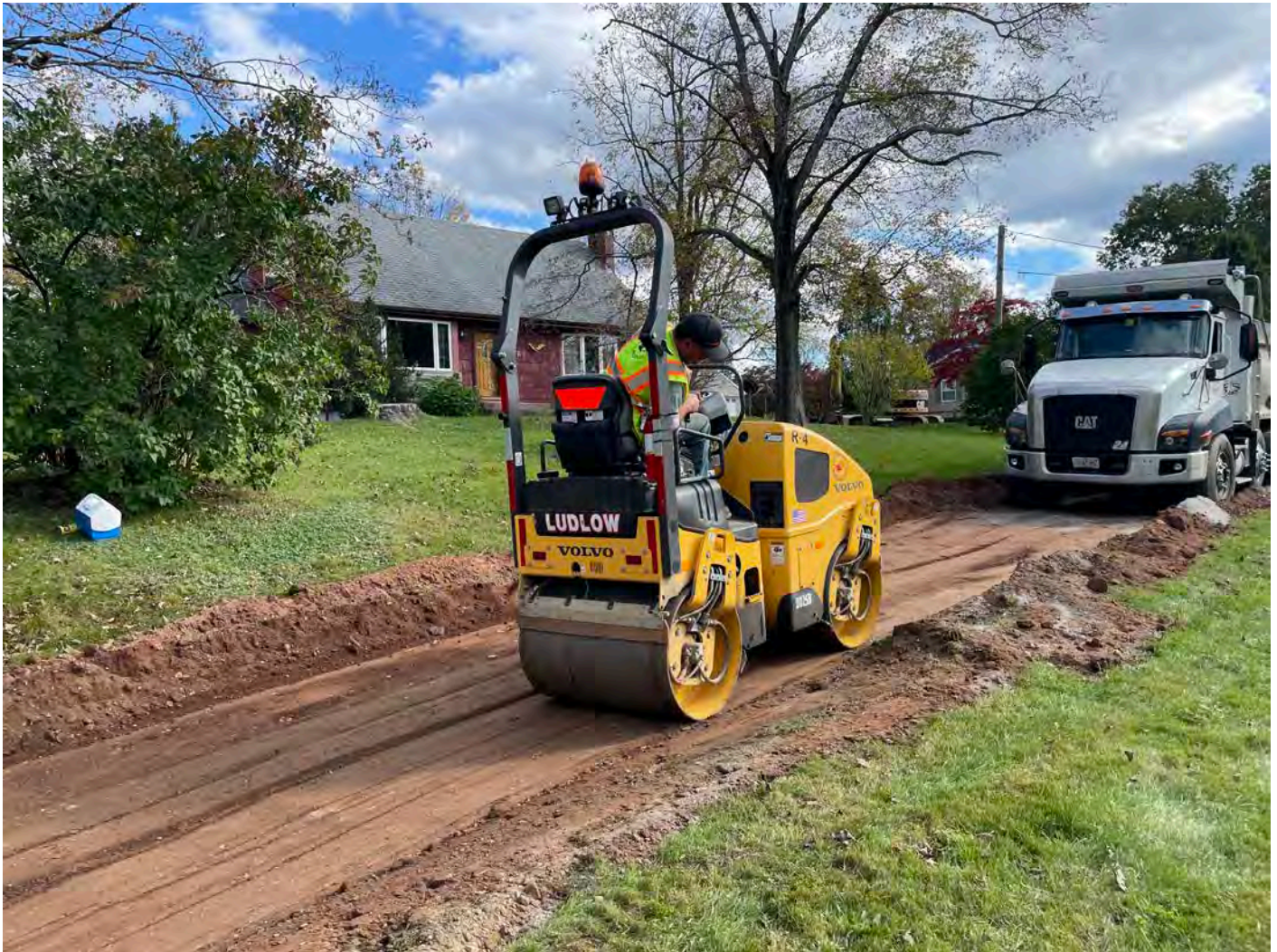
Picture 12: Ludlow compacting gravel they replaced on the driveway for the 175 Main Street property. View to southeast.
