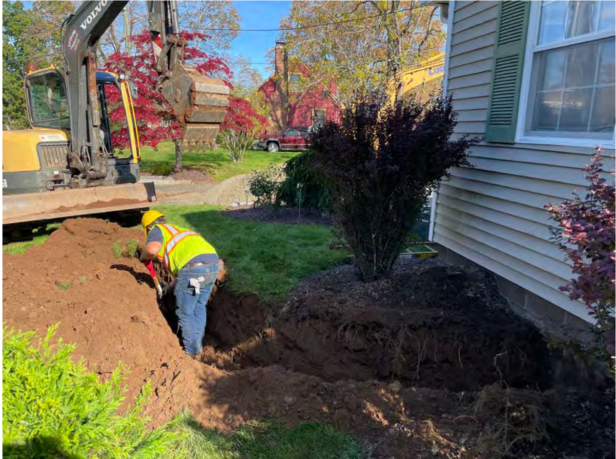
Picture 6: Ludlow excavating a trench northward for the installation of a 1.5" copper water service line at the 175 Main Street property. View to the north.
