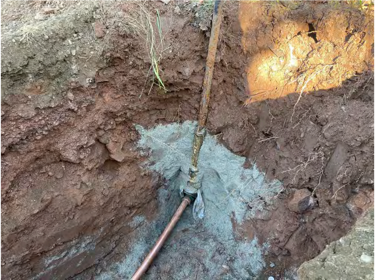
Picture 3: Curb stop that Ludlow installed at the 175 Main Street property, with 1.5" copper pipe installed on the south side of the curb stop. View to the northwest.
