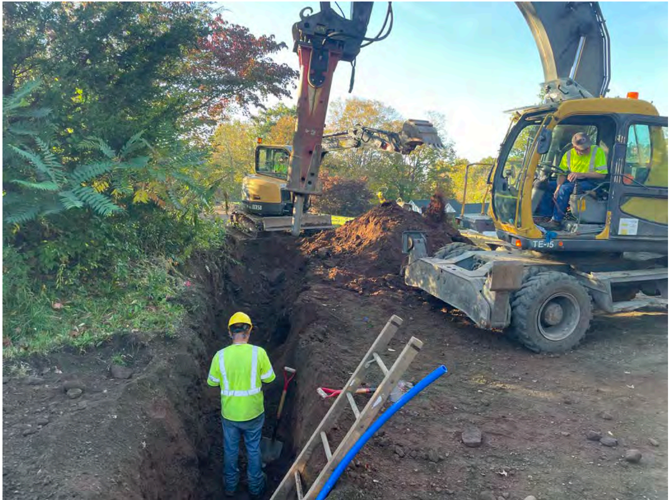
Picture 1: Ludlow preparing to hammer rock they encountered while excavating a trench for the installation of a 1.5" copper water service line at the 175 Main Street, Durham, property. View to the south.
