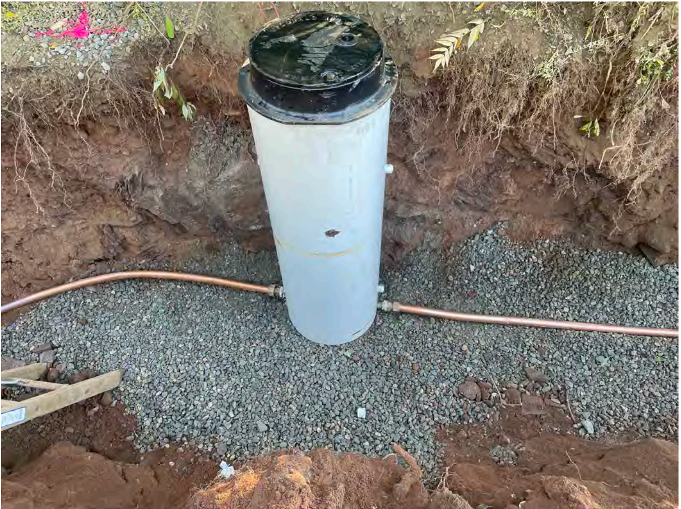
Picture 2: Meter pit that Ludlow installed at the 175 Main Street property, with 1.5" copper pipe installed on the north and south sides of the PVC riser. View to the east.
