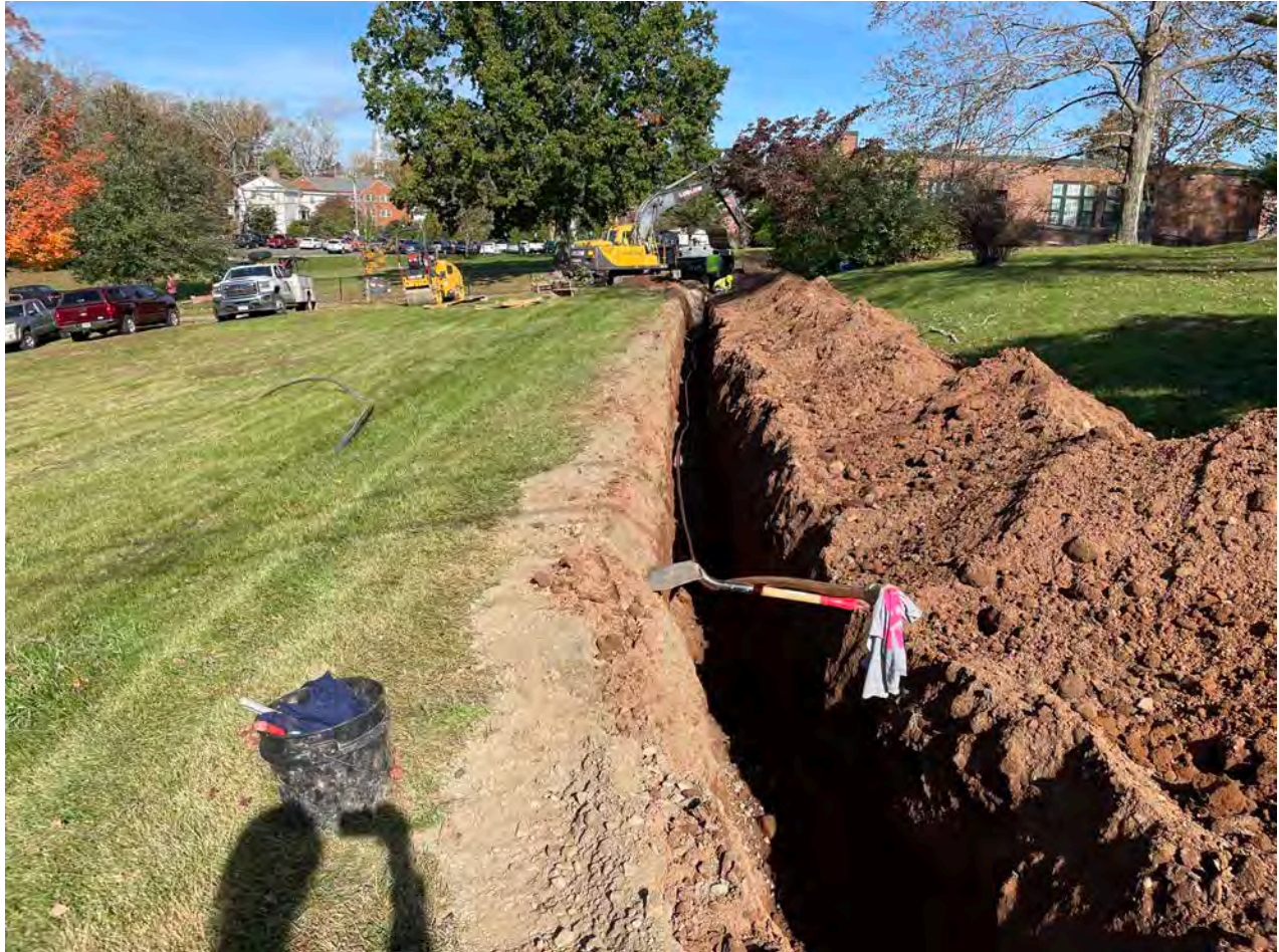
Picture 8: Ludlow in the process of installing a 1.5" copper water service line for the 175 Main Street residence. View to the north.
