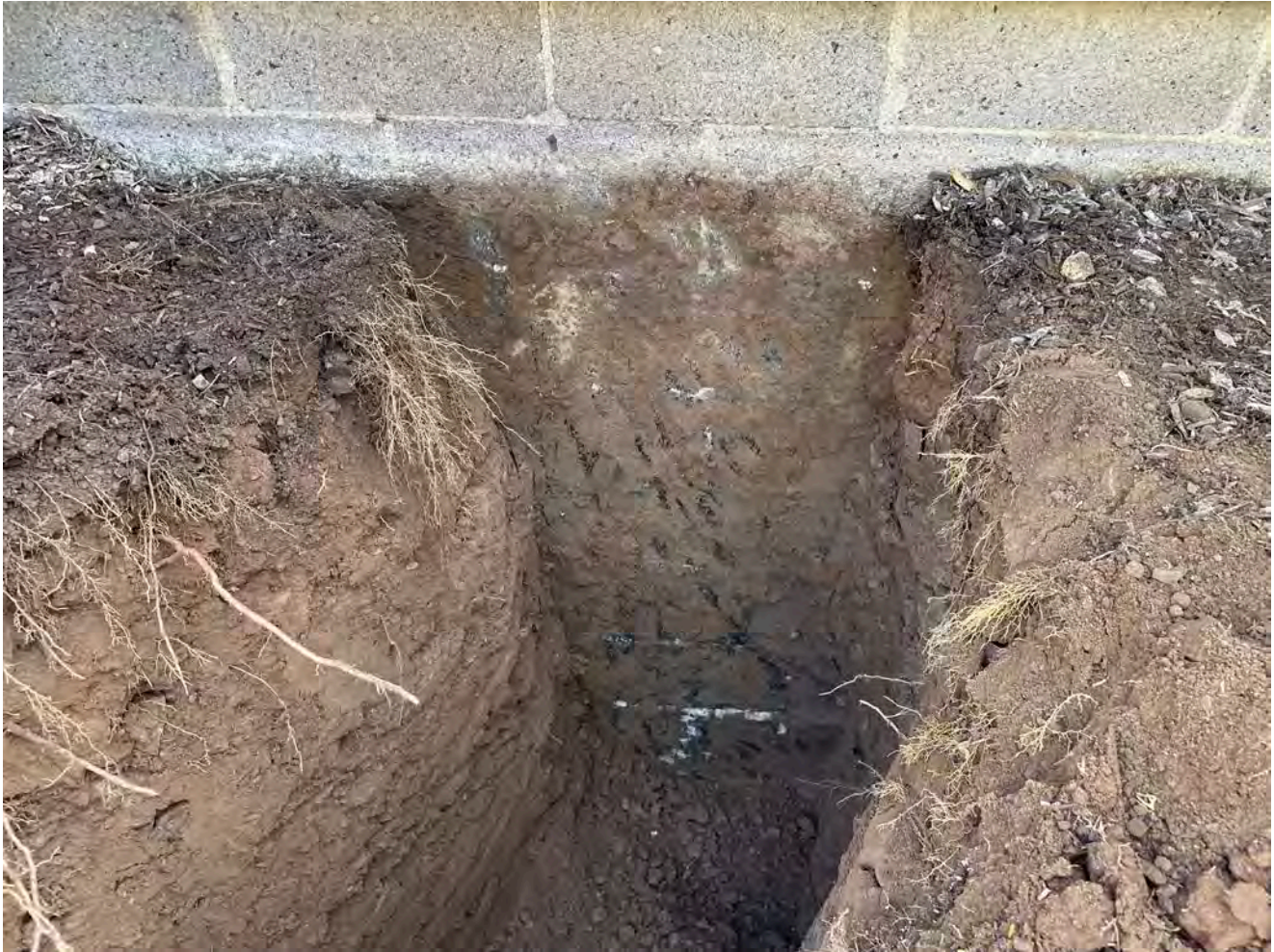
Picture 7: Cinder block foundation of the 175 Main Street residence that Ludlow daylighted on the west side of the house. View to the east.
