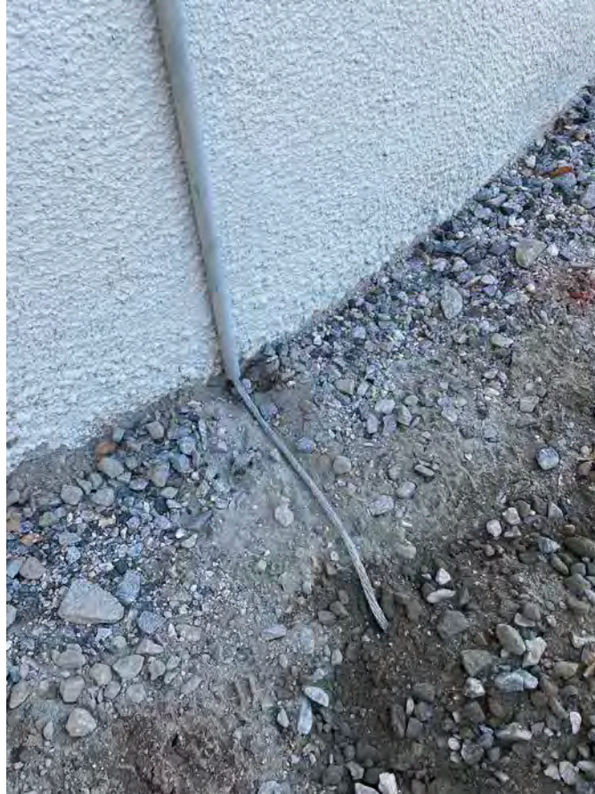
Picture 5: Grounding wire that B&B Lightning Protection installed on the side of the water tank and tied into the existing subsurface grounding wires around the perimeter of the tank. Water tank work zone located east of the Shared Access Driveway. View to south.
