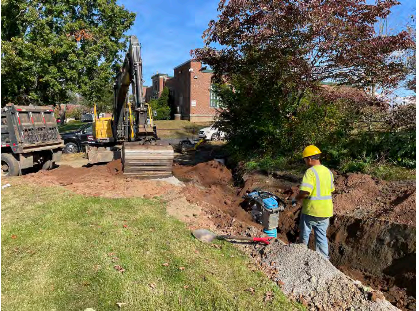
Picture 10: Ludlow compacting fill with a jumping jack they just placed over sand and caution tape as they backfill the trench where they installed a 1.5" copper water service line at the 175 Main Street property. View to northeast.
