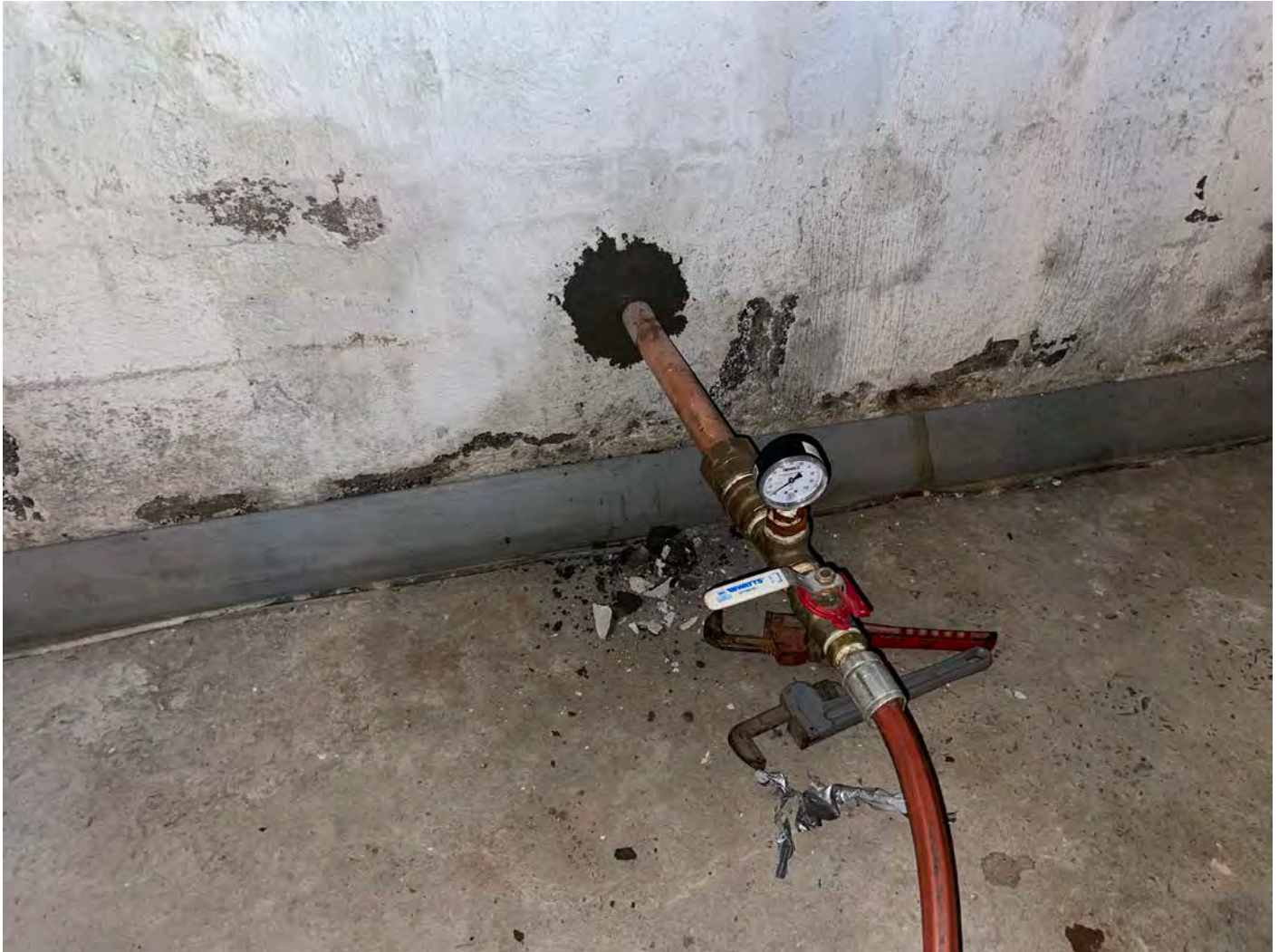
Picture 11: Pressure gauge that Ludlow placed on the 1.5" copper water service line they installed through the western foundation of the 175 Main Street residence. View to northwest.
