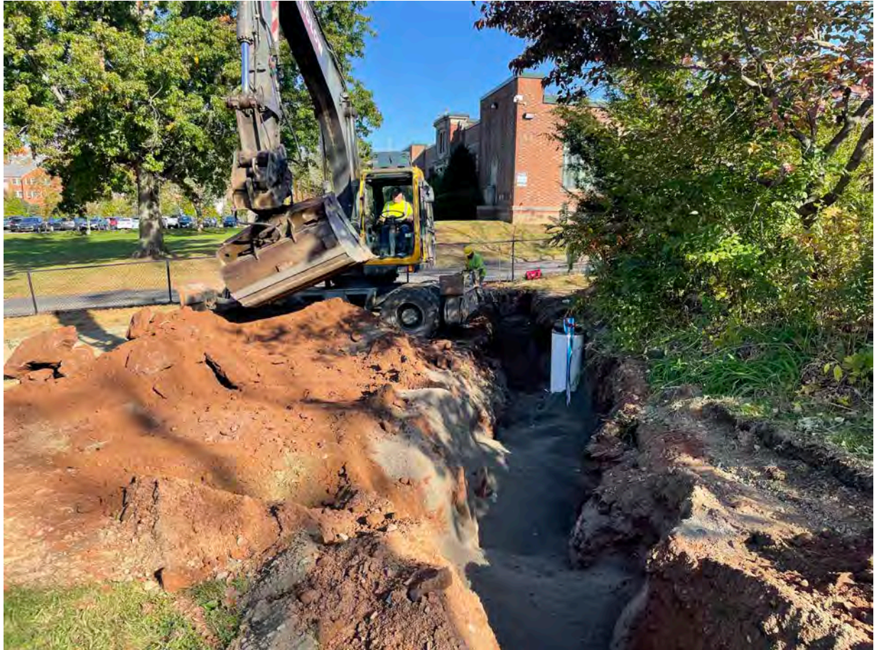
Picture 4: Ludlow backfilling over the 1.5” copper pipe they installed at the 175 Main Street property. View to the north.
