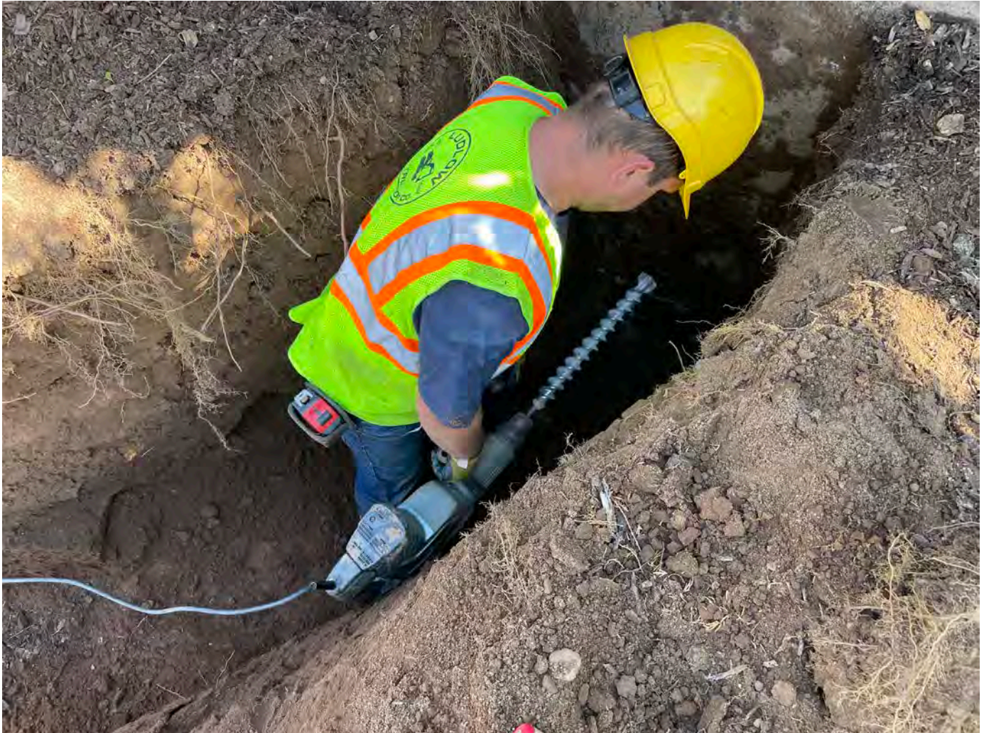
Picture 9: Ludlow preparing to penetrate the cinder block foundation of the residence located at 175 Main Street for the installation of a 1.5" copper water service line. View to northeast.
