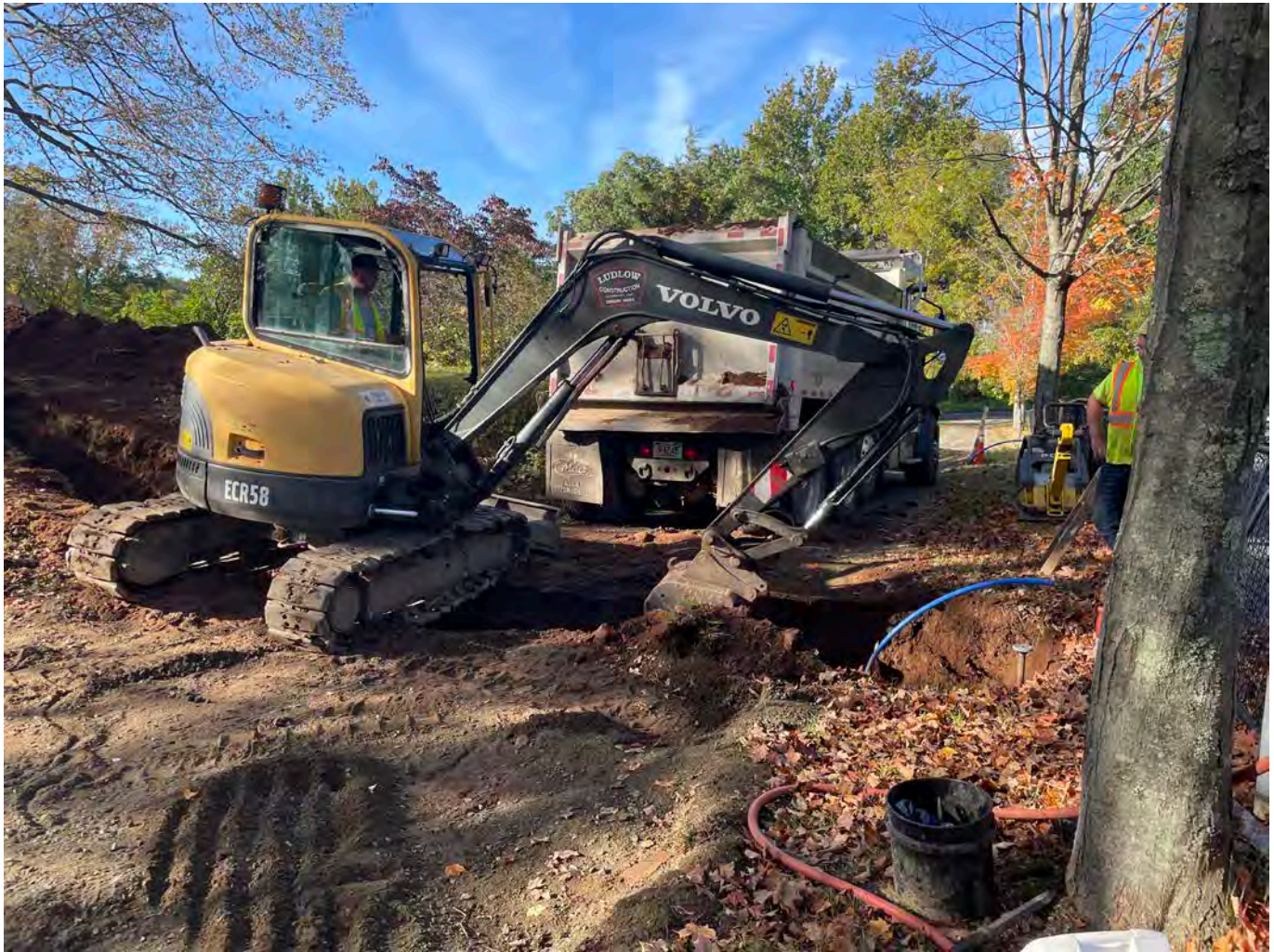
Picture 2: Ludlow excavating a trench on the south side of the curb stop for the 177R Main Street residence. View to the west.
