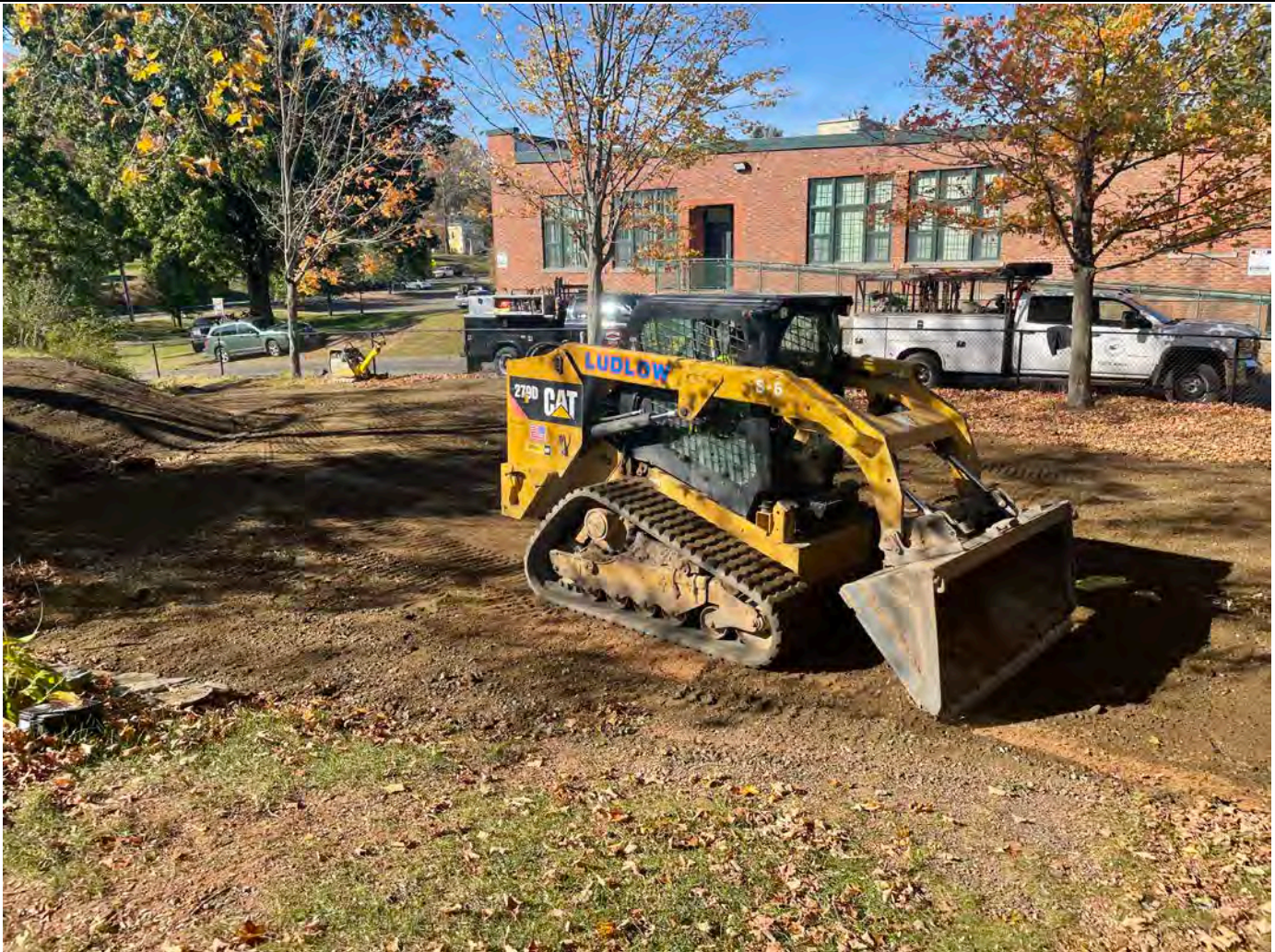
Picture 9: Ludlow grading gravel they replaced on the driveway for the 177R Main Street property. View to northwest.
