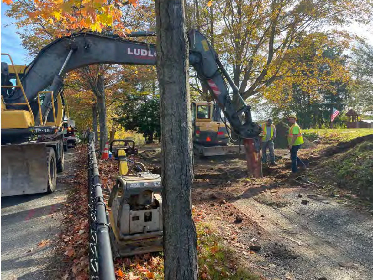
Picture 5: Ludlow hammering rock approximately 20' south of the curb stop for the 177R Main Street property. View to east.
