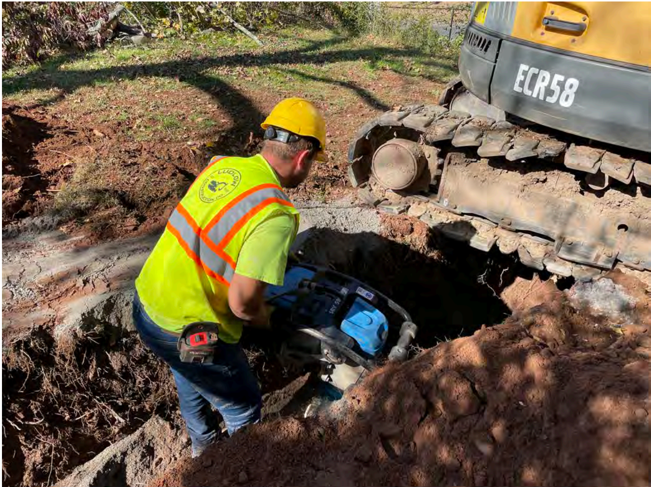
Picture 7: Ludlow compacting fill in the trench where they installed a 1" copper water service line for the 177R Main Street residence. View to northwest.
