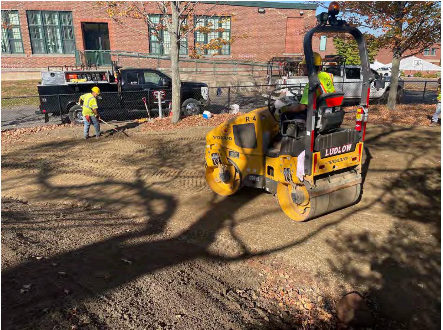
Picture 10: Ludlow compacting gravel they replaced on the driveway for the 177R Main Street property. View to north.
