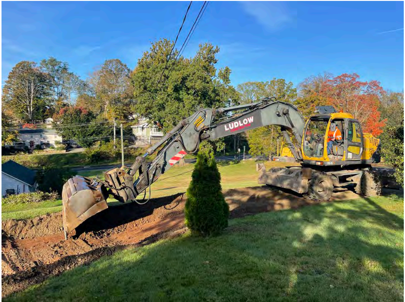
Picture 1: Ludlow removing a layer of gravel from the driveway for the 175 Main Street residence to clear a path for the installation of a 1.5" copper water service line. View to the west.
