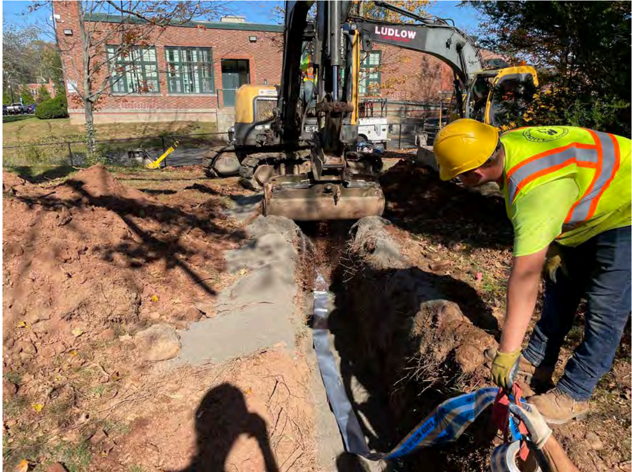
Picture 6: Ludlow placing sand and caution tape over 1" copper water service line for the 177R Main Street residence. View to the north.
