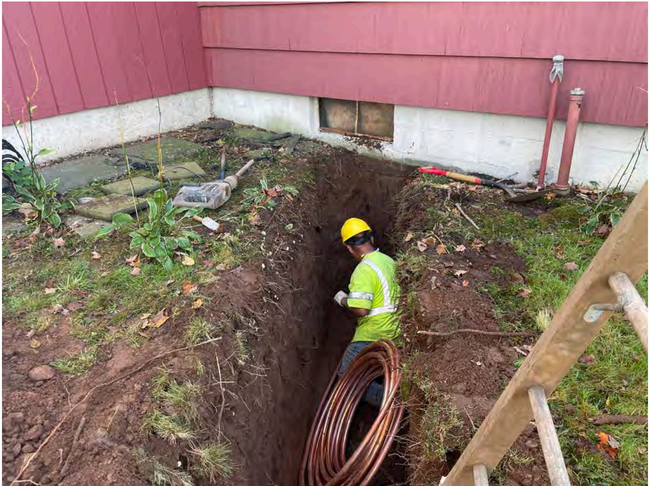
Picture 3: Ludlow inserting 1" copper pipe into the northern foundation of the 177R Main Street residence. View to the south.
