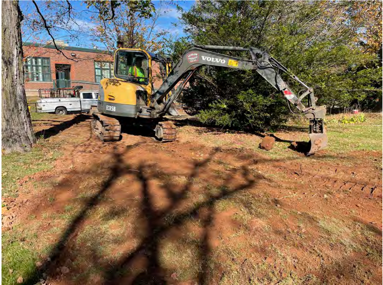
Picture 8: Ludlow placing fill as they backfill the trench they excavated for the installation of a 1" copper water service line for the 177R Main Street residence. View to the northwest.
