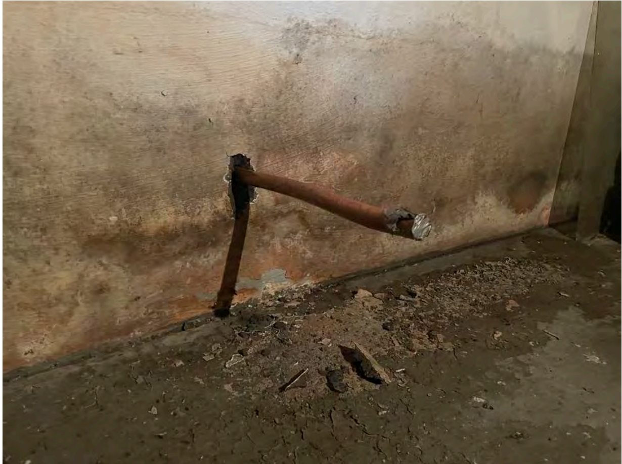
Picture 4: 1" copper pipe that Ludlow inserted through the northern foundation of the 177R Main Street residence. View to the northeast.
