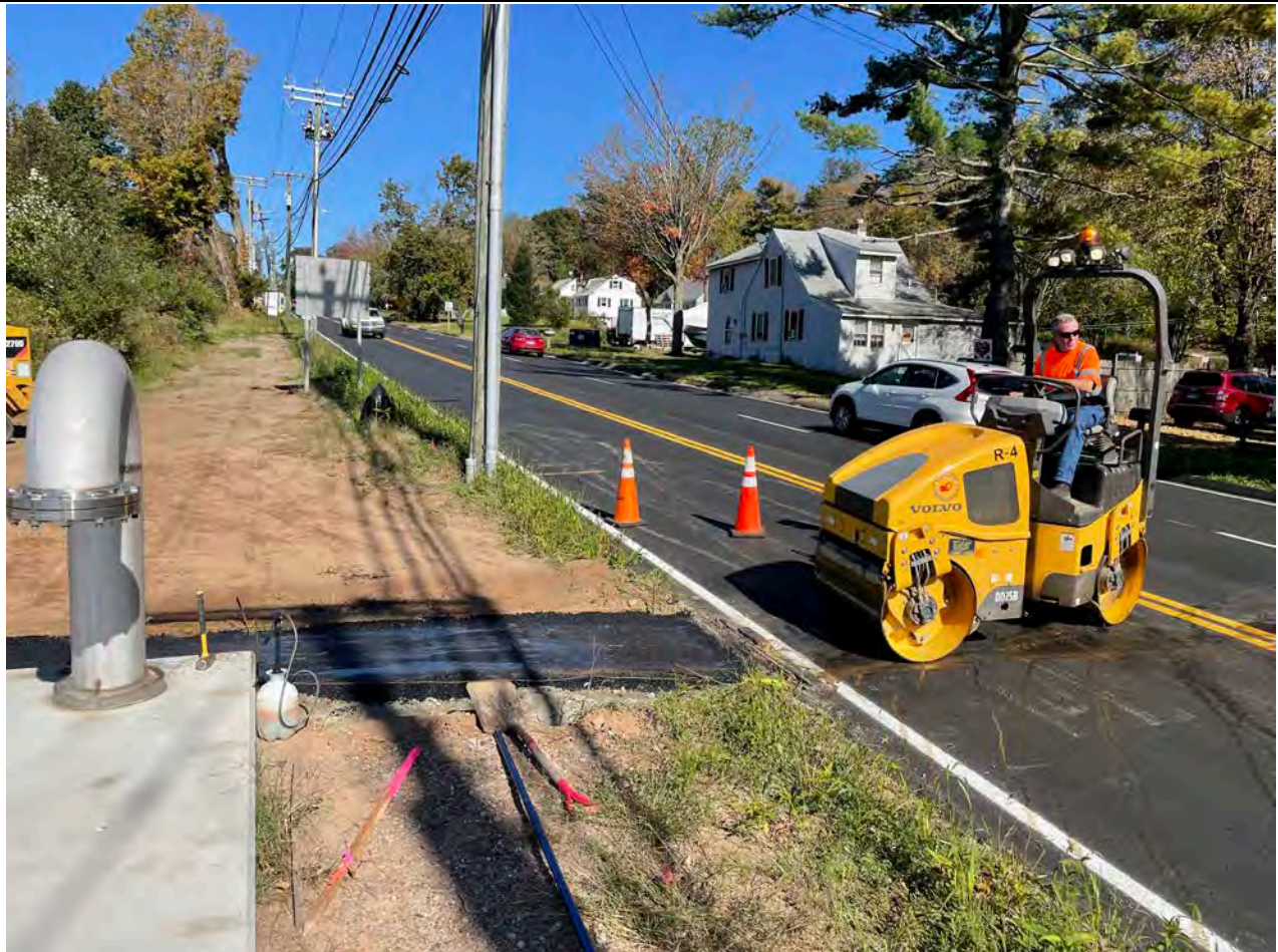
Picture 8: Ludlow compacting the first lift asphalt on the sidewalk located on the north side of the PRV vault. View to the north.
