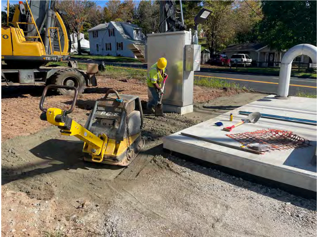
Picture 6: Ludlow working on the gravel base for the asphalt sidewalk they installed today at the PRV vault. View to northeast.
