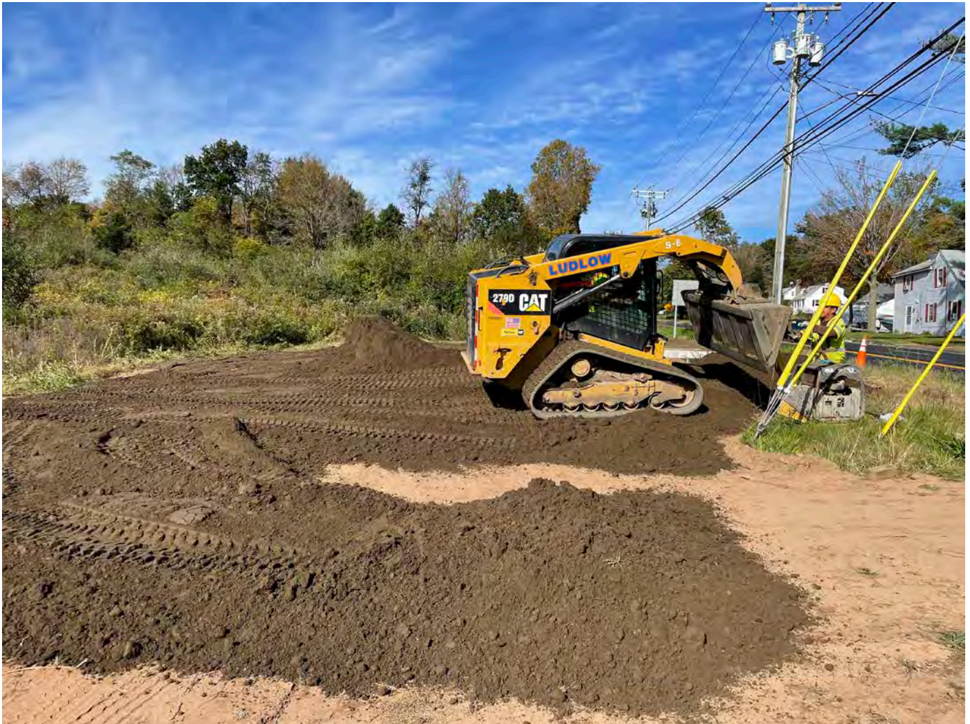
Picture 10: Ludlow placing loam on the south side of PRV vault. View to the north.
