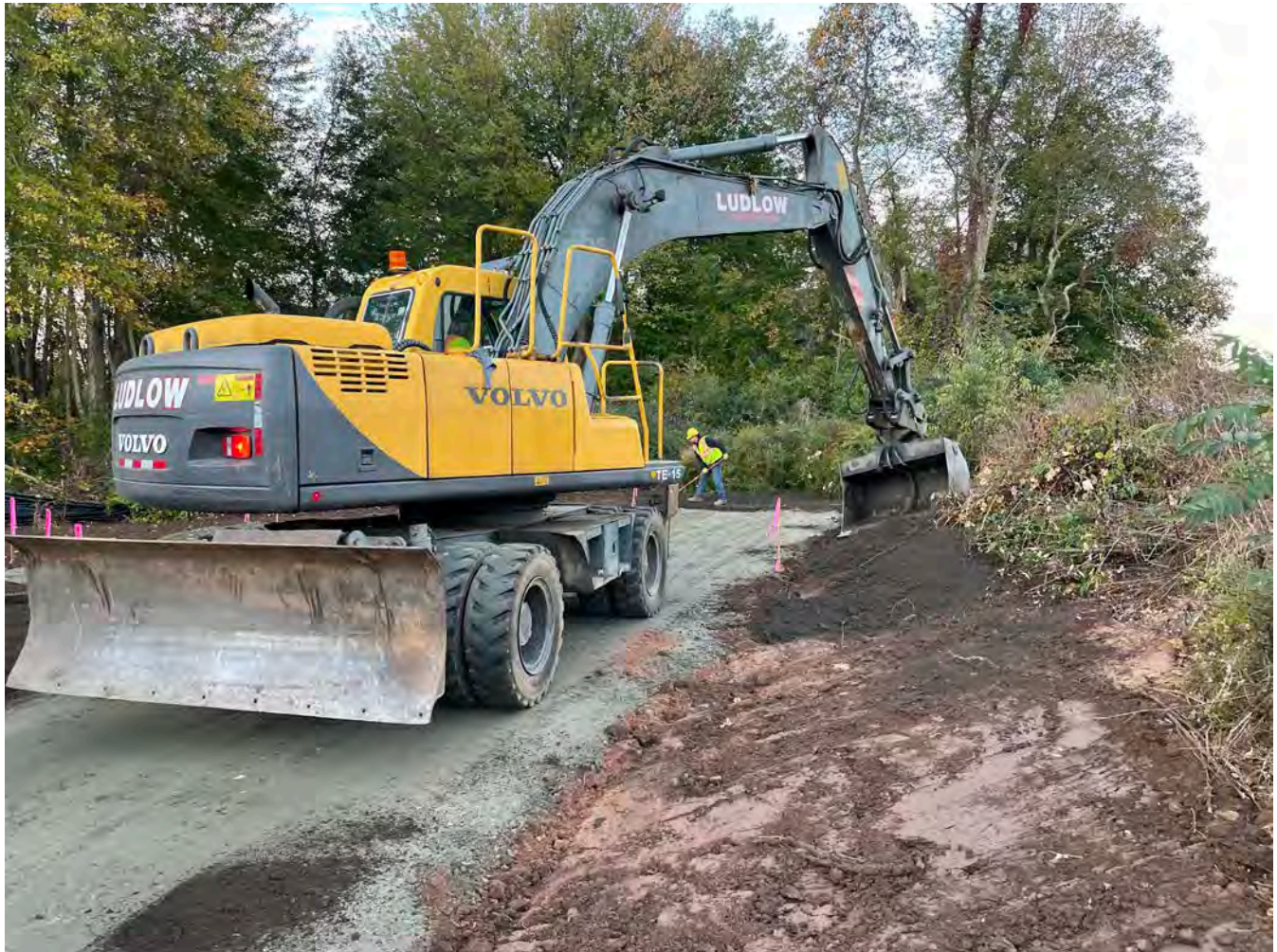
Picture 1: Ludlow placing loam on the north side of the driveway base at the booster station located at Station 750+63. View to the south.
