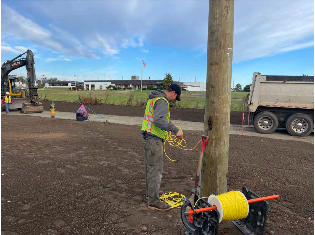
Picture 3: A&R Electrical running rope through one of the conduits coming off a newly installed pole at the booster station. View to the northwest.
