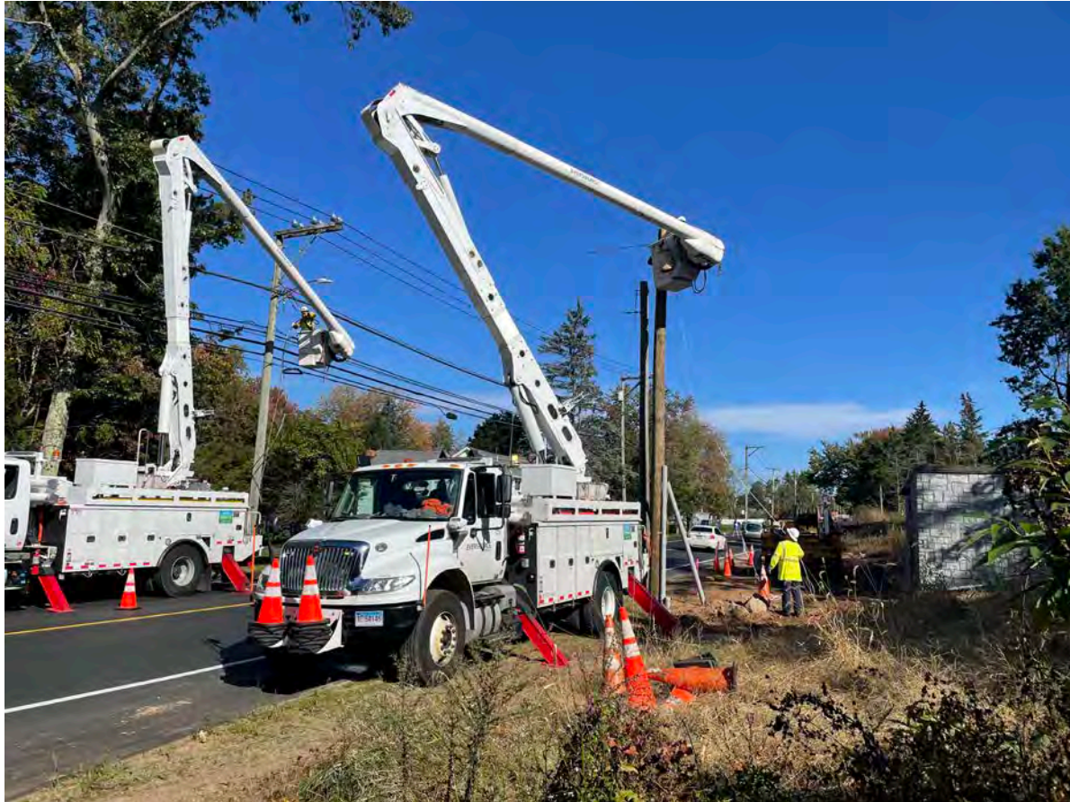
Picture 5: Eversource bringing power across S. Main Street to the new pole that was installed at the water meter building. View to north.
