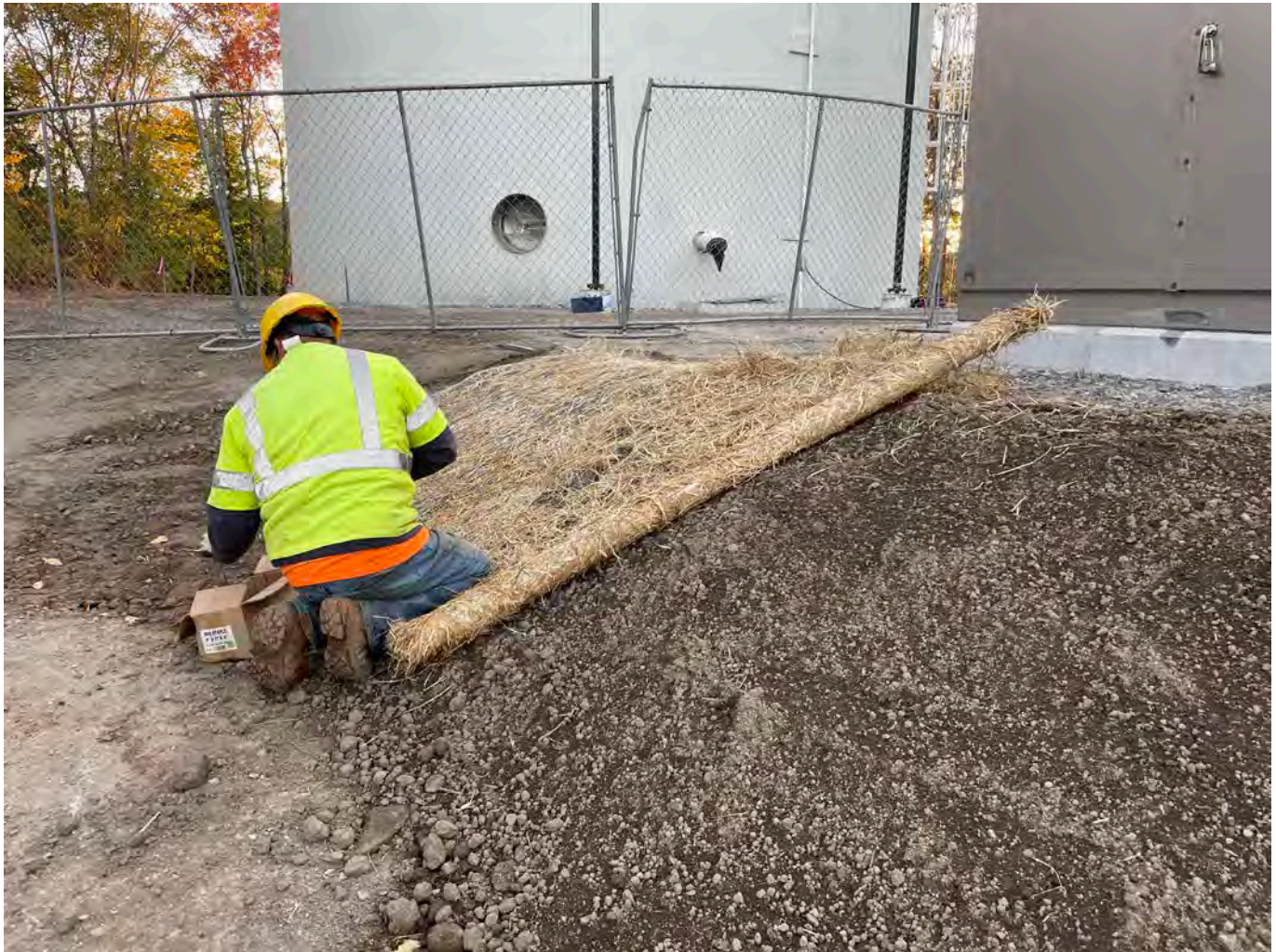
Picture 2: Ludlow placing straw erosion control mats on the north side of the electrical enclosure at the water tank work zone located east of the Shared Access Driveway in Middletown. View to the east.
