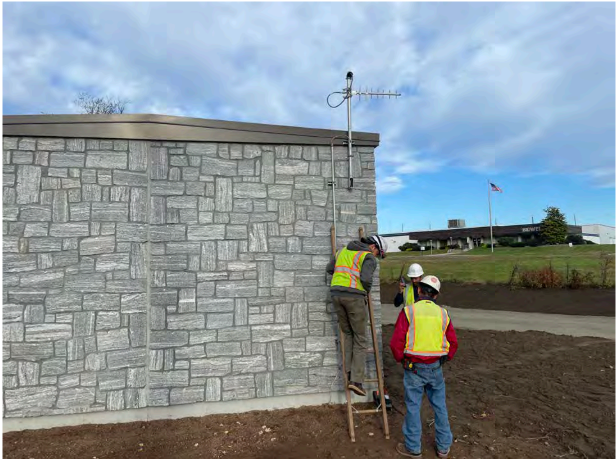
Picture 4: A&R Electrical installing an antenna on the northeast corner of the booster station. View to the northwest.
