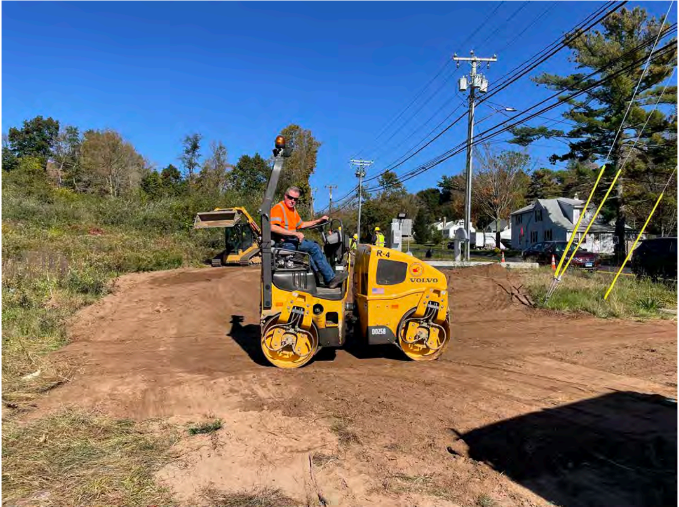
Picture 7: Ludlow compacting fill to the southwest of the PRV vault. View to north.
