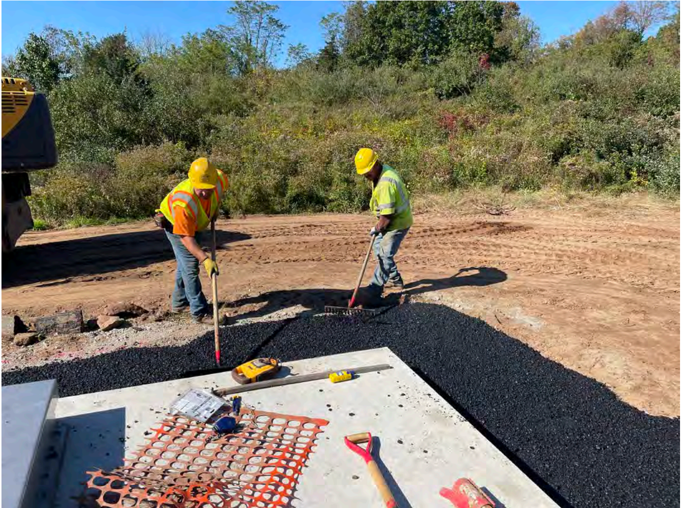
Picture 9: Ludlow raking asphalt on the sidewalk footprint on the west side of the PRV vault. View to west.
