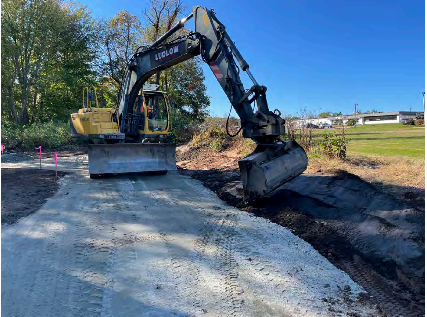
Picture 10: Ludlow placing loam on the north side of driveway base at the booster station located at Station 750+63. View to the west.
