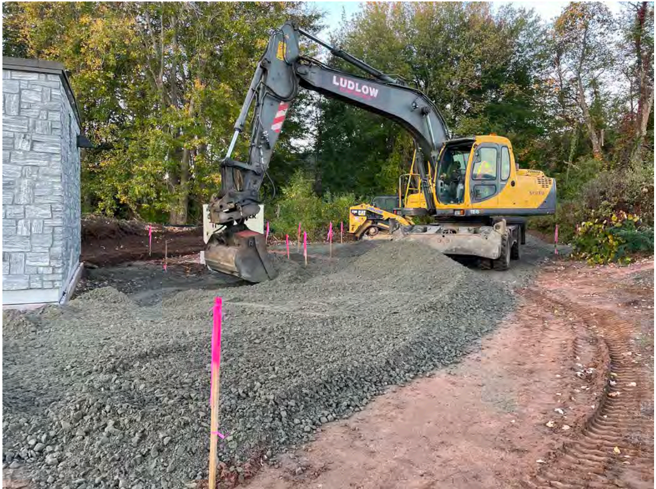
Picture 1: Ludlow placing 1.25"-minus gravel on the west side of the booster station. View to the south.
