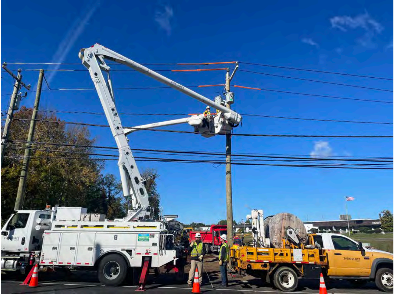
Picture 3: Eversource installing a transformer on one of the two new poles that Frontier installed next to the booster station. View to the west.
