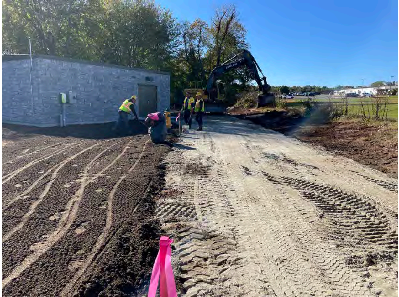
Picture 8: The north side of the booster station where Ludlow has placed and seeded loam on either side of the driveway base they constructed of compacted 1.25"-minus gravel. View to the west.
