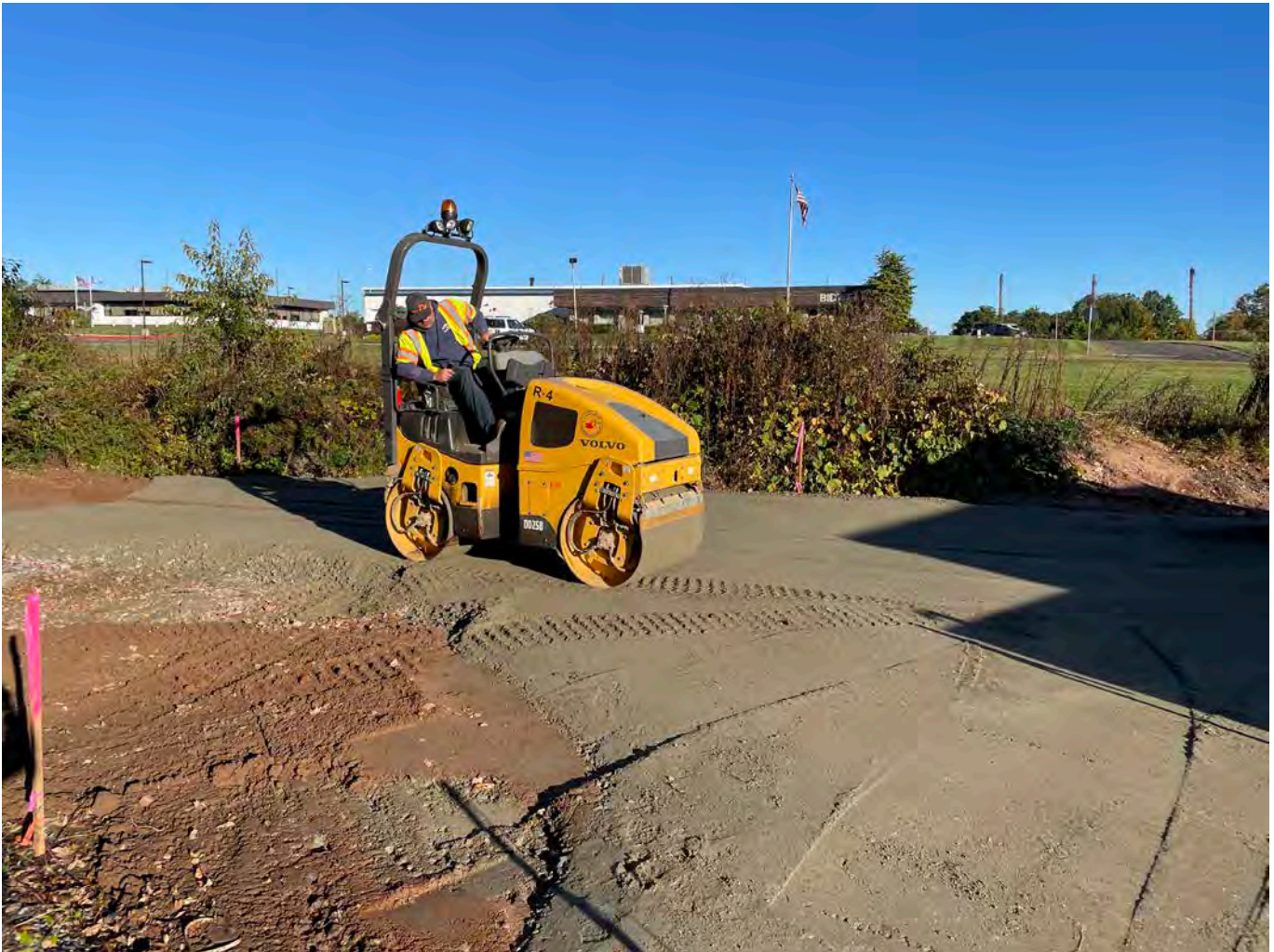
Picture 2: Ludlow compacting 1.25"-minus gravel to the northwest side of the booster station. View to the northeast.
