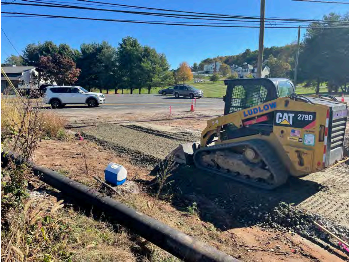
Picture 5: Ludlow placing 1.25"-minus gravel to the northeast of the booster station, building up the base for the driveway that Ludlow will be installing. View to southeast.
