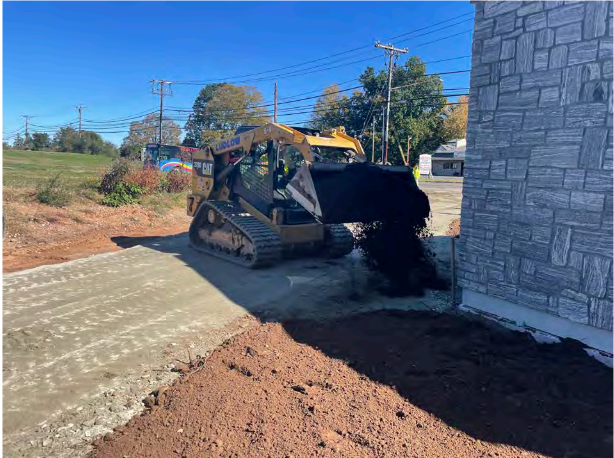
Picture 4: Ludlow placing loam on the northwest corner of the booster station. View to the northeast.
