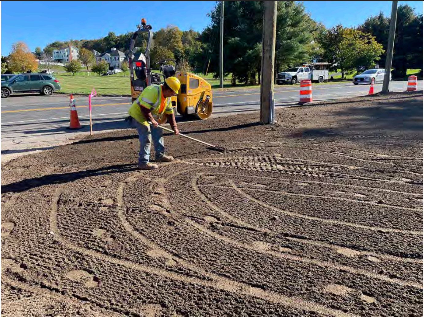
Picture 9: Ludlow raking grass seed into freshly placed loam to the northeast of the booster station. View to southwest.
