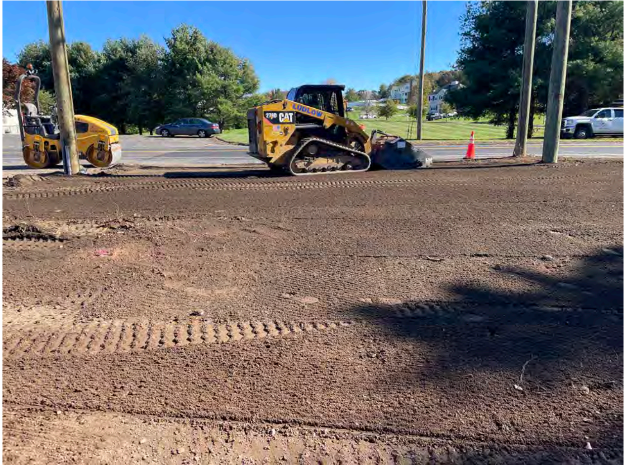
Picture 6: Ludlow sifting loam with a rockhound to the east of the booster station. View to east.
