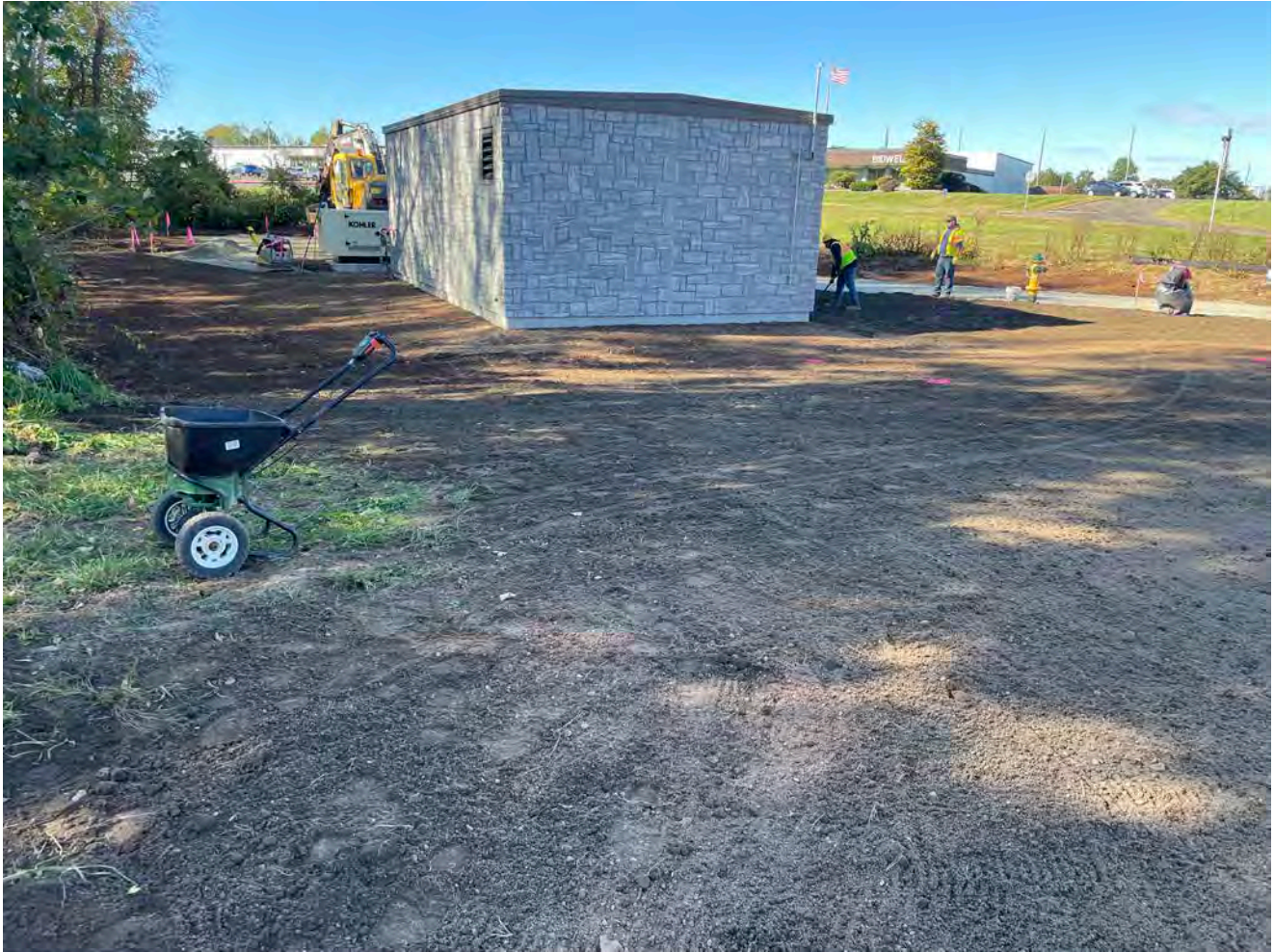
Picture 7: The booster station after Ludlow has placed and seeded loam. View to northwest.
