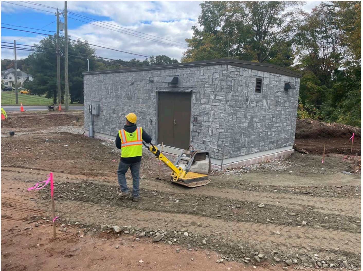
Picture 11: Ludlow compacting 1.25"-minus gravel on the northwest side of the booster station with a plate compactor. View to the southeast.
