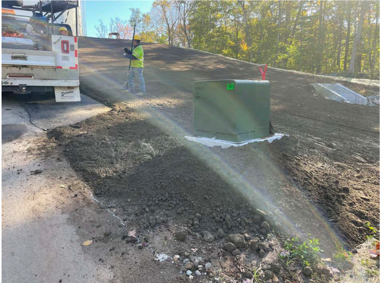
Picture 4: Loam that Ludlow has placed around the transformer and the pull-off located between Stations 11+43 and 11+78 on the south side of the Shared Access Driveway in Middletown. View to the southeast.
