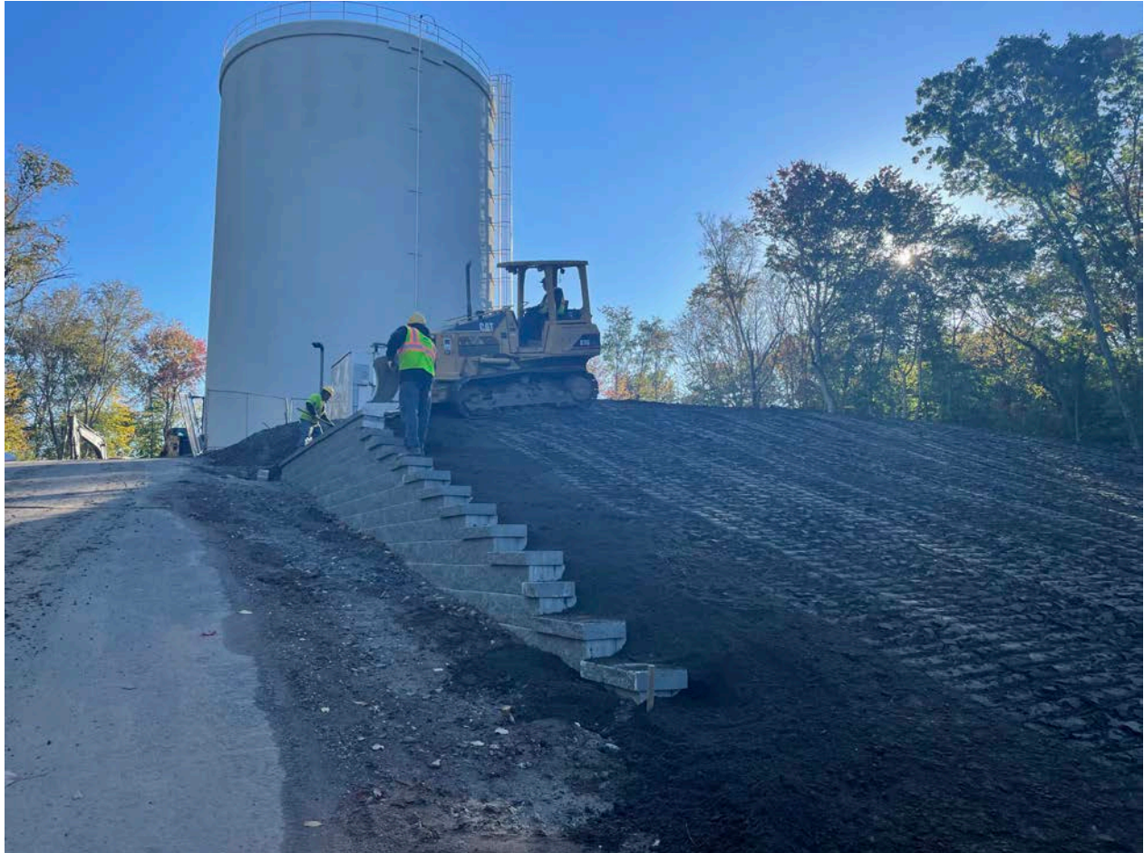
Picture 1: Ludlow raking and grading loam on the south side of the retaining wall. View to the east.
