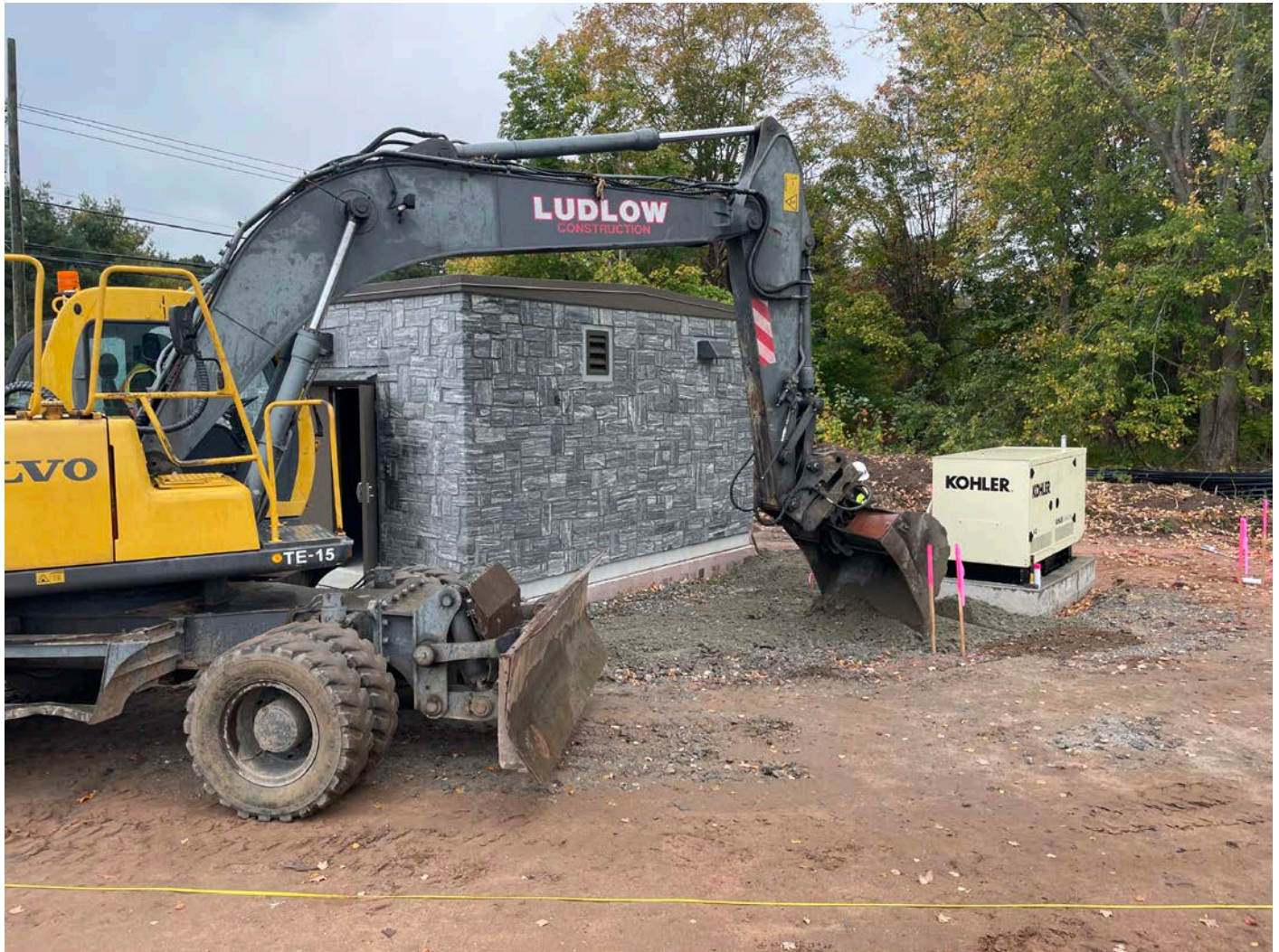
Picture 10: Ludlow grading fill on the west side of the booster station located at Station 750+63. View to the south.
