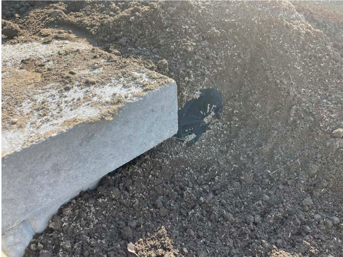
Picture 5: 4" perforated, corrugated, plastic drainpipe covered in filter fabric that is daylighted on the west end of the retaining wall on the south side of the wall. View to southeast.
