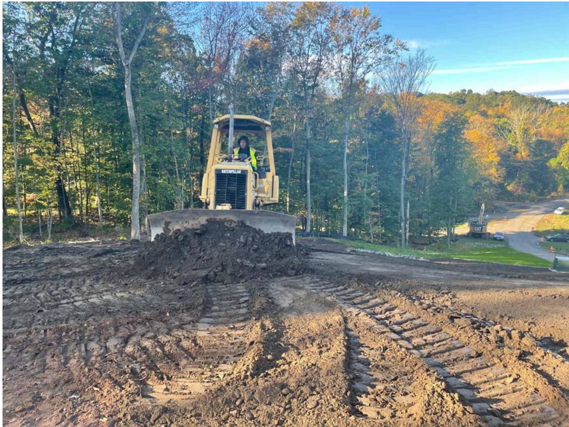
Picture 2: Ludlow grading loam on the slope located west of the altitude valve vault. View to west.
