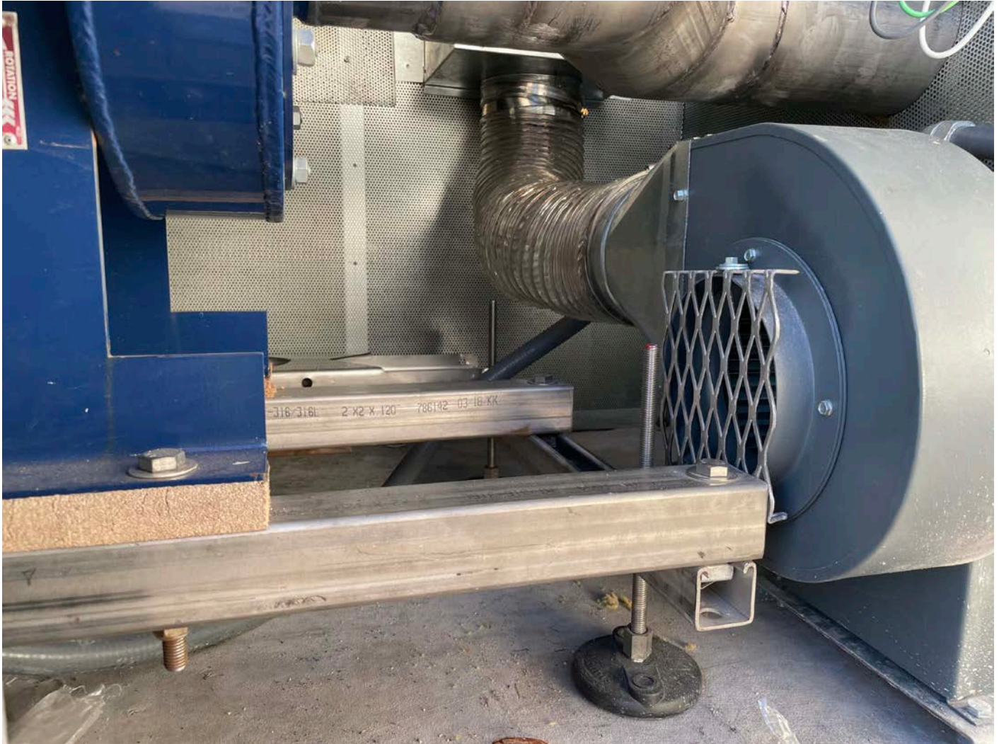
Picture 12: Flexible metal ducting that Brideau used to connect the blower to the exhaust outlet of the blower enclosure. View to the southwest.
