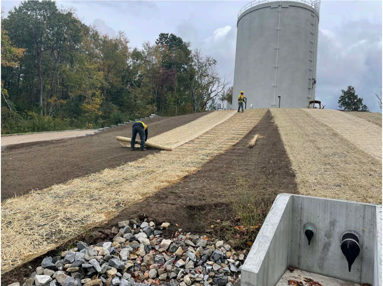
Picture 7: Ludlow placing straw erosion control mats over freshly raked and seeded loam located on the west side of the altitude valve vault. View to east.
