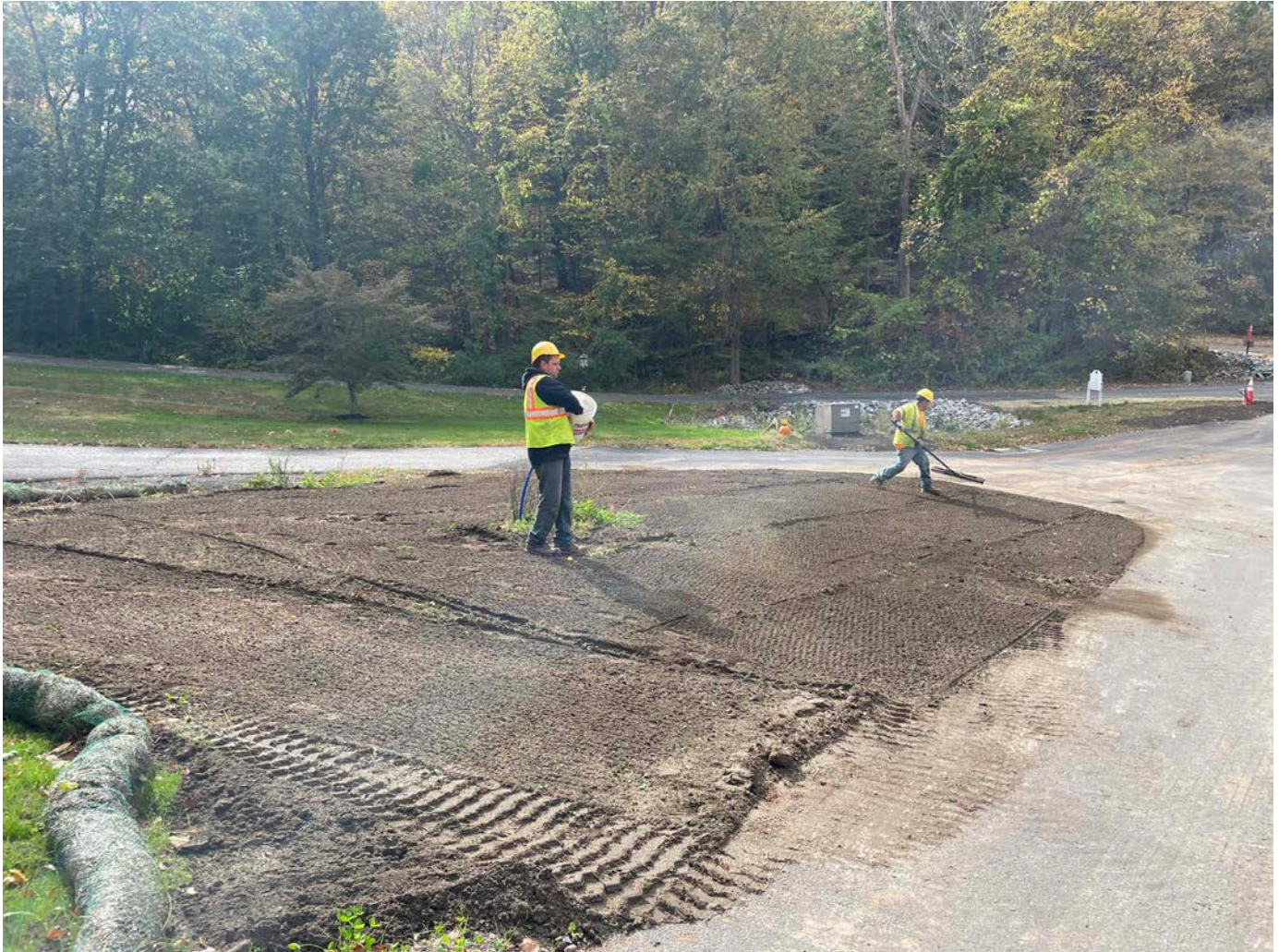
Picture 9: Ludlow placing grass seed over freshly raked loam on the south side of the Shared Access Driveway, east of the driveway for the 214 Talcott Ridge Drive property. View to southwest.
