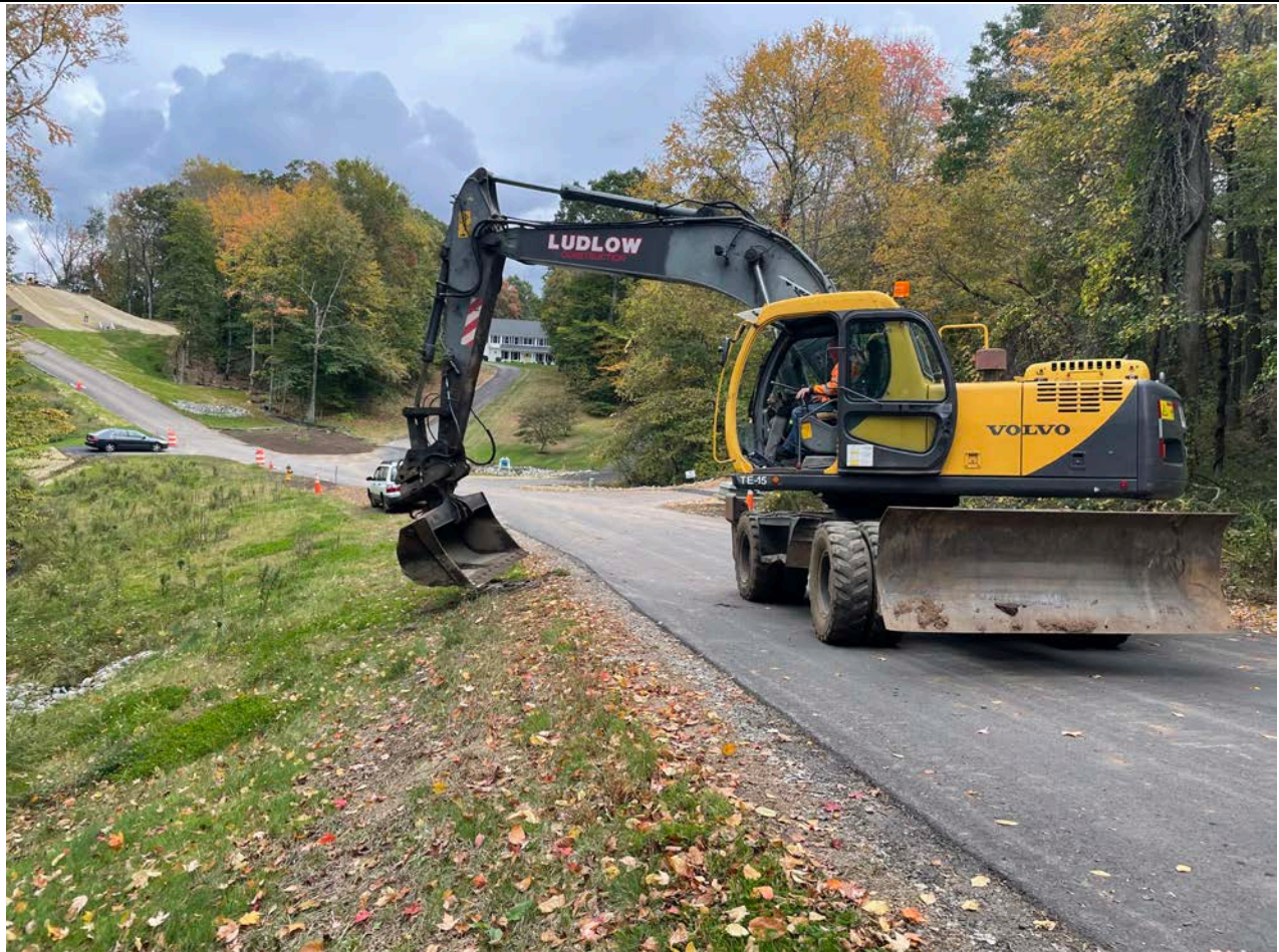
Picture 8: Ludlow refining the grade of the soil on the north side of the Shared Access Driveway at Station ~15+00. View to the east.
