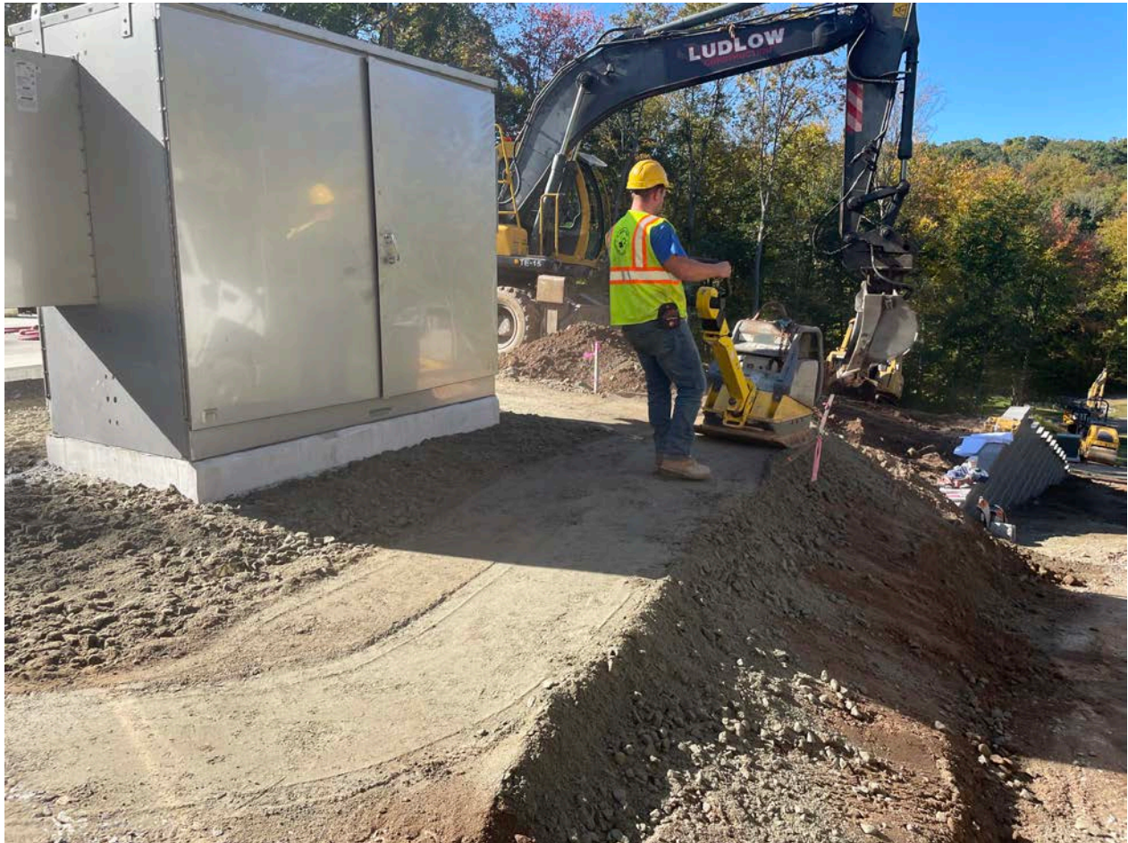
Picture 6: Ludlow using a plate compactor on 1.5"-minus gravel that was placed around the perimeter of the electrical enclosure located on the north side of the altitude valve vault at the water tank work zone. View to west.
