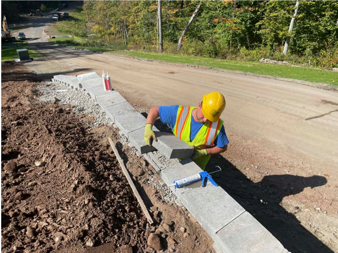
Picture 8: Ludlow securing capstones on the retaining wall located between Stations 10+83 and 11+34 with concrete adhesive. View to the west.
