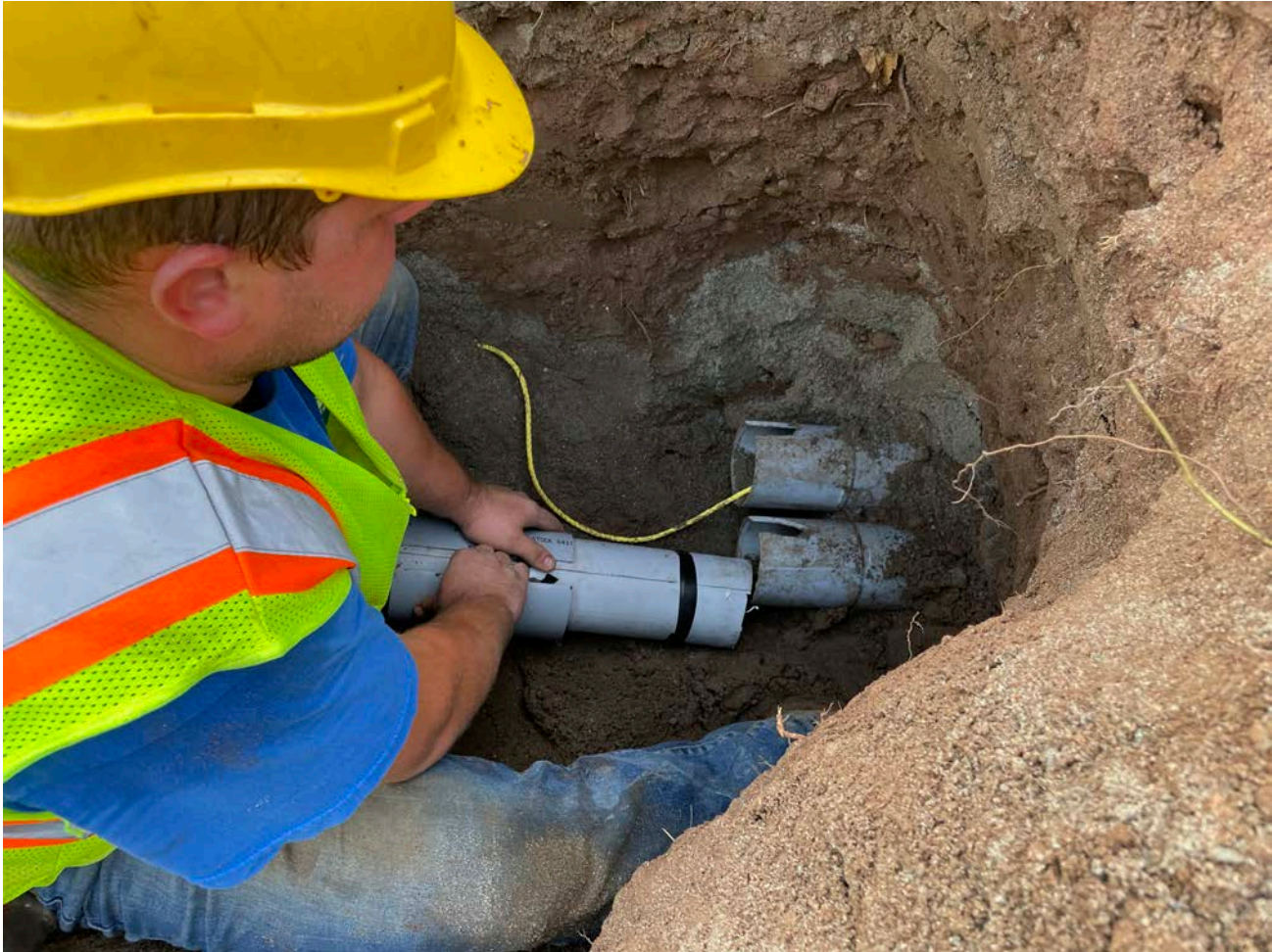
Picture 3: Ludlow repairing a 4" PVC utility conduit they previously damaged at Station ~10+90 on the Shared Access Driveway. View to the south.
