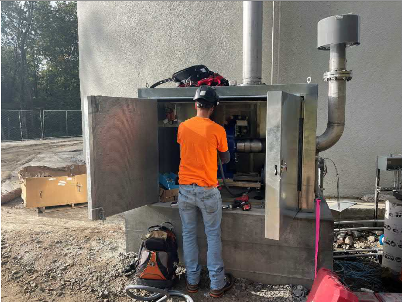
Picture 3: A&R Electrical working on wiring the blower located on the northeast side of the water tank. View to the southwest.
