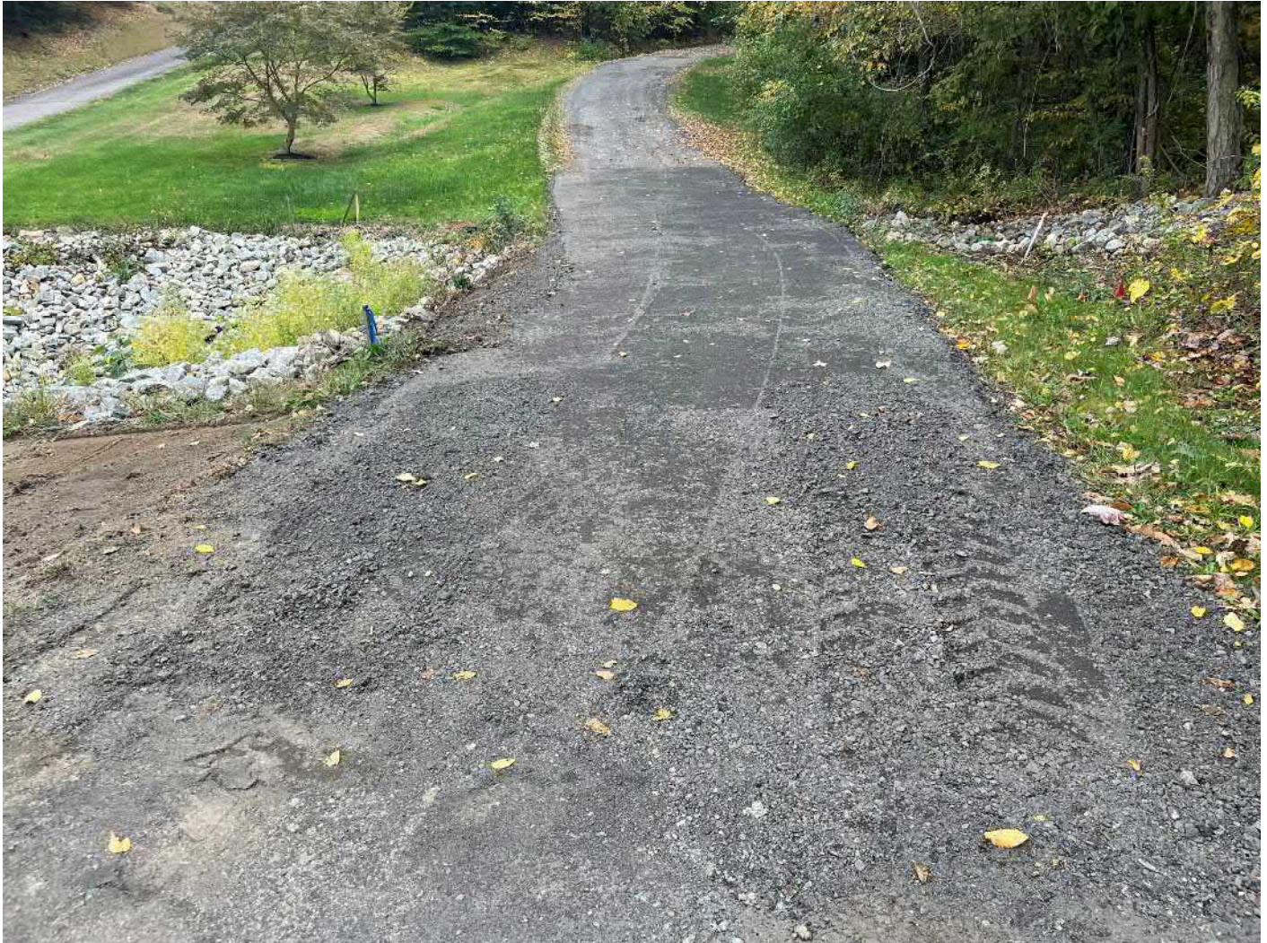
Picture 11: Driveway for the 216 Talcott Ridge Drive property that Ludlow reworked today in order to direct overland flow into the plunge bowl located on the northeast side of the driveway. View to the southeast.
