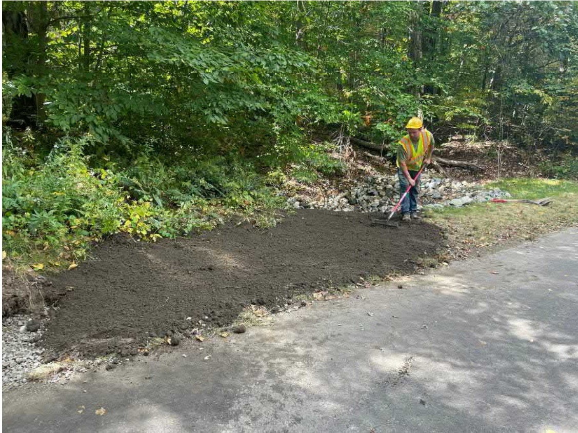
Picture 8: Ludlow raking loam that they placed over filter fabric that was placed on top of the \frac{3}{4} " stone Ludlow used to cover the 4" plastic drain pipe they just installed on the south edge of the Shared Access Road. Approximately Stations 19+60 to 19+75. View to southwest.
