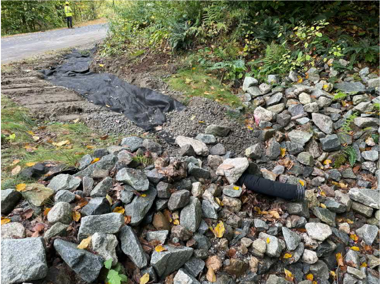
Picture 6: 4" corrugated, perforated, plastic pipe daylighting into the plunge bowl located at Station ~19+85. Ludlow later covered the black filter fabric with loam. View to the northeast.
