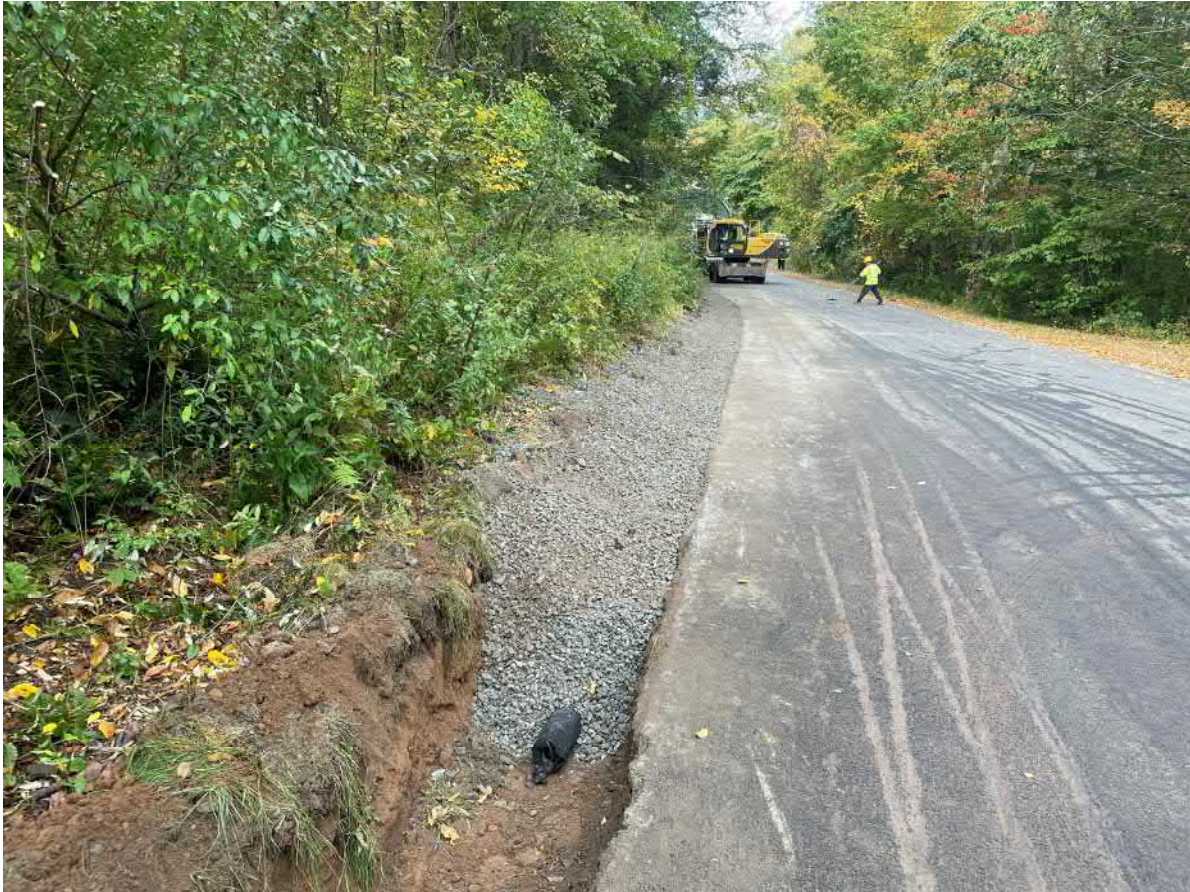
Picture 5: 4" corrugated, perforated, plastic pipe that Ludlow has covered with ¾" stone on the south edge of the Shared Access Road between Stations 18+15 and 19+75. View to west.
