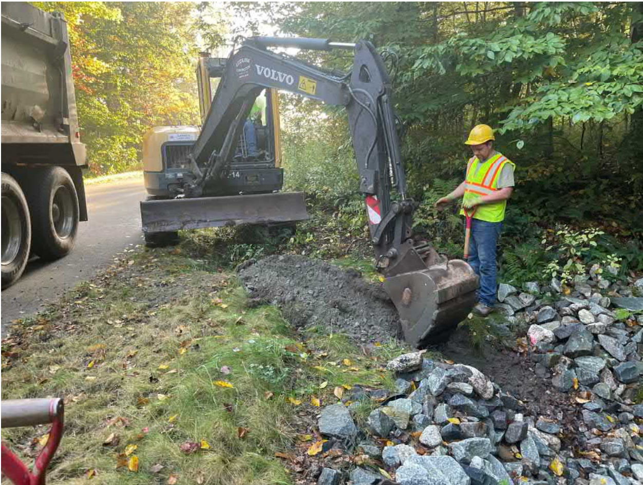
Picture 1: Ludlow beginning excavation at Station 19+75 along the south edge of the Shared Access Road and the east side of a plunge bowl, working east. View to northeast.
