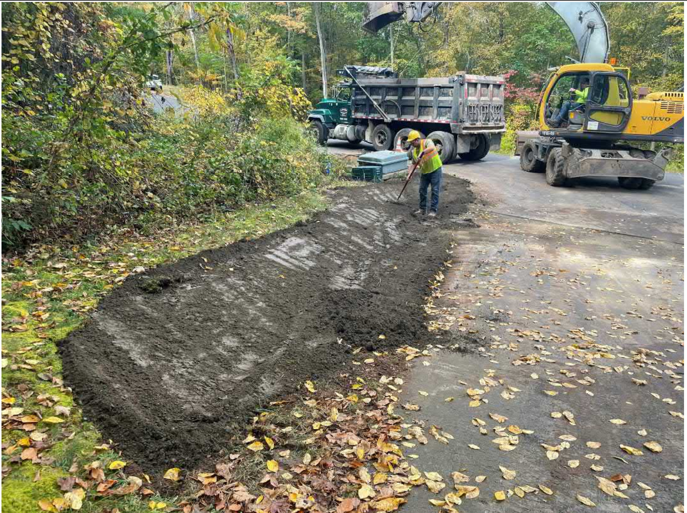
Picture 10: Ludlow raking out loam they placed on the west side of the driveway for the 224 Talcott Ridge Drive property after reshaping the soils to better direct overland flow into the catch basin located at the northwest corner of the driveway. View to the north.
