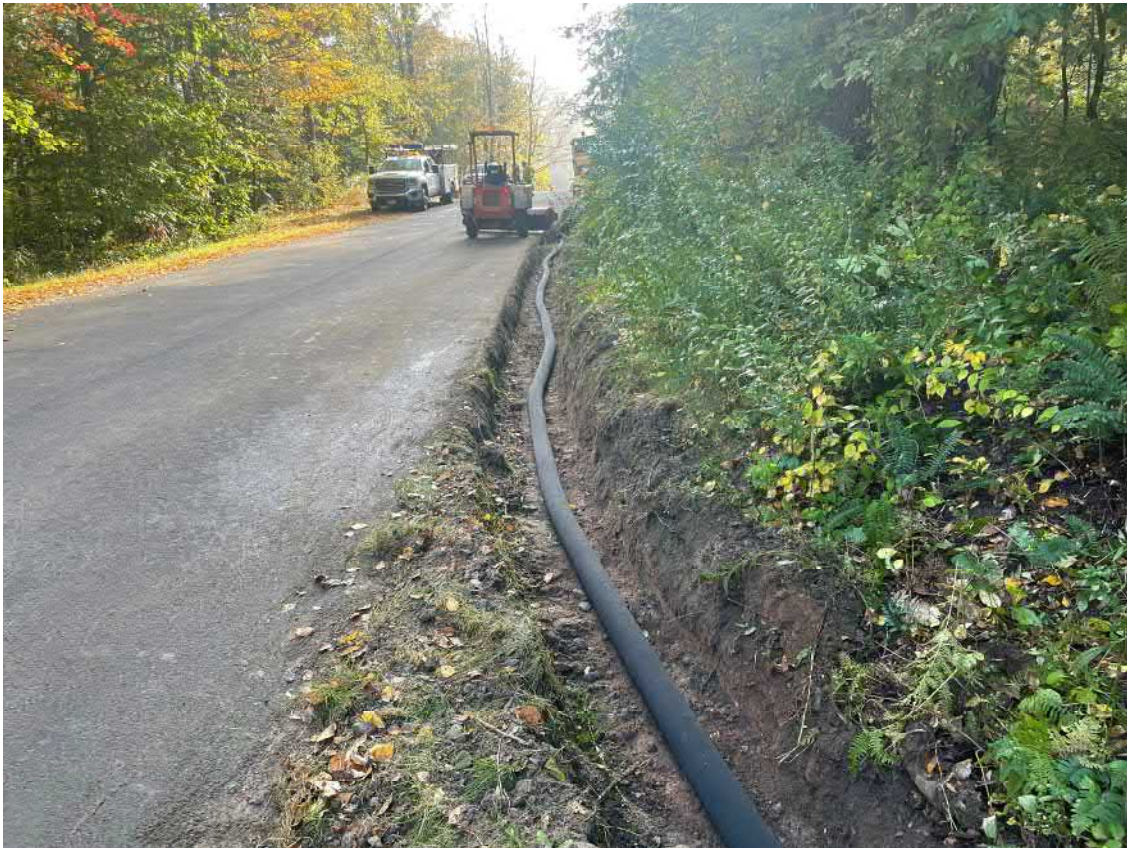
Picture 2: 4" corrugated, perforated, plastic pipe that Ludlow has placed on the south edge of the Shared Access Road between Stations 18+15 and 19+75. View to east.
