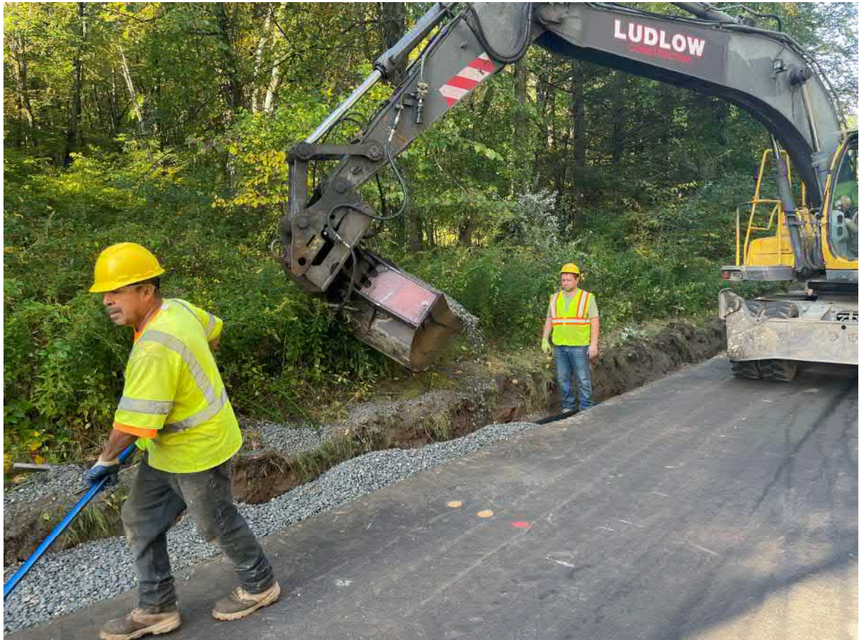
Picture 4: Ludlow placing \frac{3}{4} " stone over the 4" corrugated, perforated, plastic pipe they just placed along the south edge of the Shared Access Road. View to the southwest.
