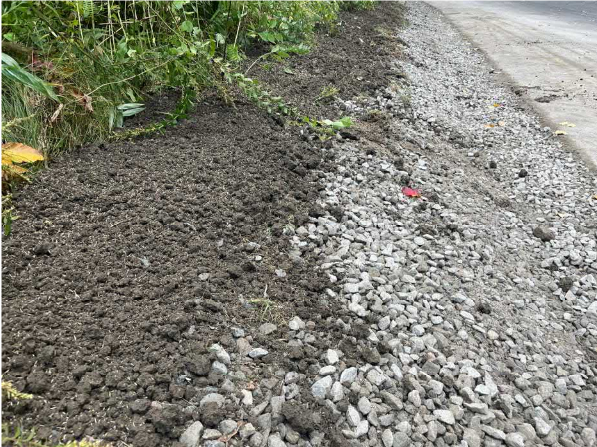
Picture 9: Seeded loam that was placed on the south edge of the 3/4" stone that Ludlow used to cover the 4" plastic drain pipe they just installed on the south edge of the Shared Access Road. View to the west.
