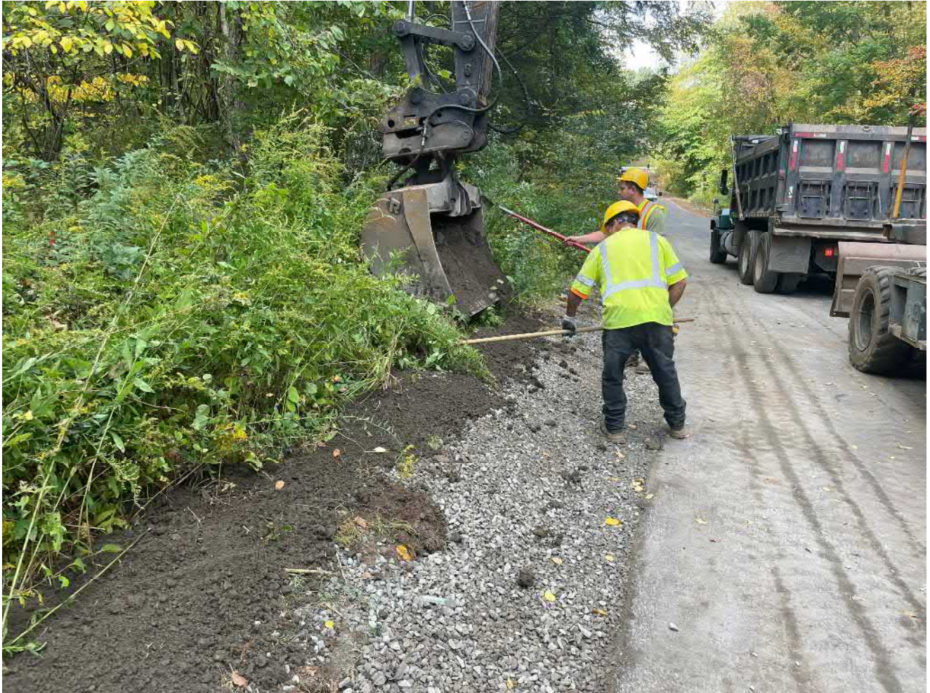
Picture 7: Ludlow placing loam on the south edge of the \frac{3}{4} " stone they placed over 4" plastic drain pipe on the south edge of the Shared Access Road. View to the west.
