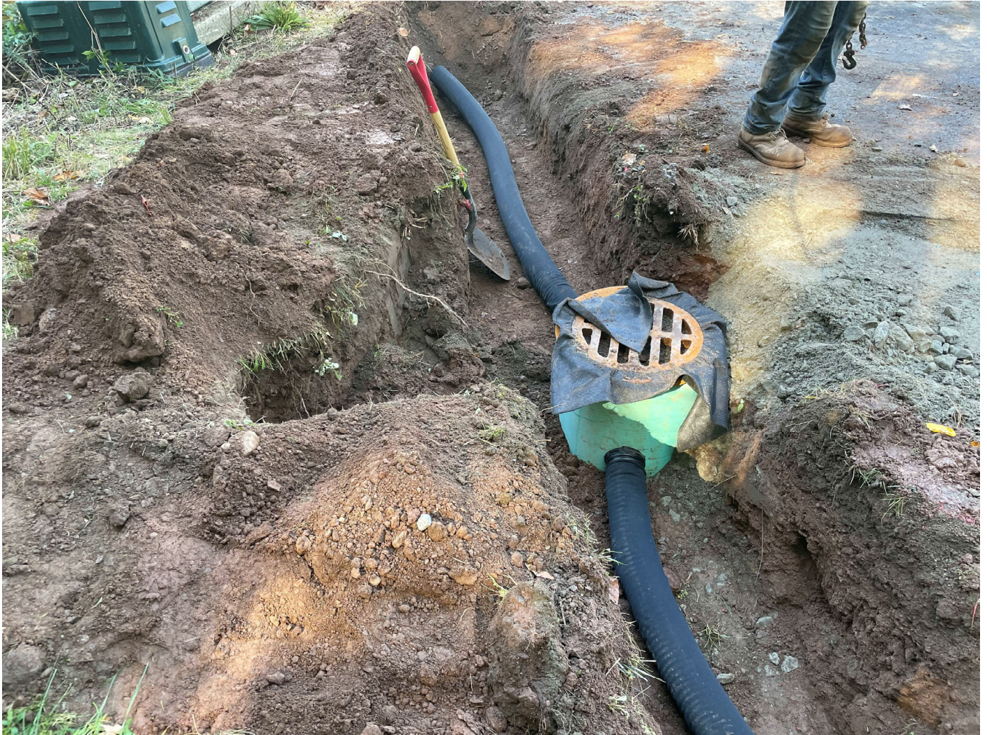
Picture 11: 4" corrugated, perforated plastic pipe (encased on a filter sock) that Ludlow placed in a trench they excavated on the west side of the driveway for the 224 Talcott Ridge Drive property. The sections of pipe connect to the 18" PVC riser of the catch basin that Ludlow installed on the west side of the driveway. View to the north.
