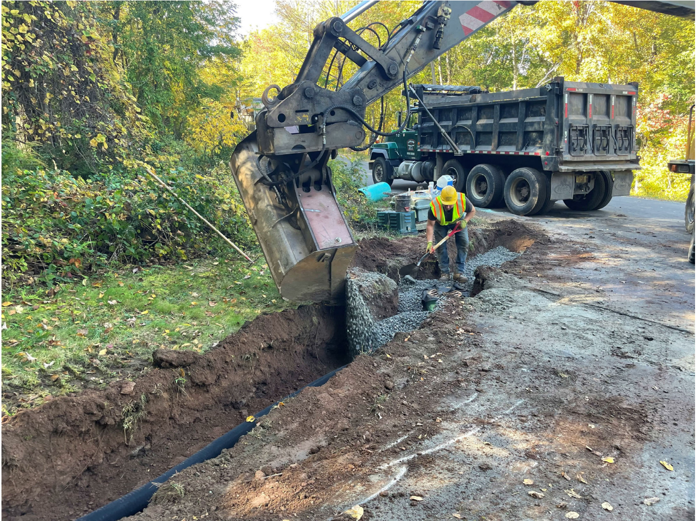
Picture 12: Ludlow placing 3/4" stone over 4" corrugated, perforated plastic pipe (encased on a filter sock) that Ludlow placed in a trench they excavated on the west side of the driveway for the 224 Talcott Ridge Drive property. View to the northwest.
