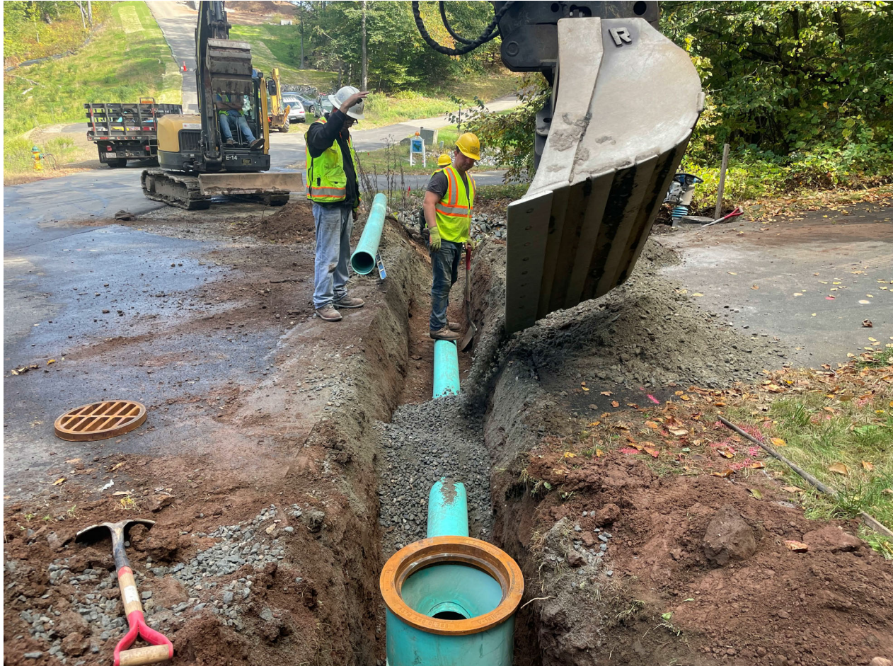
Picture 6: Ludlow placing \frac{3}{4} " stone over a section of 8" PVC pipe they have placed in the trench they excavated across the driveway for the 224 Talcott Ridge Drive property. The west side of the 8" PVC pipe terminates in the 18" PVC riser of a catch basin they just installed. View to the east.
