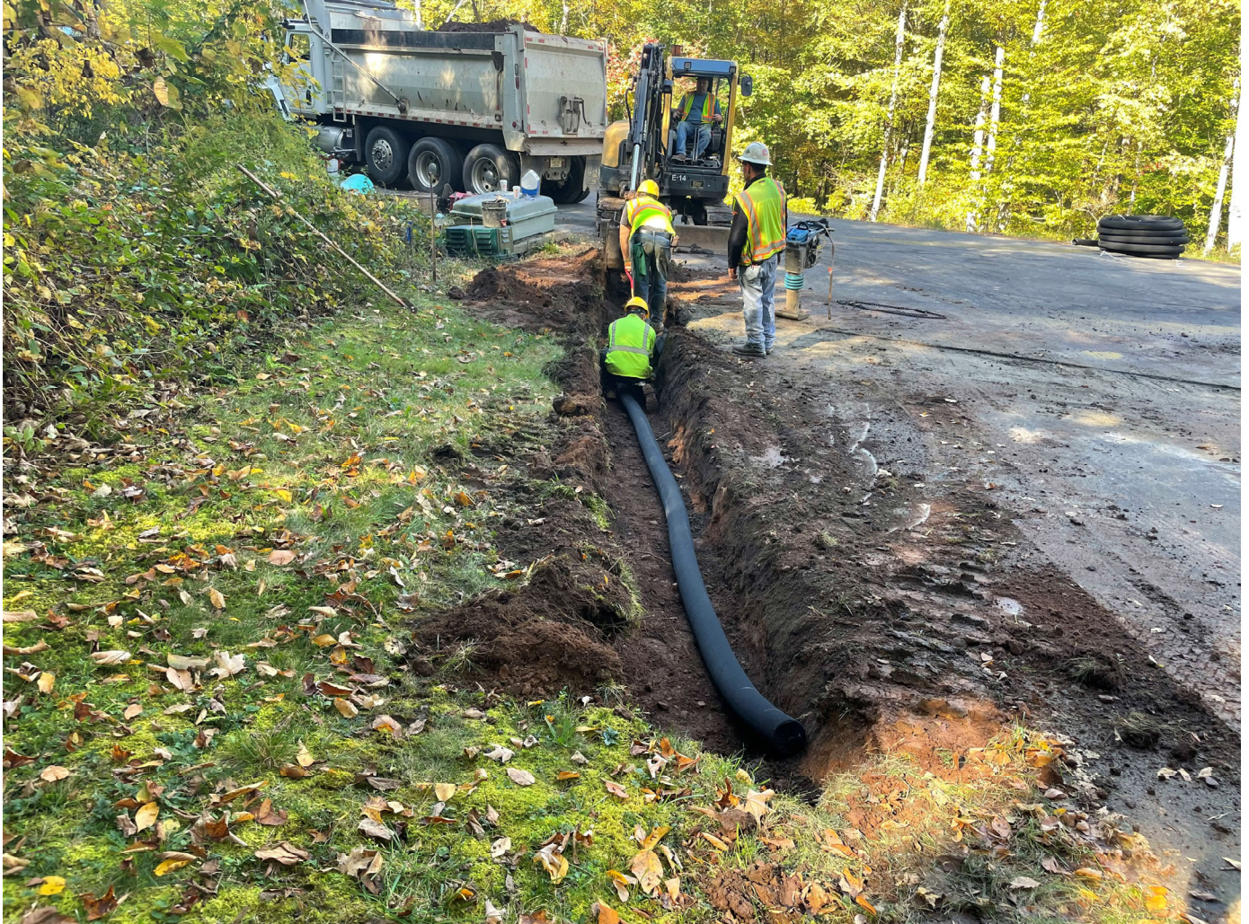
Picture 10: Ludlow placing a section of 4" corrugated, perforated plastic pipe (encased on a filter sock) in a trench they excavated on the west side of the driveway for the 224 Talcott Ridge Drive property. View to the north.
