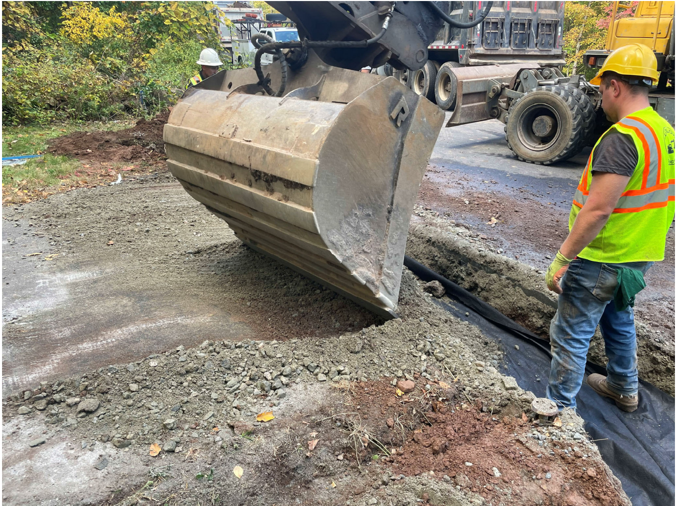
Picture 7: Ludlow placing fill over a section of filter fabric that was placed over ¾" stone that was placed over the 8" PVC pipe that Ludlow placed in the trench on the driveway for the 224 Talcott Ridge Drive property. View to pipe the northwest.
