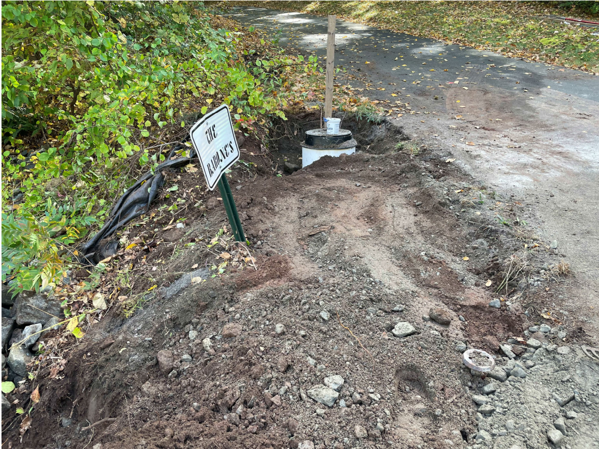
Picture 9: Meter pit that Ludlow installed 8' north of the curb stop for the 224 Talcott Ridge Drive property. View to the south.
