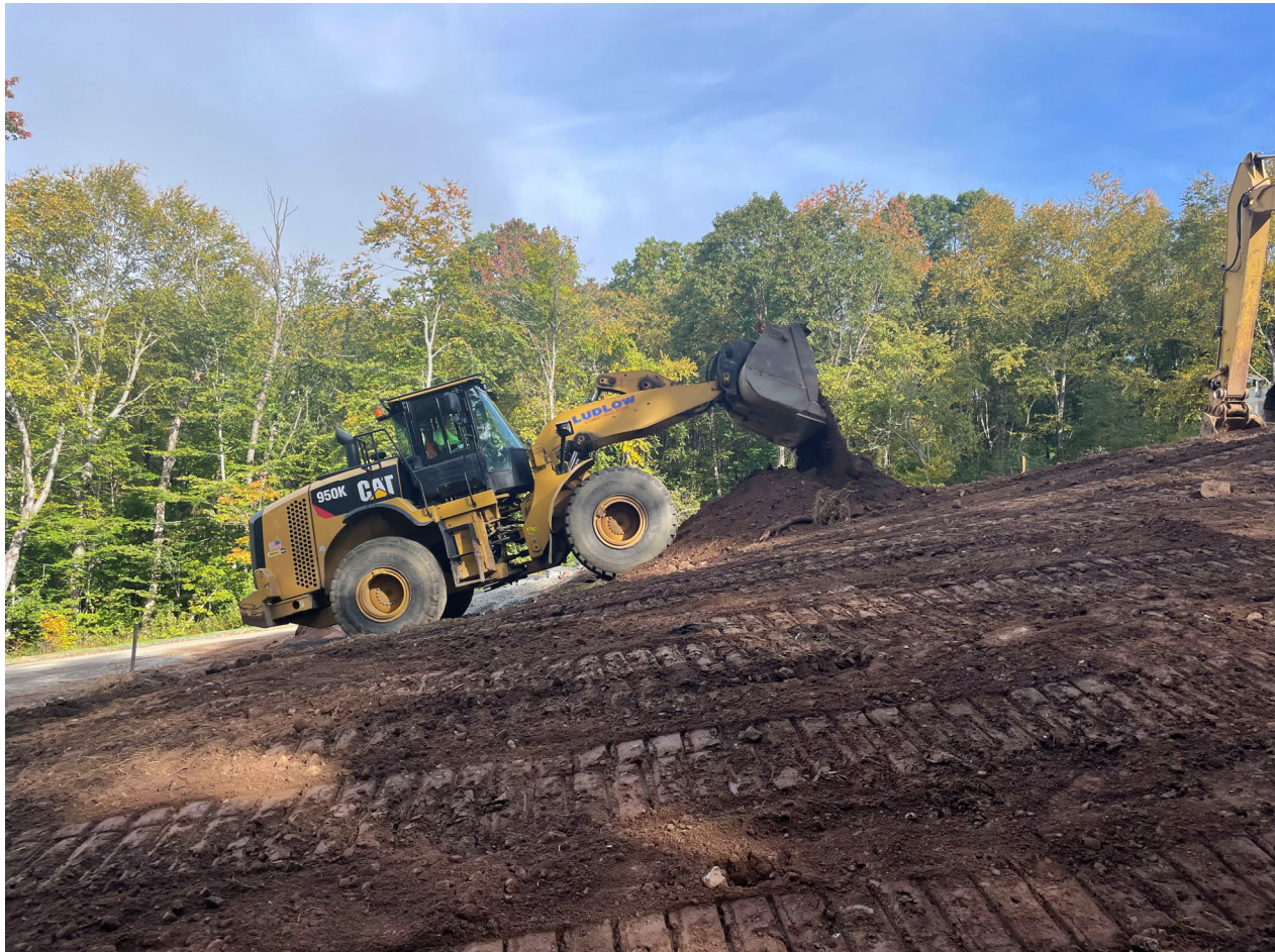
Picture 1: Ludlow placing fill on the slope located on the west side of the water tank. View to north.
