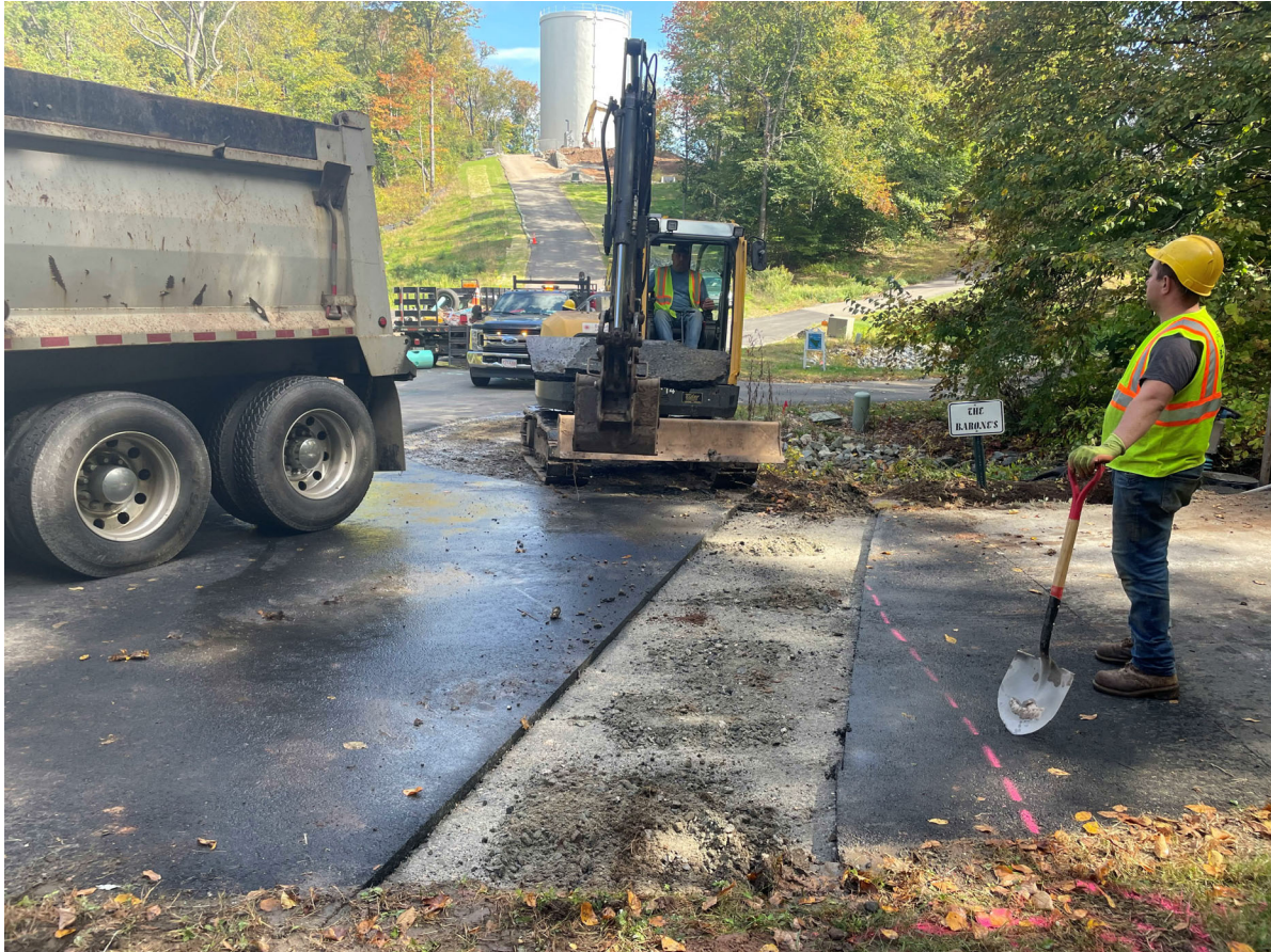
Picture 5: Trench footprint on the driveway for the 224 Talcott Ridge Drive property where Ludlow has removed asphalt as they prepare to excavate a trench. View to the east.
