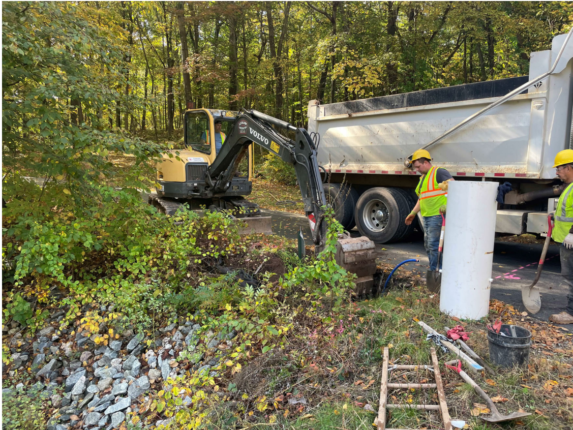
Picture 2: Ludlow excavating on the south side of the curb stop for 224 Talcott Ridge Drive for the installation 1" copper water service line that will run to a meter pit they will install approximately 8' south of the curb stop. View to southwest.
