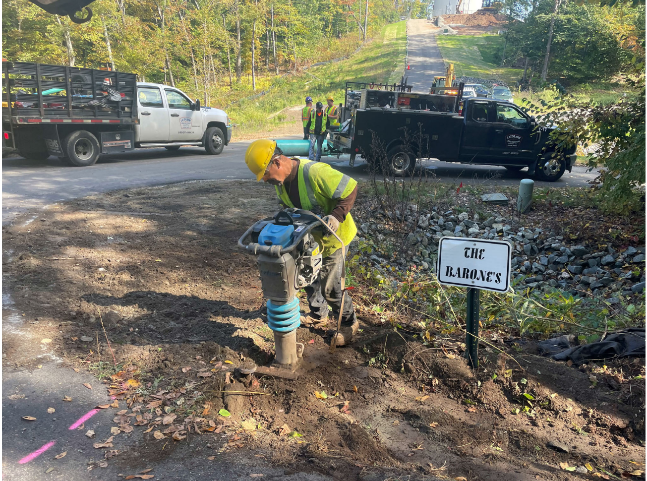
Picture 3: Ludlow compacting soil next to the curb stop for the 224 Talcott Ridge Drive after installing a 1" copper water service line on the south side of the curb stop. View to the northeast.
