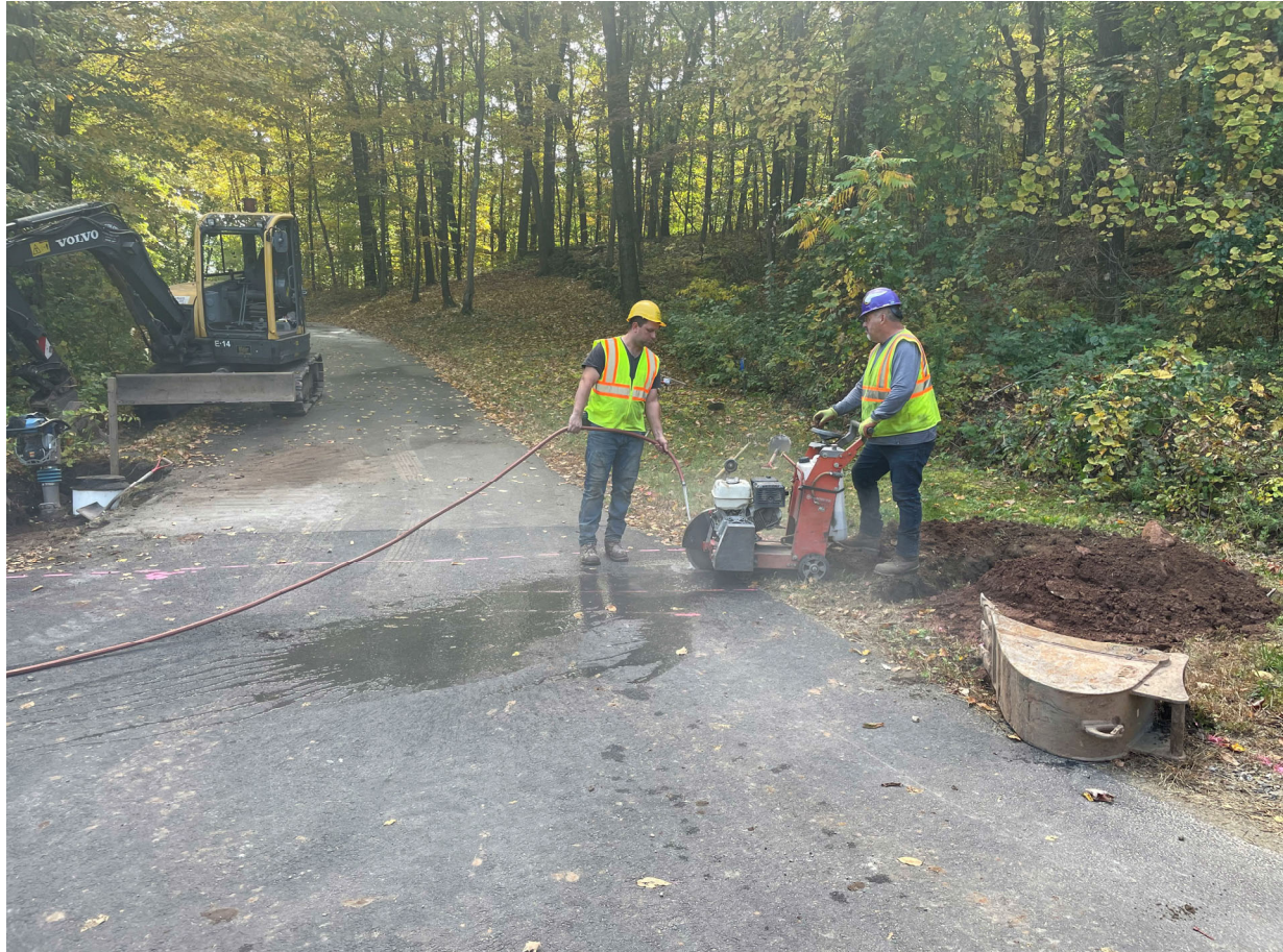
Picture 4: Ludlow saw cutting asphalt on the driveway for the 224 Talcott Ridge Drive property as they prepare to excavate a trench. View to the south.
