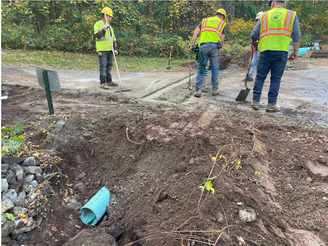
Picture 8: View of backfilled trench after Ludlow installed a section of 8" PVC pipe across the driveway for the 224 Talcott Ridge Drive property. The east side of the 8" PVC pipe discharges to the plunge bowl located on the east side of the driveway entrance. View to west.
