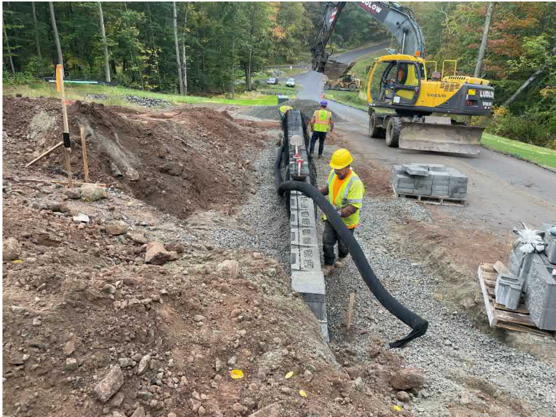
Picture 2: Ludlow placing 4" drain pipe covered in a filter sock on the south side of the retaining wall located between Stations 10+83 and 11+34. View to west.
