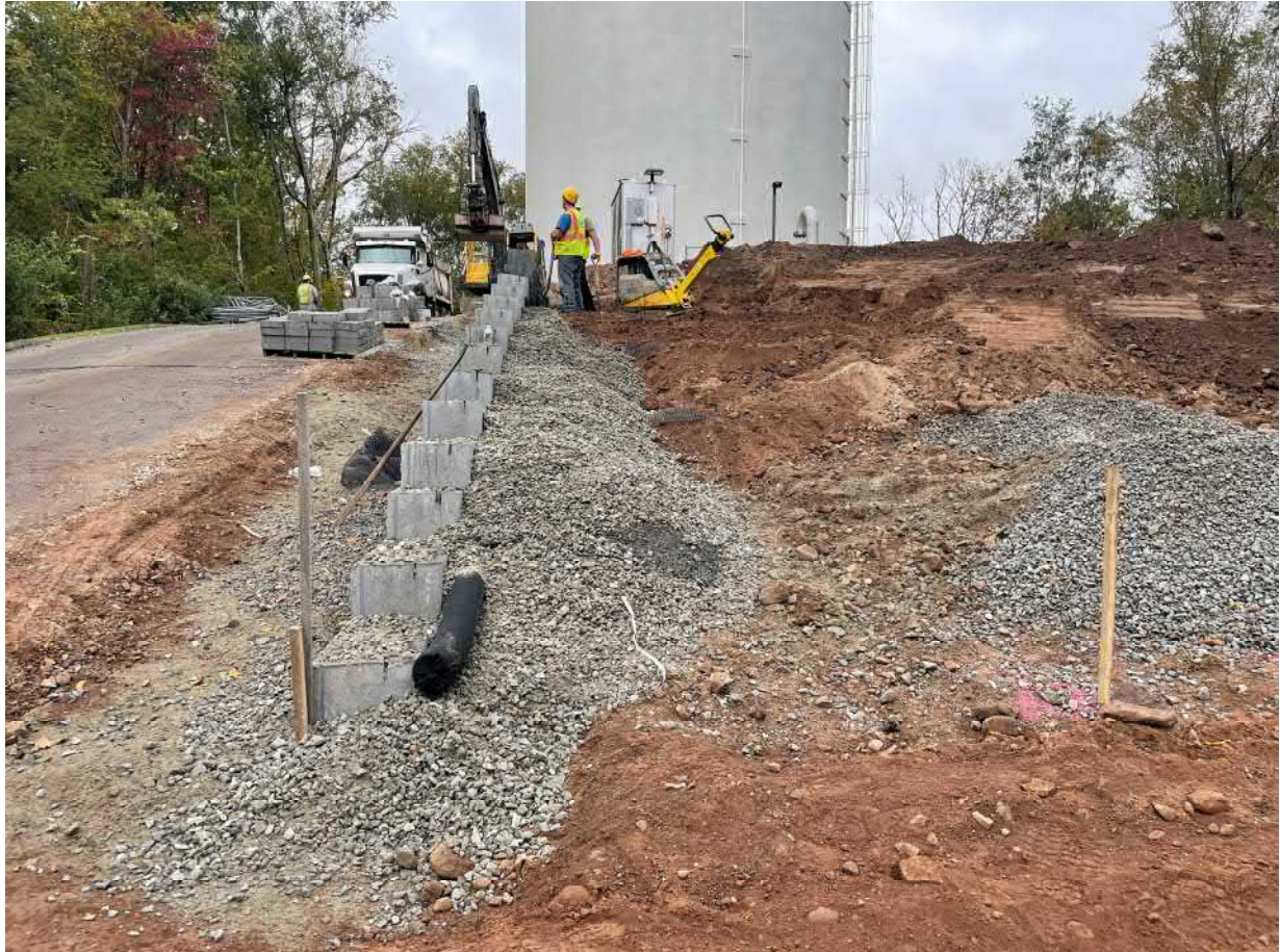
Picture 4: Ludlow 4" drainage pipe after Ludlow placed 3/4" stone over it on the south side of the retaining wall located between Stations 10+83 and 11+34. View to the east.
