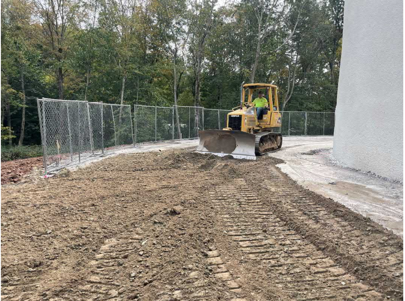
Picture 10: Ludlow grading 1.5" -minus gravel on the southeast side of the water tank. View to the southwest.
