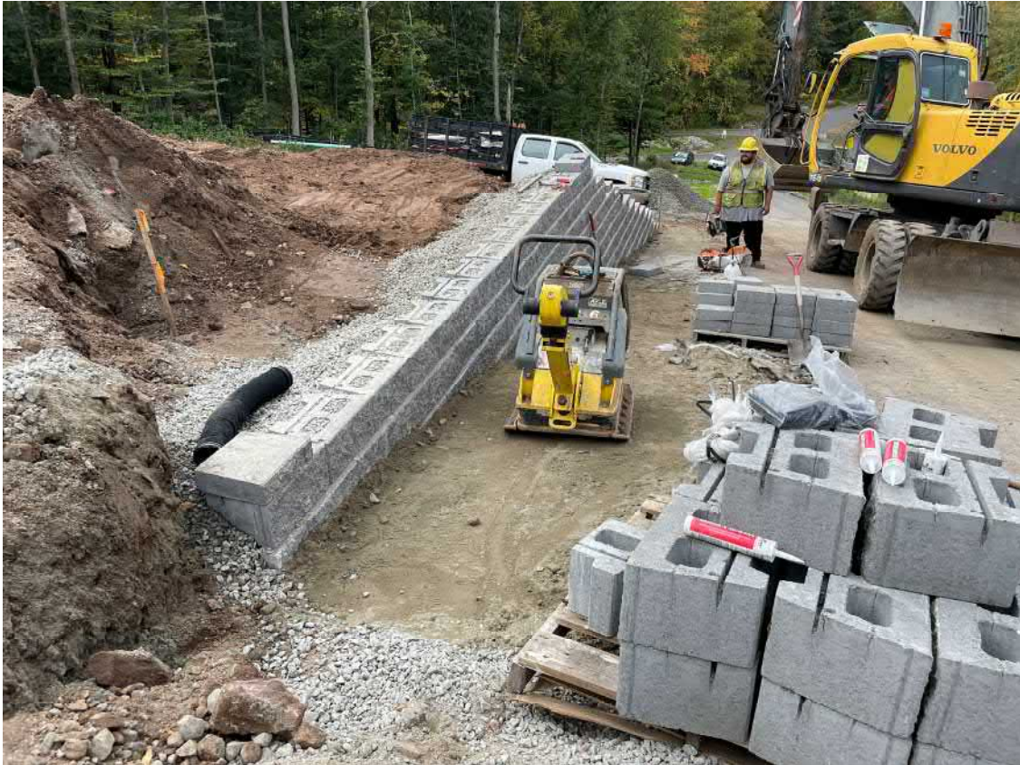
Picture 8: Ludlow used a plate compactor on the 1.5" -minus gravel they placed on the north side of the retaining wall they constructed between Stations 10+83 and 11+34. View to west.
