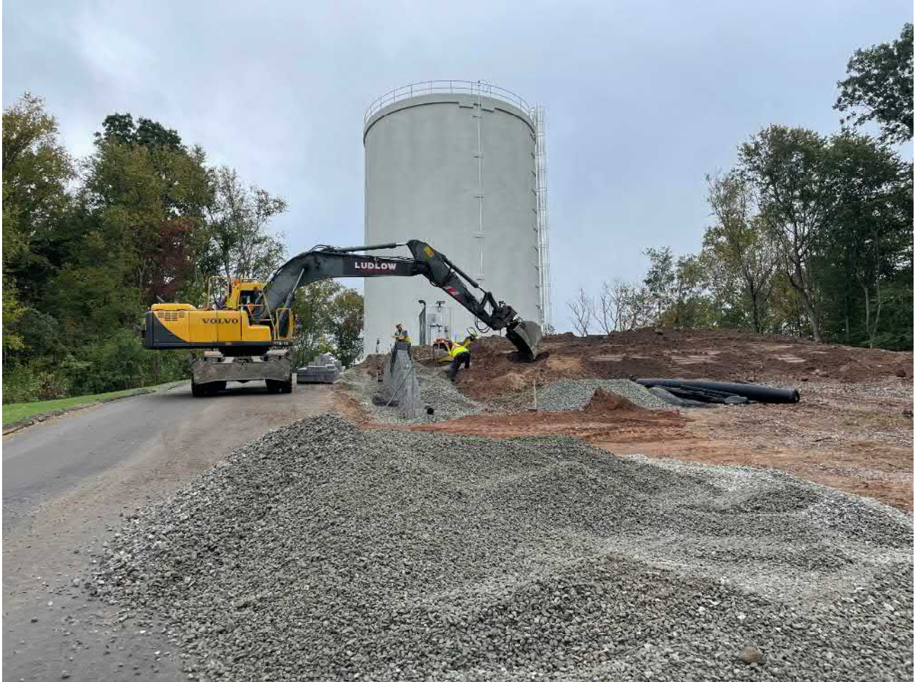
Picture 3: Ludlow placing \frac{3}{4} " stone over the 4" drainage pipe they just installed on the south side of the retaining wall located between Stations 10+83 and 11+34. View to the east.
