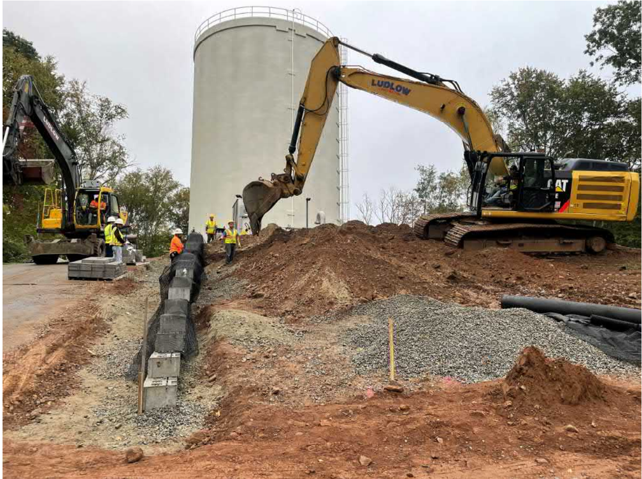
Picture 1: Ludlow pulling back fill on the south side of the retaining wall located between Stations 10+83 and 11+34 in order to place \frac{3}{4} " stone and a 4" drain pipe. View to east.
