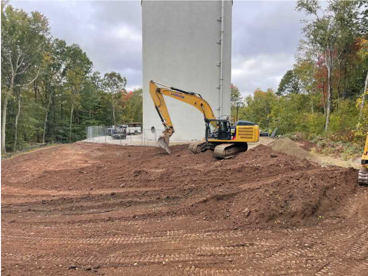
Picture 5: Ludlow performing earth work on the east side of the water tank, shaping the slope. View to the west.
