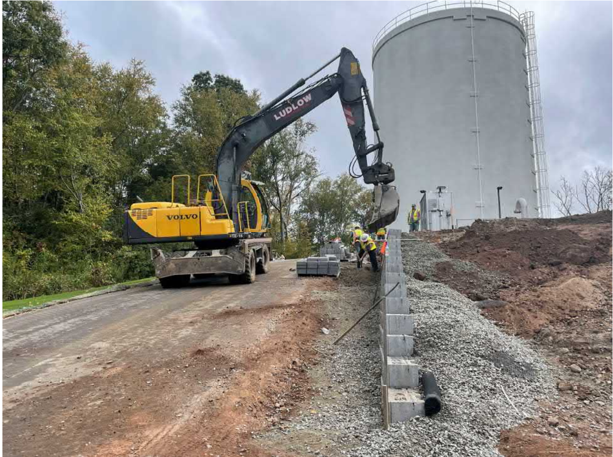
Picture 6: Ludlow placing 1.5" minus gravel on the north side of the retaining wall located between Stations 10+83 and 11+34. View to the east.
