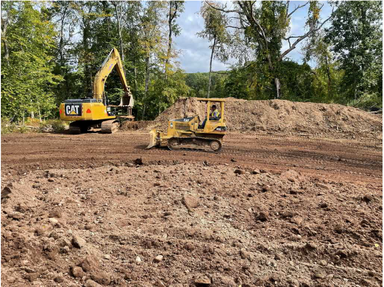
Picture 7: Picture 5: Ludlow performing earth work on the east side of the water tank, shaping the area just east of the toe of the slope. View to the east.
