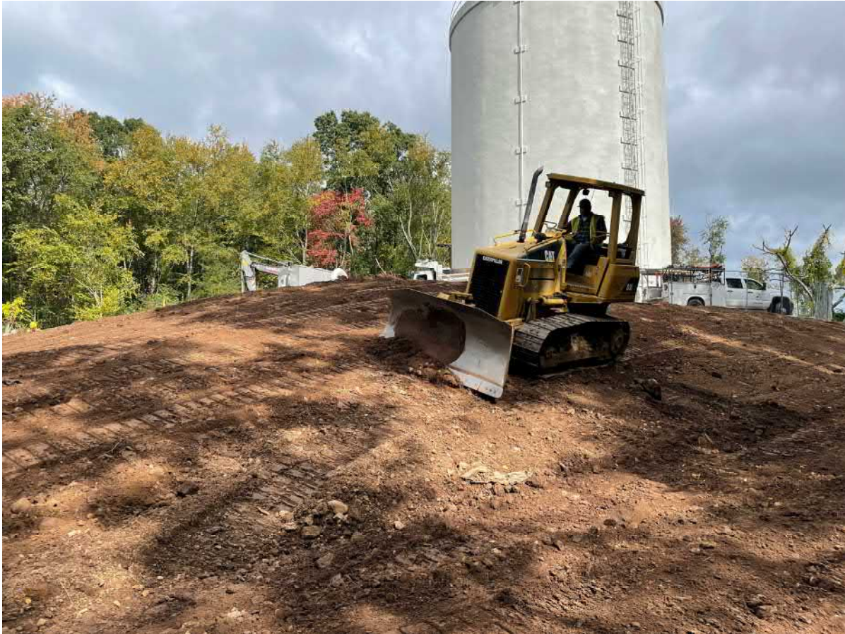
Picture 9: Ludlow grading fill on the southwest side of the water tank. View to the northeast.
