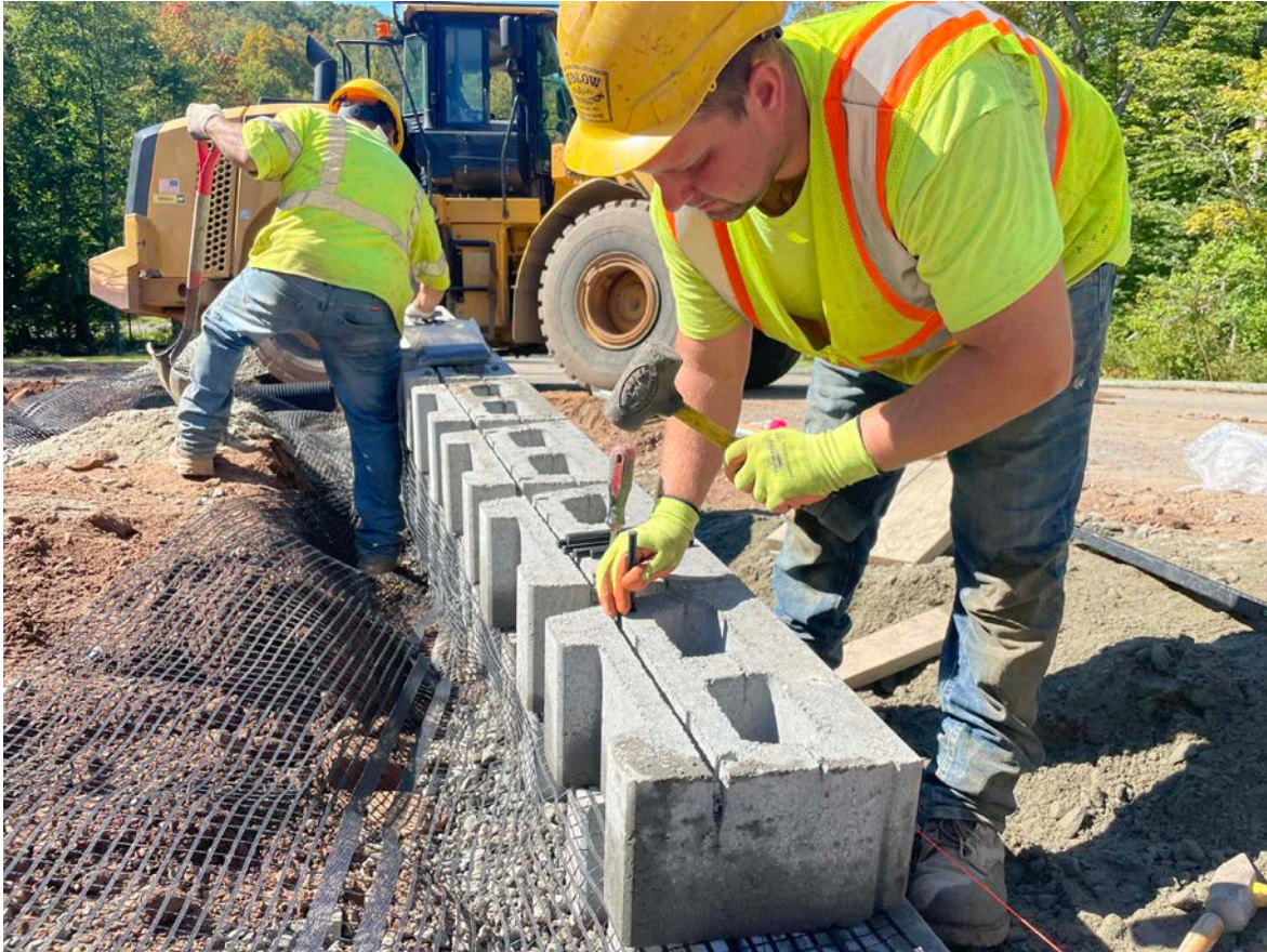
Picture 6: Ludlow securing VERSA-LOK blocks together with plastic pins as they construct a retaining wall on the south side of the Shared Access Driveway between Stations 10+83 and 11+34. View to the west.
