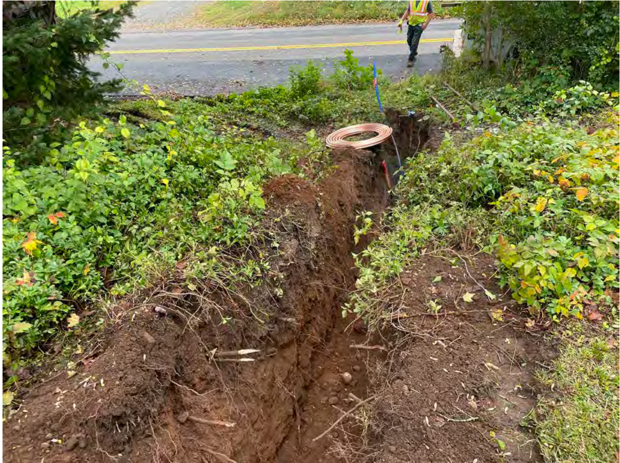
Picture 5: Trench that Ludlow excavated at the 36 Maiden Lane property for the installation of a 1” copper water service line. View to the south.
