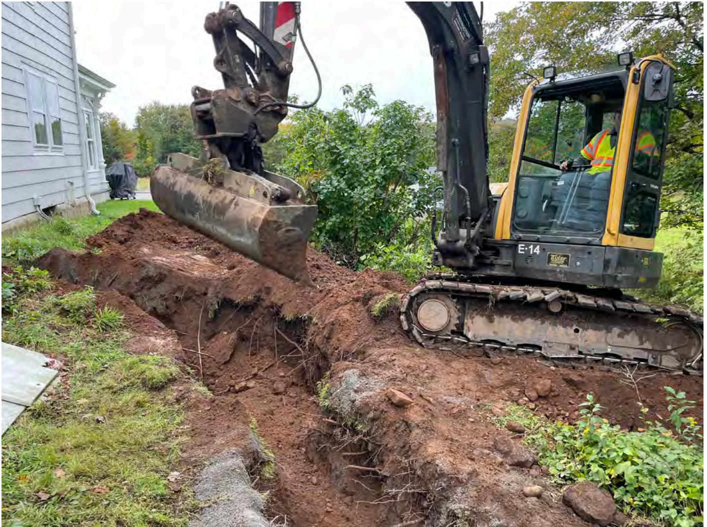
Picture 10: Ludlow placing native fill over the 6" of sand they placed over a 1" copper water service line they installed at the 36 Maiden Lane property. View to the north.
