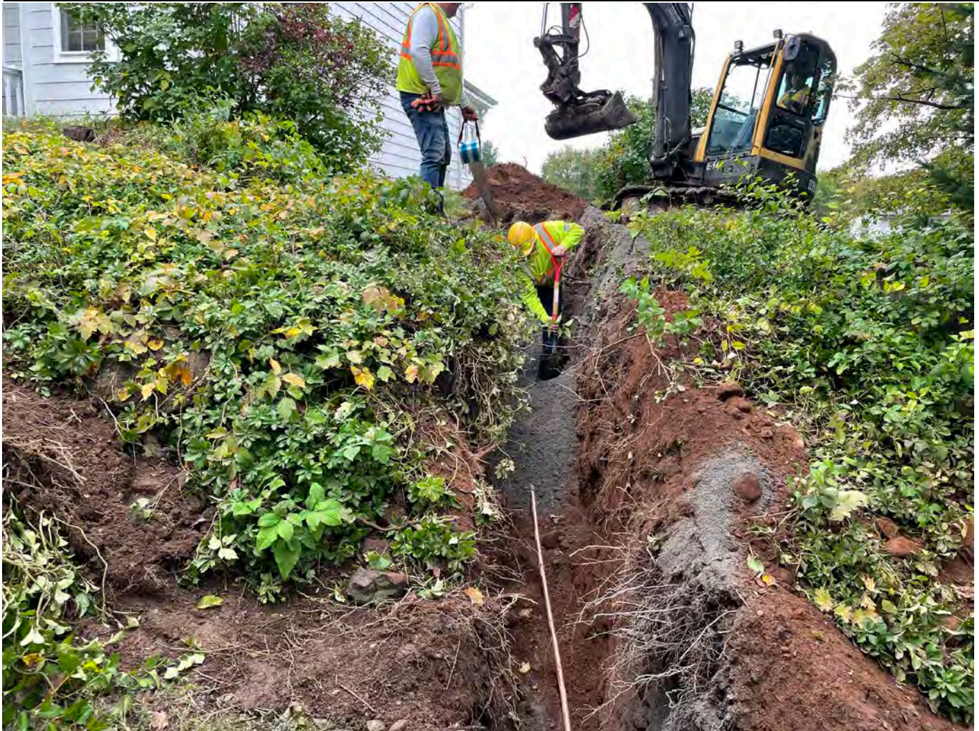
Picture 9: Ludlow placing sand bedding and warning tape over the 1" water service at the 36 Maiden Lane property. View to the north.
