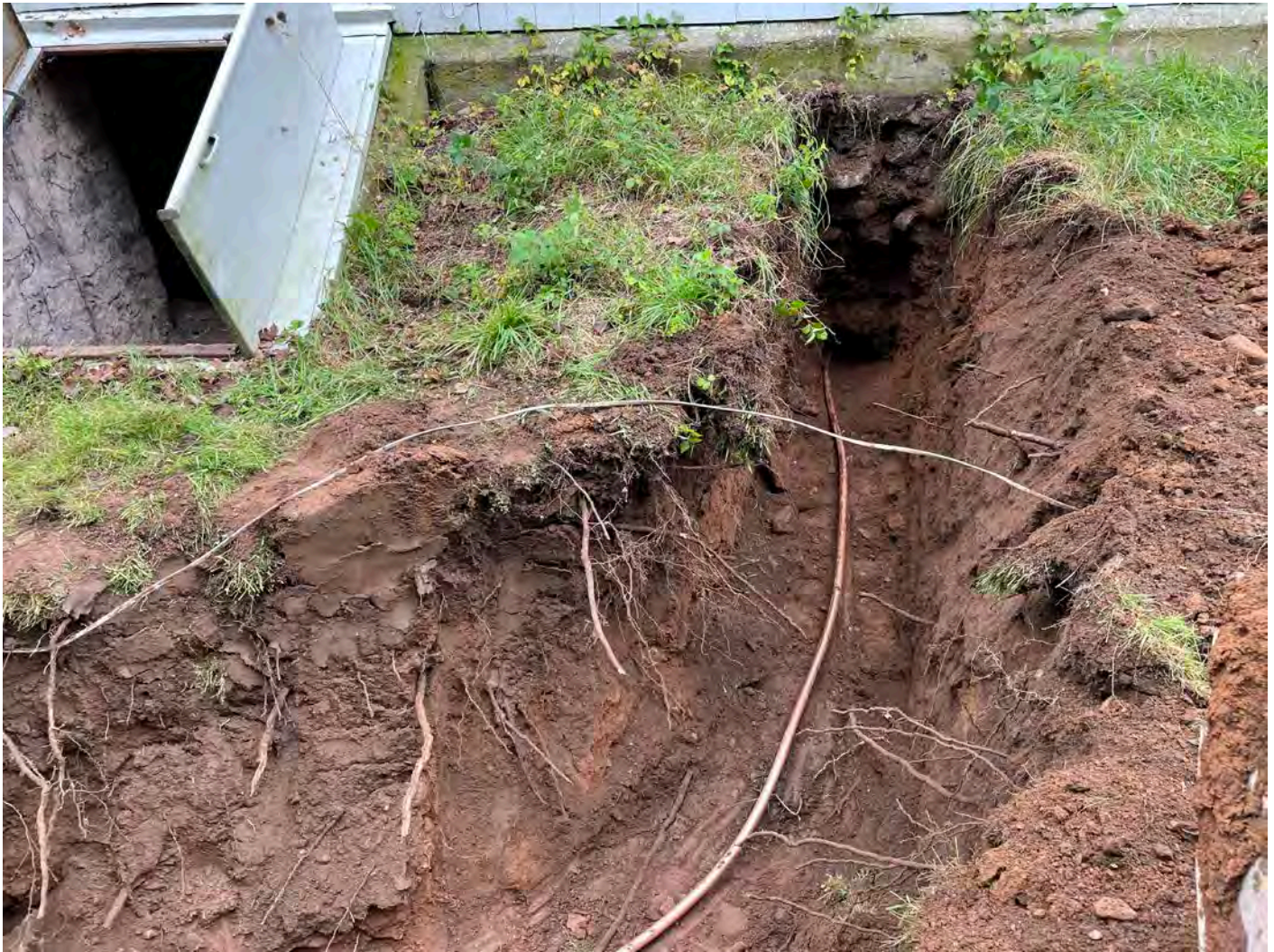
Picture 7: 1" copper water service line that Ludlow has passed through the eastern foundation wall of the 36 Maiden Lane residence. View to the west.
