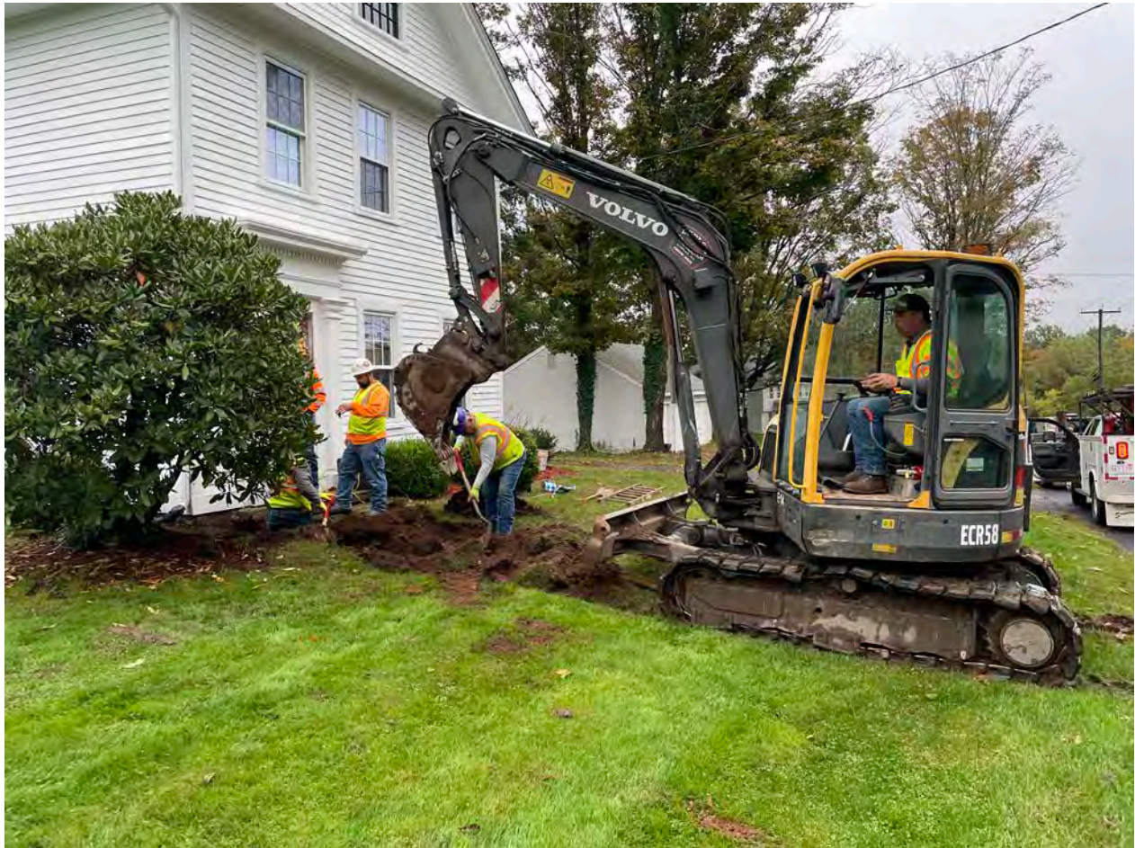
Picture 1: Ludlow excavating a trench at the 24 Maiden Lane property for the installation of a 1" copper water service line. View to the east.
