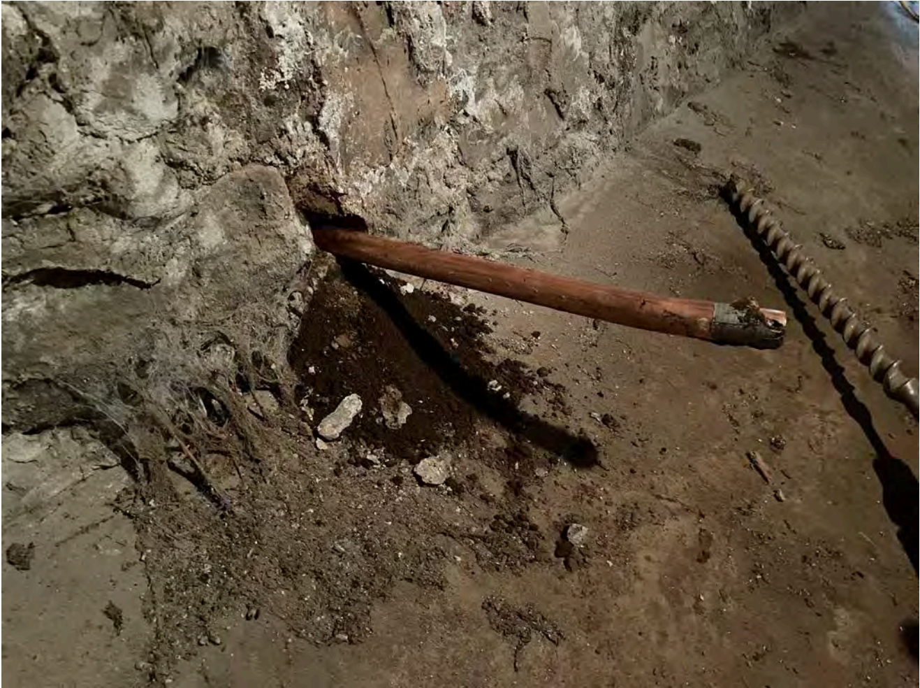
Picture 8: 1" copper water service line that Ludlow brought into the 36 Maiden Lane residence through eastern foundation wall. View to the south.
