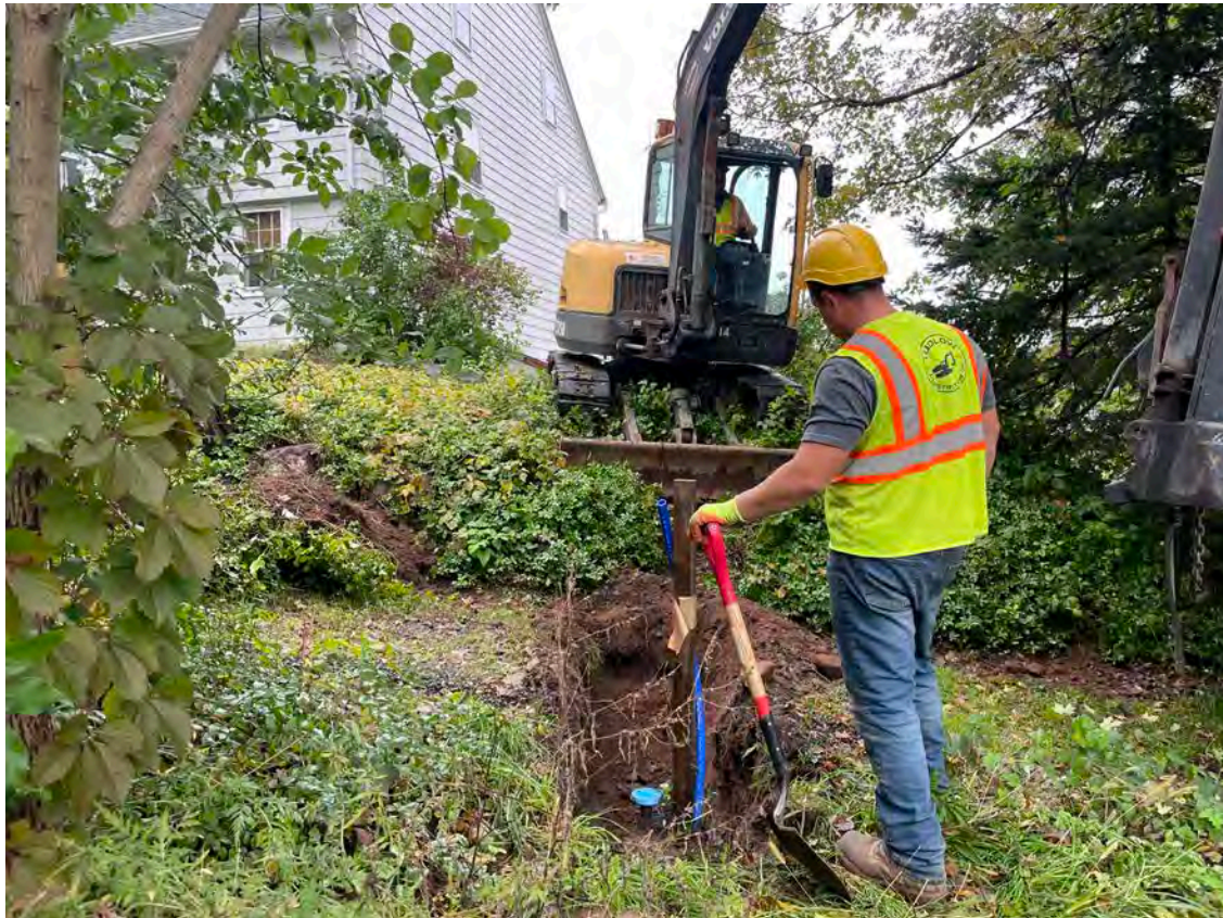
Picture 3: Ludlow beginning to excavate a trench at the 36 Maiden Lane property for the installation of a 1” copper water service line. View to the north.
