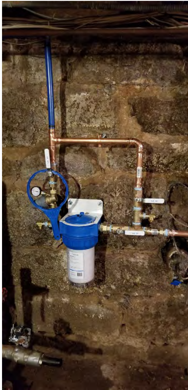
Picture 11: Final water service components that Fazzino Plumbing installed at the 308 Main Street, Durham, residence.
