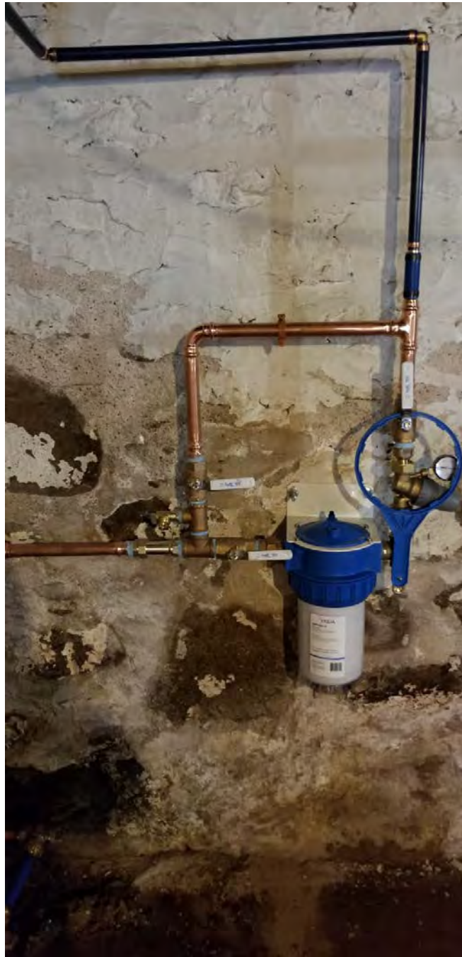
Picture 12: Final water service components that Fazzino Plumbing installed at the 316 Main Street, Durham, residence.
