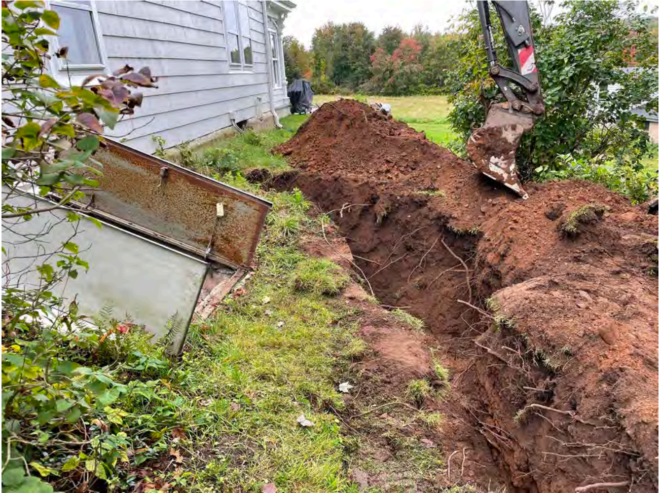
Picture 4: Trench that Ludlow excavated at the 36 Maiden Lane property for the installation of a 1" copper water service line. View to the north.
