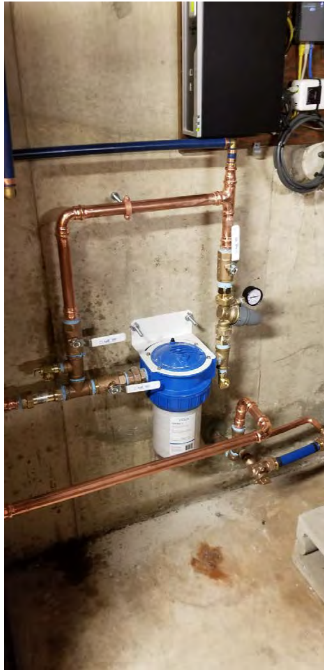
Picture 13: Final water service components that Fazzino Plumbing installed at the 321 Main Street, Durham, residence.
