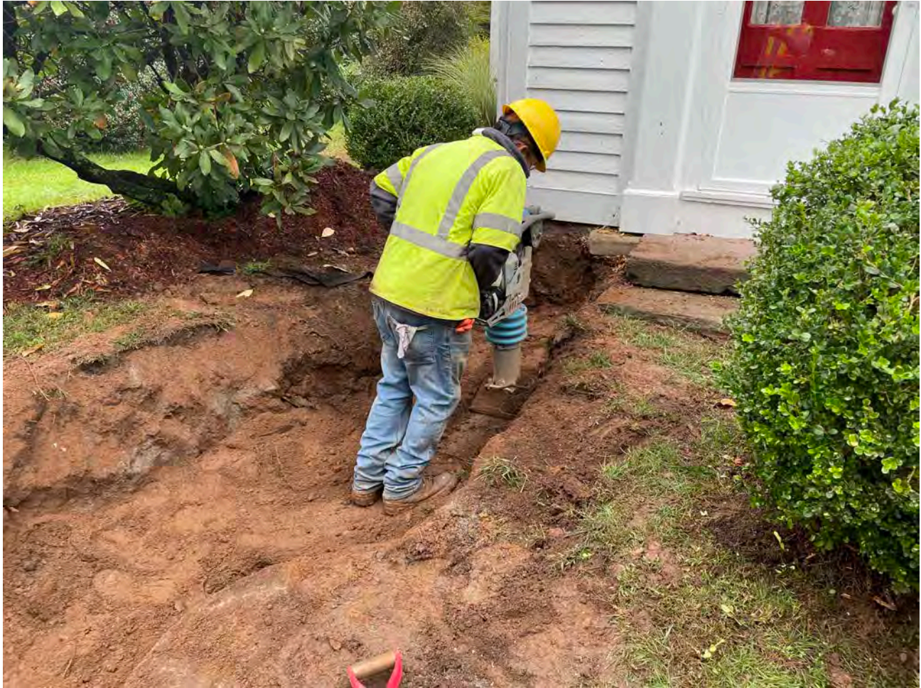
Picture 2: Ludlow compacting fill with a jumping jack compactor in the trench that Ludlow excavated at the 24 Maiden Lane property for the installation of a 1" copper water service line. View to the northwest.
