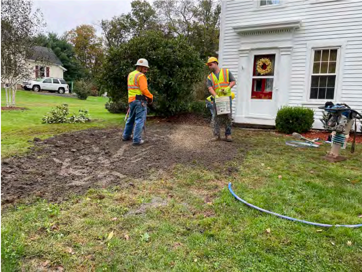
Picture 6: Ludlow spreading grass seed on a portion of the lawn of the 24 Maiden Lane residence that was disturbed during the installation of a 1" copper water service line. View to the northwest.
