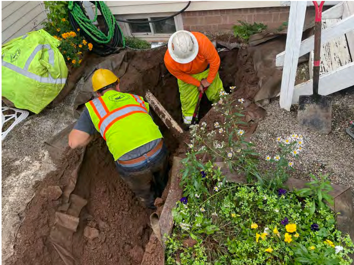
Picture 3: Ludlow hand excavating around a 4" PVC drain line located on the west side of the 18 Maiden Lane residence in Durham. View to the east.
