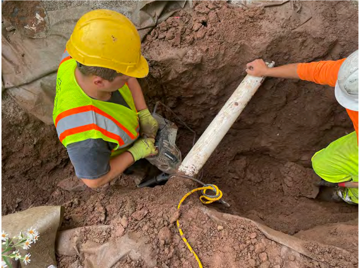
Picture 5: Ludlow jackhammering bedrock in the trench they excavated for the installation of a 1" copper water service line. View to the west.
