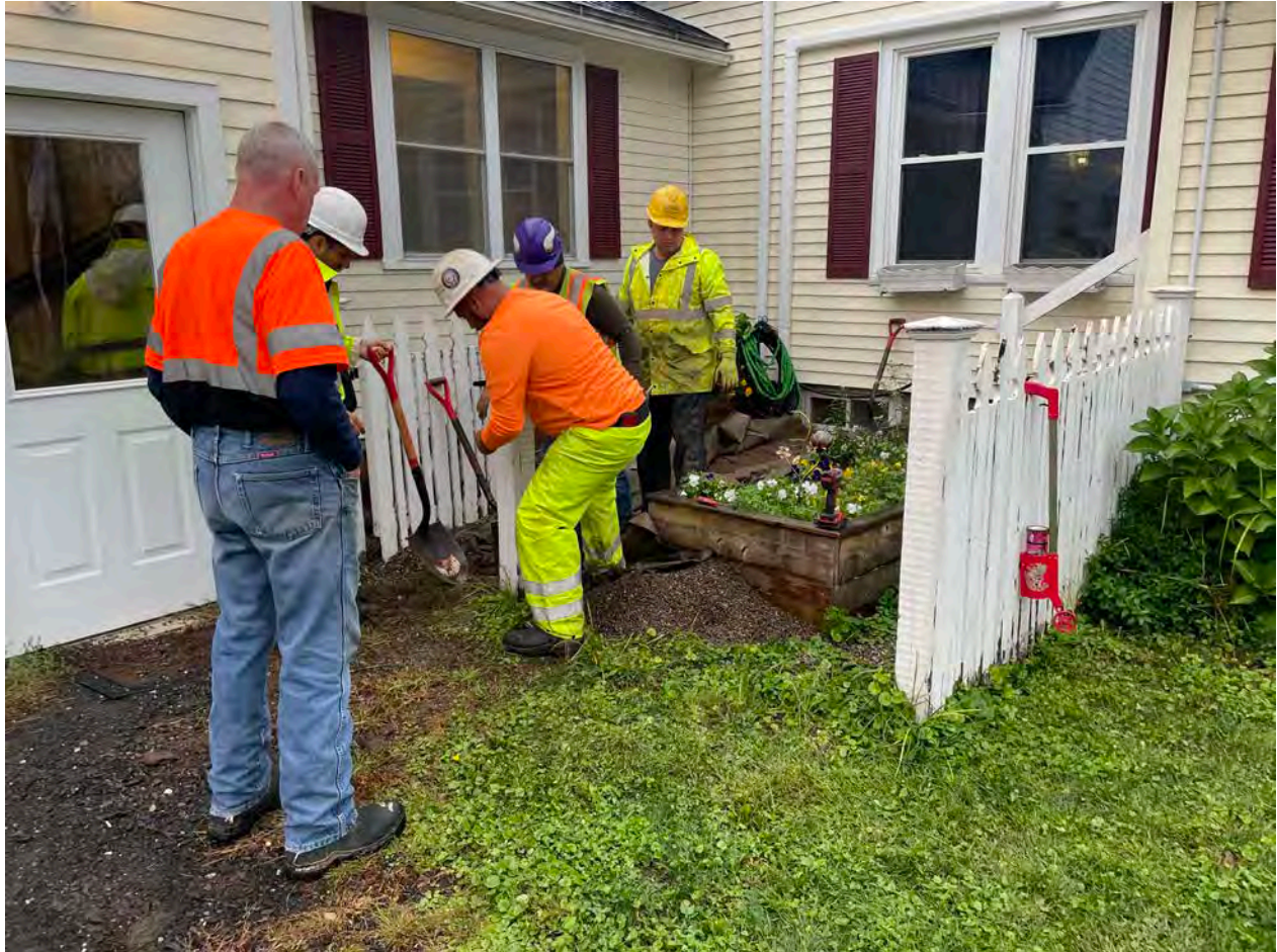
Picture 1: Ludlow removing a section of fence at the 18 Maiden Lane property that was in the pathway of the new route they chose to install a 1" copper water service line. The original route (which had the pipe entering the house on the south side next to the southwest corner) was deemed infeasible, as the entry point led into a section of the house that is not underlain by the home's basement. View of the west side of the house, looking to the northeast.
