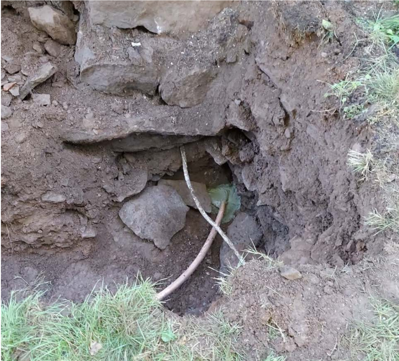
Picture 4: Ludlow drills the foundation for the 17 Maiden Lane residence for the 1" copper service line to enter the house through. The hole with the 1" copper tubing is sealed using hydraulic cement. View to the East.
