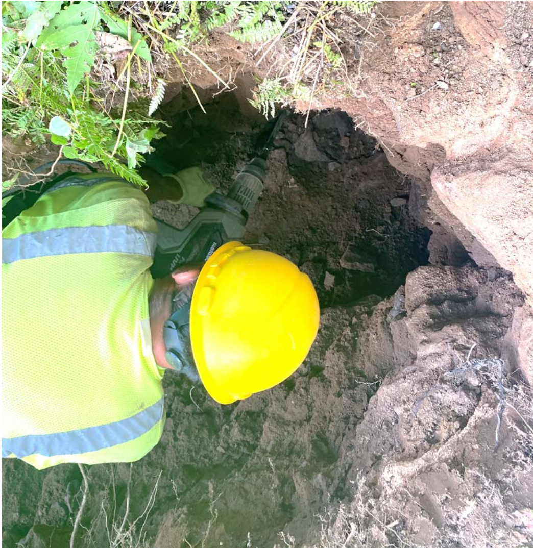
Picture 8: Ludlow drills an area of rock in the trench near the NW corner of the 19 Maiden Lane residence near the point of connection at the house. View to the South.
