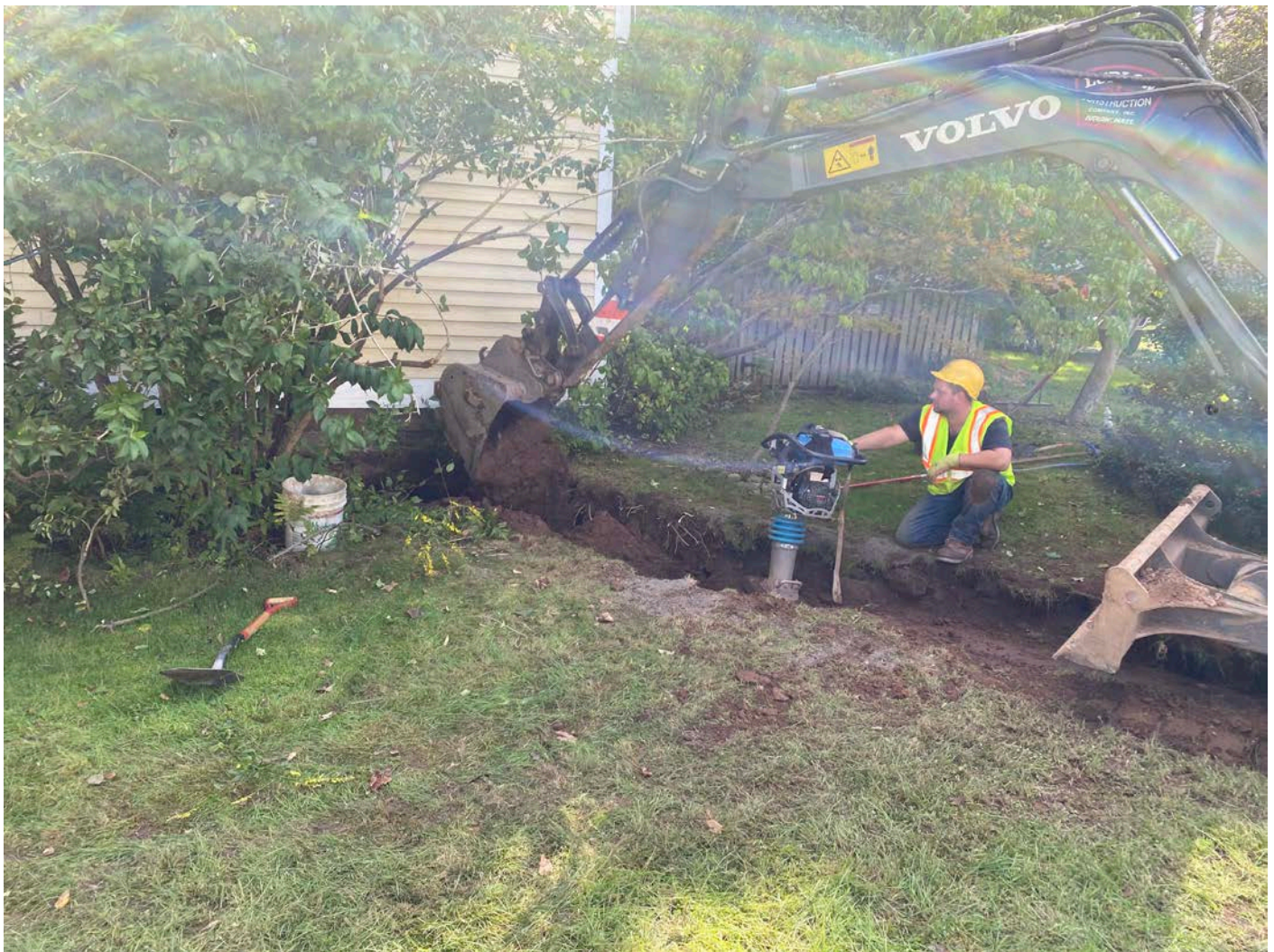
Picture 12: Ludlow compacts native fill that has been backfilled into the trench at the 19 Maiden Lane residence with a compactor. View to the South.
