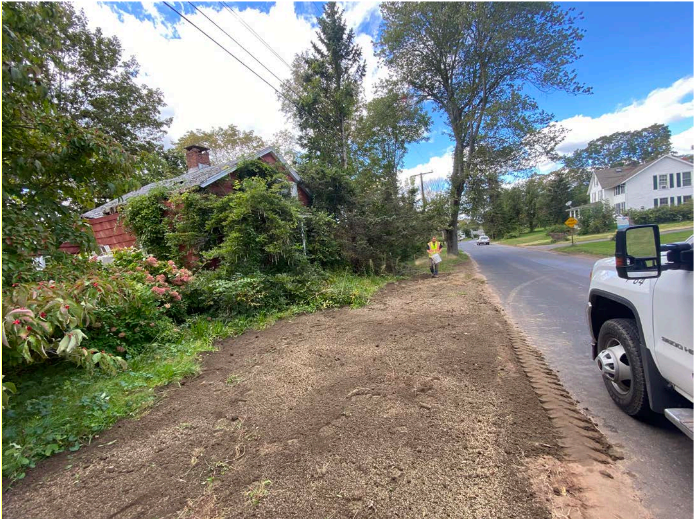
Picture 14: Ludlow restores the portions of the property that were disturbed during construction on the 126 Maple Avenue property in Durham CT. Ludlow places seed and hay mats over area for restoration. View to the Northwest.
