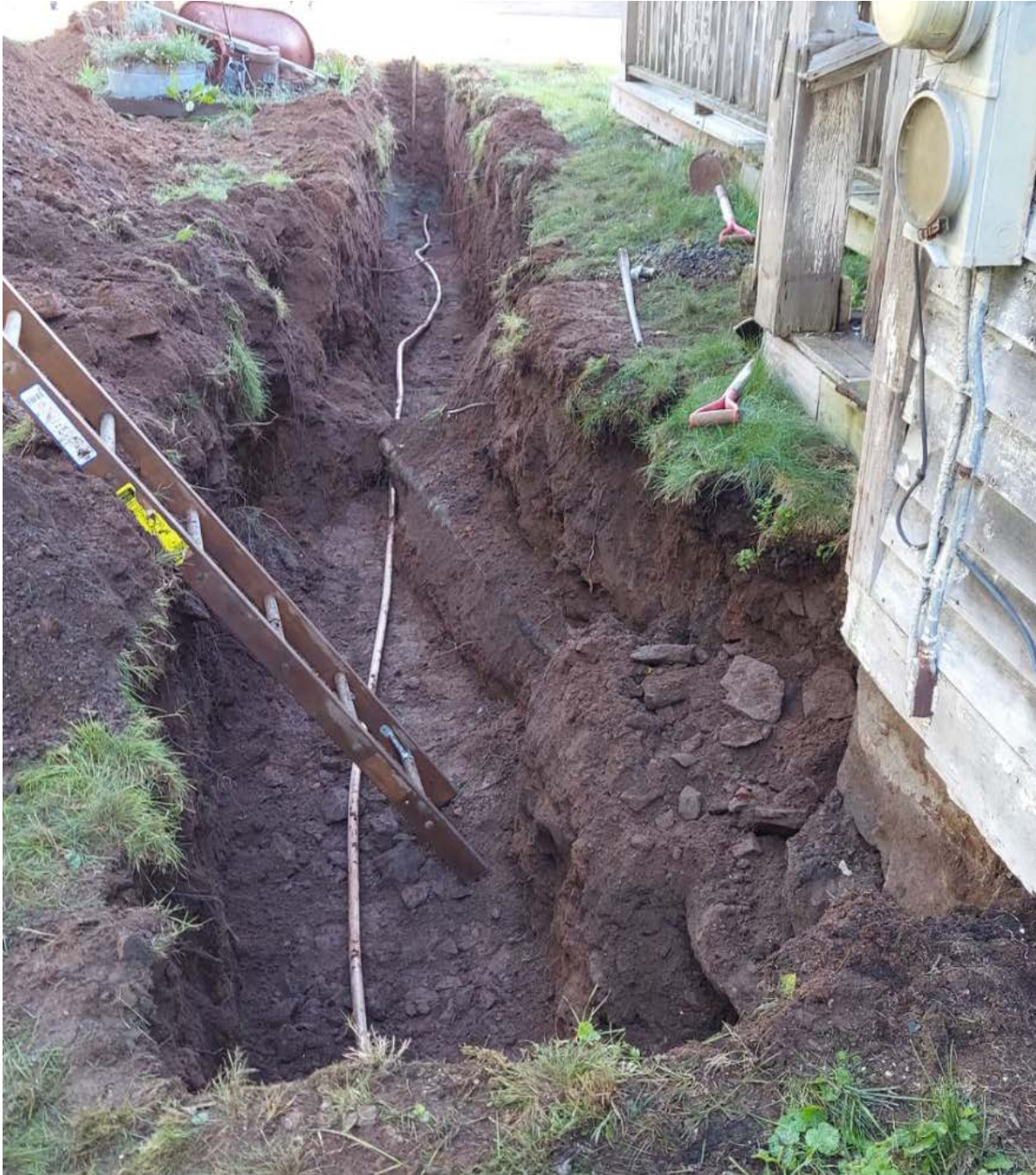
Picture 3: Ludlow places 1" copper tubing in trench for the service connection for the 17 Maiden Lane residence. View to the North.
