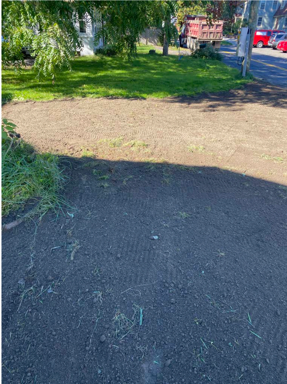
Picture 6: Ludlow grades the compacted backfill and places loam and seed on the surface over the trench for the 1" copper service line at the 17 Maiden Lane residence. View to the West.
