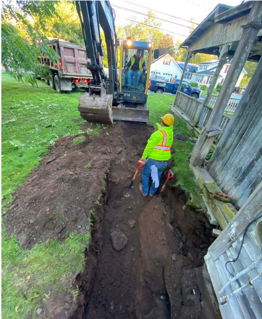
Picture 1: Ludlow excavates a trench for the 1" copper service line down the West side of the house for the 17 Maiden Lane residence in Durham, CT.
