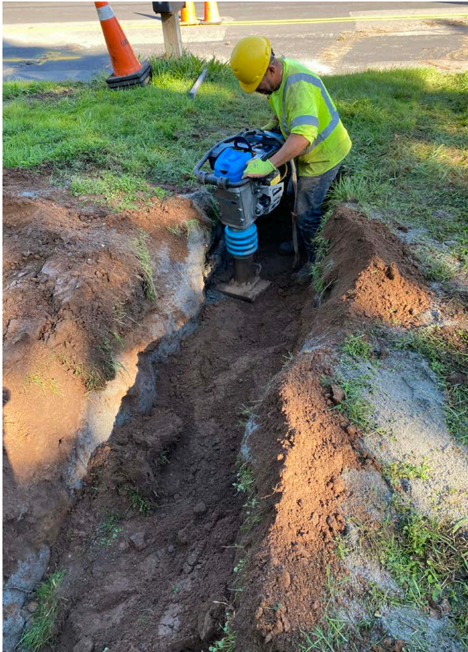
Picture 5: Ludlow compacts native fill that has been backfilled into the trench at the 17 Maiden Lane residence with a jumping jack compactor. View to the North.
