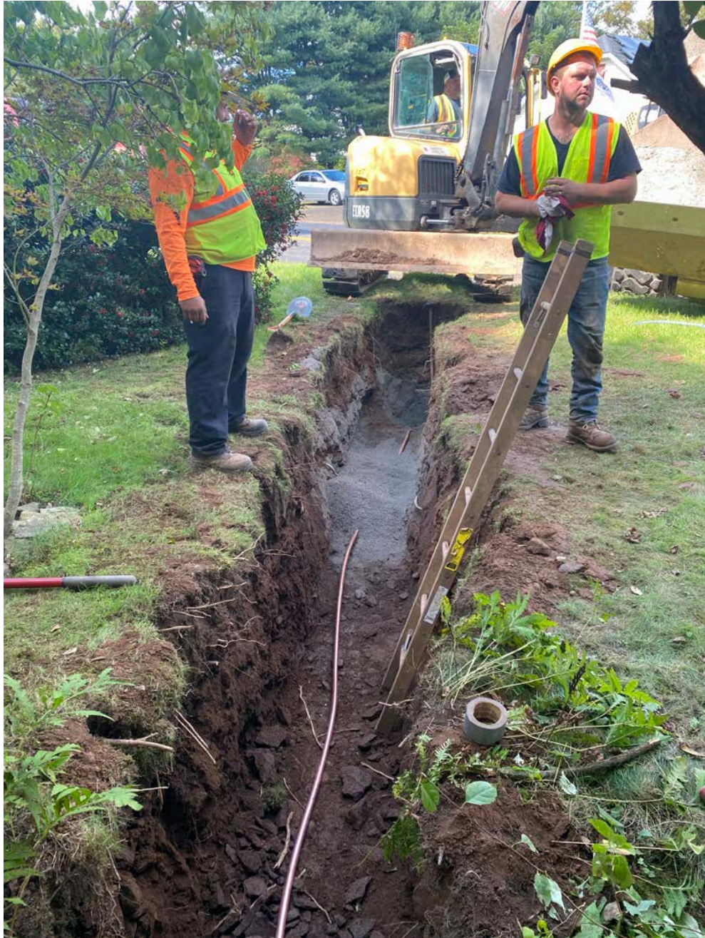
Picture 9: Ludlow places 1" copper tubing in trench for the service connection for the 19 Maiden Lane residence. View to the North.
