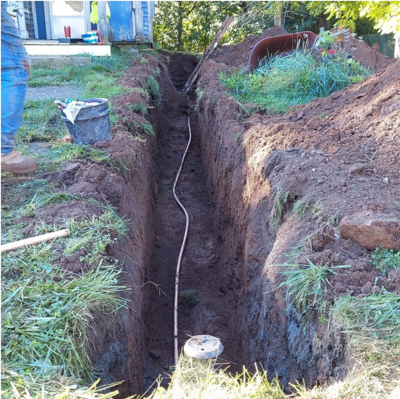
Picture 2: Ludlow places 1" copper tubing in trench for the service connection for the 17 Maiden Lane residence. View to the South.
