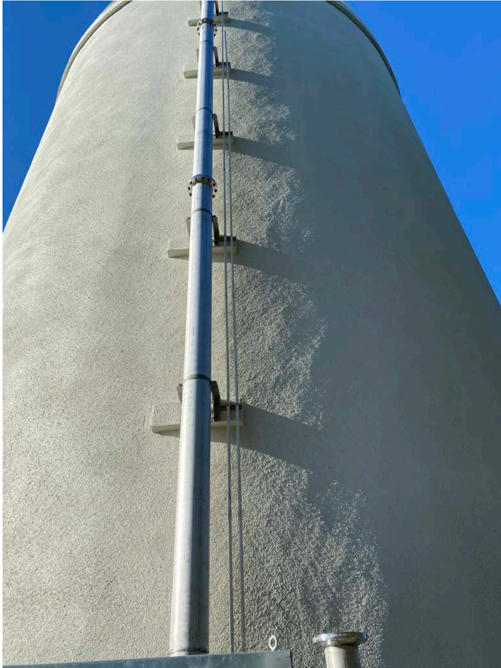
Picture 15: A & R Electric ran electric lines through conduit up the North side of the water tank on Talcott Ridge Drive.
