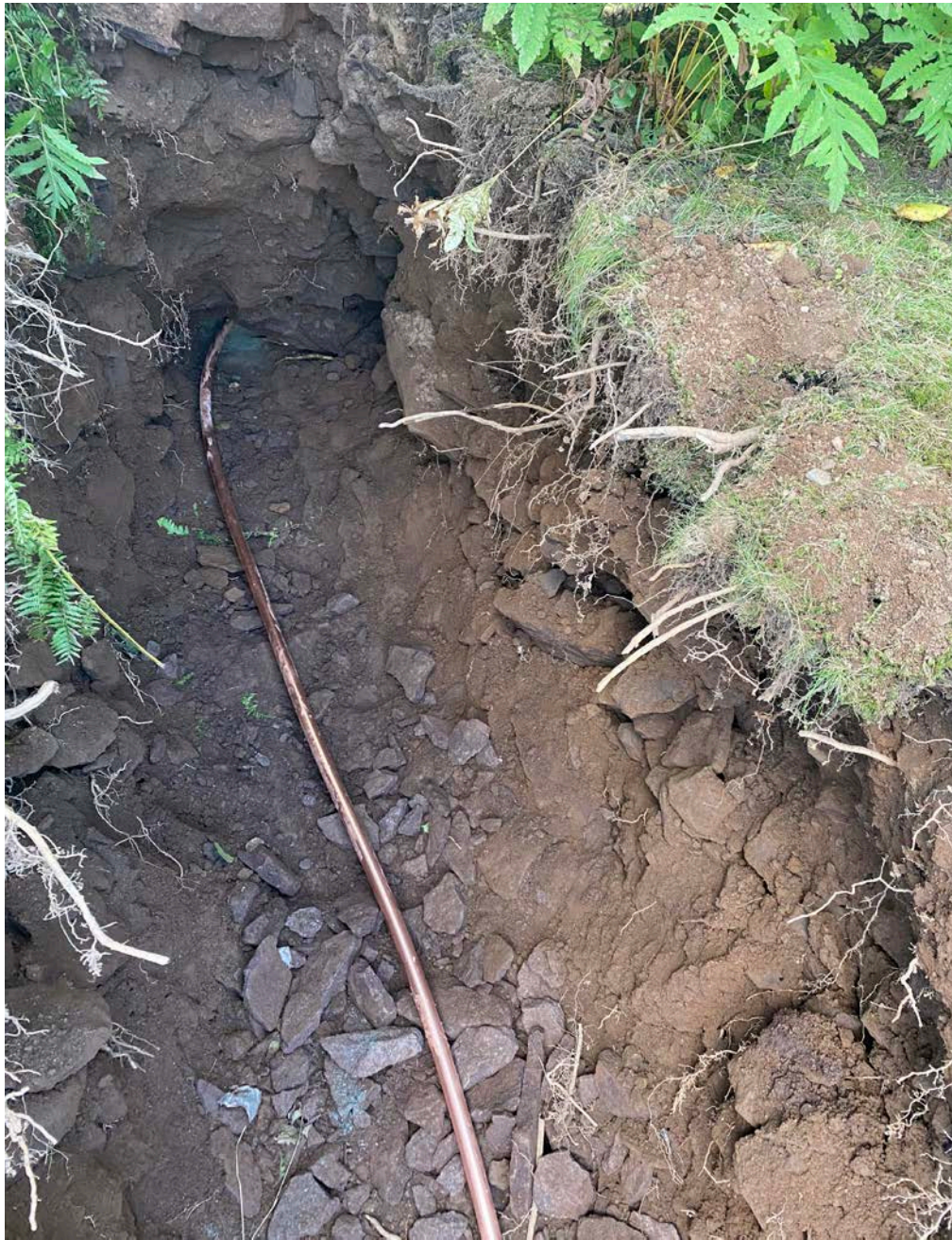
Picture 11: Ludlow installed the 1" copper service line to enter the house at 19 Maiden Lane. The hole with the 1" copper tubing is sealed using hydraulic cement. View to the South.
