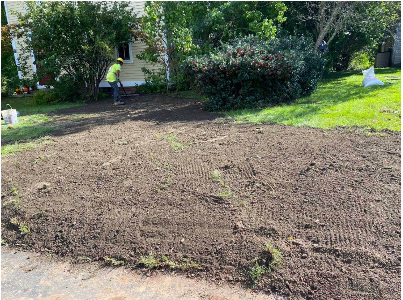
Picture 13: Ludlow grades the compacted backfill and places loam and seed on the surface over the trench for the 1” copper service line at the 19 Maiden Lane residence. View to the South.
