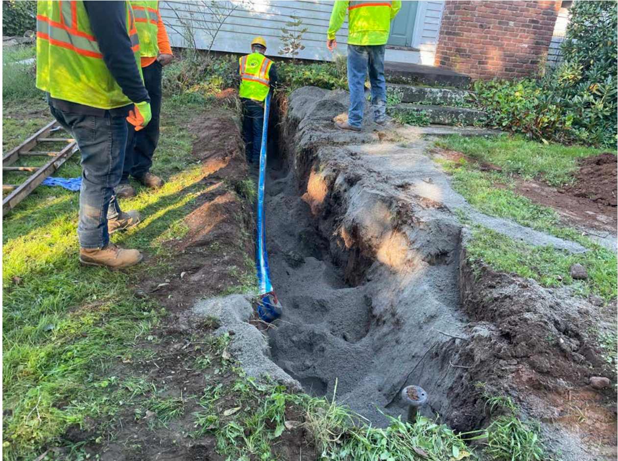
Picture 1: Ludlow placing caution tape over sand that was placed on top of 1" copper water service line at the 110 Maple Avenue residence in Durham. View to the west.
