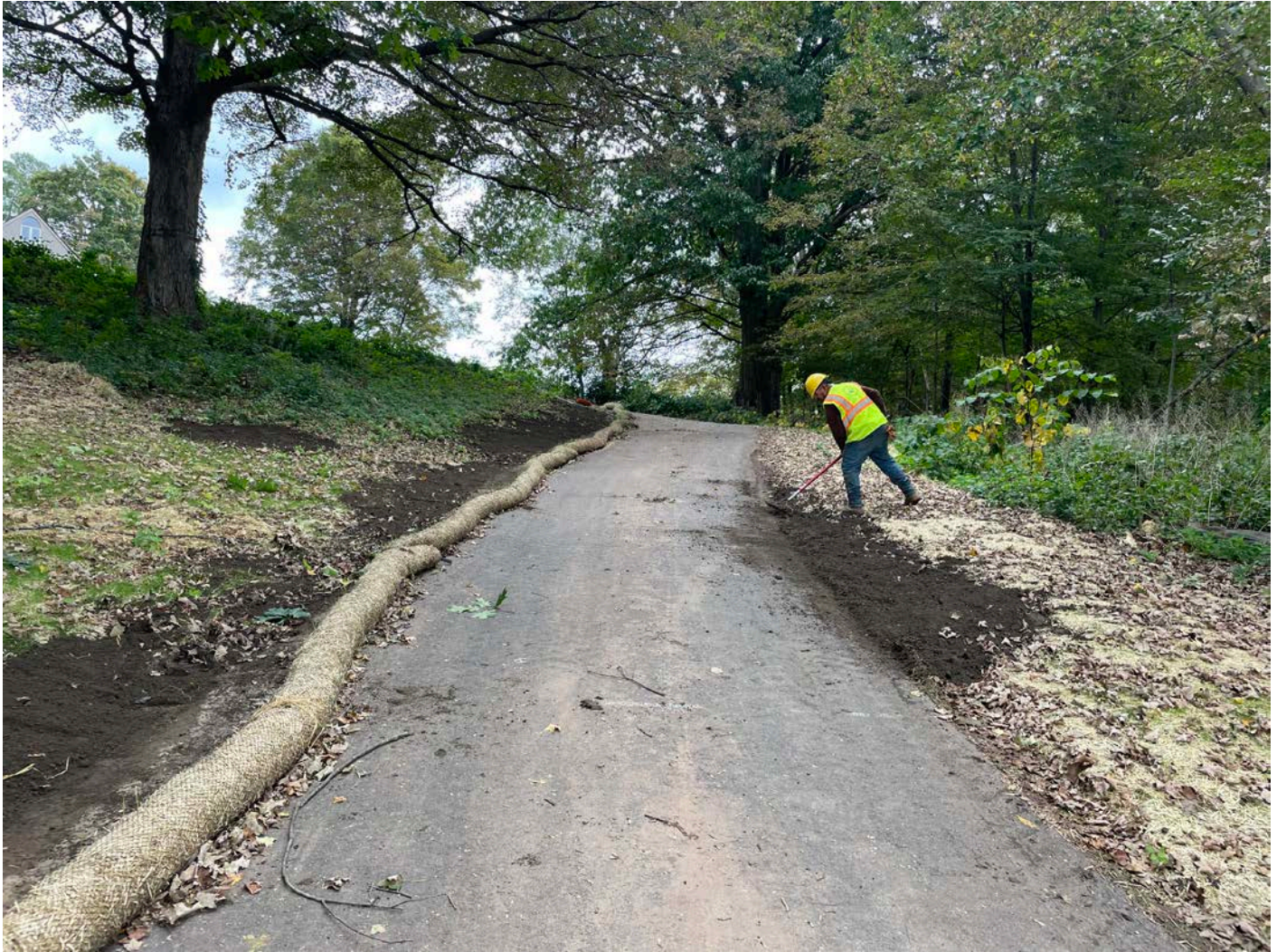
Picture 10: Ludlow raking out loam that they placed on the south side of the driveway for the residence located at 95R Maple Avenue in Durham. View to the east.
