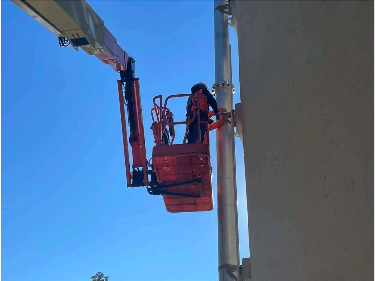
Picture 2: DN Tanks working on 12" air duct they installed on the northeast side of the water tank located east of the Shared Access Driveway in Middletown. View to the southeast.
