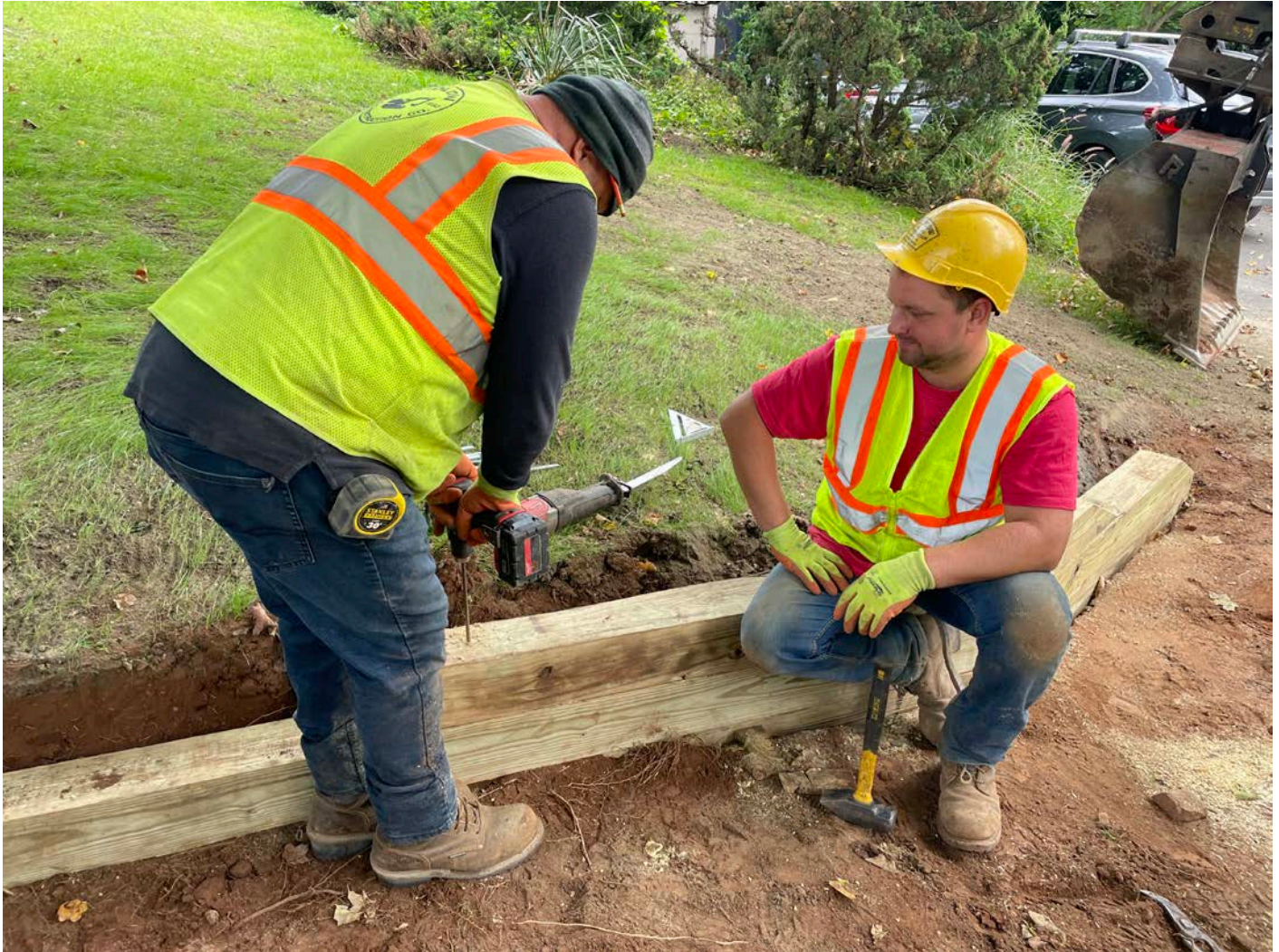
Picture 9: Ludlow building a short wooden retention wall on the east side of the driveway turnout at the 95R Maple Avenue property. View to the east.
