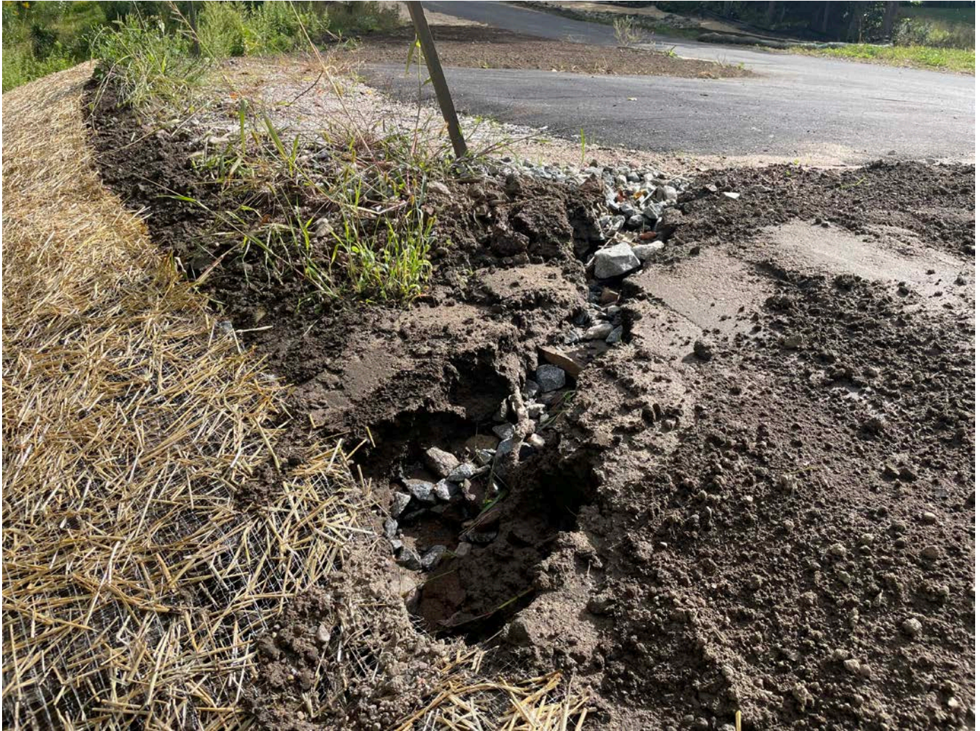
Picture 7: Erosion observed on the northwest corner of the turnout located at Station 14+00. View to the east.
