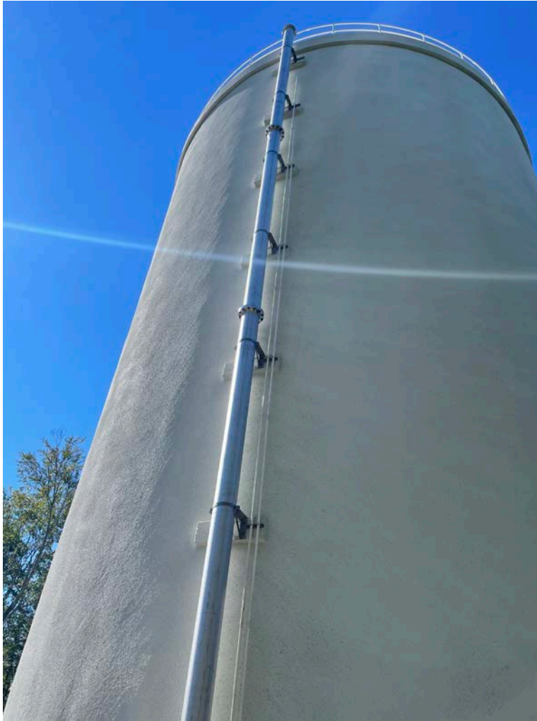
Picture 5: 1" conduit that DN Tanks installed on the west side of the 12" stainless steel air duct on the northeast side of the water tank located east of the Shared Access Driveway in Middletown. View to the south.
