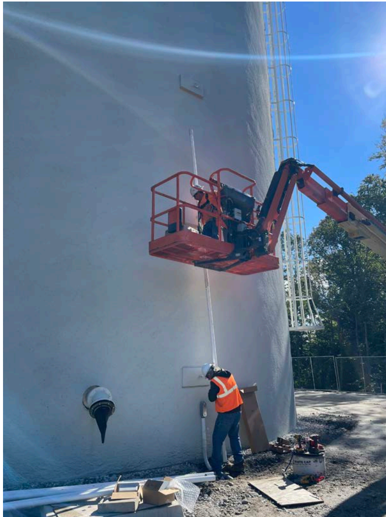
Picture 6: DN Tanks installing 2" conduit on the west side of the water tank located east of the Shared Access Driveway. View to the southeast.
