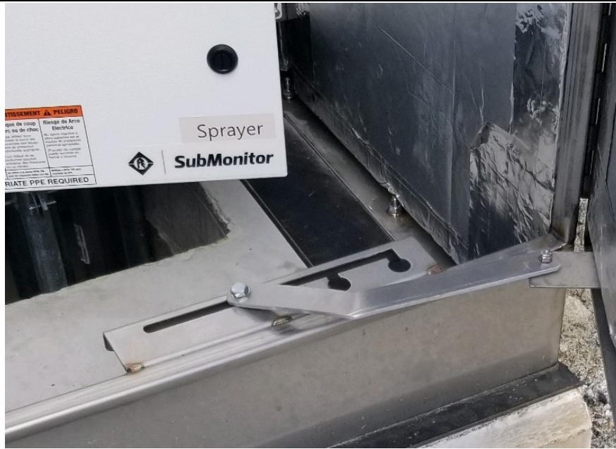
Picture 8: Bent arm observed on the electrical enclosure located north of the altitude vault. View to the northeast.
