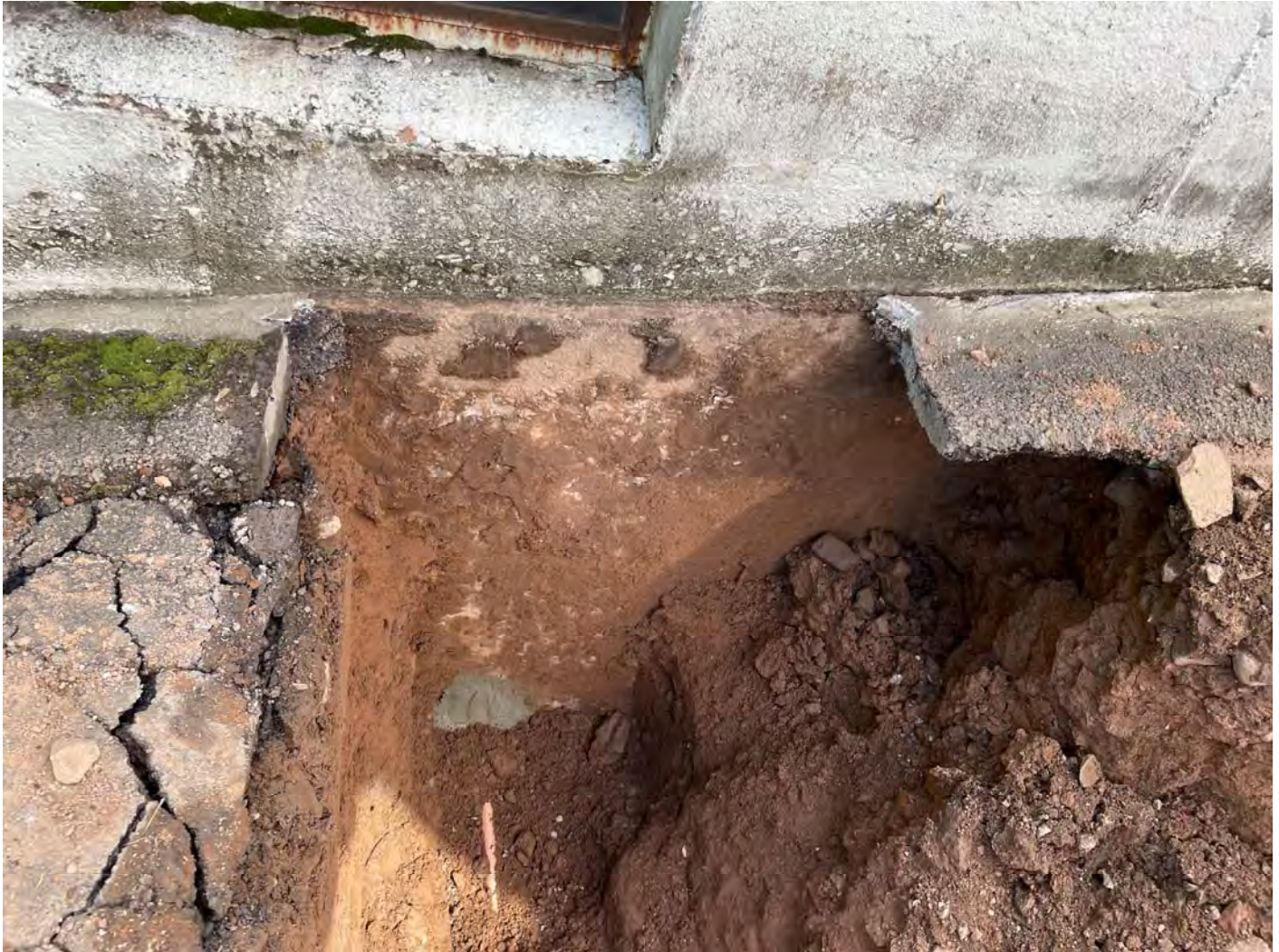
Picture 7: Poured concrete foundation that Ludlow has exposed on the north side of the 325 Main Street, Durham, building as they work to install a 1" copper water service line. View to the south.
