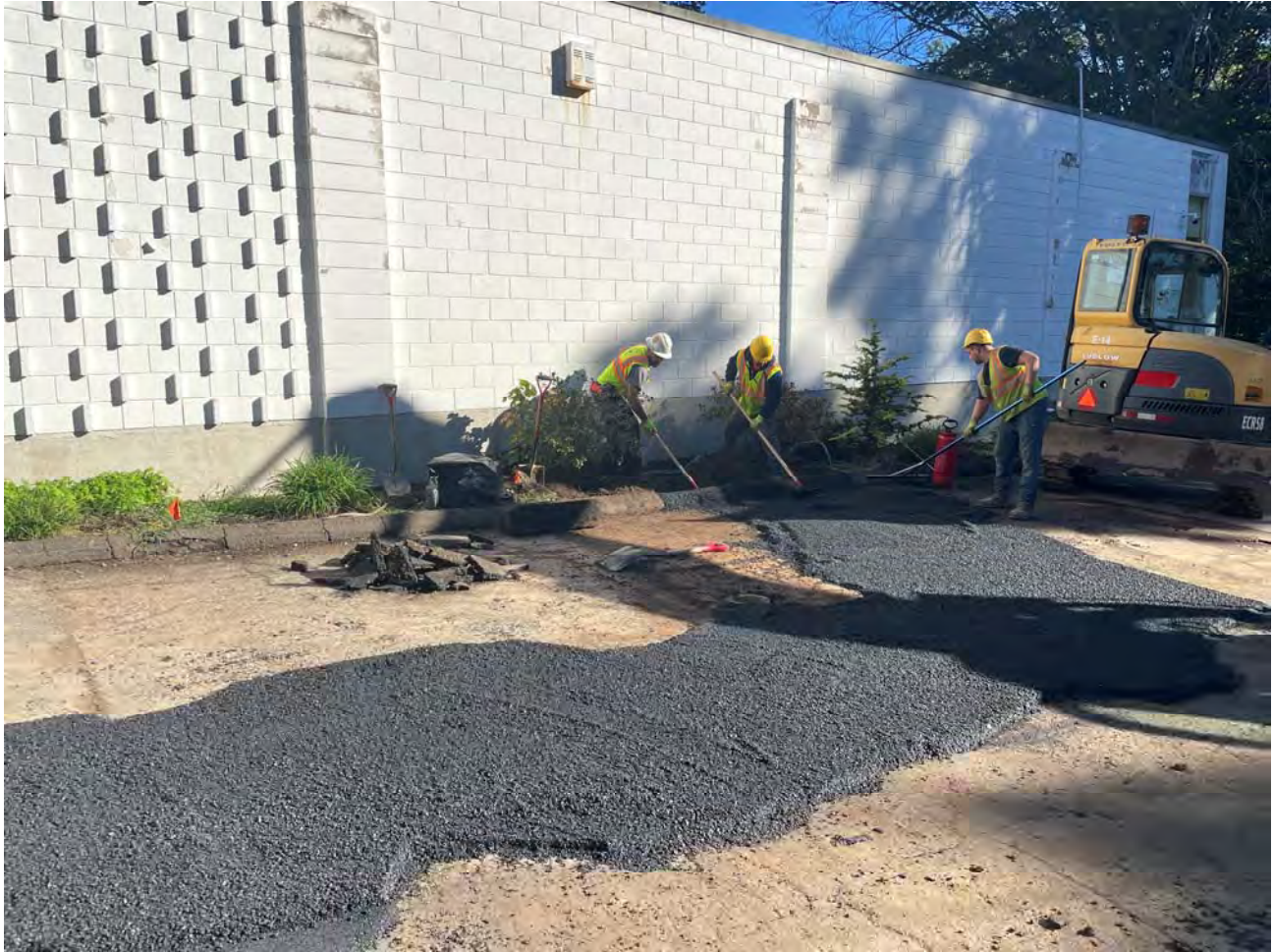
Picture 2: Ludlow raking out asphalt they placed on the south side of the 321 Main Street building over the trench they are backfilling after having installed a 1" copper water service line. View to the northeast.
