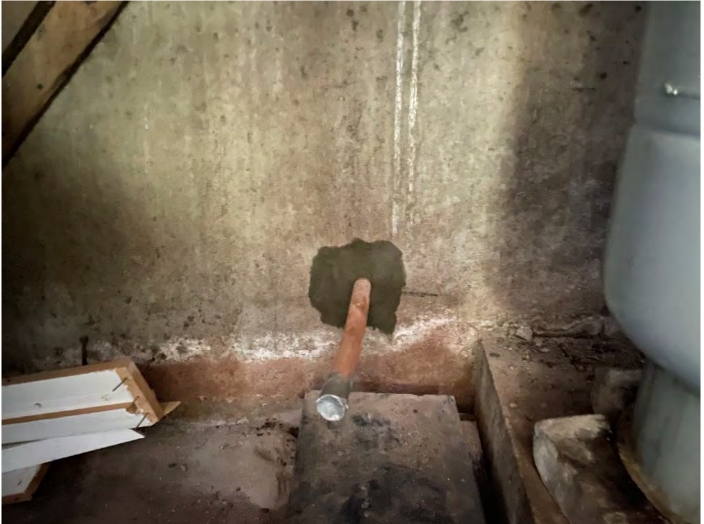
Picture 9: 1" copper water service line that Ludlow has installed through the northern foundation of the 325 Main Street building and has secured with non-shrink grout. View to the north.
