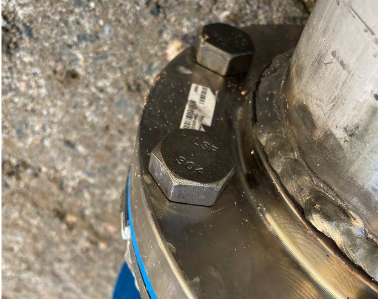
Picture 1: 304 stainless steel bolts used to connect sections of 12" stainless steel air duct piping on the northeast side of the water tank located east of the Shared Access Driveway.
