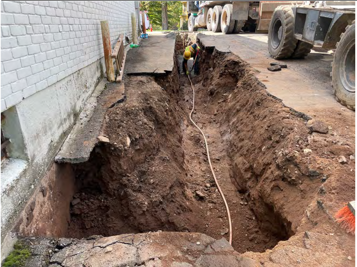
Picture 8: 1" copper water service line that Ludlow has installed on the north side of the 325 Main Street, Durham, building. View to the west.
