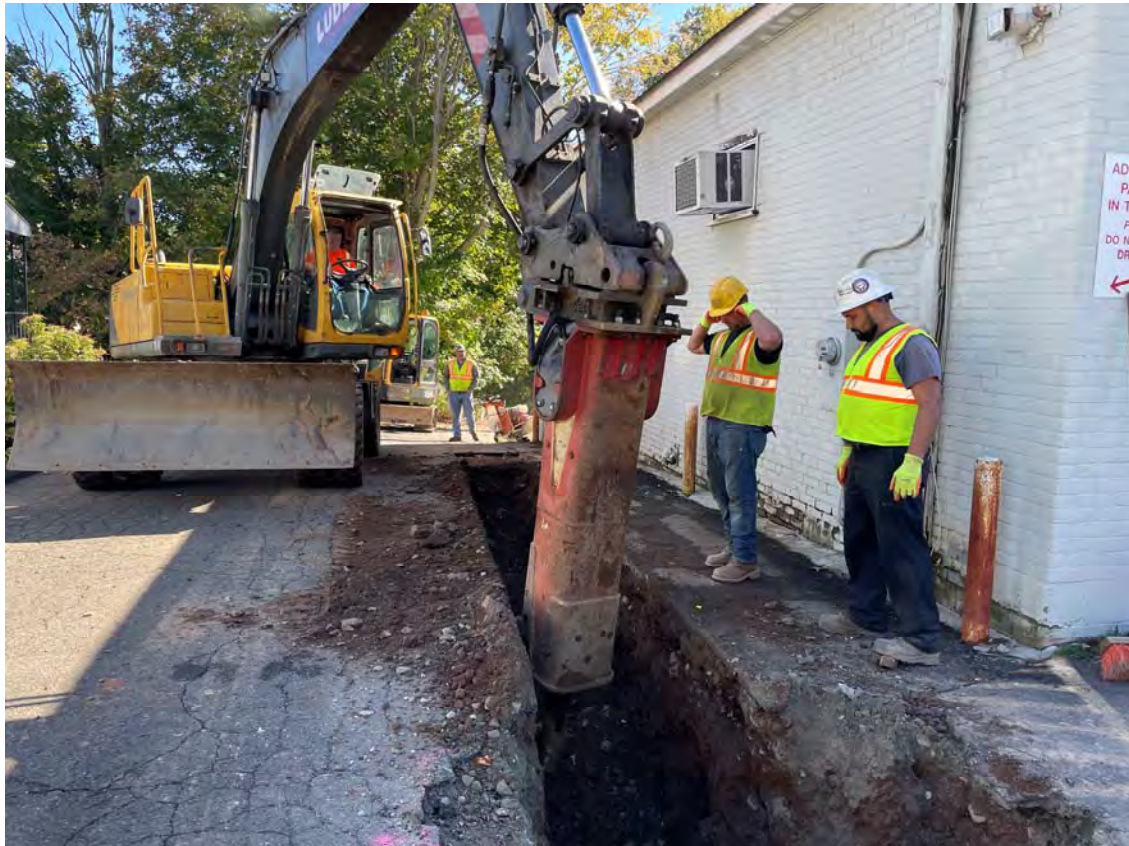
Picture 3: Ludlow hammering rock on the north side of the 325 Main Street building as they work to install a 1" copper water service line. View to the east.
