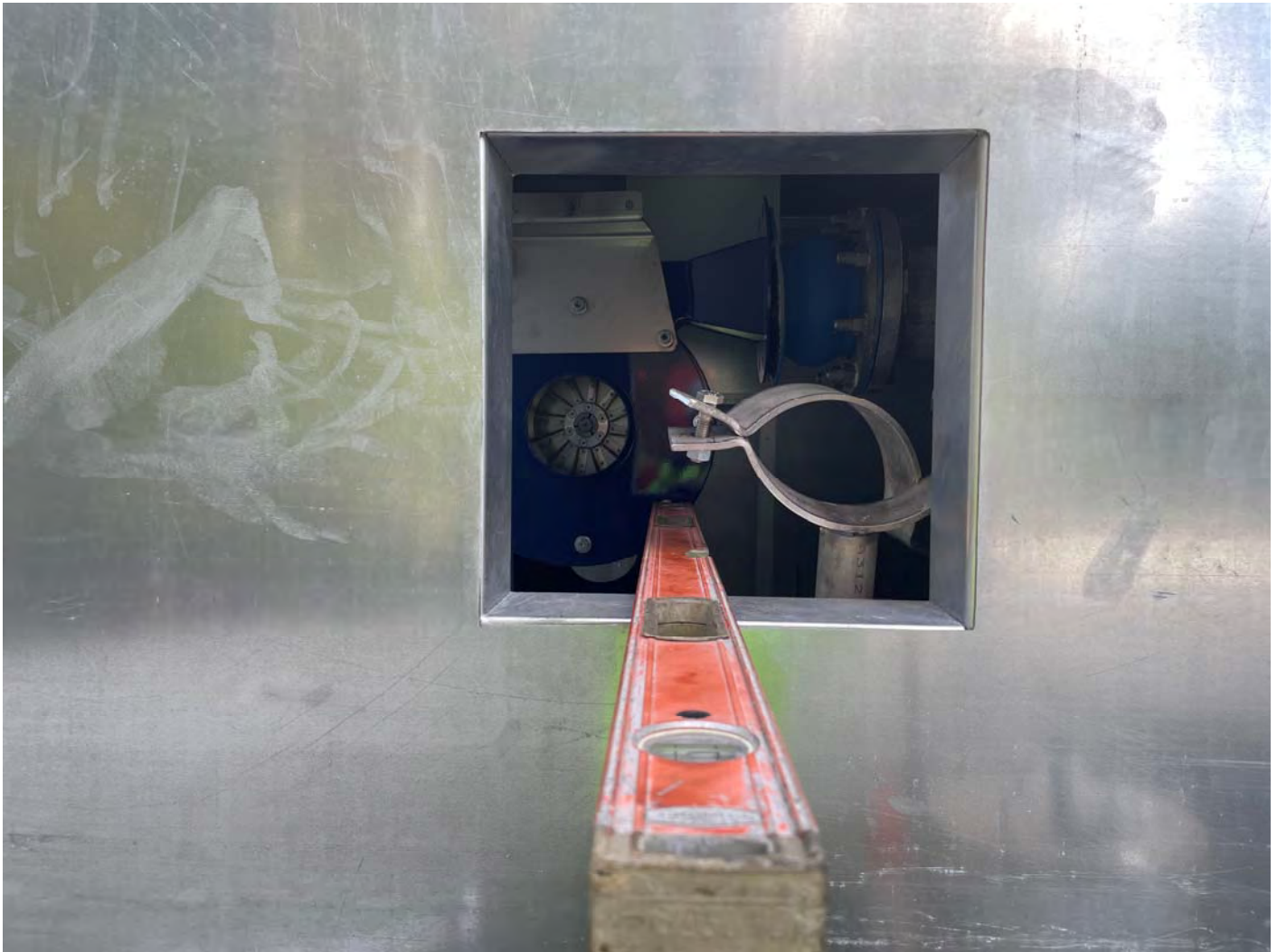
Picture 11: View into the blower enclosure on its west side. View to the east.
