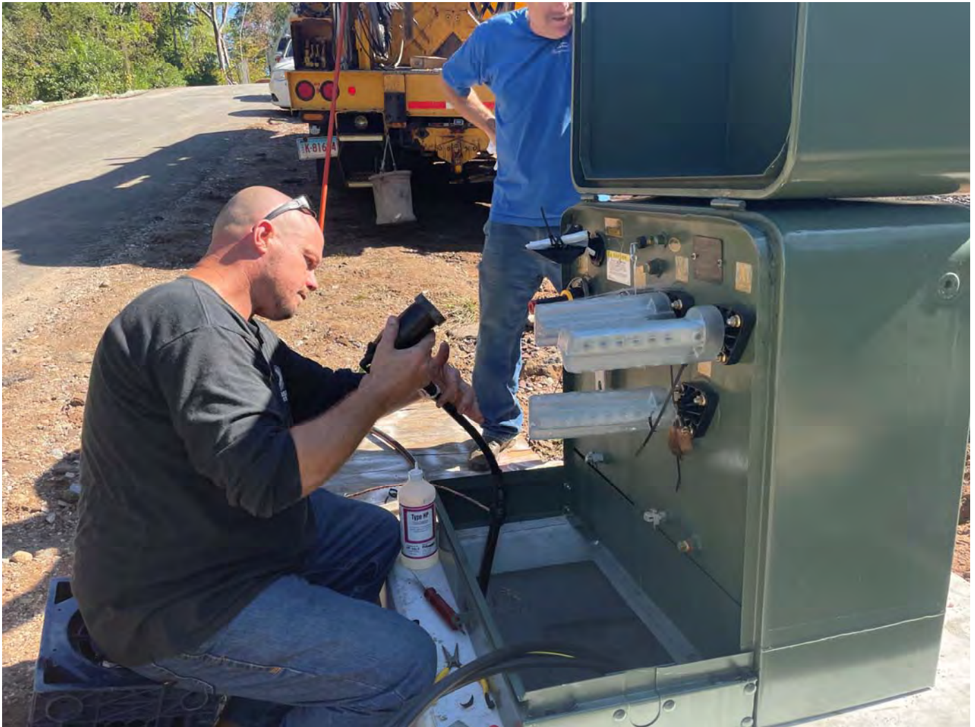
Picture 4: Eversource connecting a primary line to the transformer located at Station 12+00 on the Shared Access Driveway in Middletown. View to the east.
