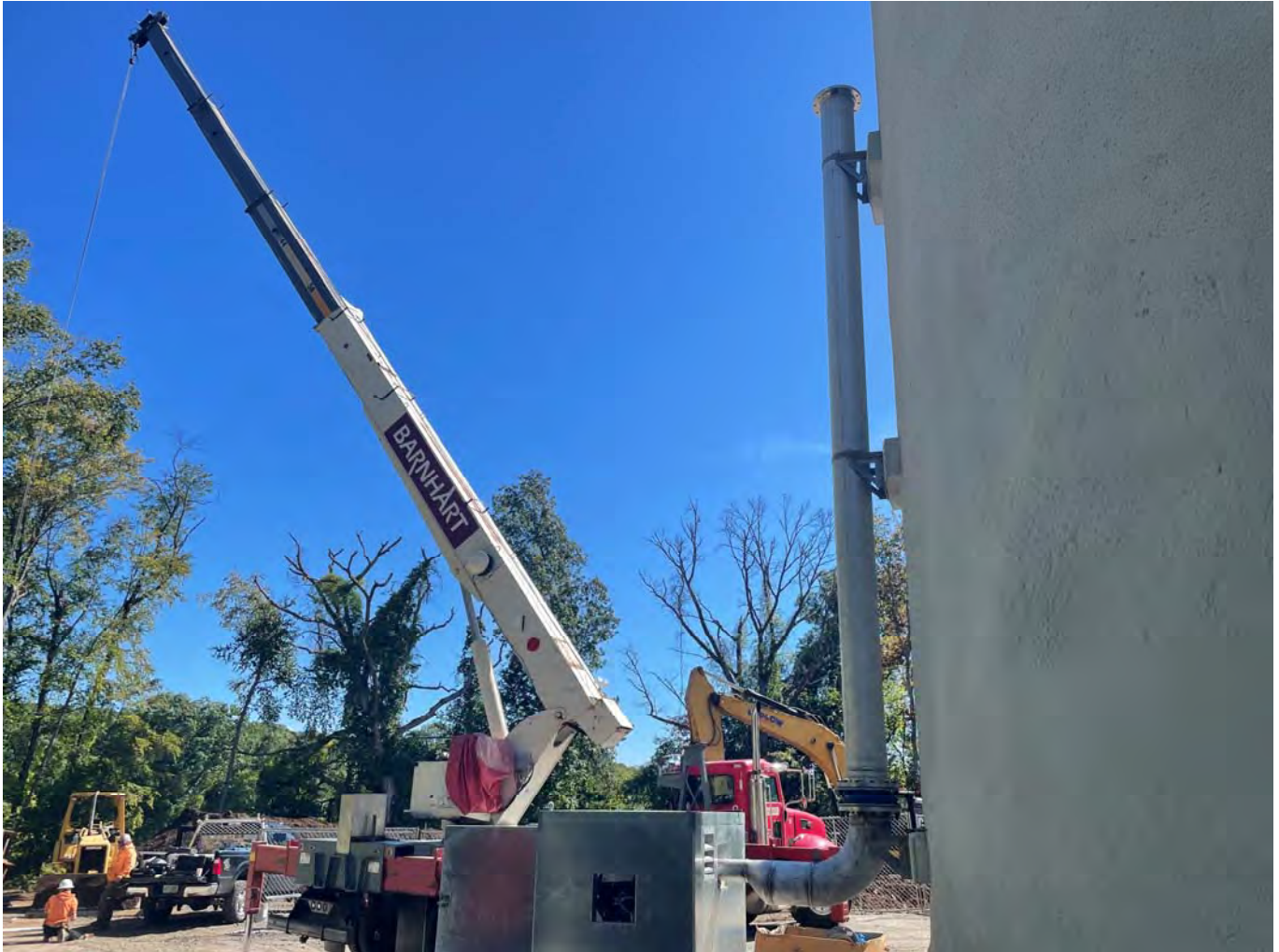
Picture 5: 20' section of 12" stainless steel air duct that DN Tanks has attached to the southwest side of the blower and the northeast side of the water tank located east of the Shared Access Driveway in Middletown. View to the southeast.
