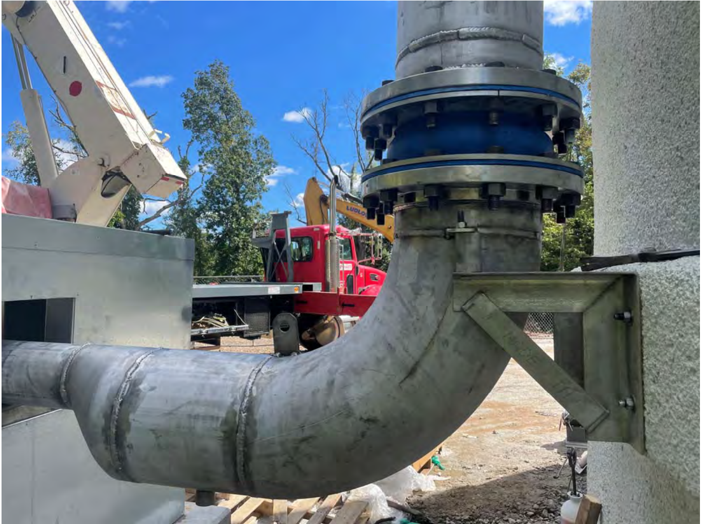
Picture 6: Stainless steel elbow exiting the southwest side of the blower, connected to 12" stainless steel air duct with a 12" Garlock Style 8400 expansion joint. View to the southeast.
