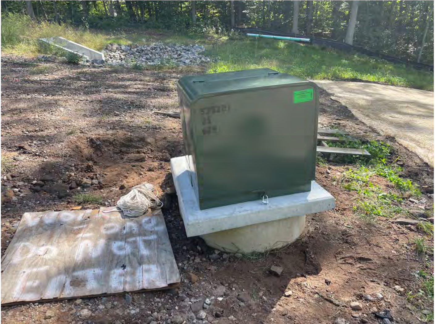
Picture 10: Transformer set in place by Eversource at Station 12+00. View to the south.
