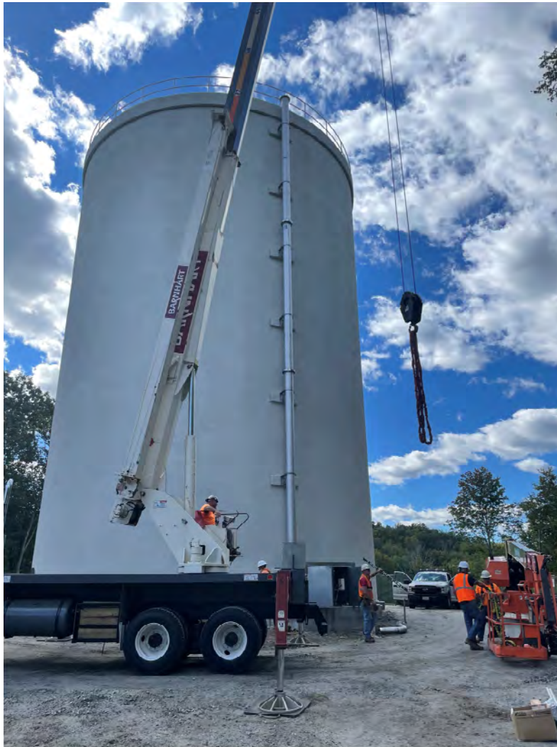
Picture 12: View of the water tank located east of the Shared Access Driveway in Middletown, with 12” stainless steel air duct installed and secured in place by DN Tanks today. View to the west.
