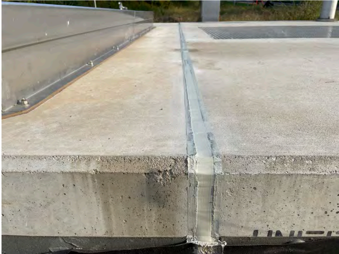
Picture 3: New caulking that United Concrete applied to the seam between the two halves of the PRV vault roof. View to the north.
