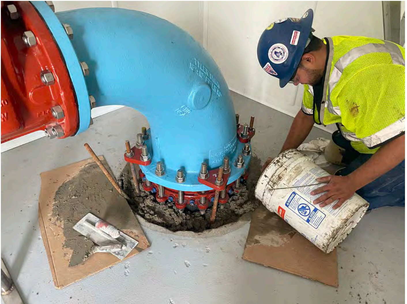
Picture 9: United Concrete placing 5500 PSI concrete around the penetration in the floor of the water meter building where the 16" water line passes through the floor. View to the southeast.
