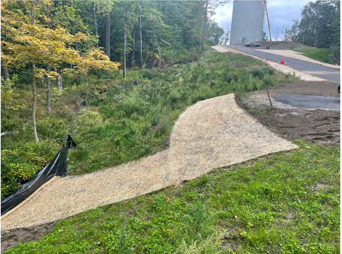
Picture 12: Straw erosion control mats that Ludlow placed on the north side of the turnout located at Station 14+00 on the Shared Access Driveway in Middletown. View to the east.
