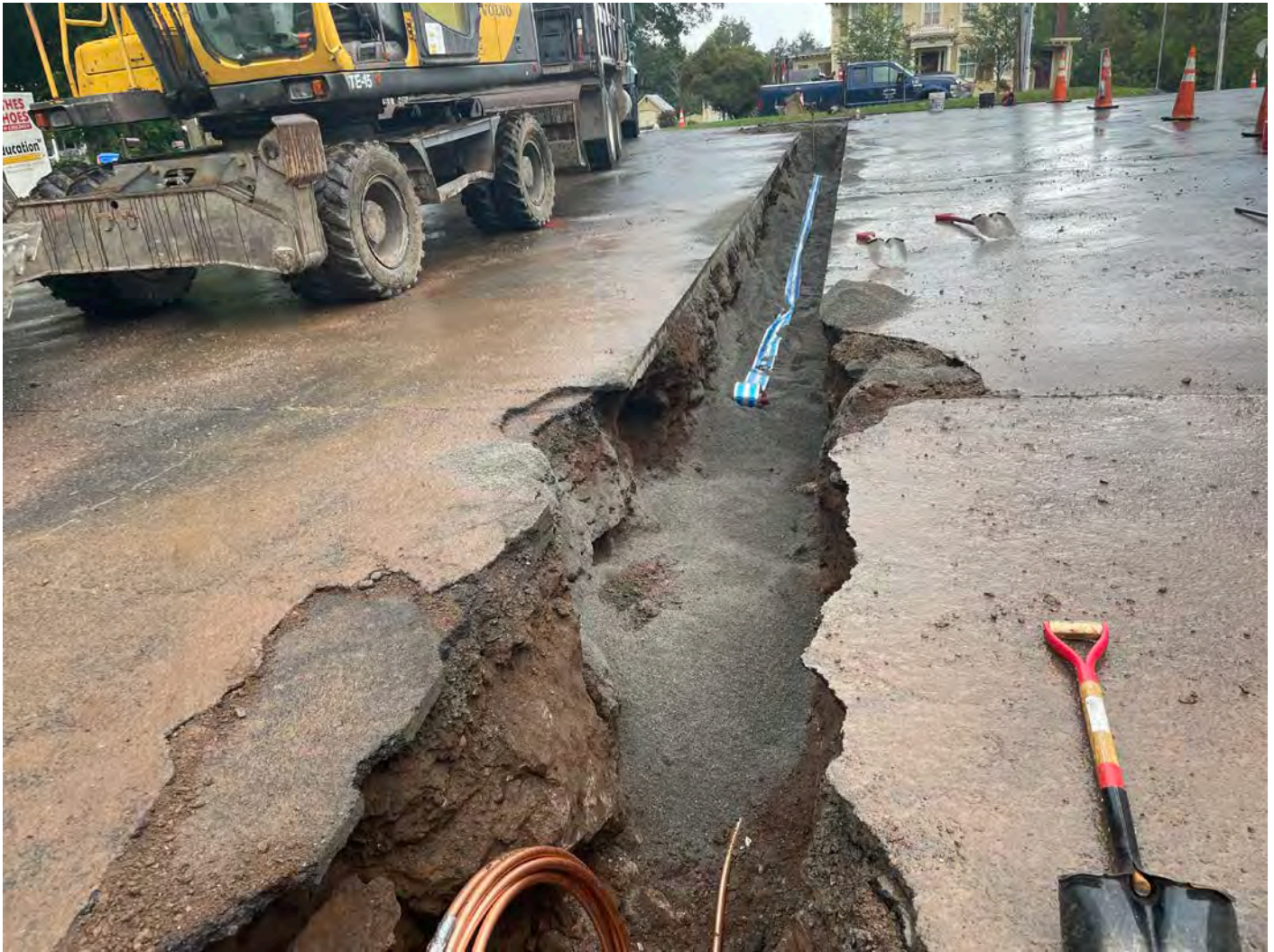
Picture 14: Sand and caution tape that Ludlow has placed over 1" copper water service line at the 321 Main Street property. View to the west.
