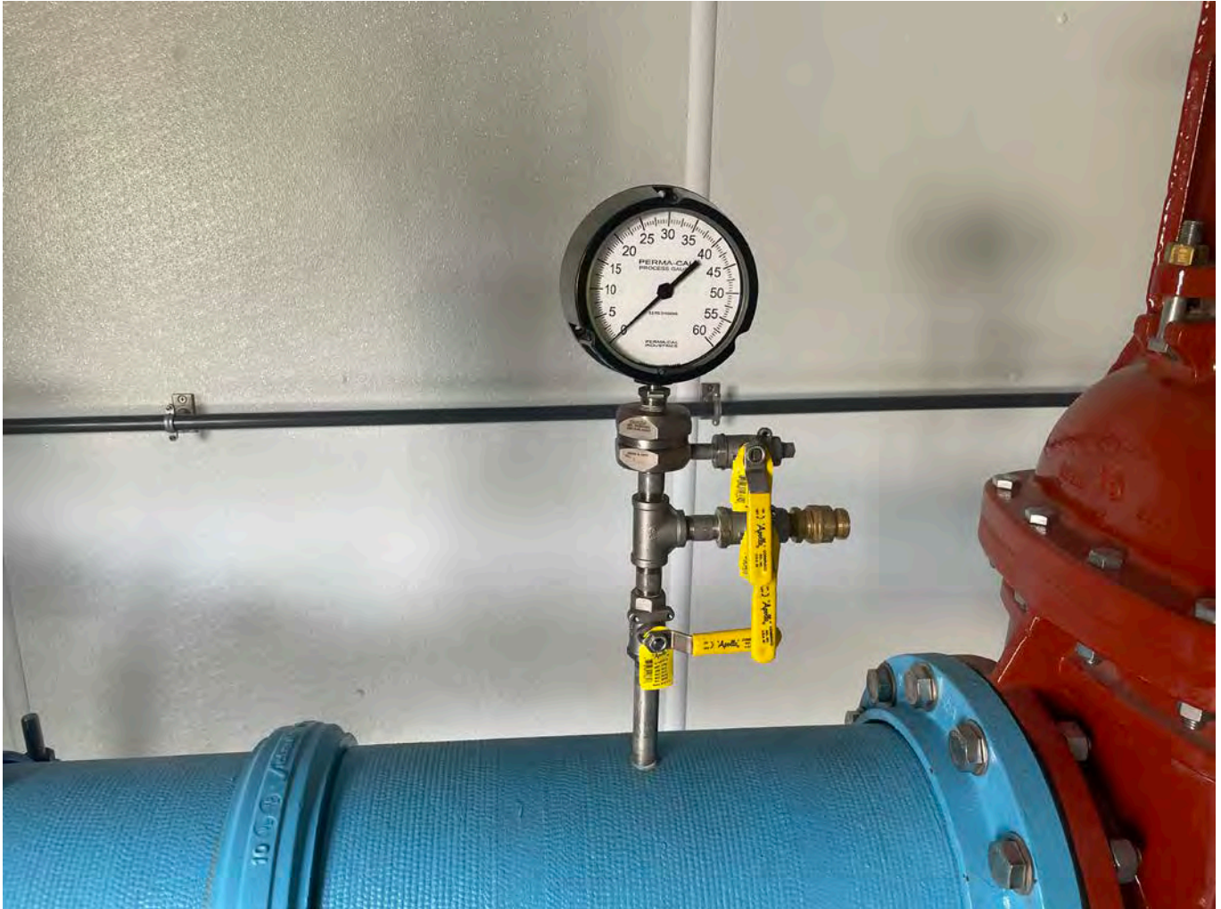
Picture 5: 60 PSI gauge that United Concrete will change out today with a 150 PSI gauge on the 16" DIP waterline located inside of the water meter building located at Station 126+80.
