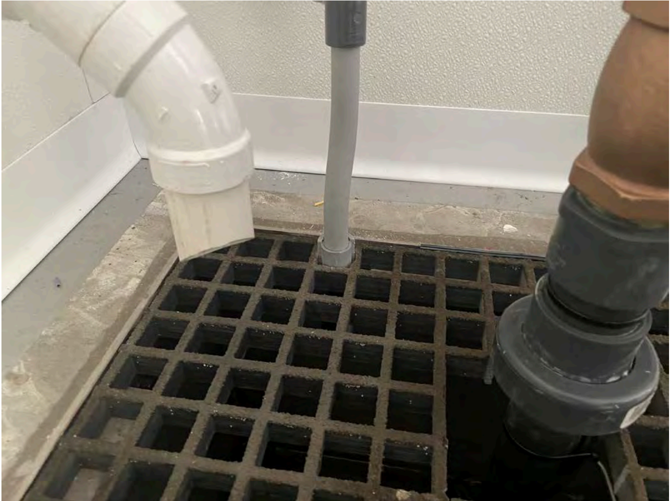
Picture 6: Gray 1/2 PVC conduit that was installed through the fiberglass grate at the northeast corner of the water meter vault located at Station 126+80. United Concrete will cut a larger hole in the grate around the PVC conduit. View to the east.
