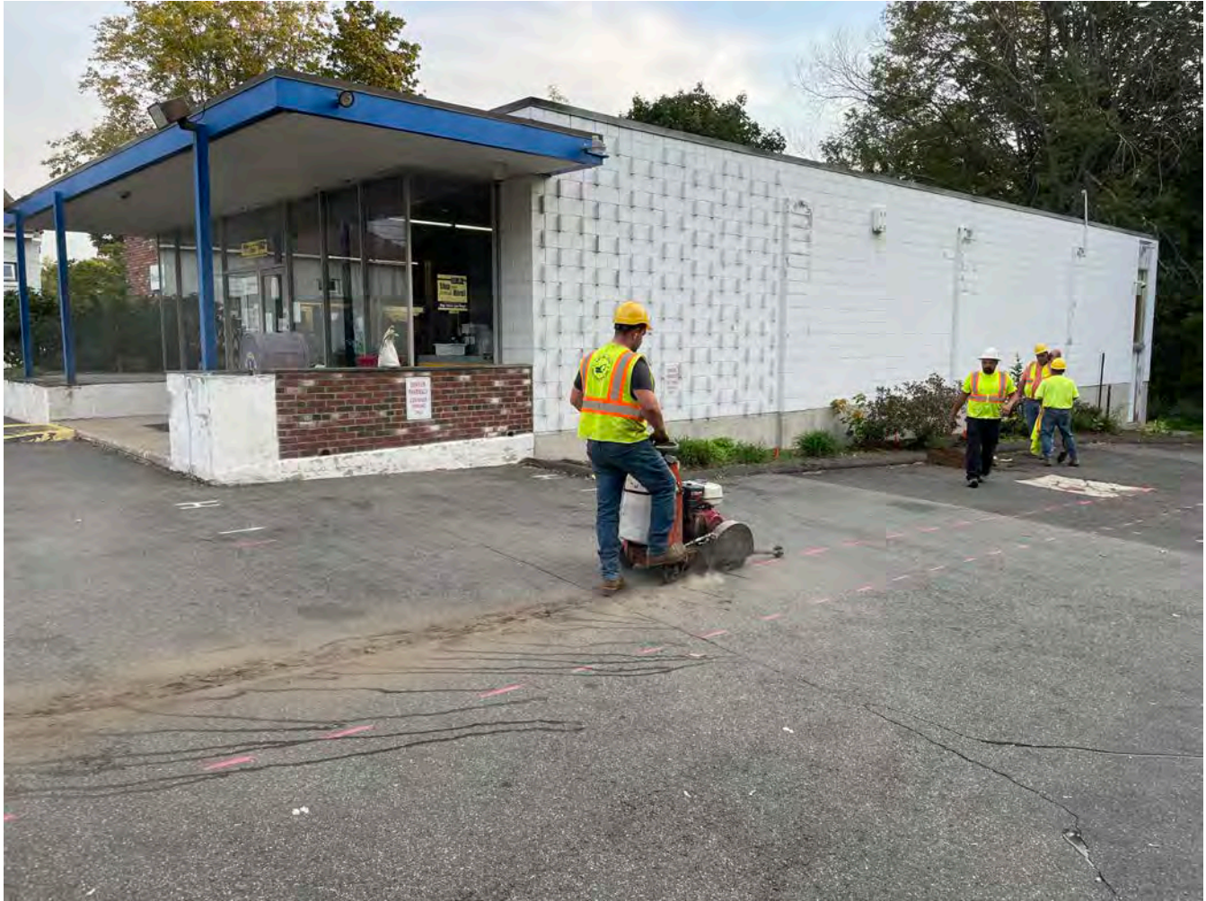
Picture 1: Ludlow saw cutting pavement in the driveway of the 321 Main Street property for the installation of a 1" copper water service line. View to the northeast.
