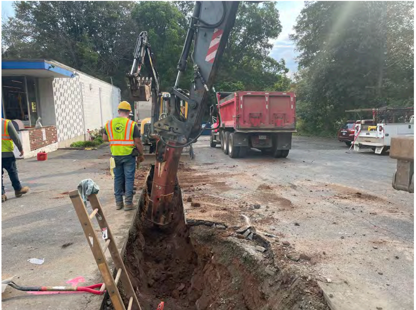
Picture 8: Ludlow hammering rock that they encountered while excavating a trench for the installation of a 1" copper water service line at the 321 Main Street property in Durham. View to the east.
