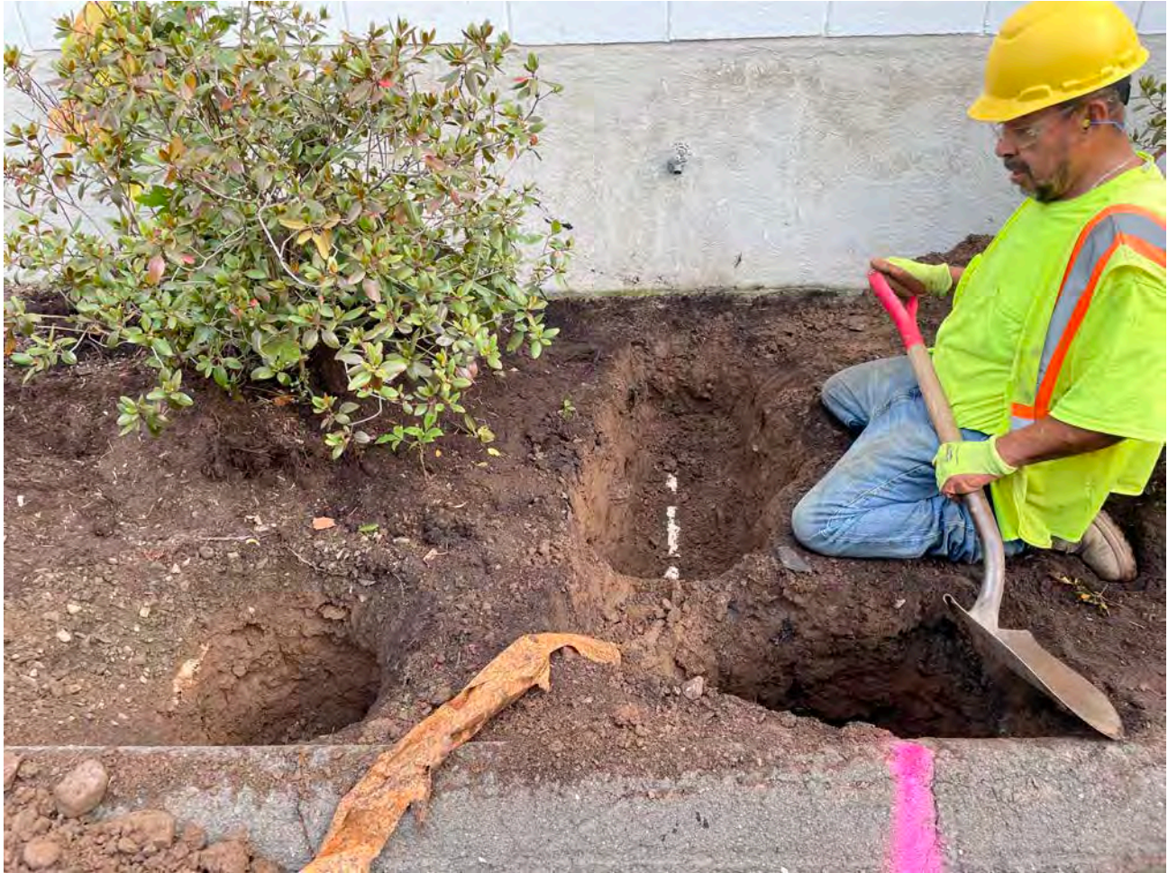
Picture 2: Ludlow hand excavating on the south side of the 321 Main Street building to identify the location of utilities prior to the installation of a 1" copper water service line. View to the north.
