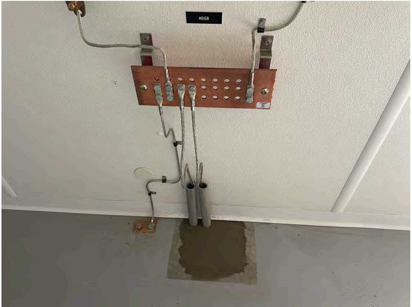
Picture 10: 5500 PSI concrete that United Concrete placed around a penetration in the floor on the west side of the water meter vault. View to the west.
