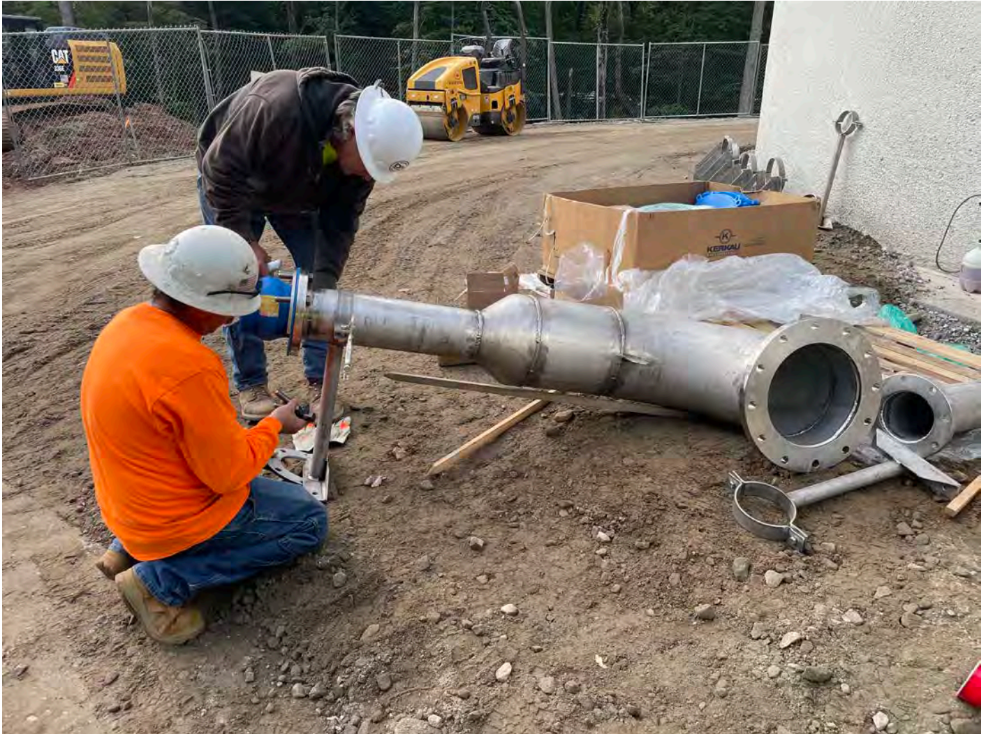
Picture 4: DN Tanks assembling sections of the air duct that will be installed on the northeast side of the water tank located east of the Shared Access Driveway in Middletown. View to the south.
