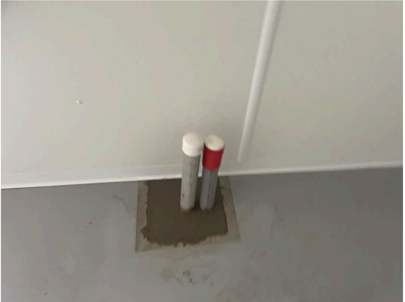
Picture 11: 5500 PSI concrete that United Concrete placed around another penetration in the floor on the west side of the water meter vault. View to the west.
