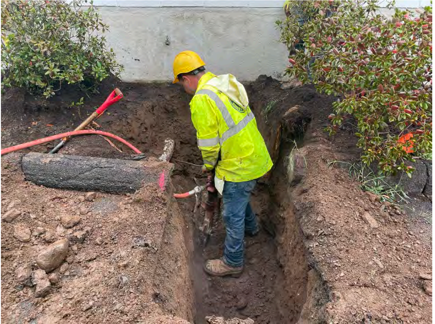
Picture 13: Ludlow jackhammering rock on the south side of the 321 Main Street building for the installation of a 1" copper water service line. View to the north.
