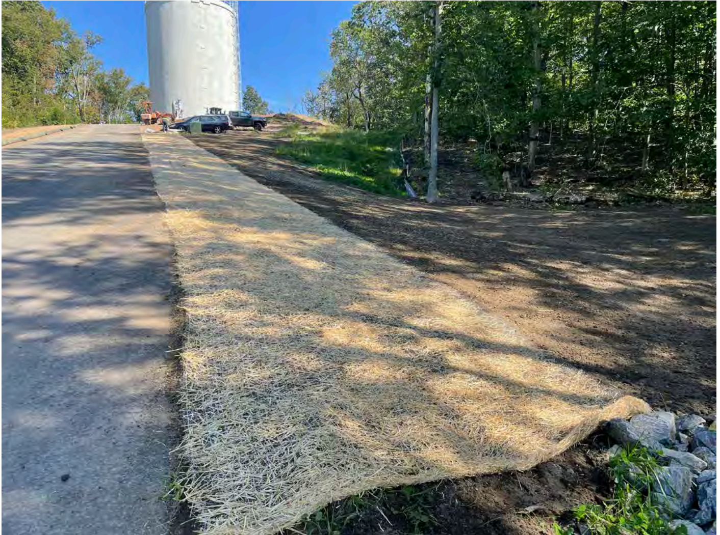
Picture 11: Straw mats that Ludlow has placed on top of freshly-placed loam and grass seed on the south side of the Shared Access Driveway in Middletown. View to the east.
