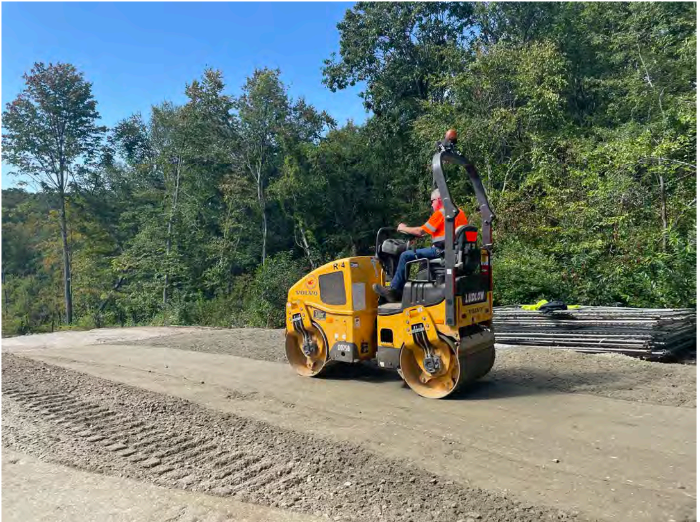
Picture 8: Ludlow compacting 1.5"-minus gravel on the north and northwest side of the water tank located east of the Shared Access Driveway in Middletown. View to the northwest.
