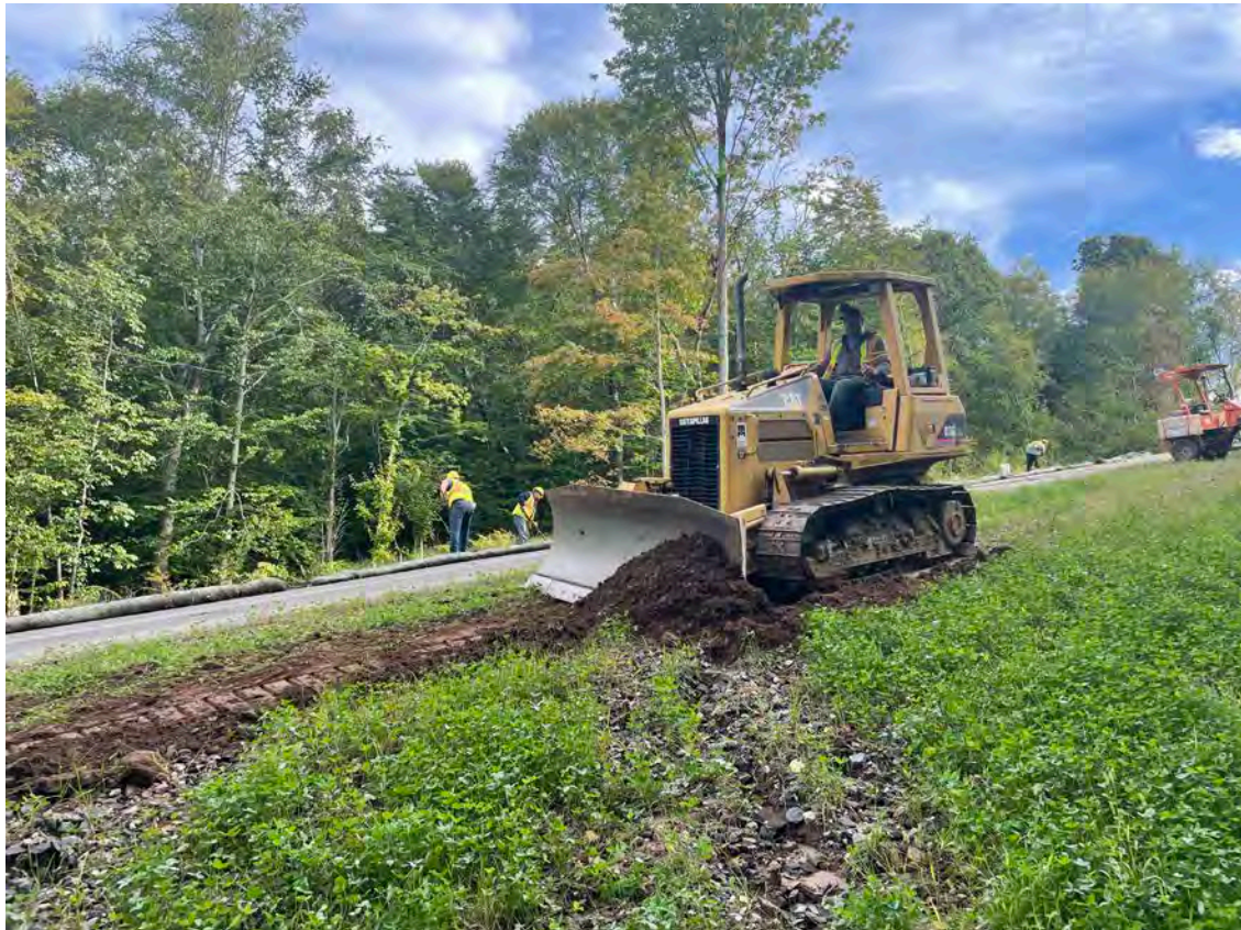
Picture 3: Ludlow grading soil on the south side of the Shared Access Driveway in Middletown. View to the east.
