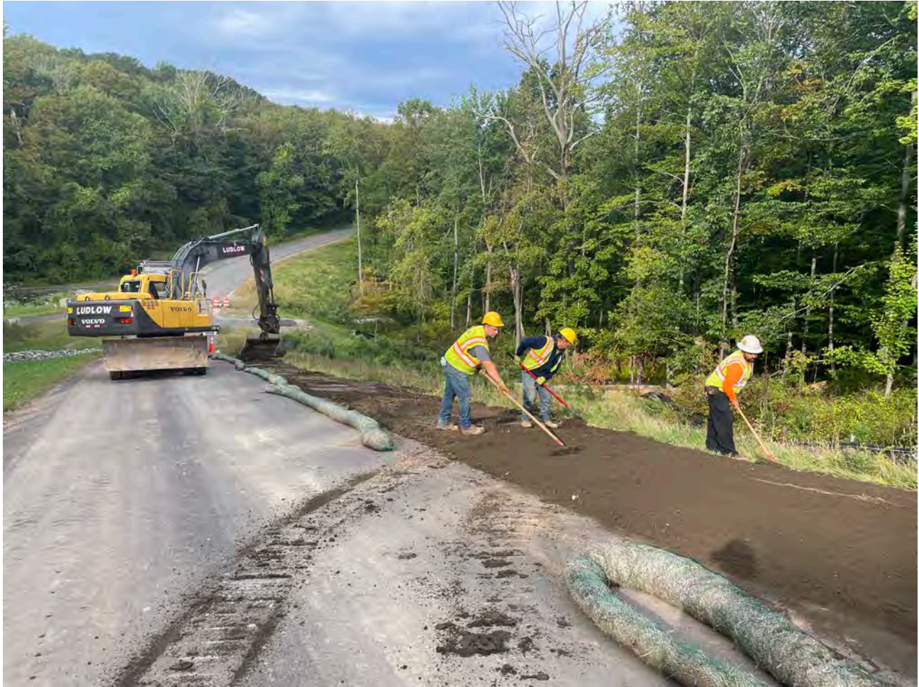
Picture 2: Ludlow placing and raking loam on the north side of the Shared Access Driveway in Middletown. View to the northwest.
