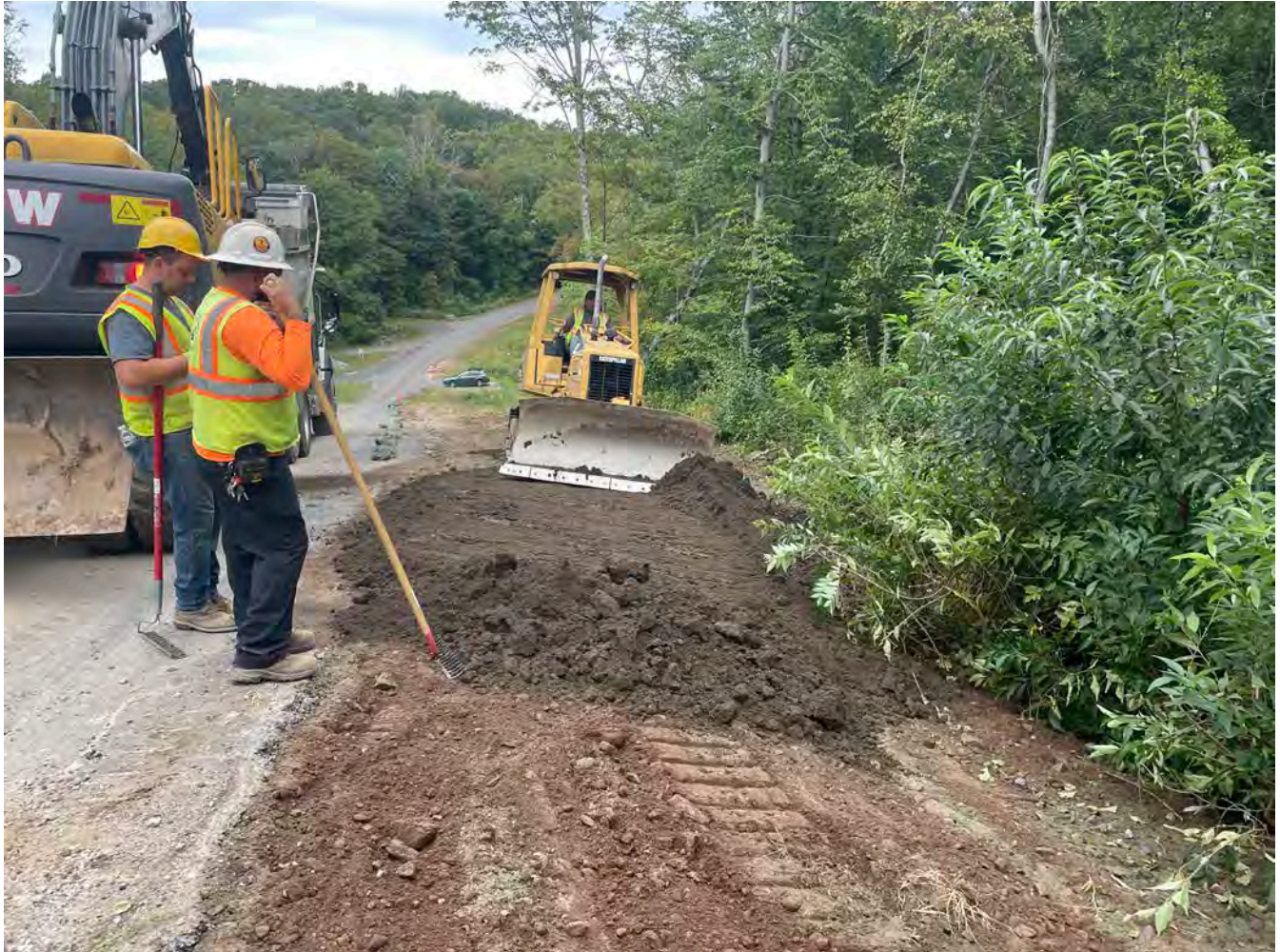
Picture 1: Ludlow placing and grading loam on the north side of the Shared Access Driveway in Middletown. View to the northwest.
