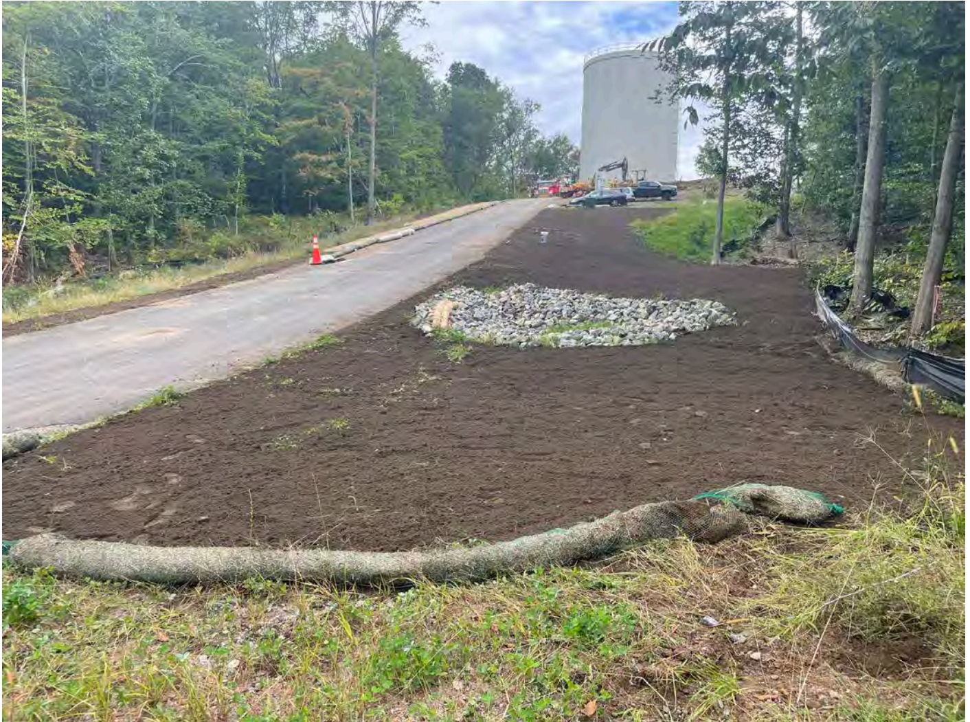
Picture 4: View of Ludlow's earthwork on the south side of the Shared Access Road in Middletown. View to the east.
