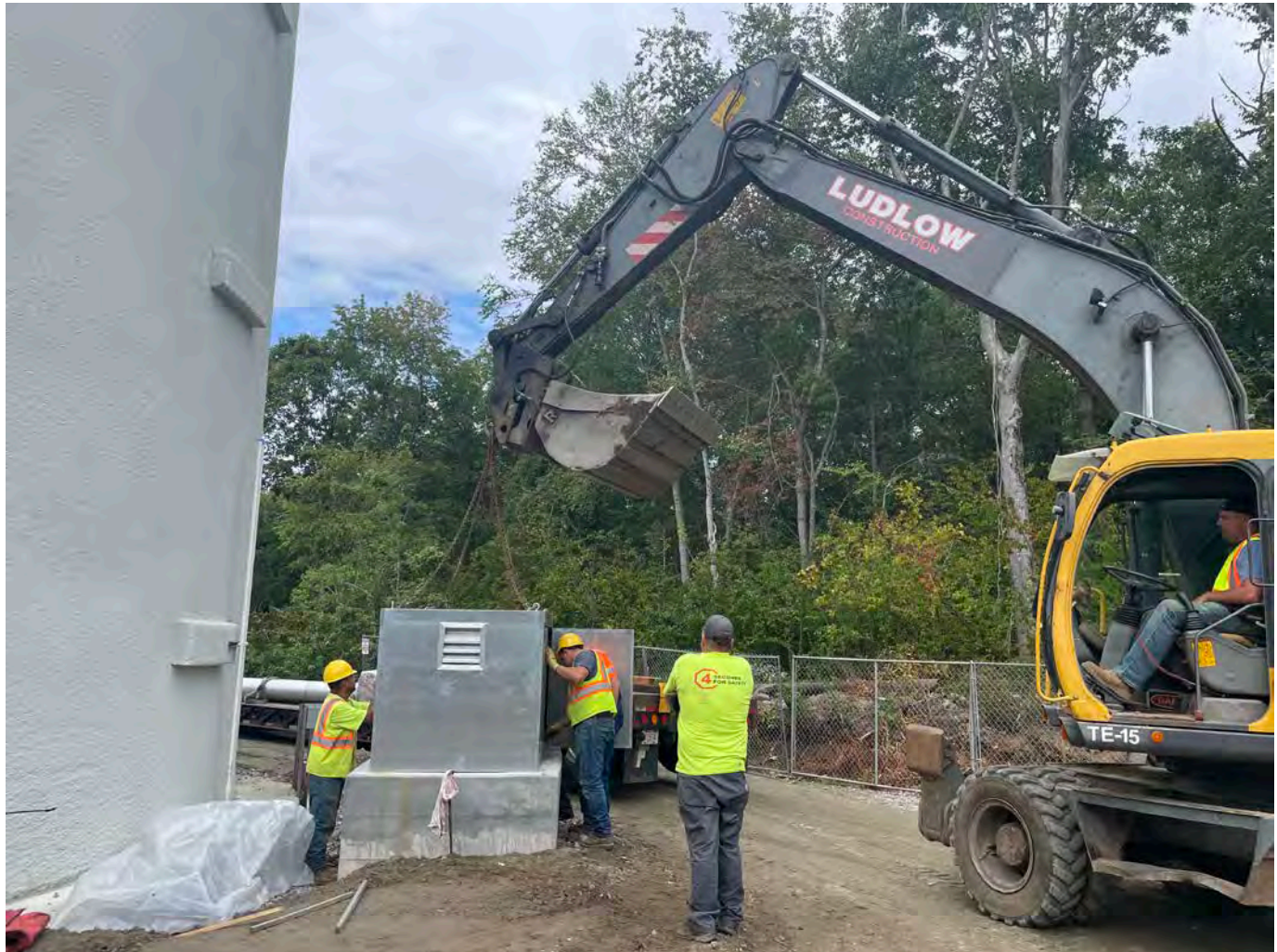
Picture 6: Ludlow placing a cabinet over the blower located on the northeast side of the water tank that is located east of the Shared Access Driveway in Middletown. View to the northeast.
