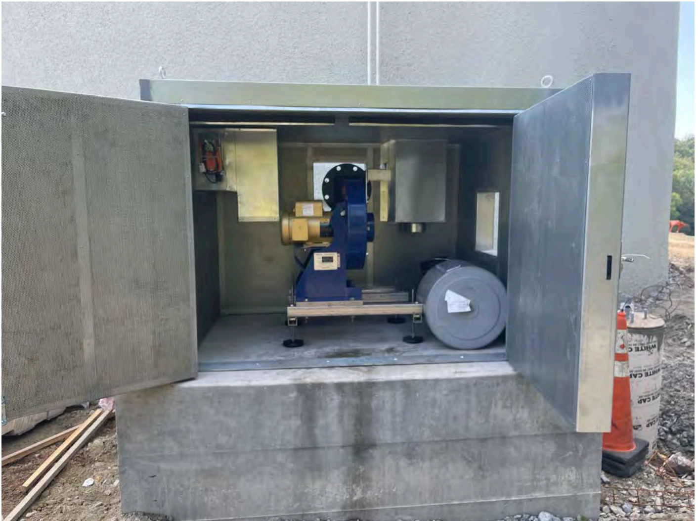
Picture 9: Blower inside of the cabinet that Ludlow placed over it on the northeast side of the water tank located east of the Shared Access Driveway in Middletown. View to the south.
