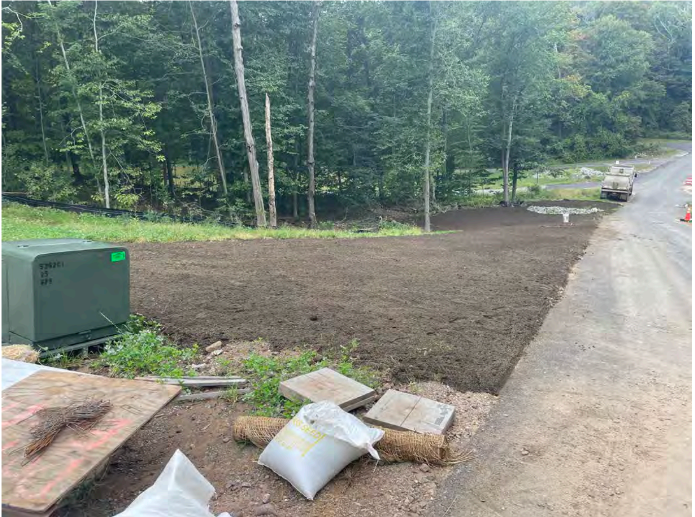
Picture 5: View of Ludlow's earthwork on the south side of the Shared Access Driveway in Middletown. View to the west.
