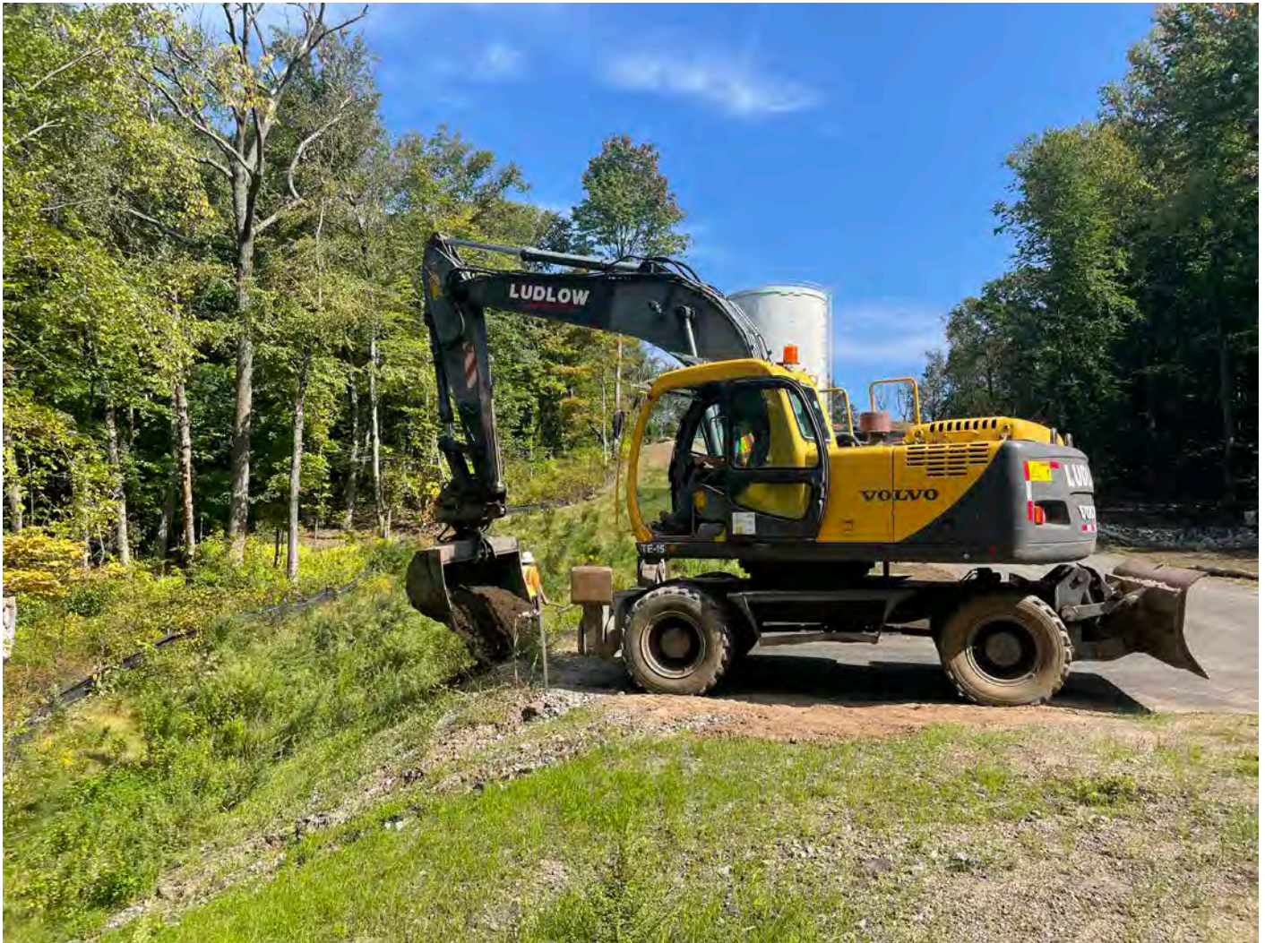
Picture 7: Ludlow placing loam on the north side of the turnout located at Station 14+00. View to the east.
