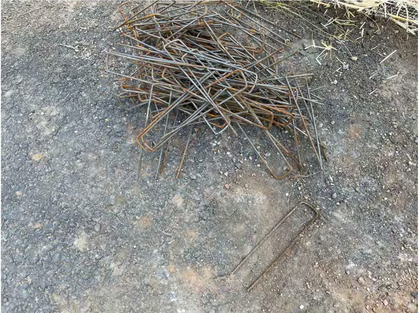
Picture 12: Steel staples that Ludlow is using to secure straw mats in place on the north and south side of the Shared Access Driveway in Middletown.
