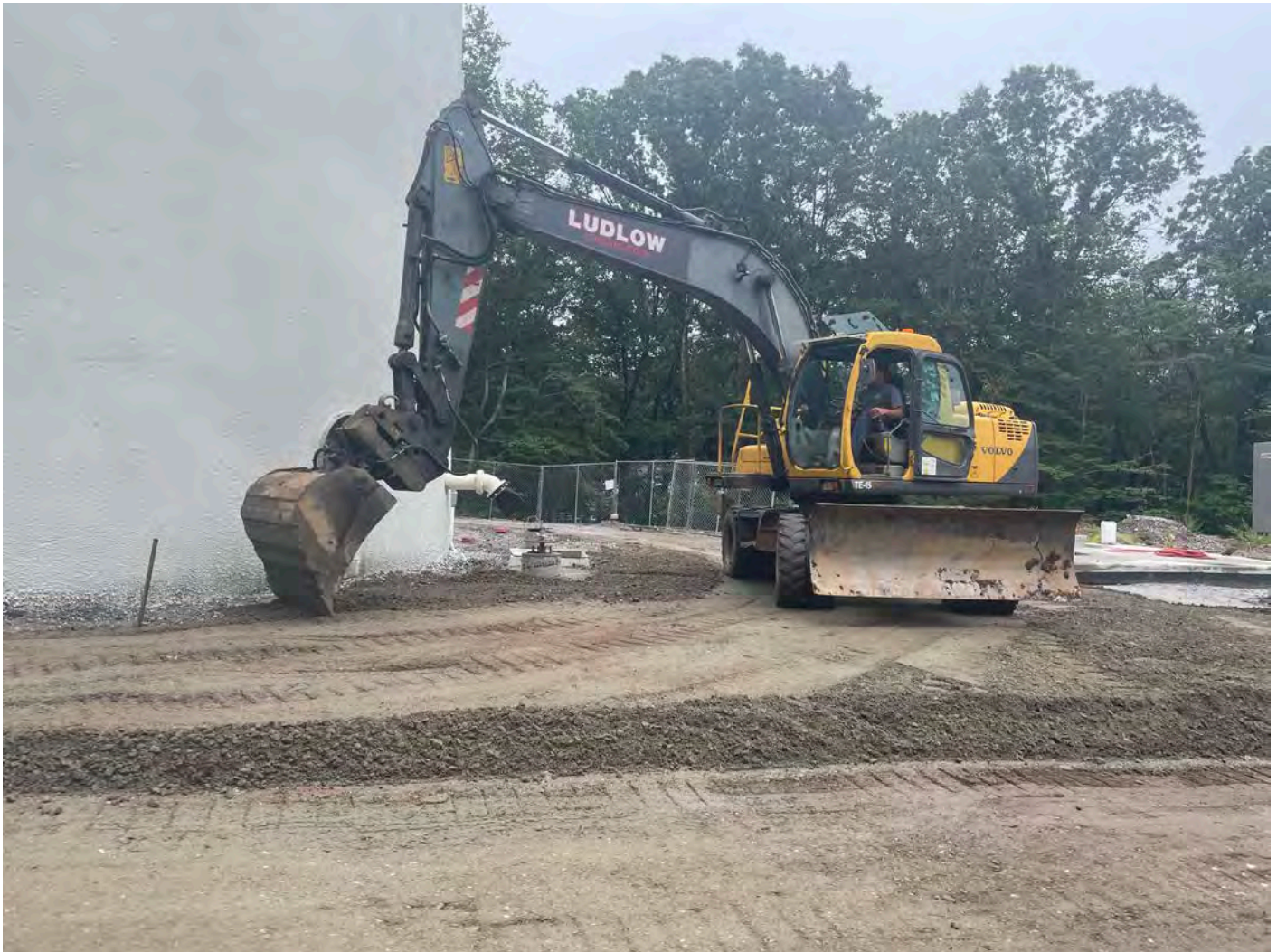
Picture 4: Ludlow grading 1.5"-minus gravel on the south side of the water tank located east of the Shared Access Driveway. View to the north.
