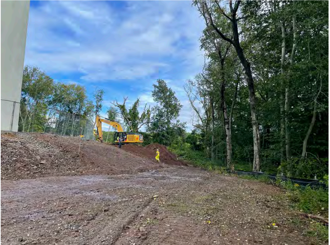
Picture 5: Current view of Ludlow's earthwork on the south side of the water tank located east of the Shared Access Driveway in Middletown. View to the east.
