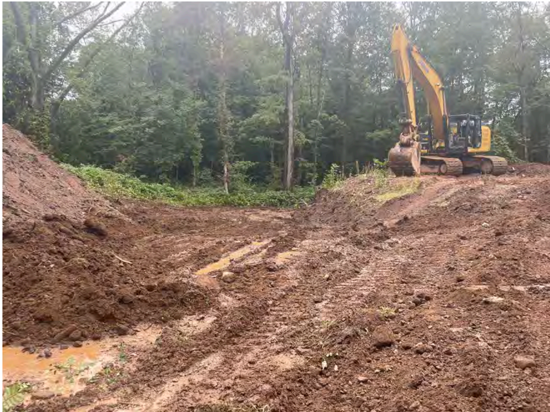
Picture 3: Current view of the area that Ludlow is performing earth work on the east side of the water tank. View to the south.
