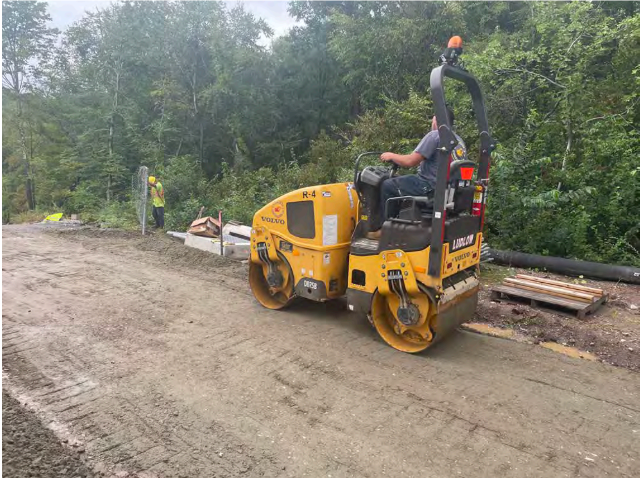
Picture 2: Ludlow compacting 1.5"-minus gravel on the north/northeast side of the water tank located east of the Shared Access Driveway in Middletown where they recently removed a section of asphalt. View to the northwest.
