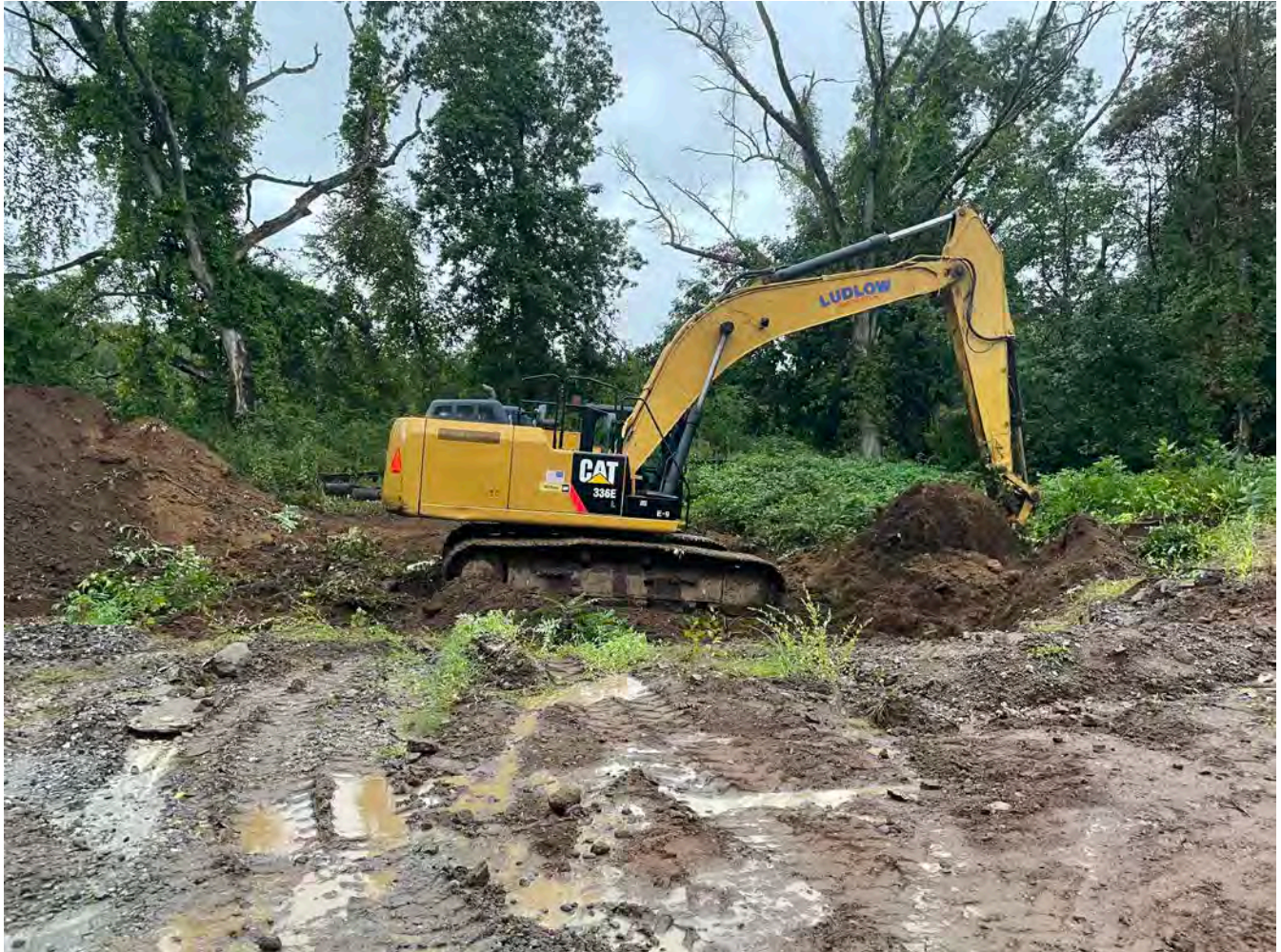
Picture 1: Ludlow performing earth work on the east side of the water tank located east of the Shared Access Driveway. Ludlow is shaping the soil to create the final ground contours. View to the east.
