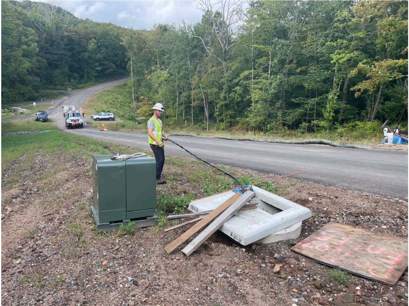
Picture 9: Eversource pulling the electrical cable from the vault located at Station ~11+50 that they fed into the conduit located on the west side of the electrical enclosure located north of the altitude vault. View to the west.
