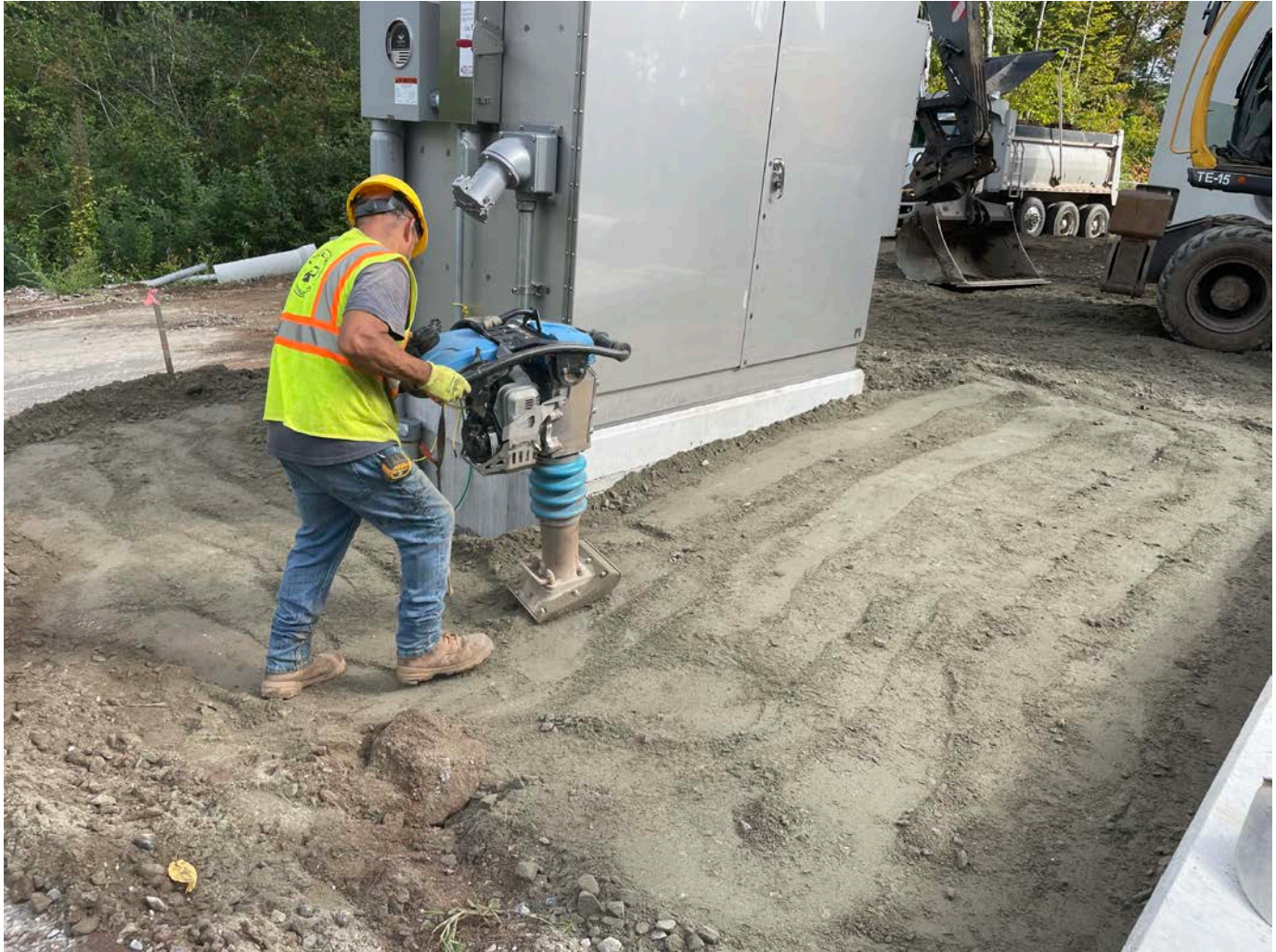
Picture 6: Ludlow compacting fill around the electrical enclosure located on the north side of the altitude vault. View to the northeast.
