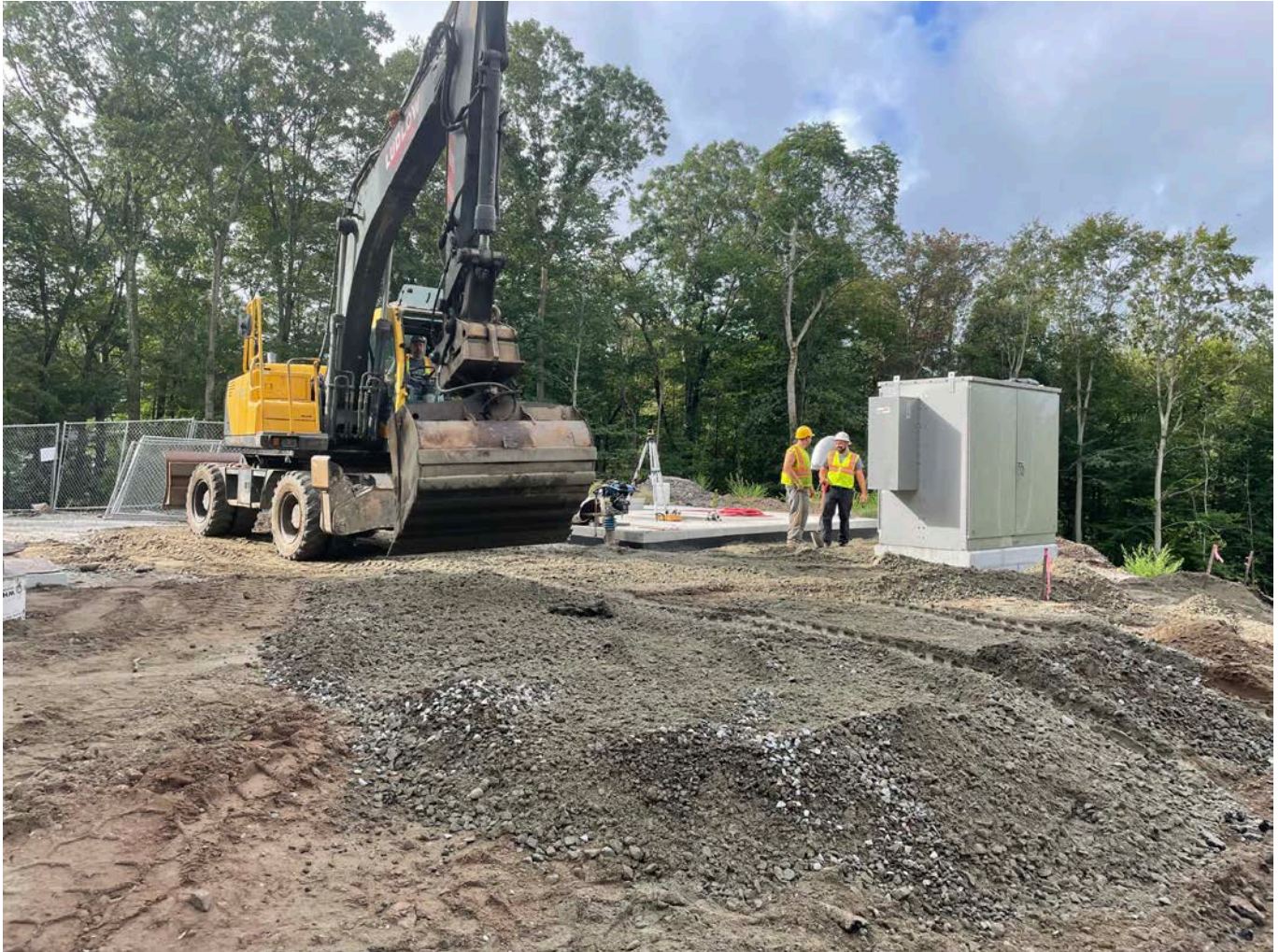
Picture 5: Ludlow grading 1.5"-minus gravel on the west side of the water tank located on the east side of the Shared Access Driveway. View to the southwest.
