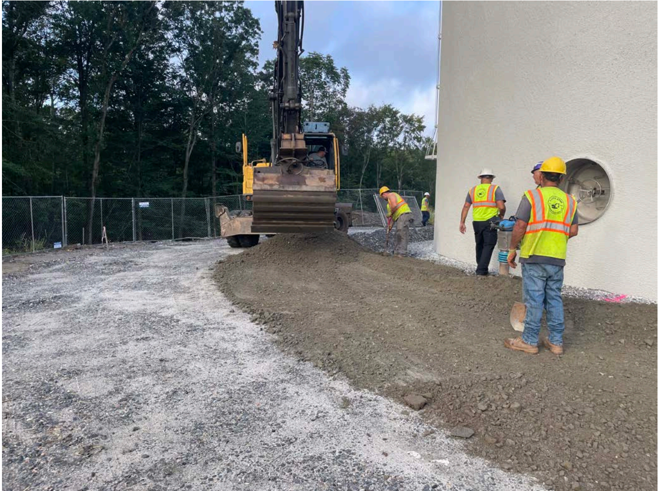
Picture 1: Ludlow placing 1.5"-minus gravel around the southeast side of the water tank located east of the Shared Access Driveway in Middletown. View to the west.
