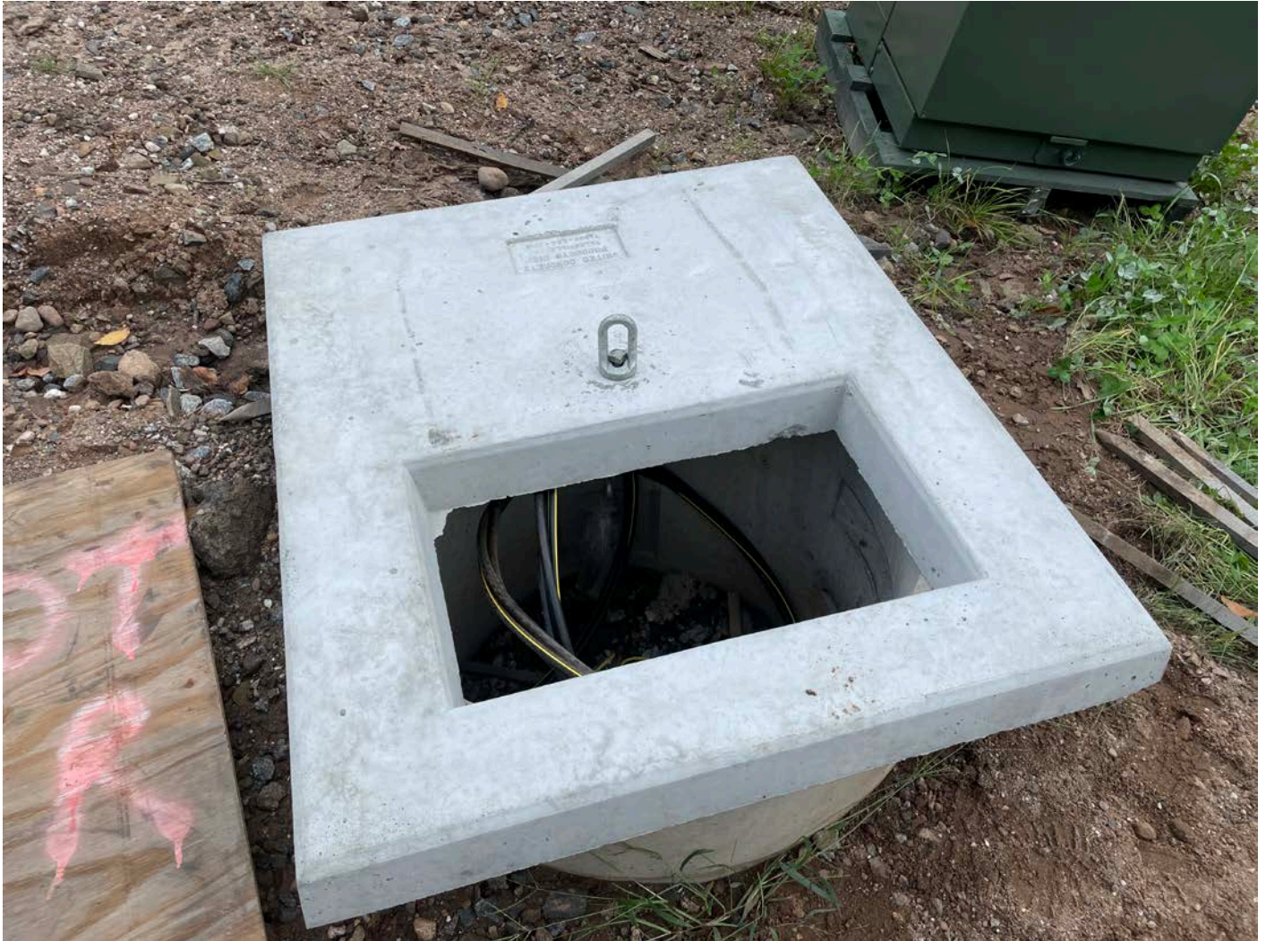
Picture 4: New transformer slab at that Ludlow picked up from United Concrete today and placed at Station ~11+50.
