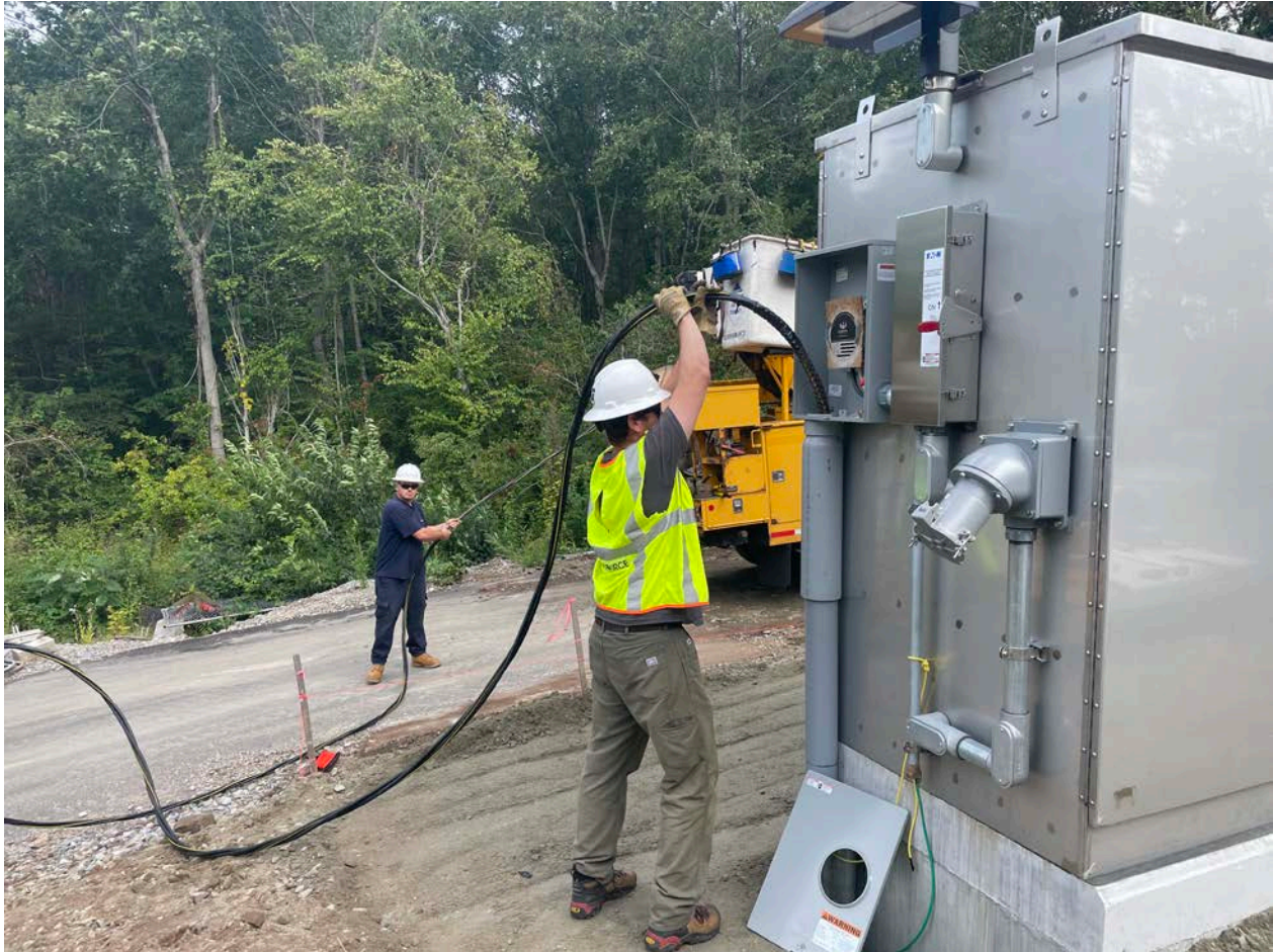
Picture 8: Eversource feeding electrical cables into conduit located on the west side of the electrical enclosure located north of the altitude vault. View to the north.
