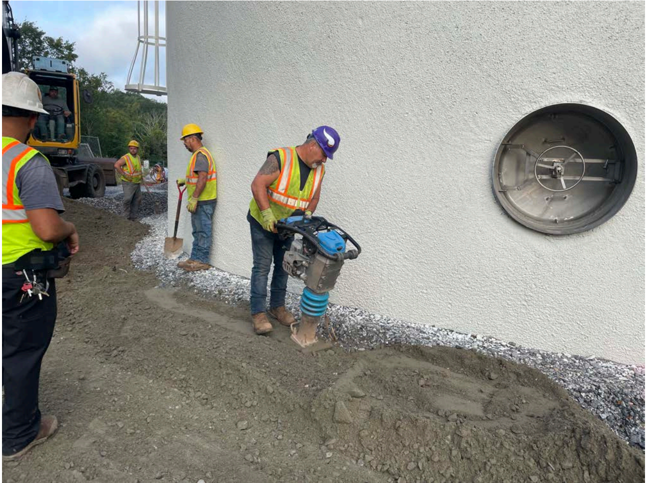
Picture 2: Ludlow compacting 1.5"-minus gravel along the edge of southeast side of the water tank located east of the Shared Access Driveway in Middletown. View to the west.
