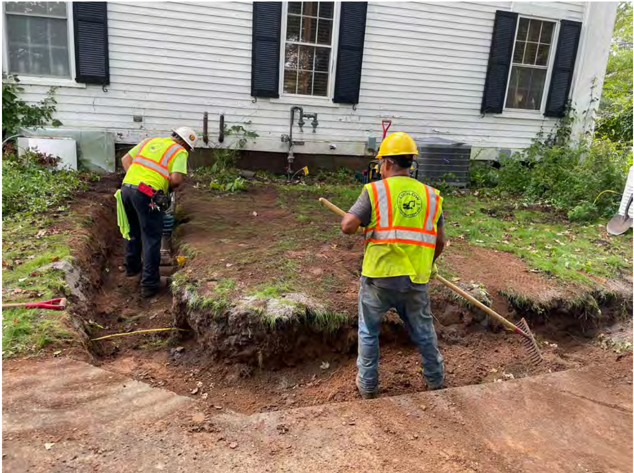
Picture 8: Ludlow compacting fill with a jumping jack that they placed over the 1" copper water service line they installed at the 313 Main Street residence. View to the south.
