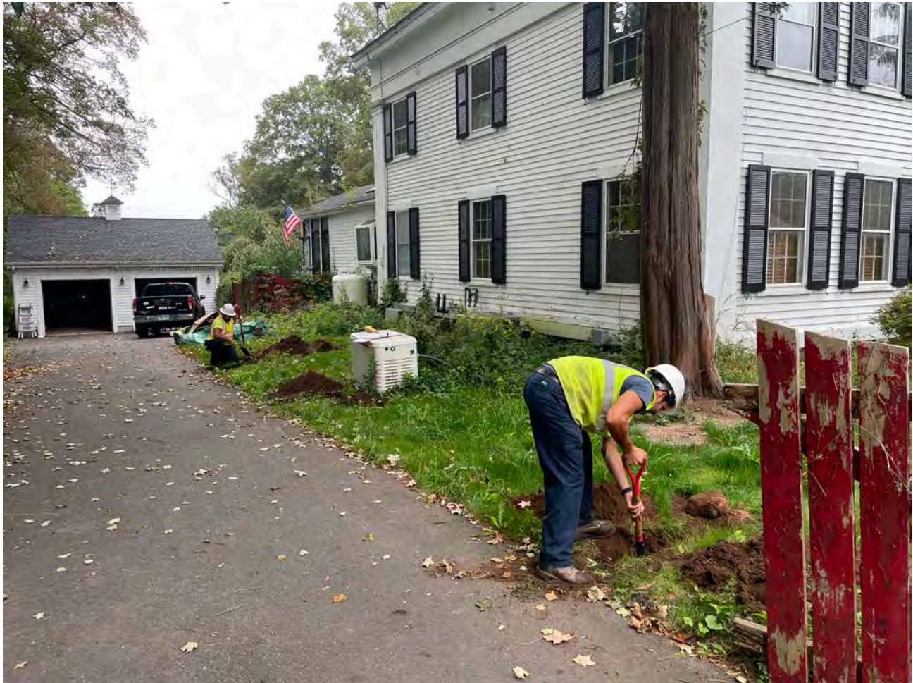
Picture 2: Ludlow hand excavating at the 313 Main Street, Durham, property to locate a recently-installed gas line that conflicts with the planned route that Ludlow had planned to run a 1" copper water service line to the residence. View to the east.
