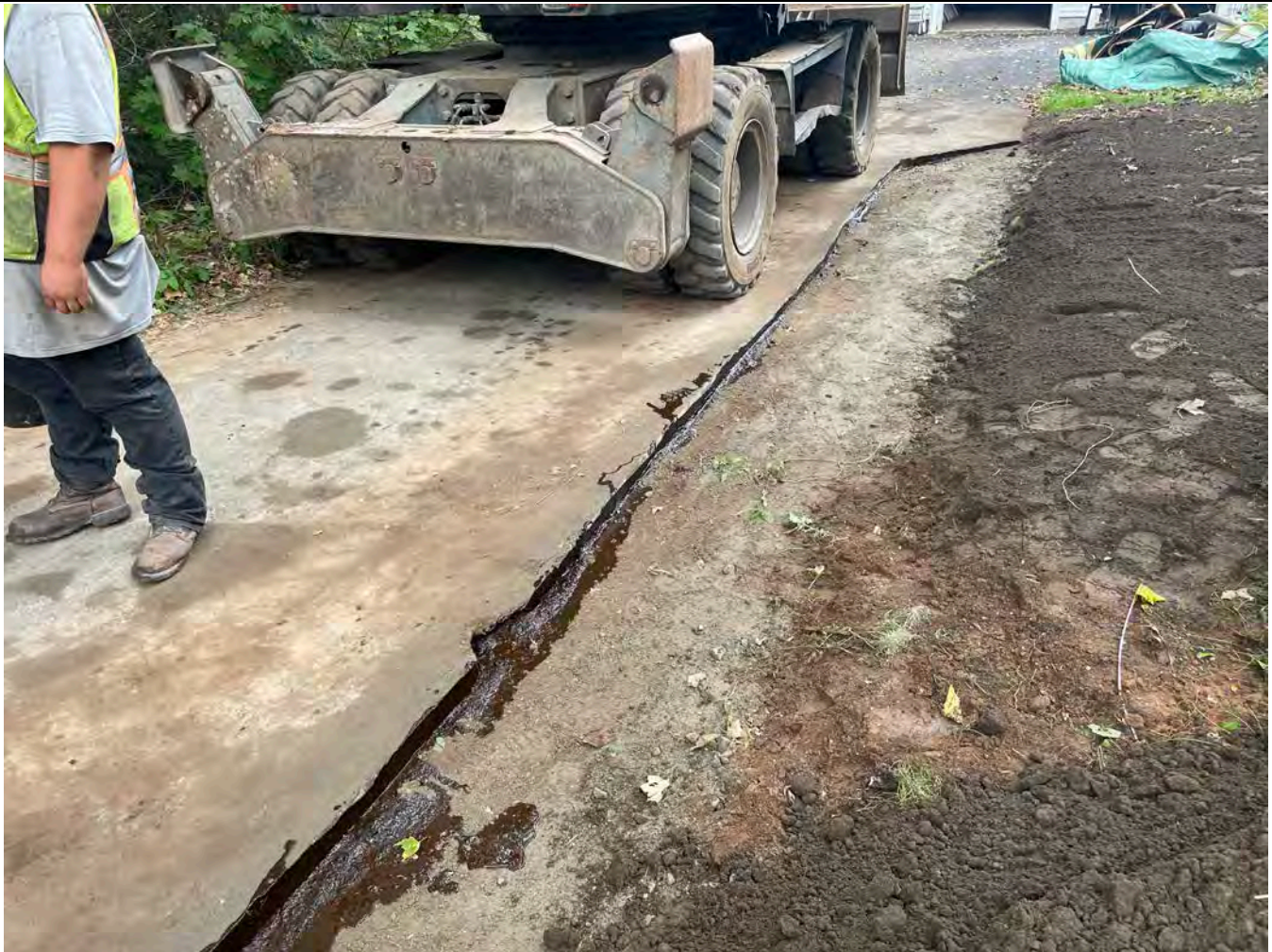
Picture 9: Tack coating that Ludlow placed on the cut edges of driveway pavement on the north side of the 313 Main Street residence for the installation of a 1" copper water service line. View to the east.
