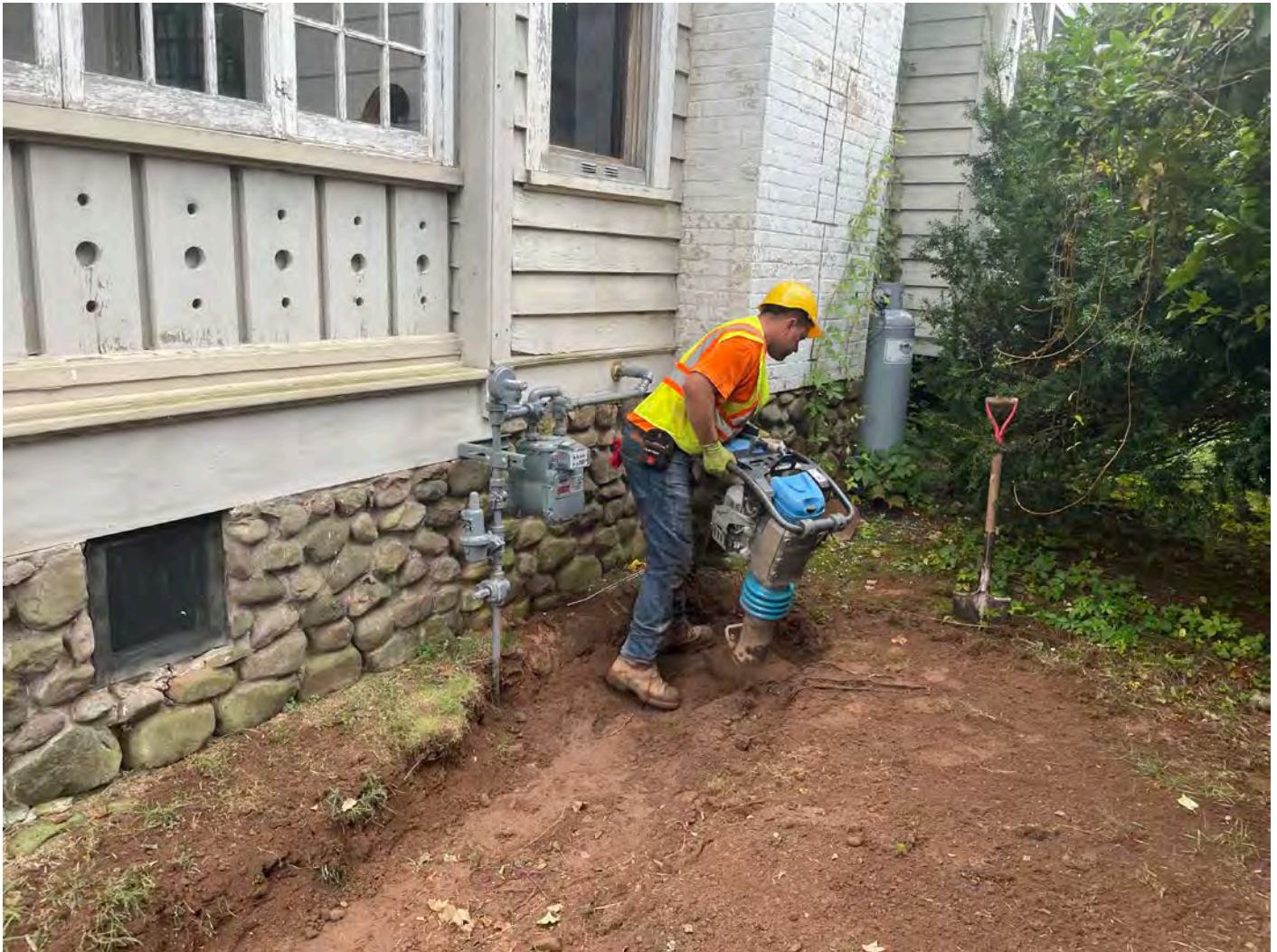
Picture 4: Ludlow using a jumping jack to compact fill that they used to backfill the trench they excavated during the installation of a 1" copper water service line on the north side of the 316 Main Street residence. View to the southwest.
