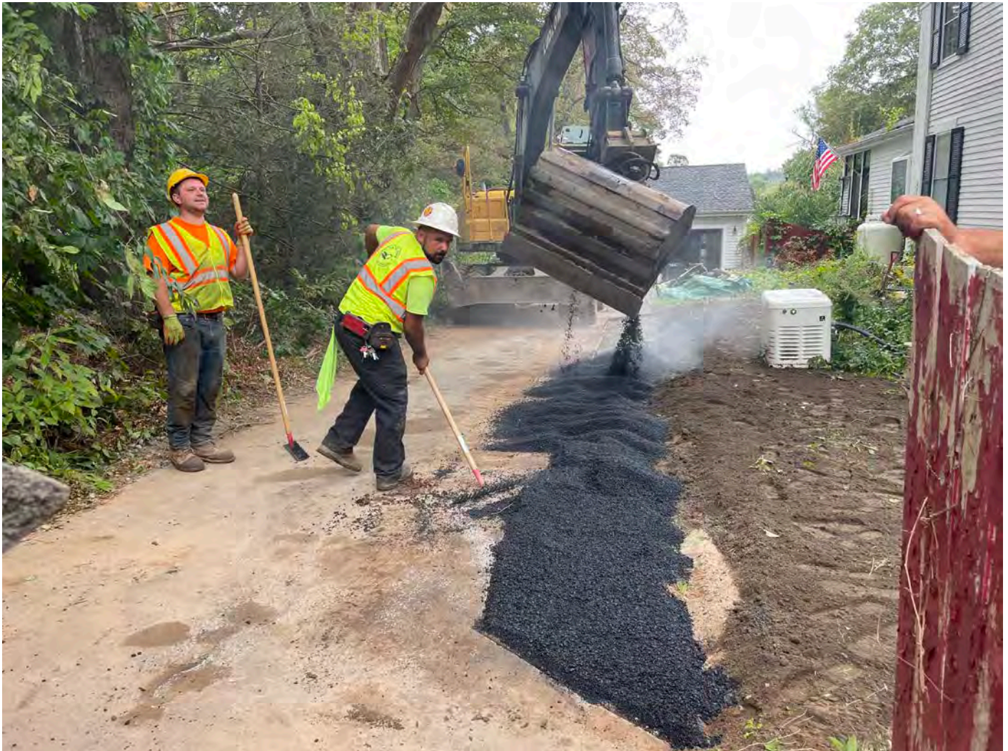
Picture 10: Ludlow placing asphalt at the 313 Main Street residence to repair the driveway after having cut out the south side of it for the installation of a 1" copper water service line. View to the east.
