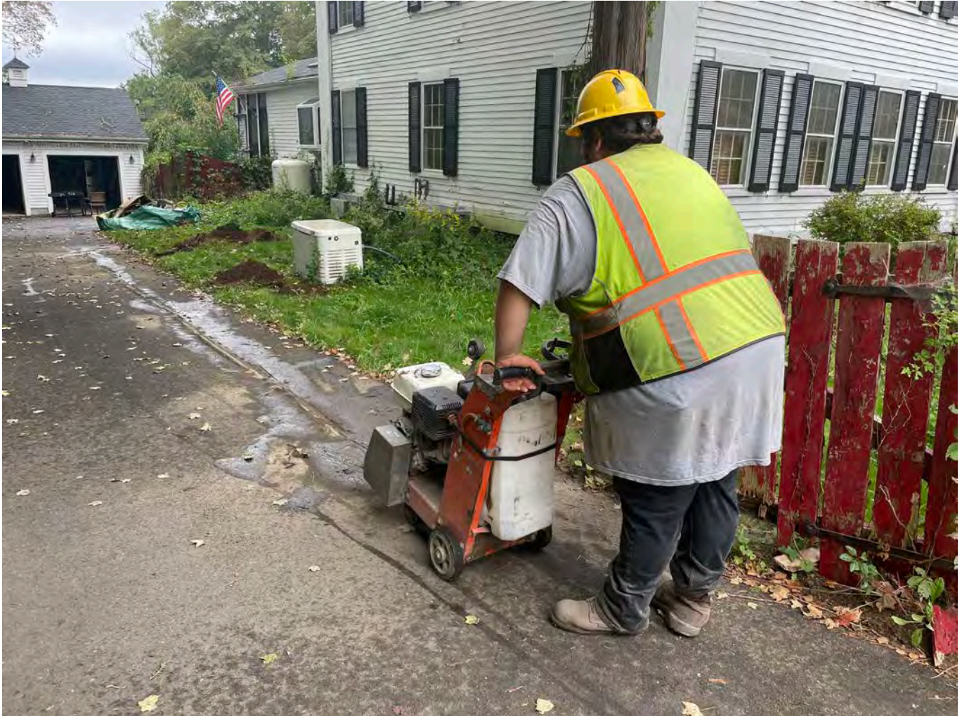
Picture 5: Ludlow saw cutting asphalt on the south side of the driveway of the 313 Main Street residence for the installation of a 1" copper water service line. View to the southeast.
