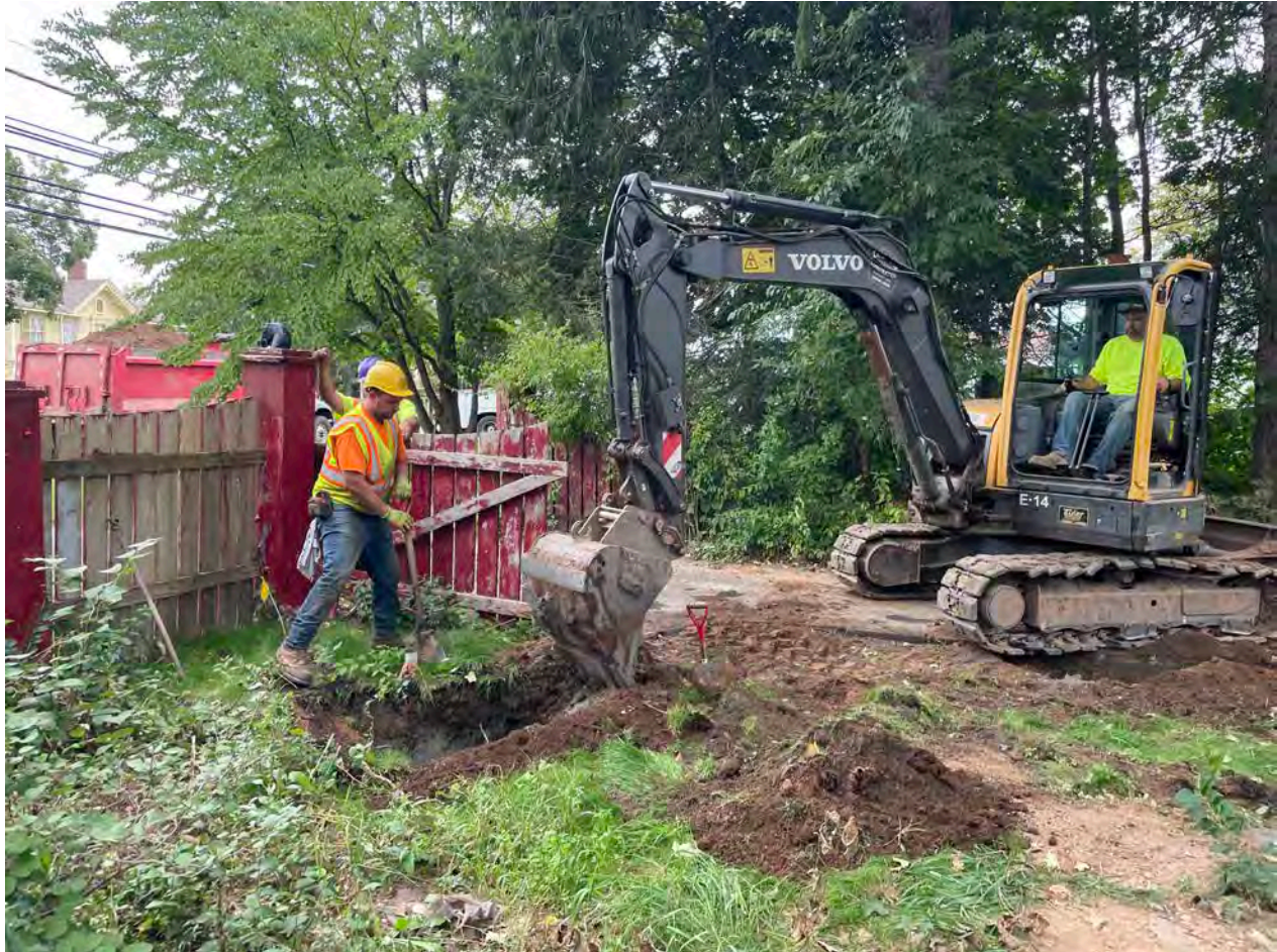
Picture 7: Ludlow excavating next to the curb stop for the 313 Main Street residence for the installation of a 1" copper water service line. View to the northwest.
