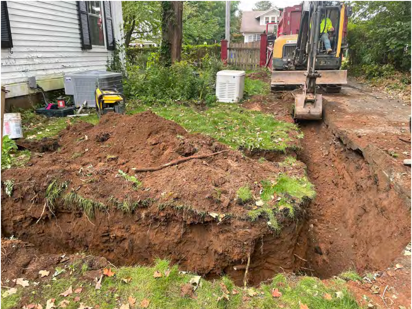
Picture 6: Ludlow excavating a trench on the north side of the 313 Main Street residence for the installation of a 1" copper water service line. View to the east.
