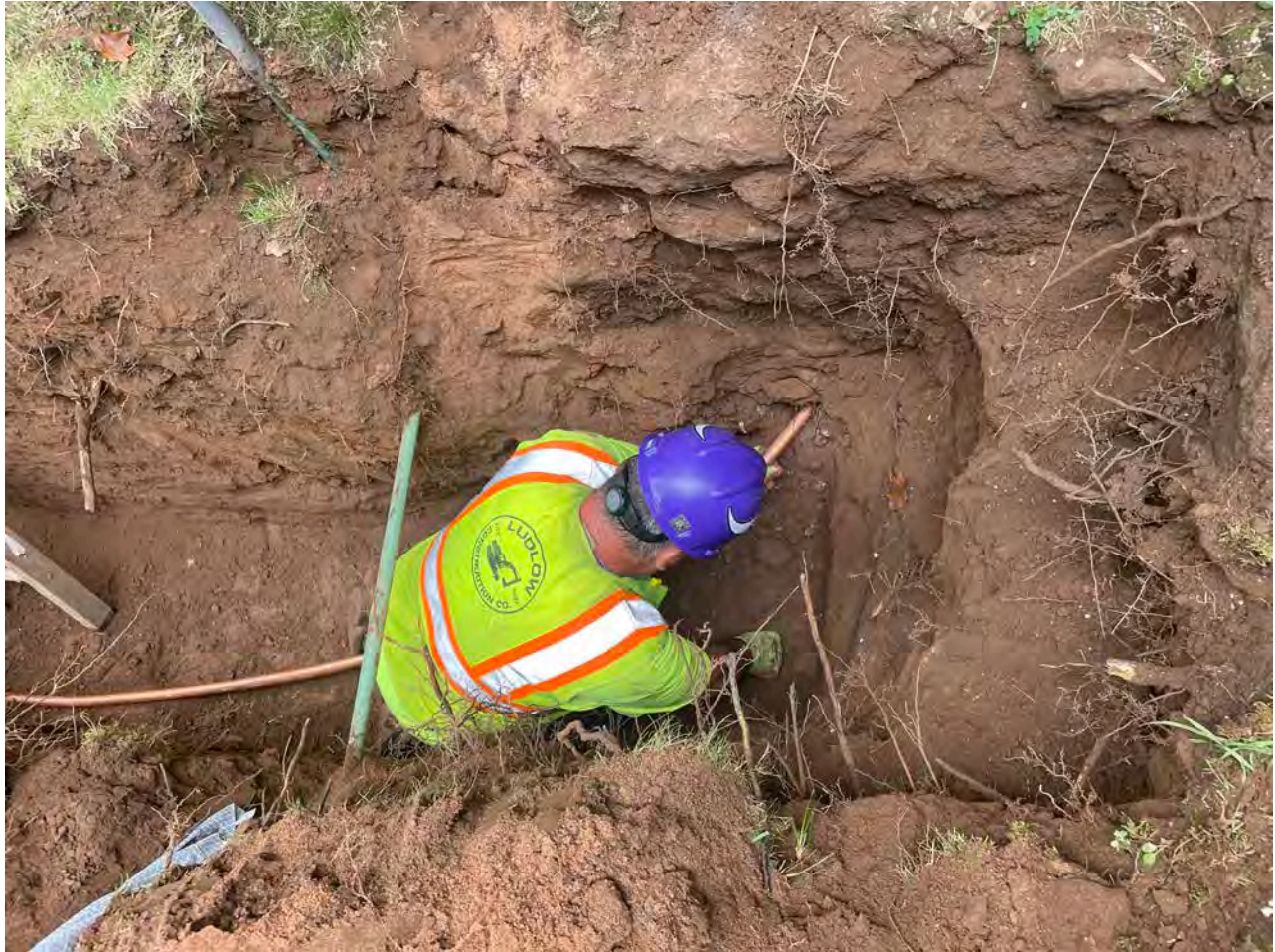
Picture 3: Ludlow inserting 1” copper water service line through a penetration they made through the north side of the foundation of the 316 Main Street residence.
