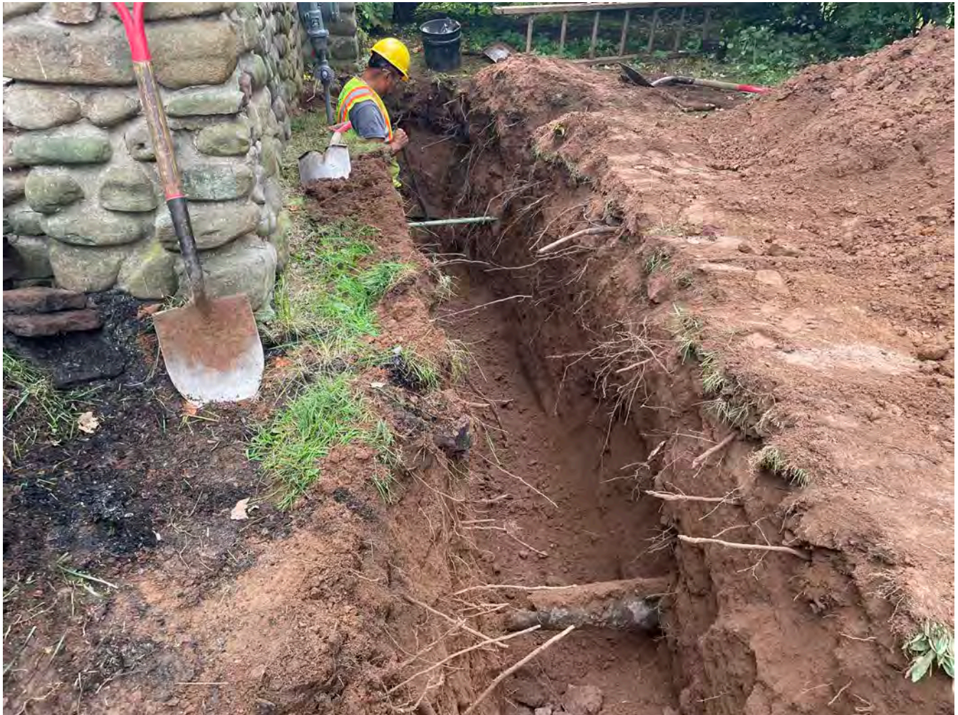
Picture 1: Trench that Ludlow excavated on the north side of the 316 Main Street, Durham, residence for the installation of a 1" copper water service line. View to the west.
