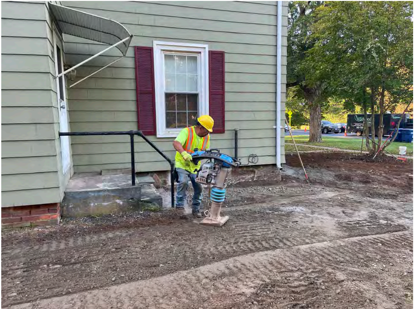
Picture 1: Ludlow compacting sand on the north side of the 303A/303B Main Street, Durham, residence. View to the southwest.
