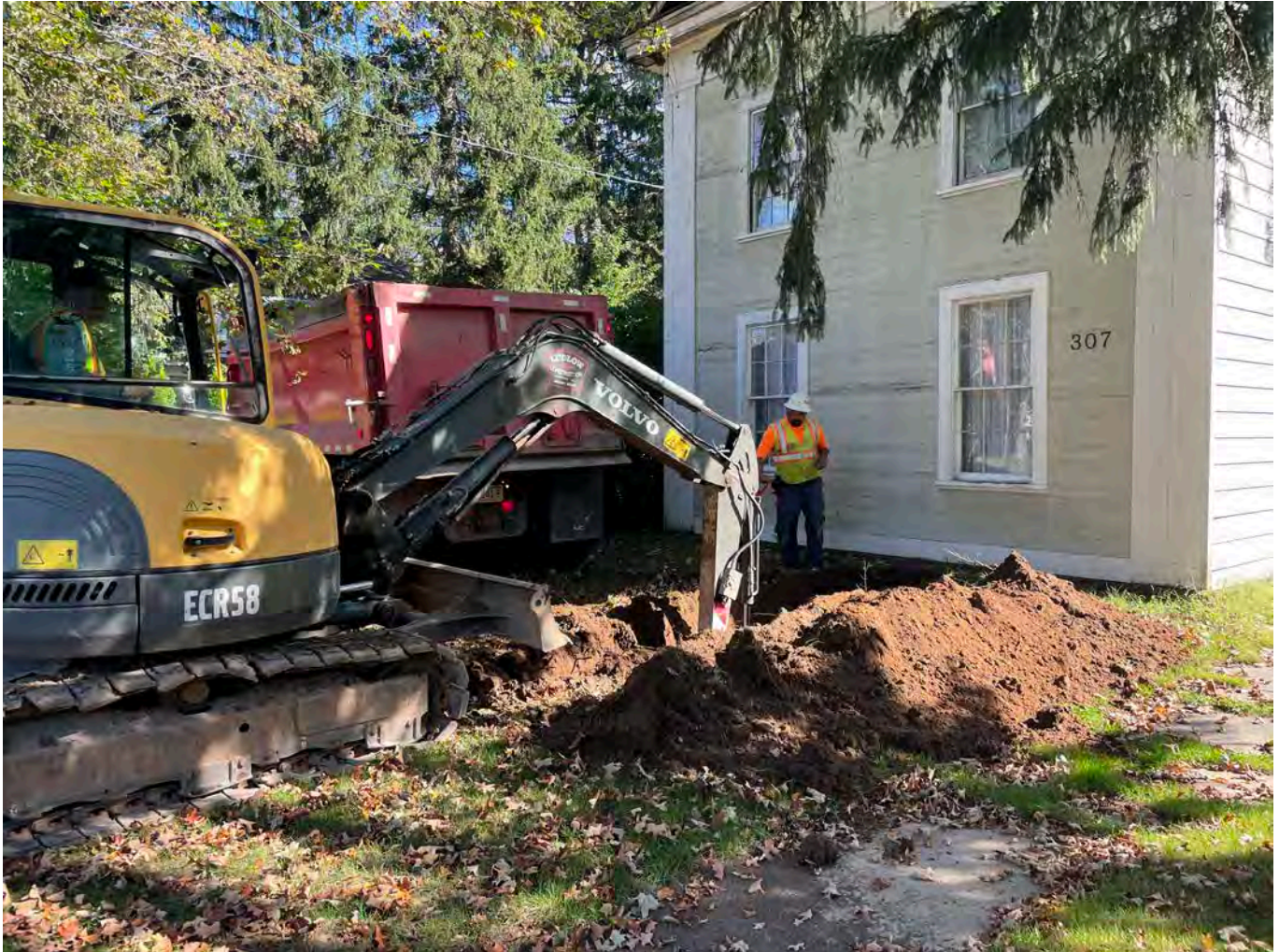
Picture 5: Ludlow excavating for the installation of a 1" copper water service line on the west side of the 307 Main Street residence. View to the northeast.
