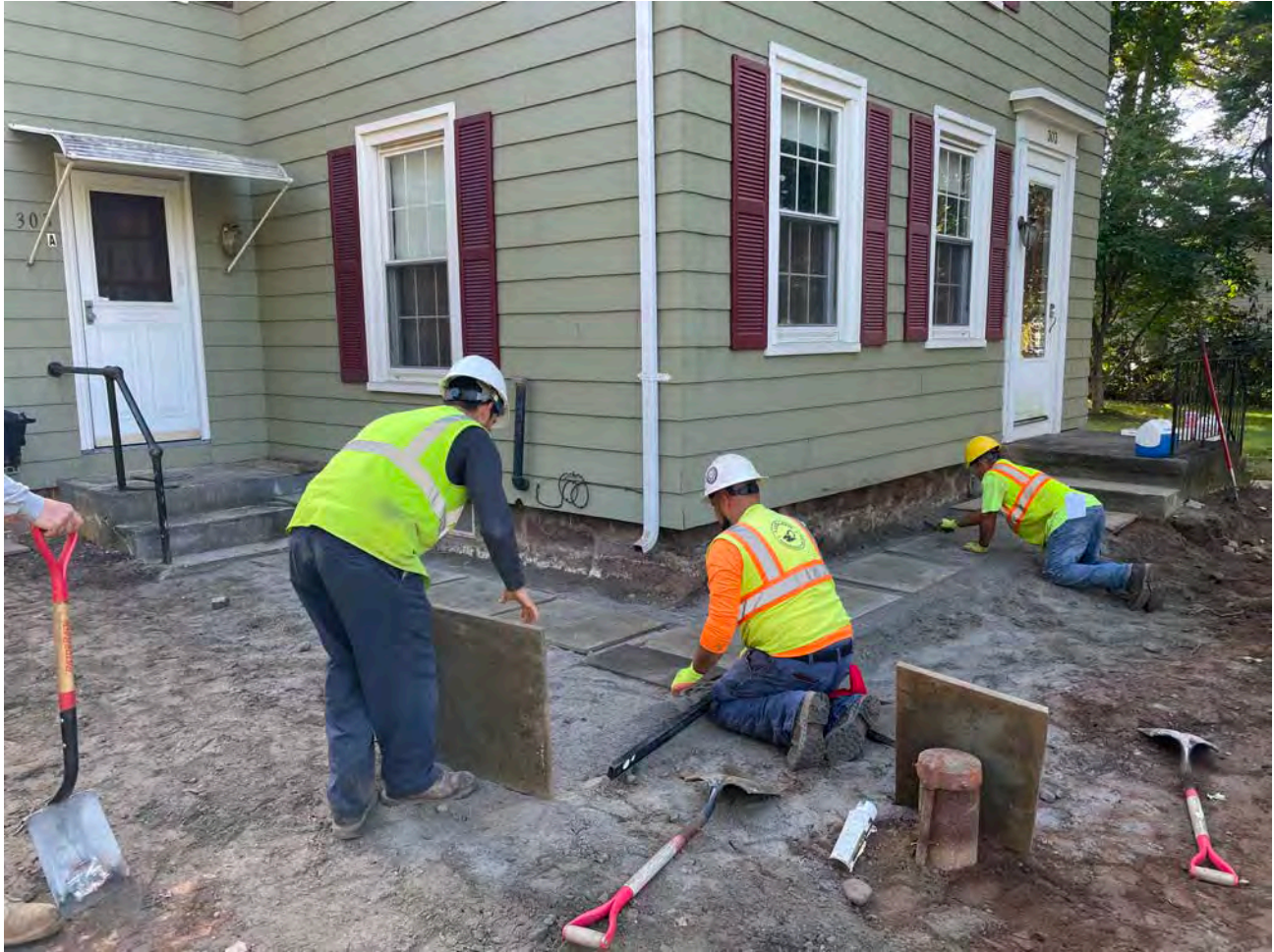
Picture 2: Ludlow replacing pavers on the northwest corner of the 303A/303B Main Street, Durham, residence. View to the southeast.
