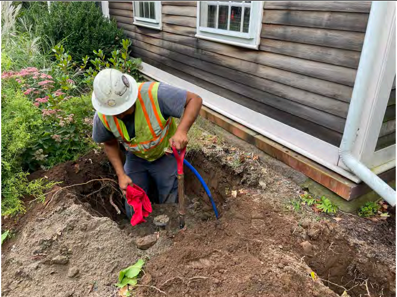
Picture 9: Ludlow daylighting the eastern foundation of the 308 Main Street residence to install a 1" copper water service line at the residence. View to the southwest.
