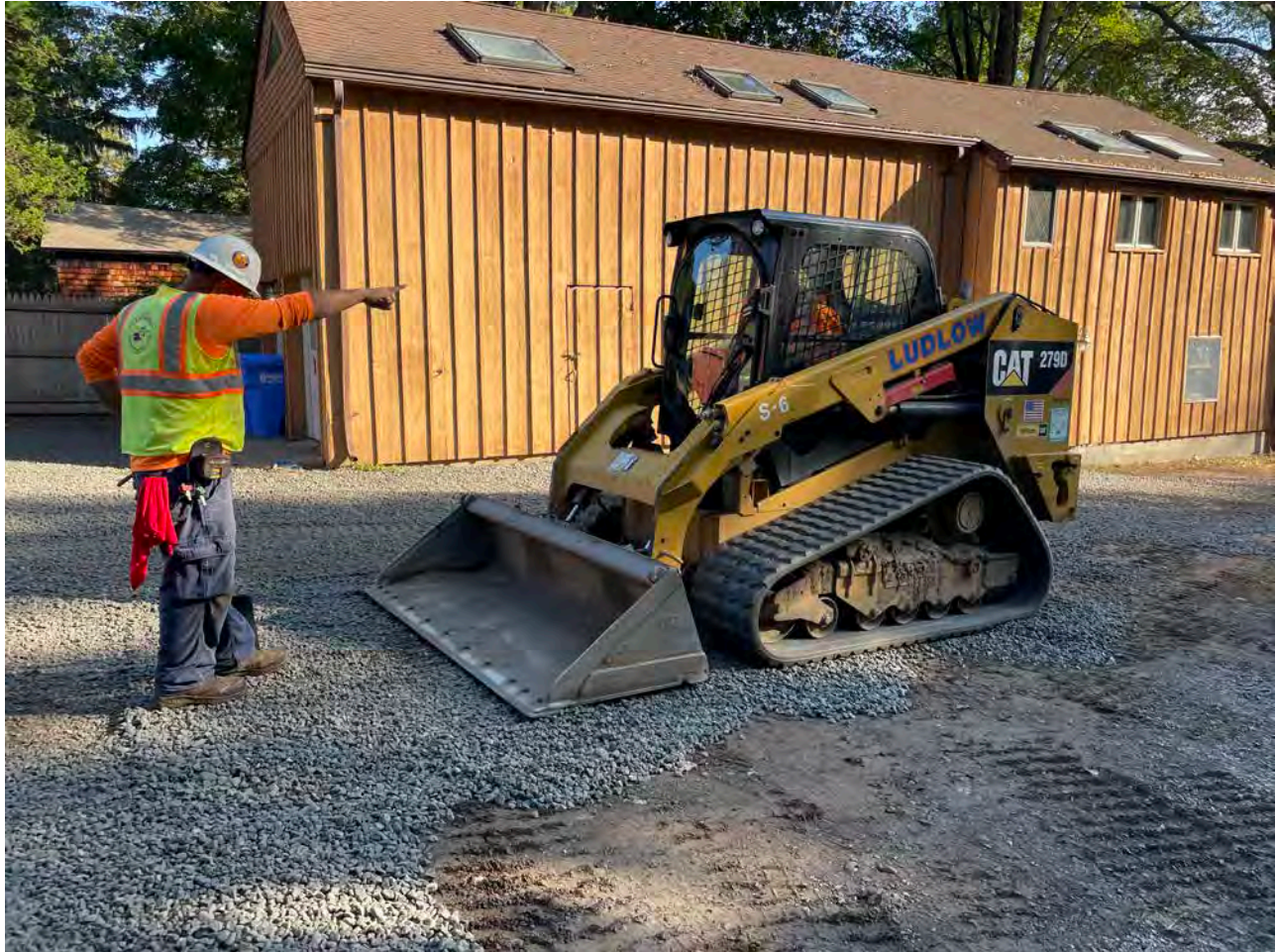
Picture 3: Ludlow grading ¾” stone they placed on the portion of the driveway located between the 303A/303B Main Street residence and the 305R Main Street residence. View to the north.
