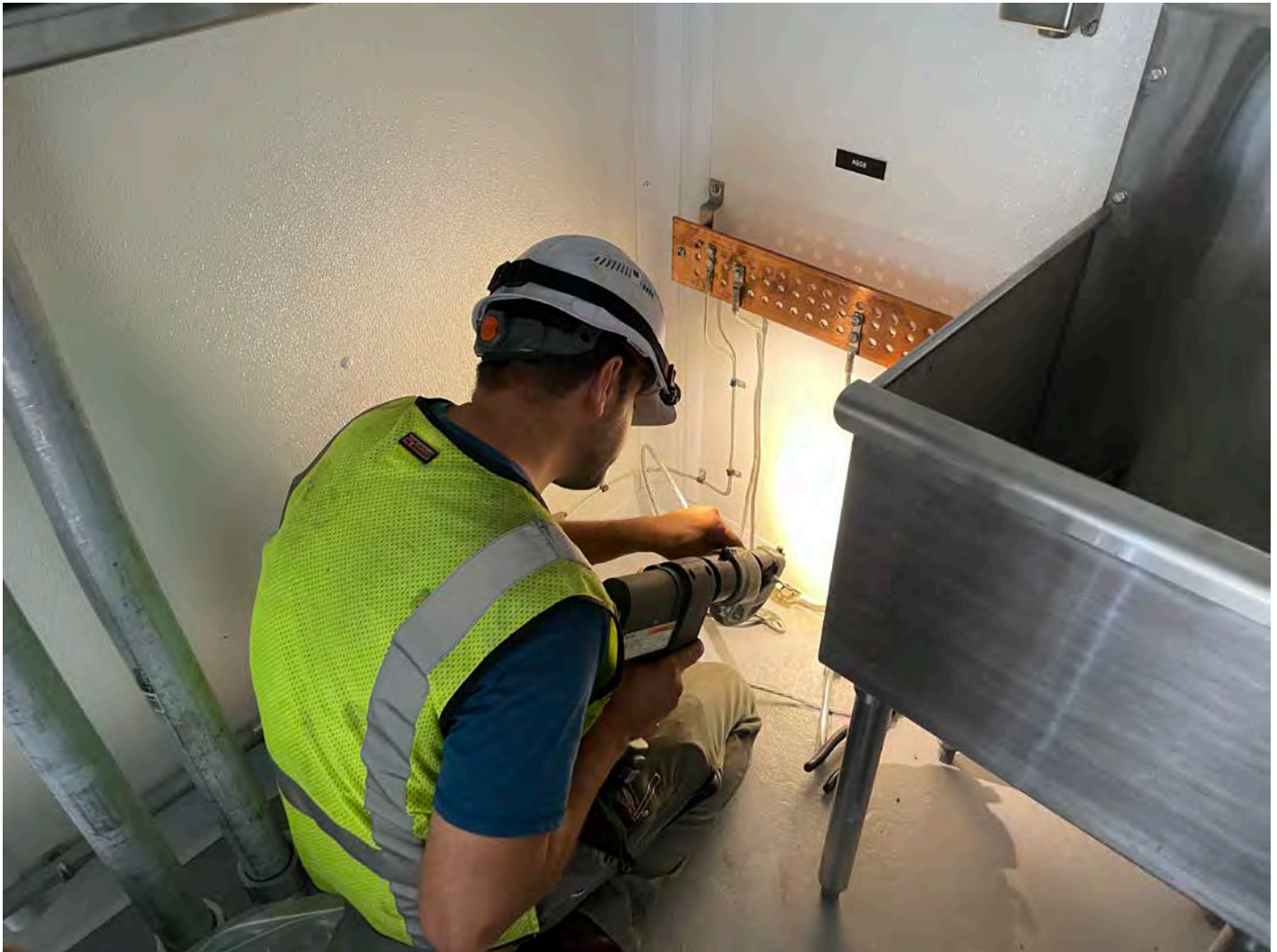
Picture 4: A&R Electrical installing a grounding line at the northeast corner of the booster station interior. View to the northeast.
