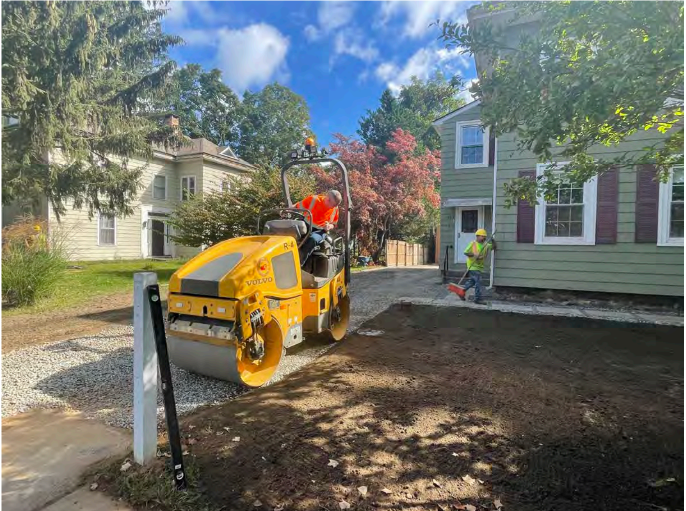
Picture 6: Ludlow compacting ¾" stone that they placed on the driveway of the 303A/303B Main Street residence. View to the northeast.
