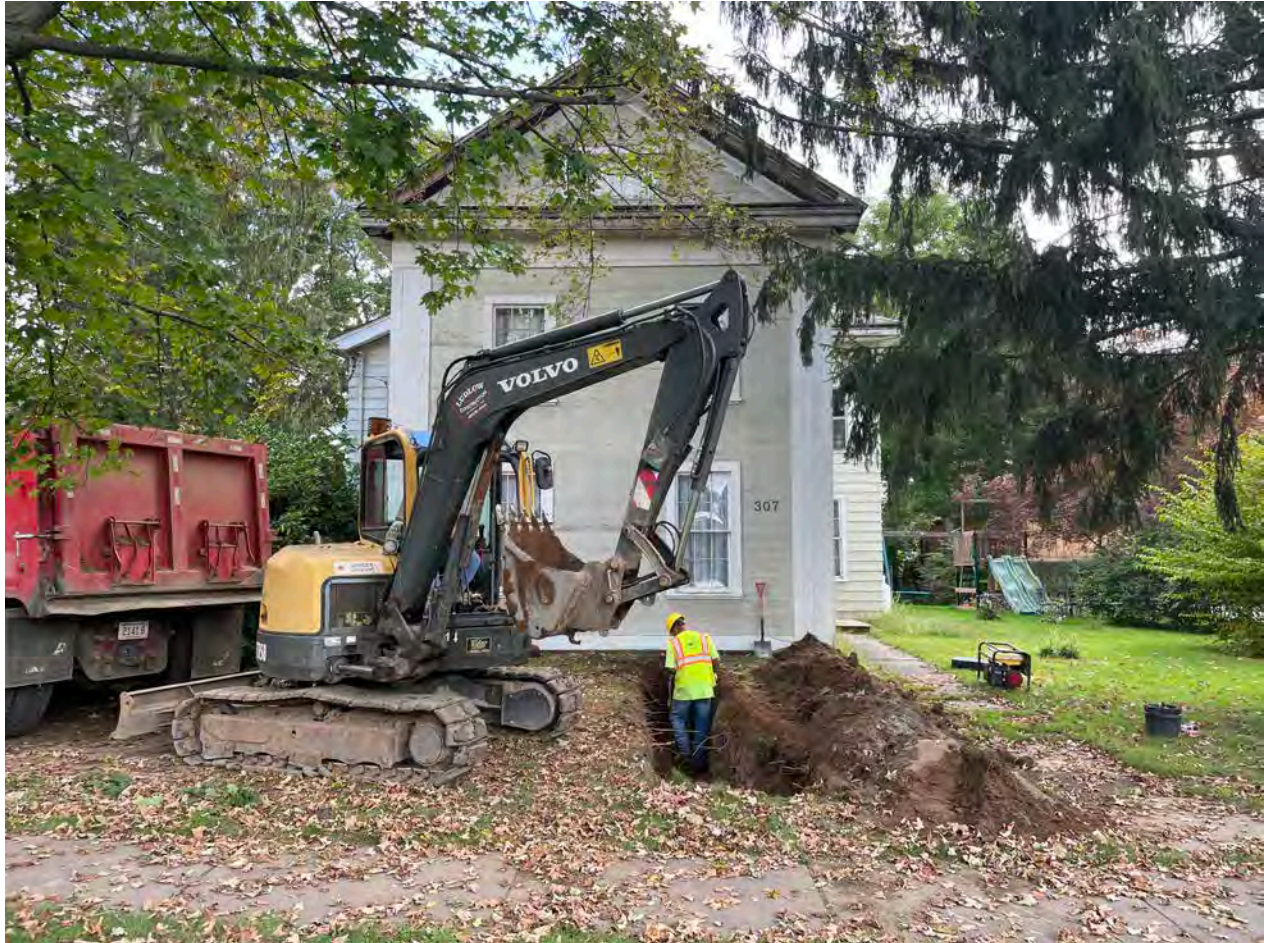
Picture 7: View of the excavation that Ludlow has made for the installation of a 1" copper water service line on the west side of the 307 Main Street residence. View to the east.
