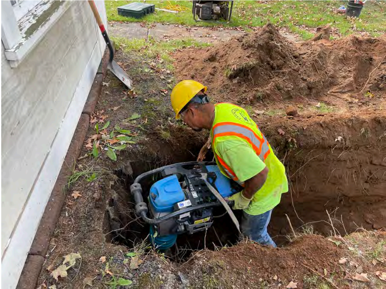
Picture 8: Ludlow compacting native fill that has been placed over the caution tape and sand that they placed over the 1" copper water service line at the 307 Main Street residence. View to the south.
