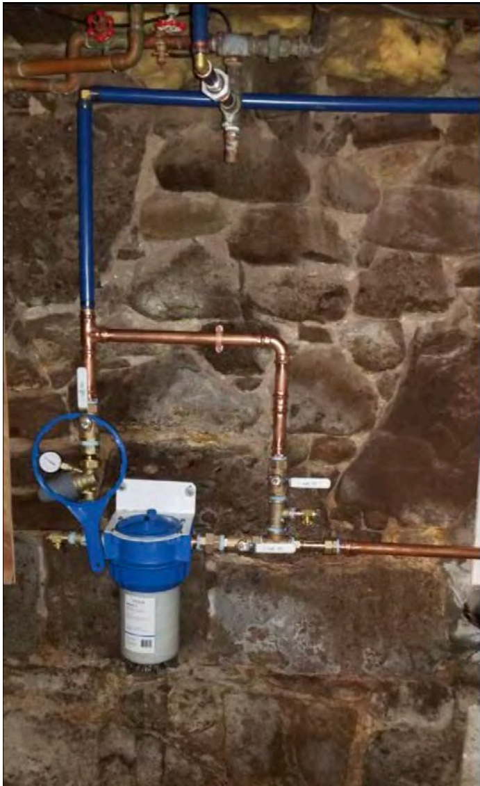
Picture 12: Final water service components that Fazzino Plumbing installed today at the residence located at 303 Maple Avenue, Durham. (Photo on right is of submeters)
