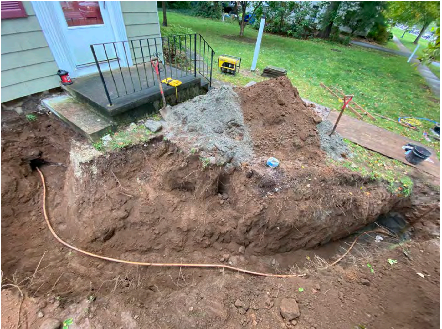
Picture 2: The complete connection of the 1" copper service line for the 305 Main Street residence.
