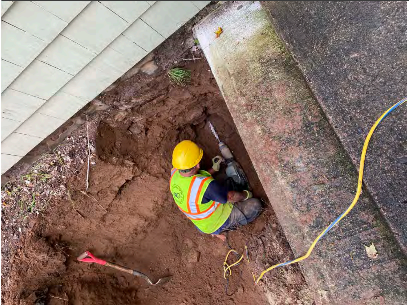
Picture 1: Ludlow drilling through the western foundation of the 305 Main Street residence with a rotary hammer.
