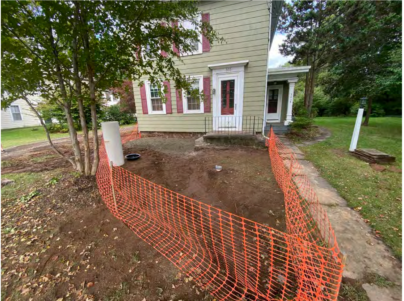
Picture 11: Ludlow places a safety fence around the trench South of the 303 Main Street residence.
