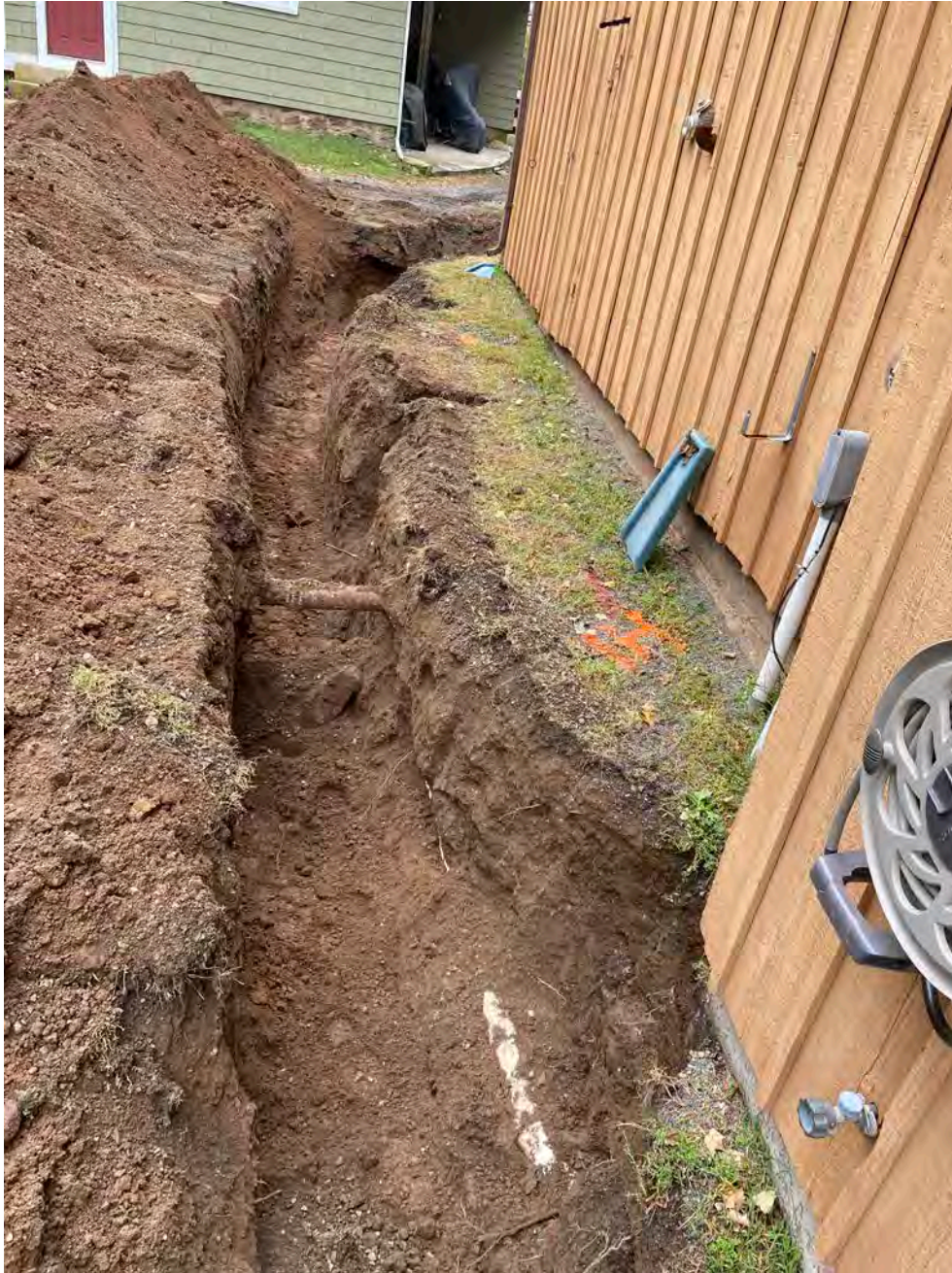
Picture 6: Ludlow excavates on the South side of residence 305R Main Street and locates the point of connection of the existing well to the residence.
