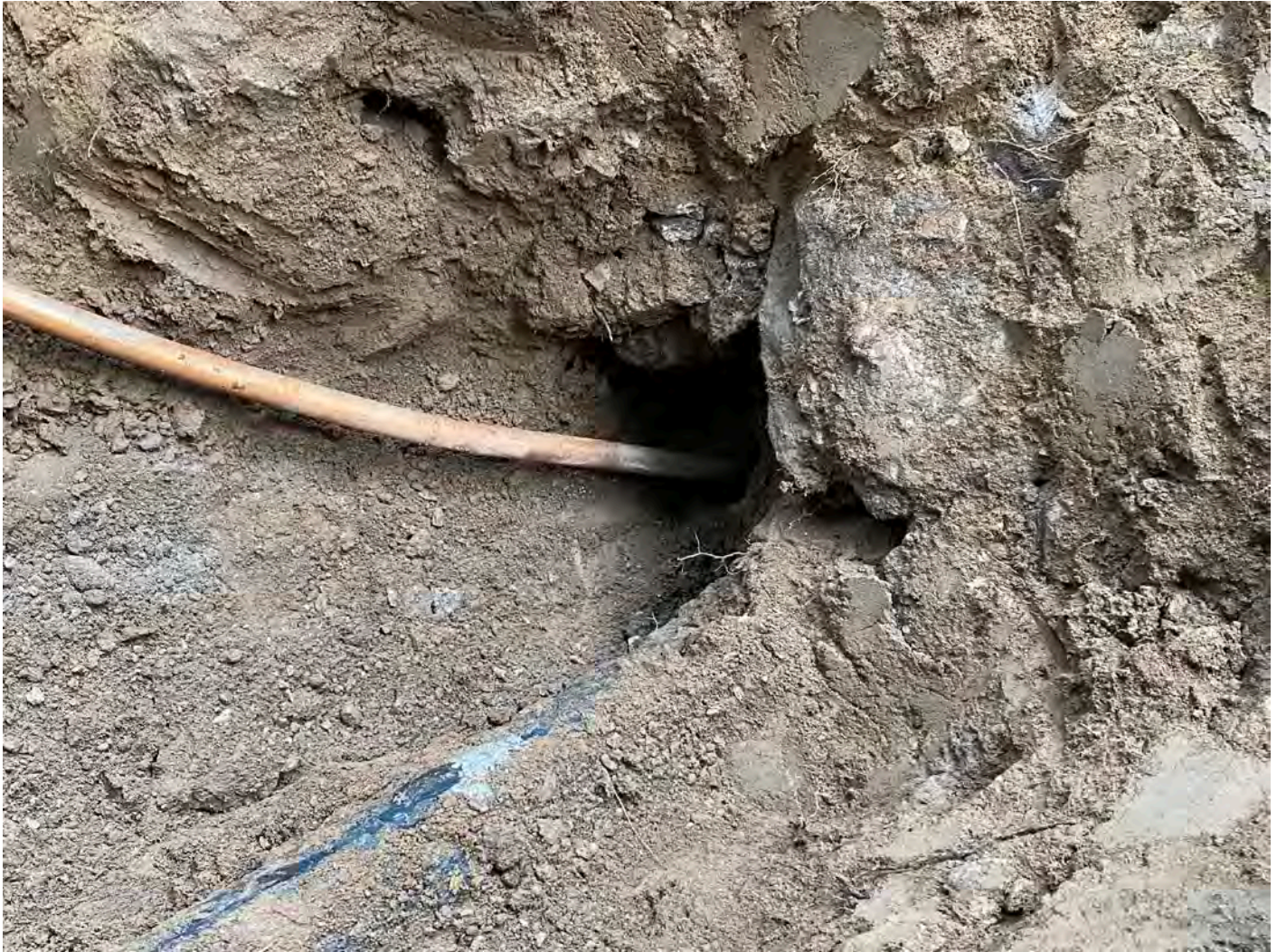
Picture 3: Ludlow connecting 1" copper water service line to the house for the 303 Main Street residence property in Durham.
