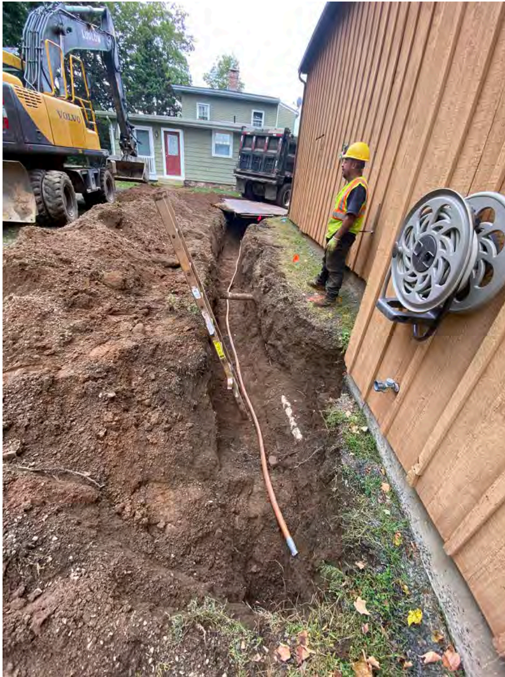
Picture 7: Ludlow placing a segment of the 1.5" copper service line in the trench for the 305R Main Street residence property in Durham.
