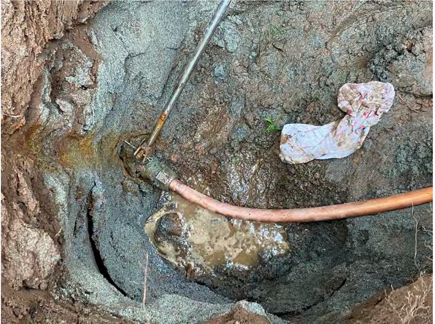
Picture 4: Ludlow connecting 1" copper water service line to the curb stop for the 303 Main Street residence property in Durham.
