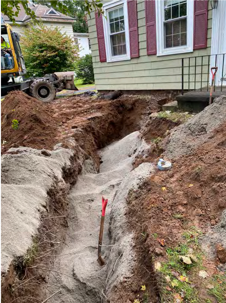
Picture 5: Ludlow places sand on top of the new 1” copper water service line for the 303 Main Street residence.
