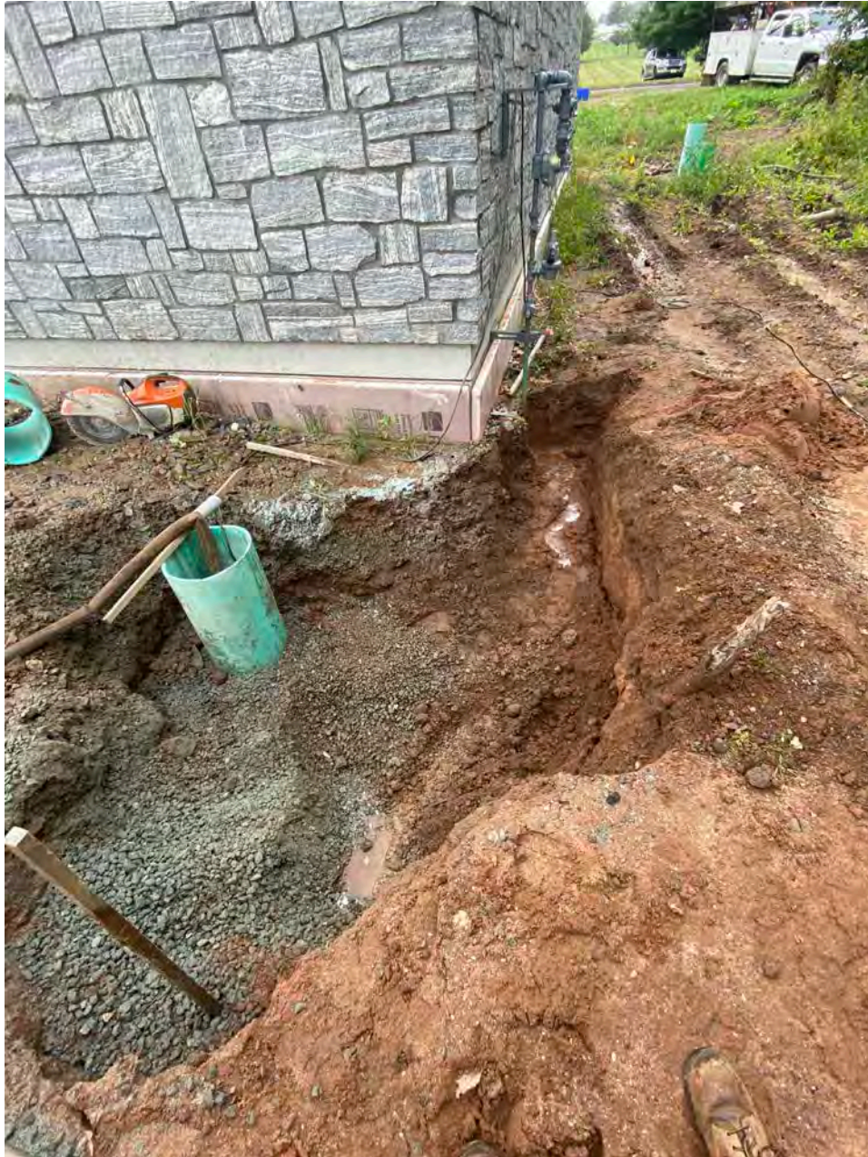
Picture 4: Ludlow excavates trench from the generator set to the Booster Station for gas line connection. View to the east.
