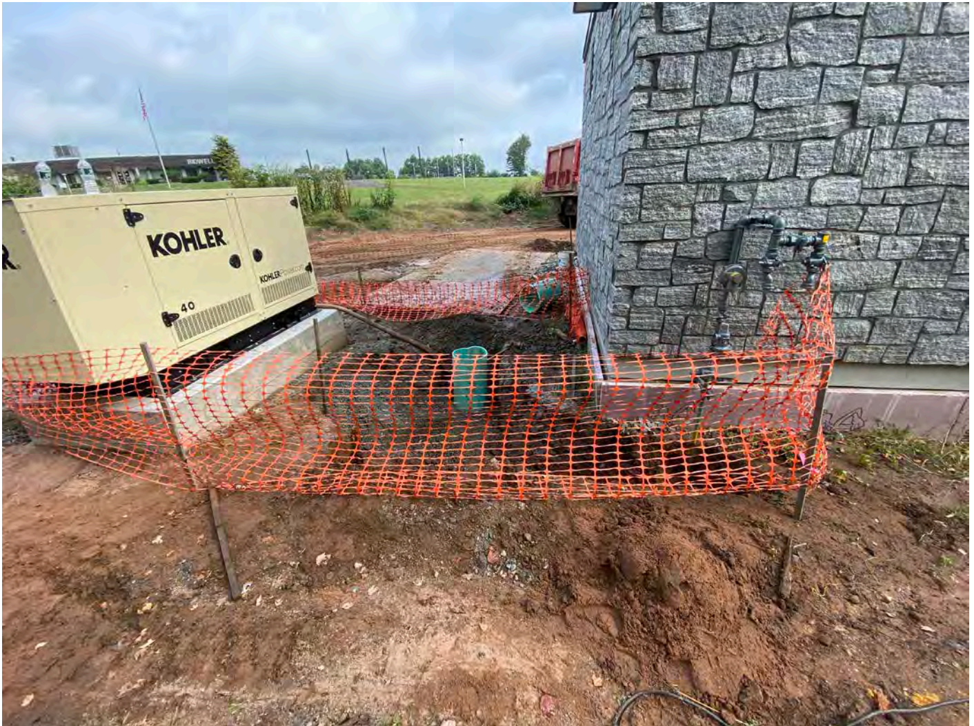
Picture 6: Ludlow puts up a safety fence around trench for gas line connection at the Booster Station. View to the north.
