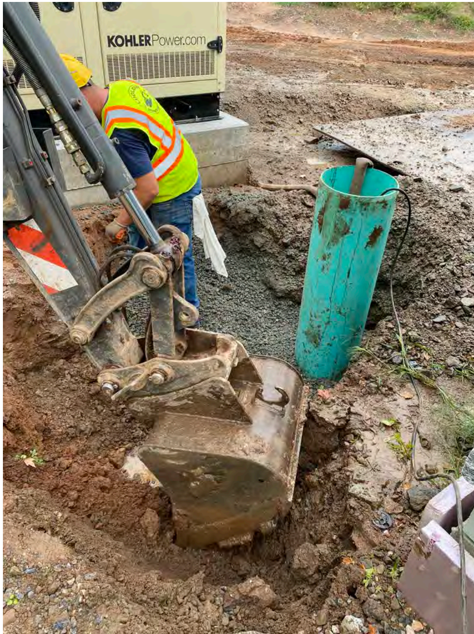
Picture 1: Ludlow creates a sump to pump out some water and continues excavating for the gas line for connection from the Booster Station to the generator. View to the northwest.
