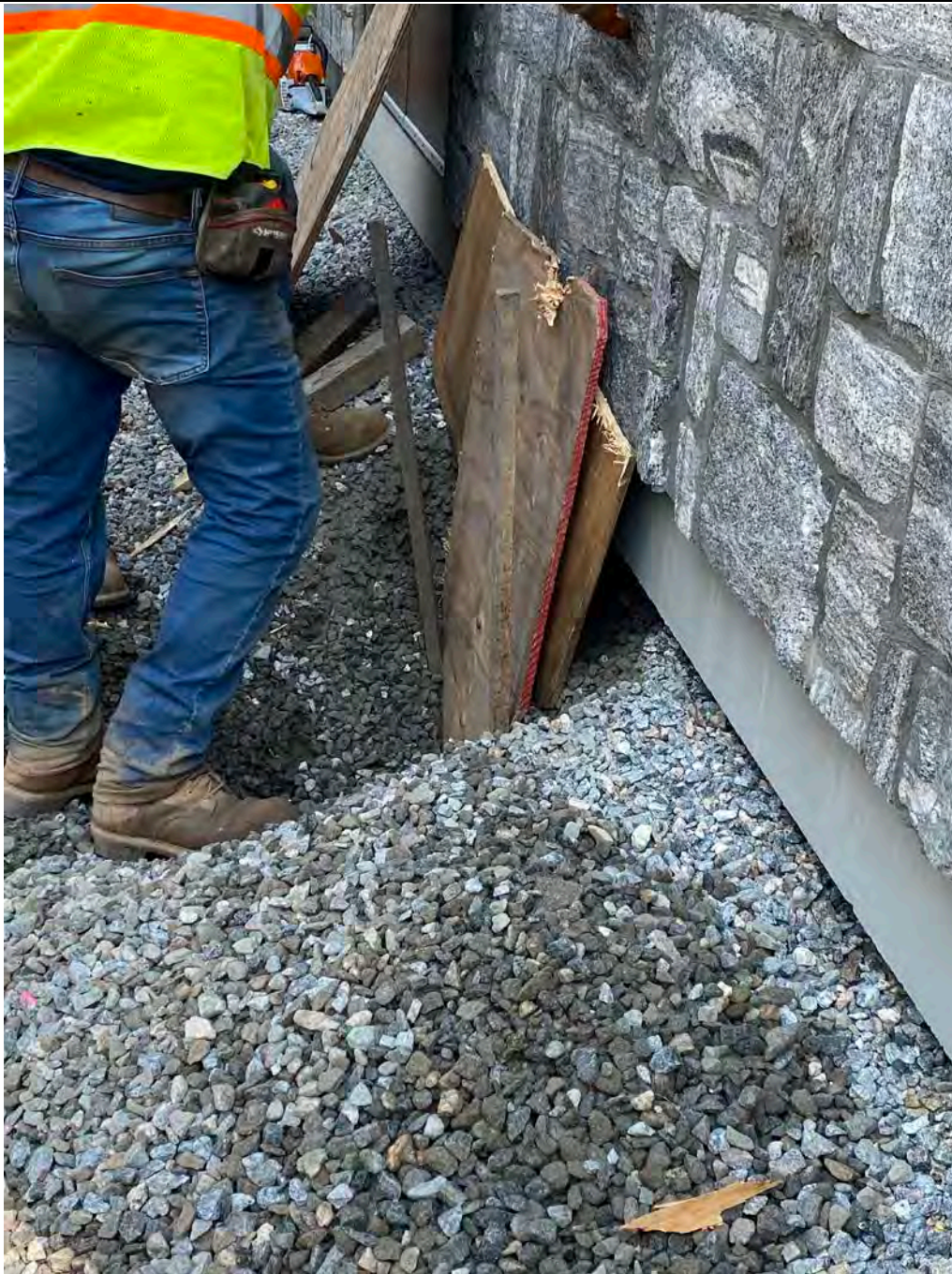
Picture 9: Ludlow constructs and inserts a temporary wall against the Meter Vault to restrain loose aggregate upon excavation. View to the north.
