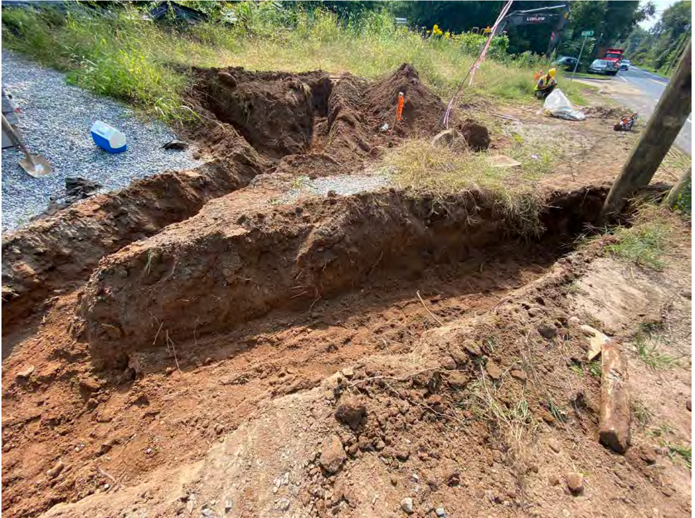
Picture 8: Ludlow excavates trench for power and communication connection to the Meter Vault, South Main Street, Middletown. View to the south.
