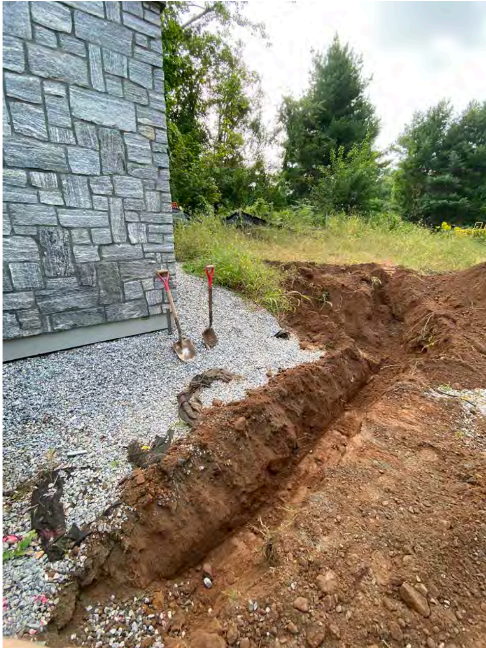
Picture 7: Ludlow excavating a trench for electrical grounding grid at the Meter Vault, South Main Street, Middletown. View to the south.
