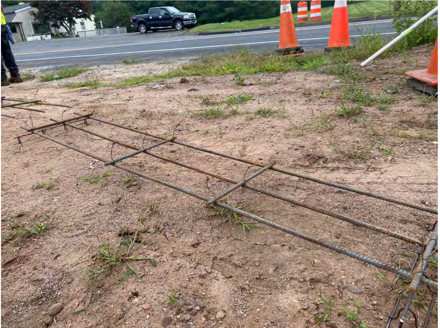
Picture 5: Ludlow assembles reinforcing cage for electric conduit at the Booster Station.
