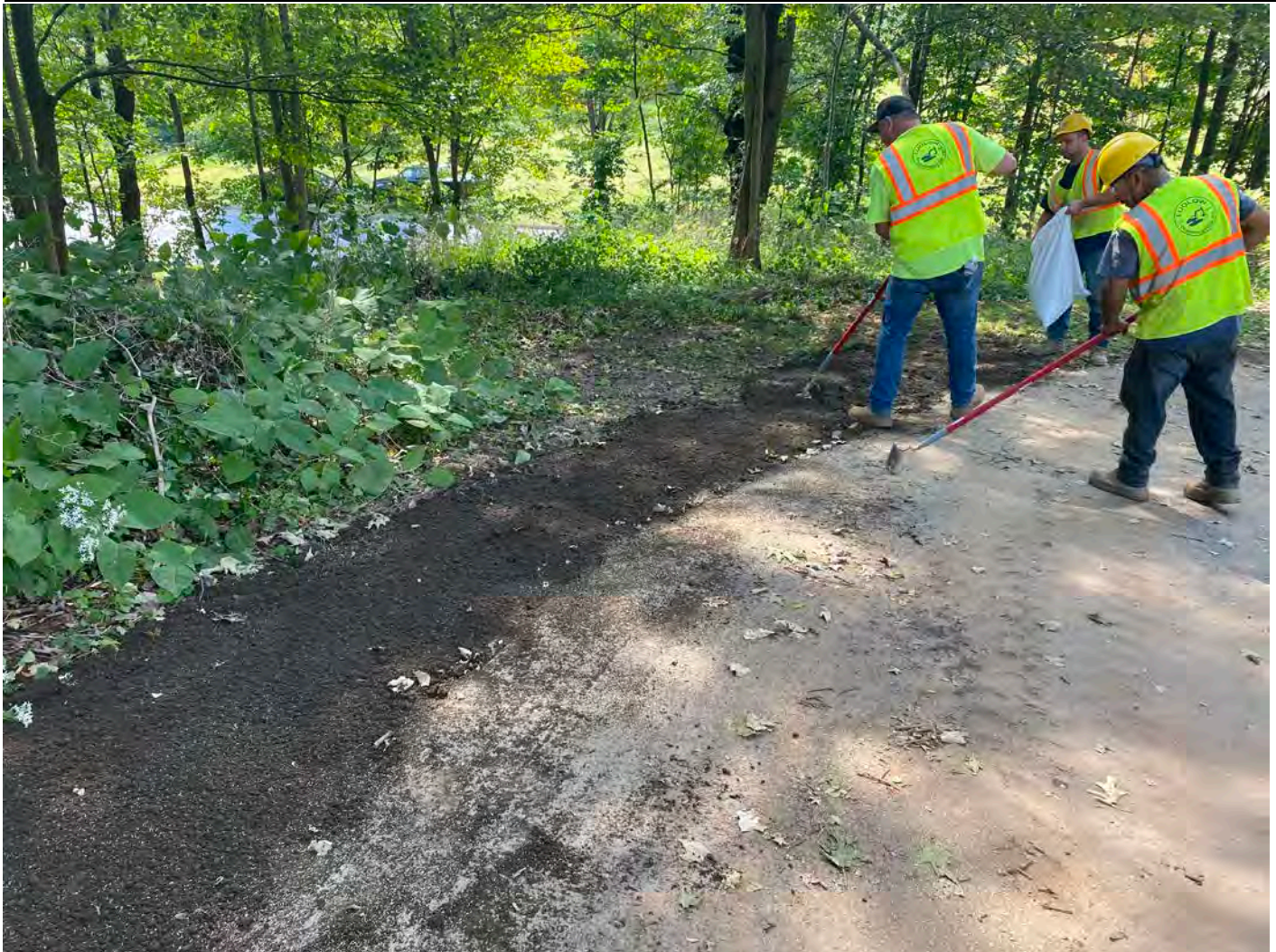
Picture 11: Ludlow placing loam and seed on the areas of the 95R Maple Avenue property that were disturbed during the installation of water service line. View to the west.
