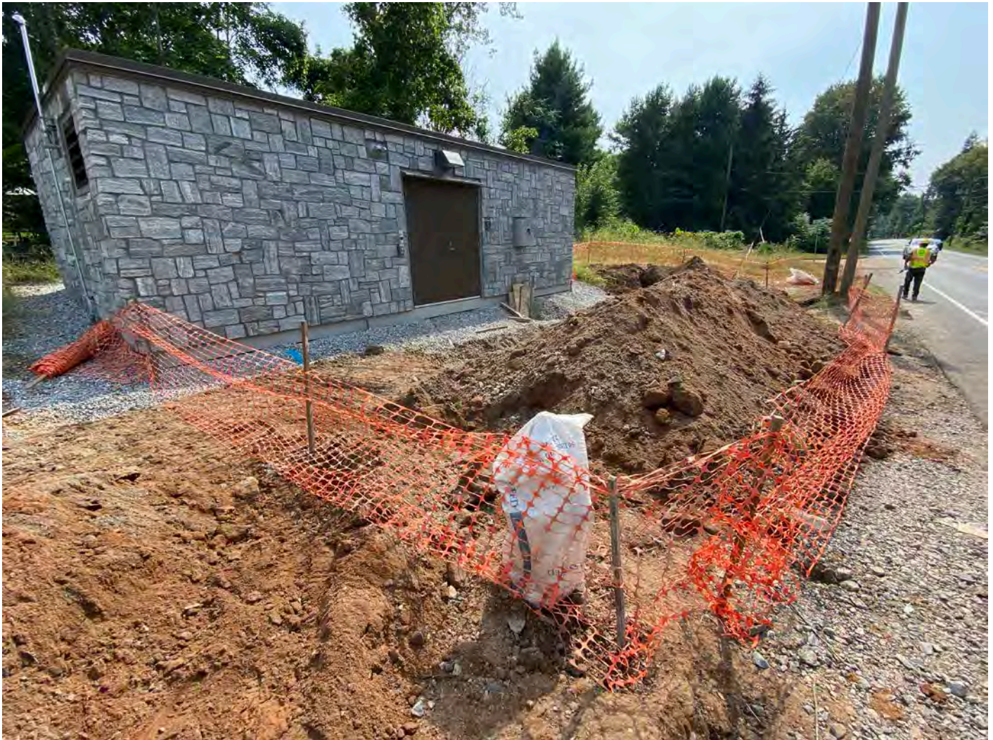
Picture 10 : Ludlow puts up a safety fence around the open trench for grounding grid and electric connection at the Meter Vault. View to the south.
