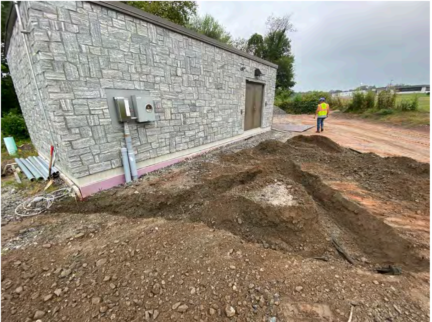
Picture 2: Ludlow excavating a trench for electrical grounding grid at the Booster Station in Middletown. View to the west.
