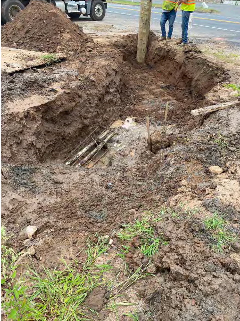
Picture 3: Ludlow locates and exposes existing electrical conduit and excavates the rest of the trench to the utility pole at the Booster Station. View to the northeast.
