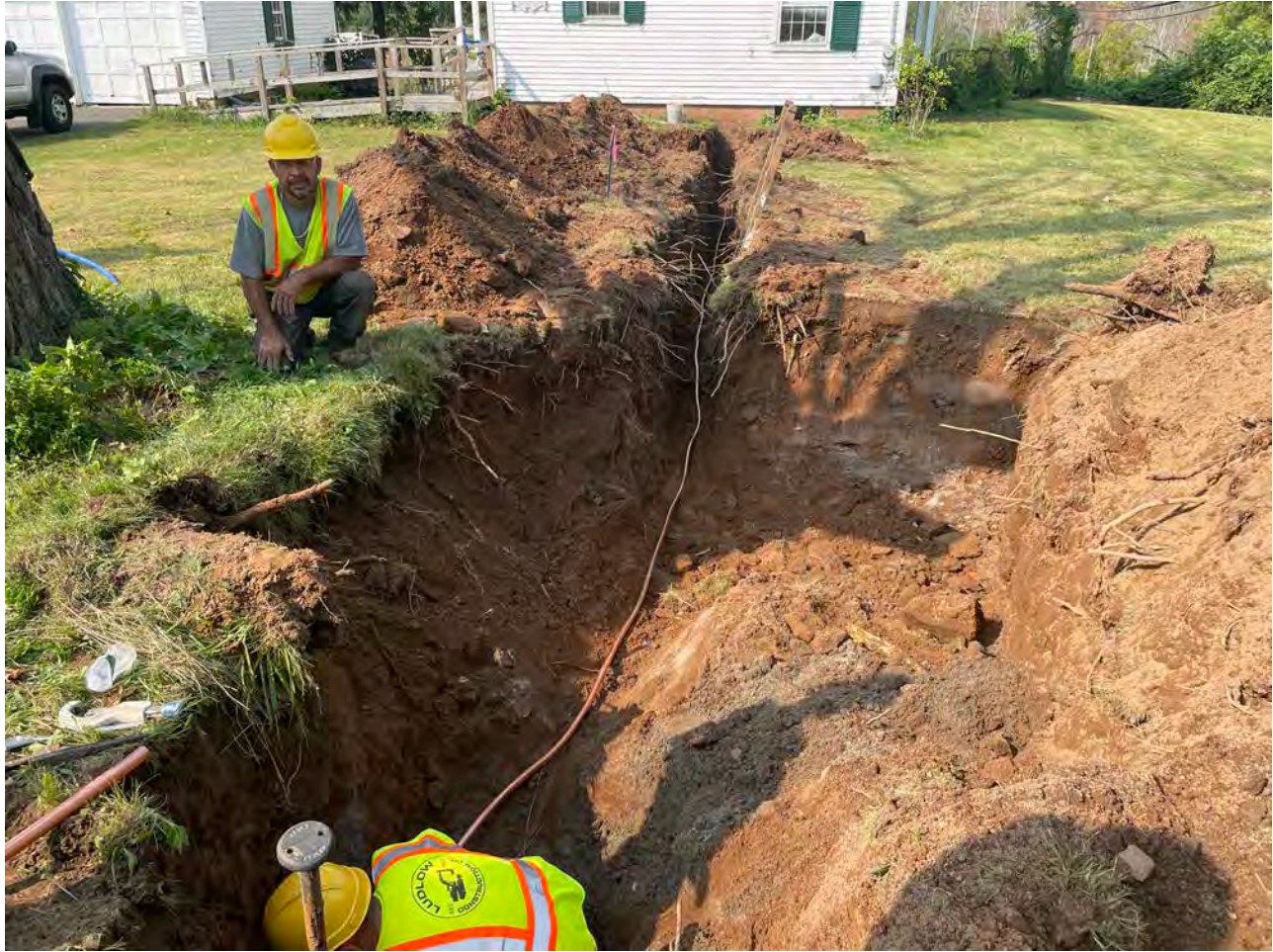
Picture 3: Ludlow placing 1" copper water service line in the trench they excavated at the 148 Maple Avenue property in Durham. View to the west.
