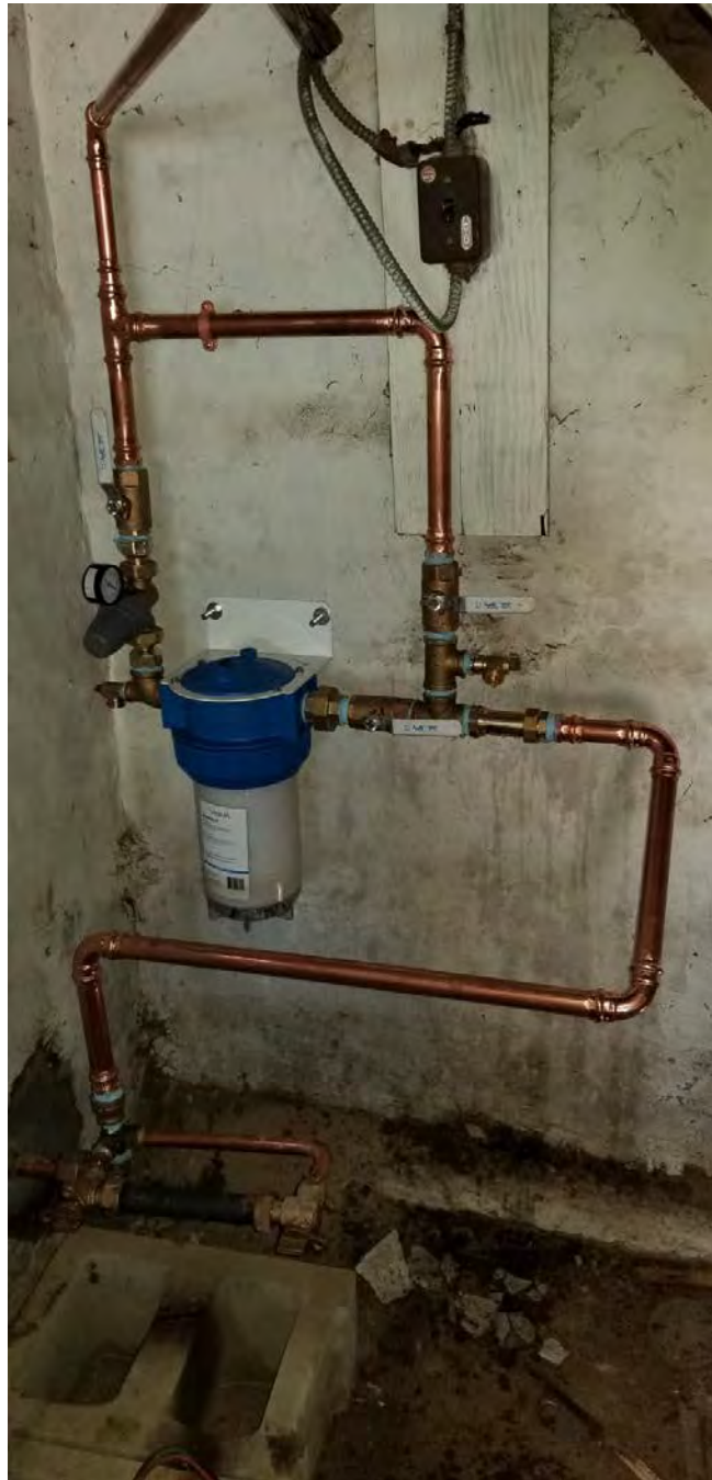
Picture 12: Final water service components that Fazzino Plumbing installed today at the residence located at 47 Wallingford Road, Durham.
