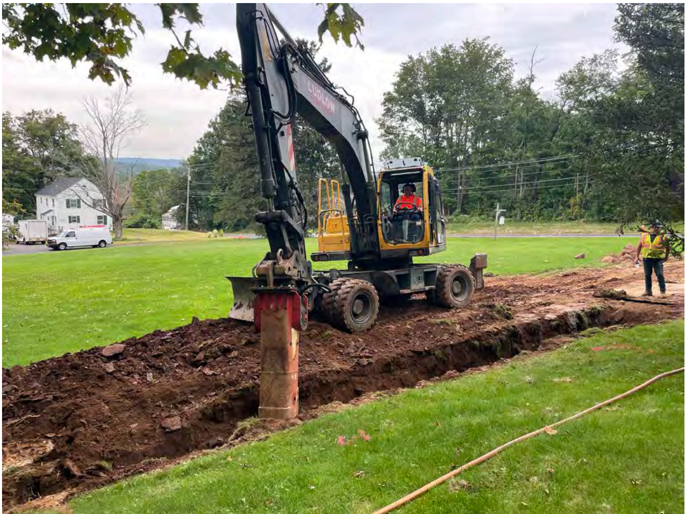
Picture 1: Ludlow breaking up rock as they continue to excavate a trench at the 22 Wallingford Road, Durham, residence for the installation of a 1.5" copper water service line. View to the northwest.
