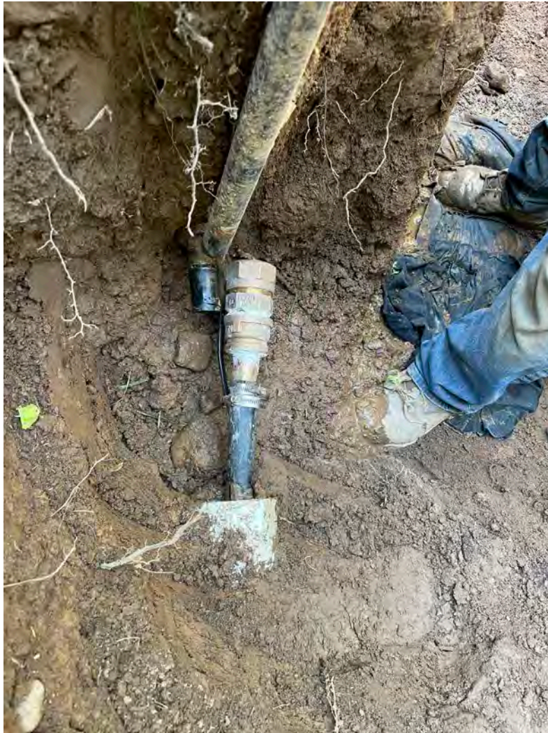
Picture 8: Brass fitting that Ludlow connected to the 1" HDPE well water line that penetrates the western foundation of the 22 Wallingford Road property in Durham. Ludlow ended up connecting the 1.5" copper water service line to the compression fitting located on the opposite end of the brass fitting.
