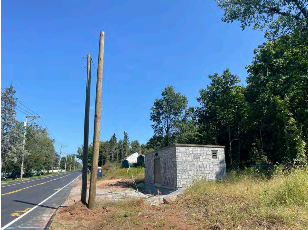
Picture 7: One pole that Frontier installed today at the water meter building. View to the north.
