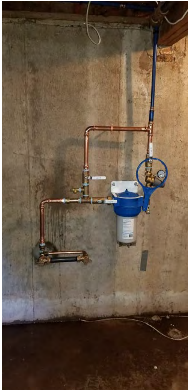
Picture 10: Final water service components that Fazzino Plumbing installed today at the residence located at 17 Wallingford Road, Durham.
