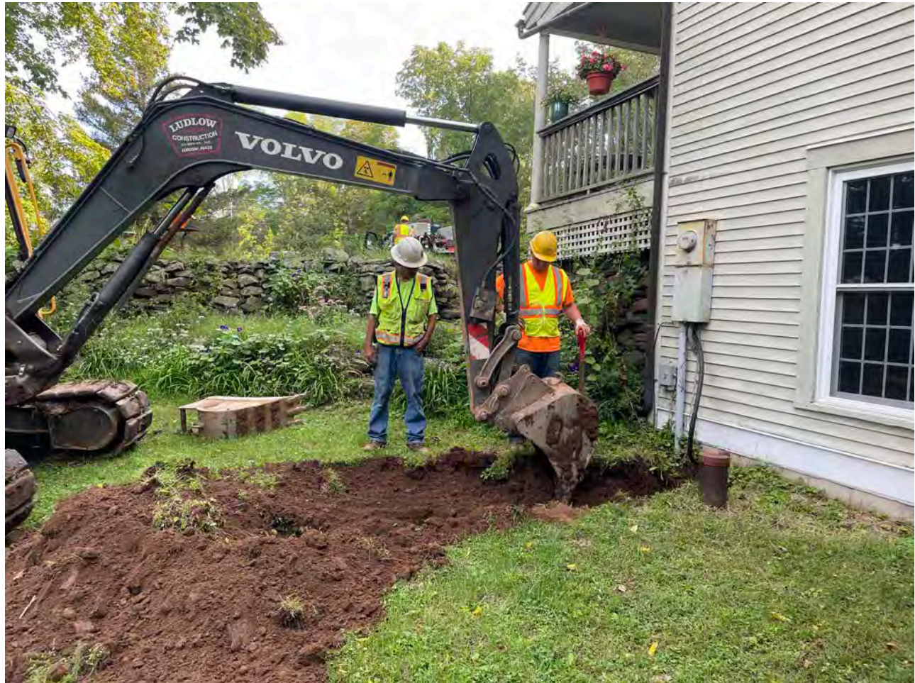
Picture 3: Ludlow excavating a trench on the west side of the residence located at 22 Wallingford Road for the installation of a 1.5" copper water service line. View to the northeast.
