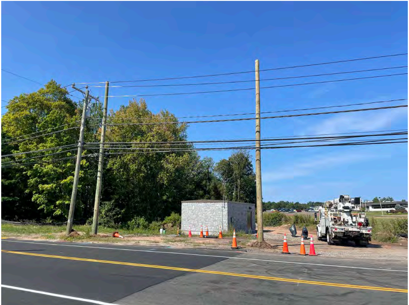
Picture 6: Two poles that Frontier installed today at the booster station. View to the west.
