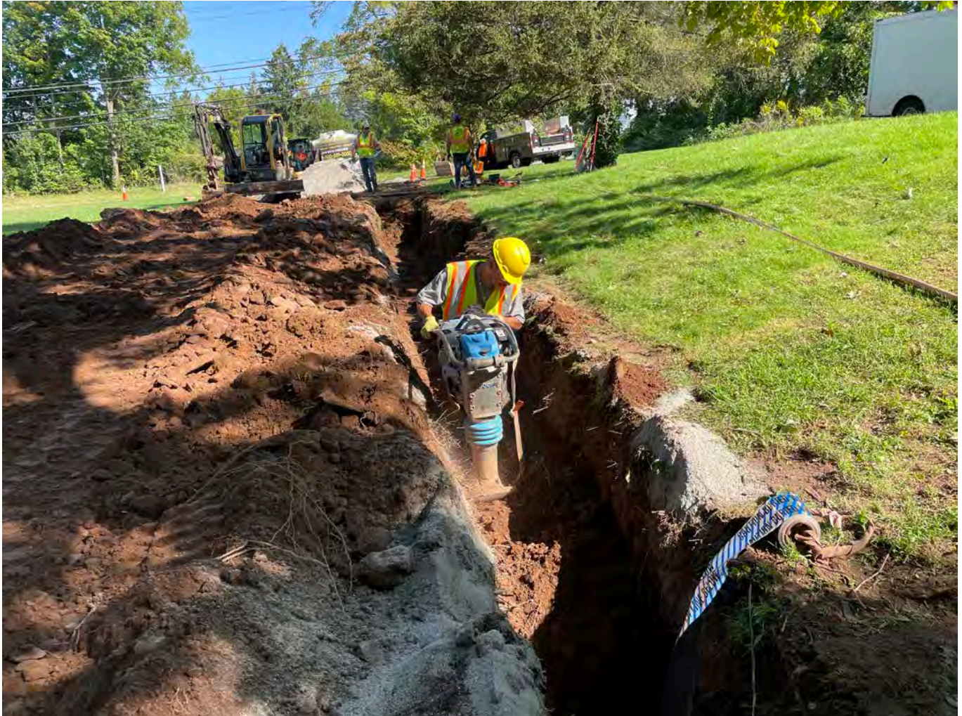
Picture 5: Ludlow compacting native fill that they placed over the sand and caution tape they placed over the 1.5" copper water service line they installed at the 22 Wallingford Road property. View to the north.
