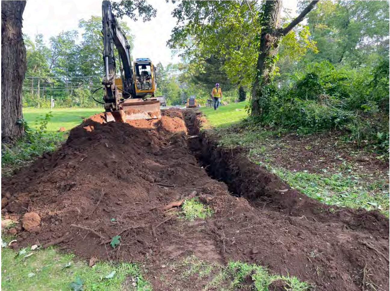
Picture 2: View of the trench that Ludlow is excavating at the 22 Wallingford Road, Durham, residence for the installation of a 1.5" copper water service line. View to the north.
