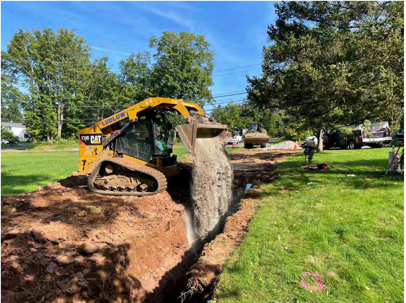
Picture 4: Ludlow placing sand over the 1.5” copper water service line they are installing at the 22 Wallingford Road, Durham, residence. View to the north.
