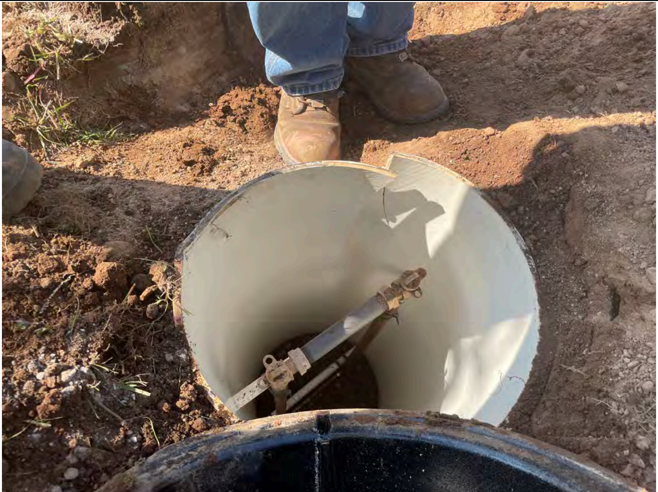
Picture 9: Meter pit located at the 22 Wallingford Road property that was damaged when one of the construction trucks backed over it.
