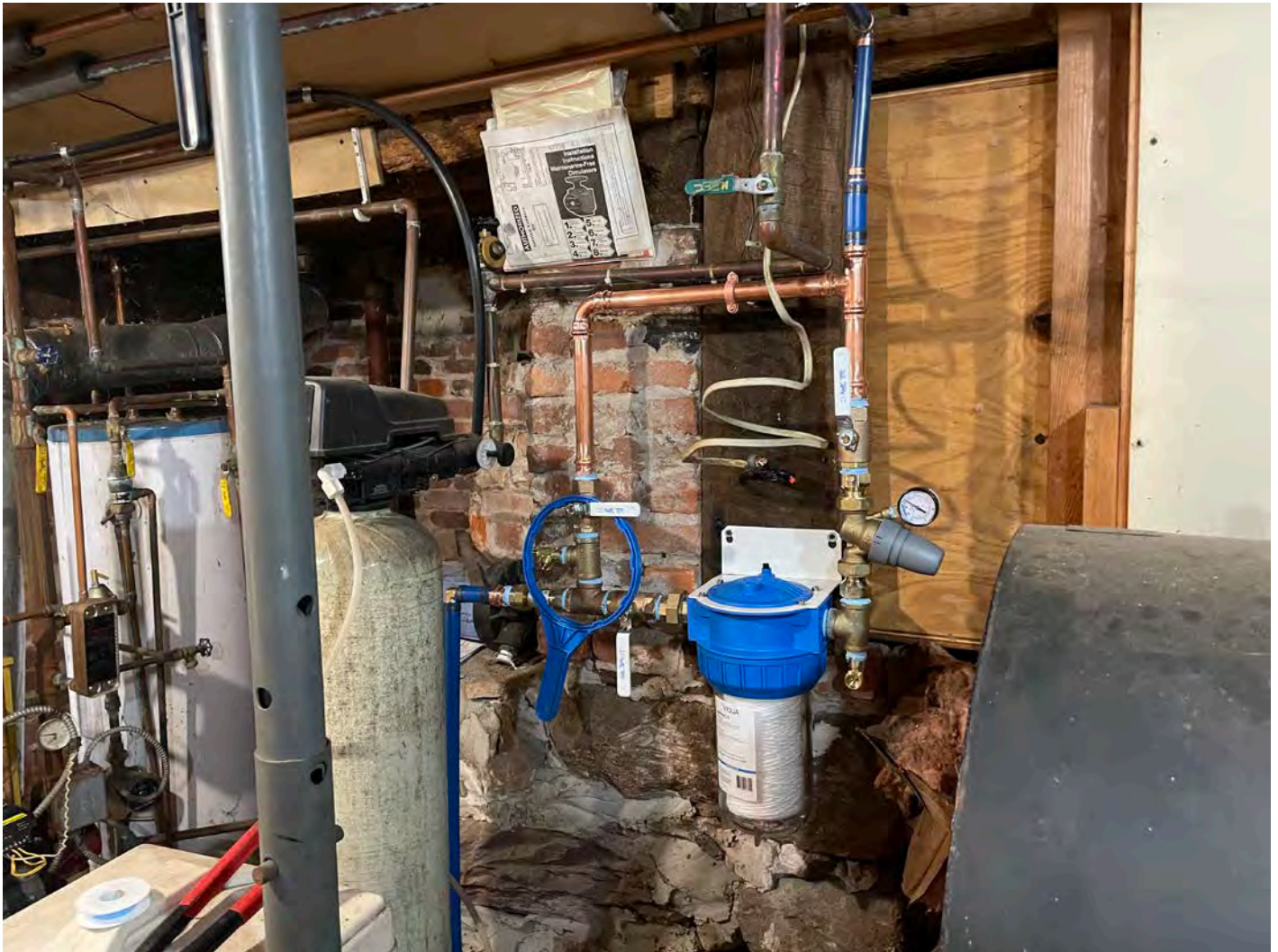
Picture 11: Final water service components that Fazzino Plumbing installed today at the residence located at 22 Wallingford Road, Durham.
