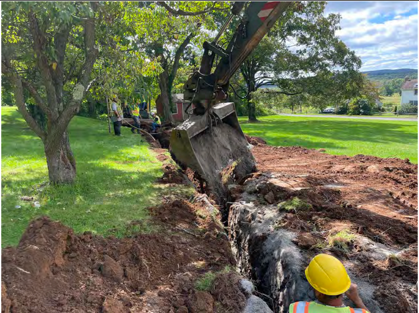
Picture 9: Ludlow placing sand over 1.5" copper water service line at the 22 Wallingford Road property. View to the southwest.
