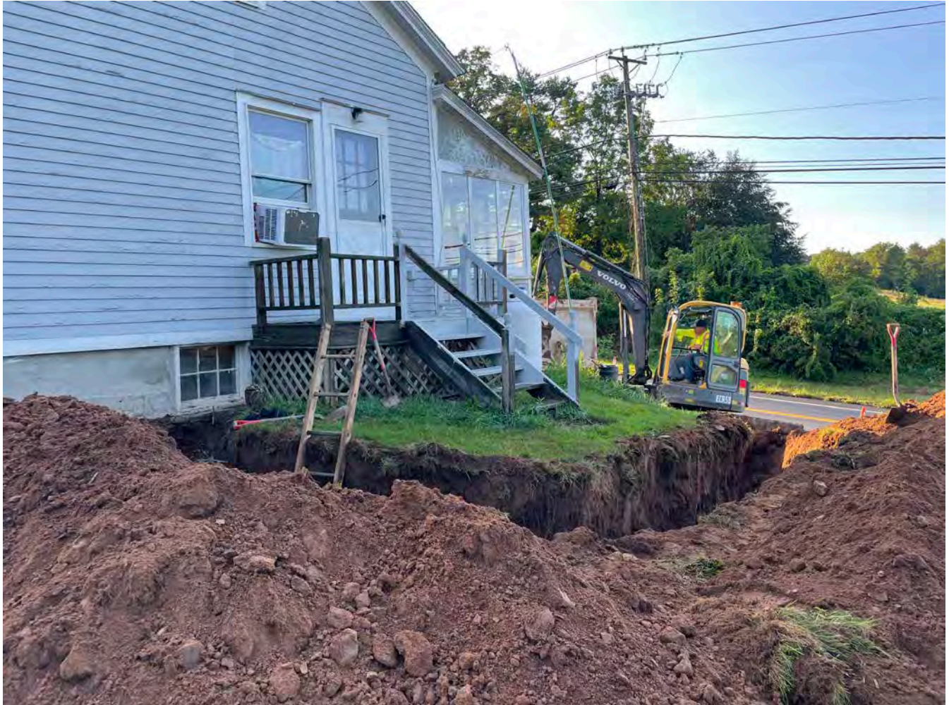
Picture 1: Ludlow excavating on the west side of the 47 Wallingford Road, Durham, residence for the installation of a 1" copper water service line. View to the south.
