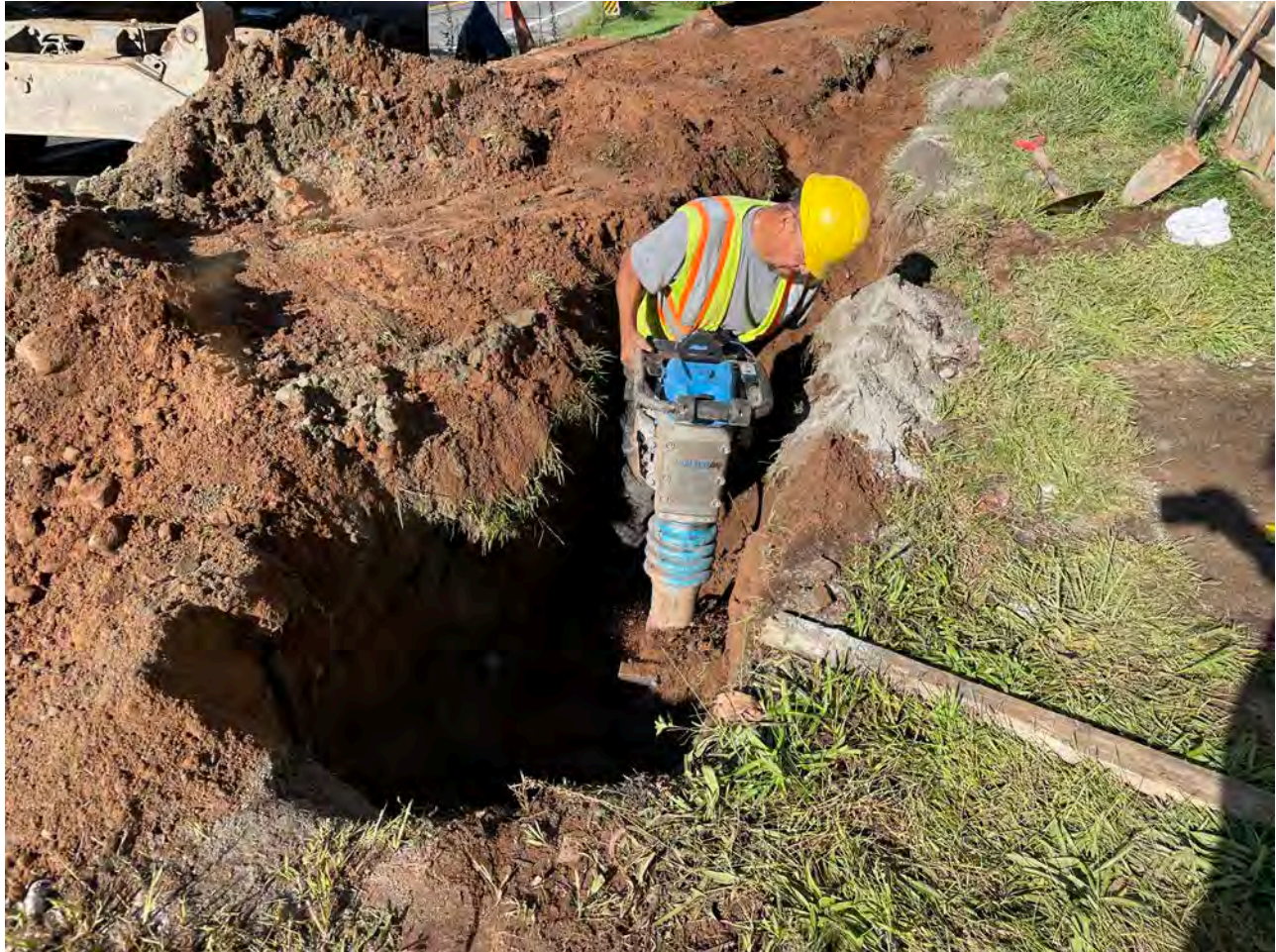
Picture 3: Ludlow compacting backfill with a jumping jack as part of the water service installation activities at the 47 Wallingford Road residence. View to the west.
