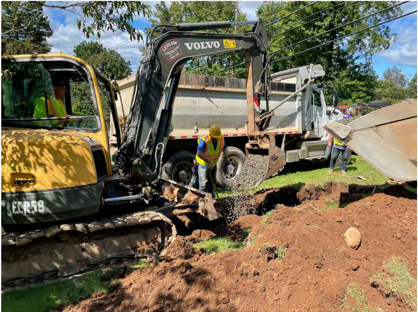
Picture 6: Ludlow placing a bed of gravel for the placement of a meter pit at the 22 Wallingford Road property. View to the west.
