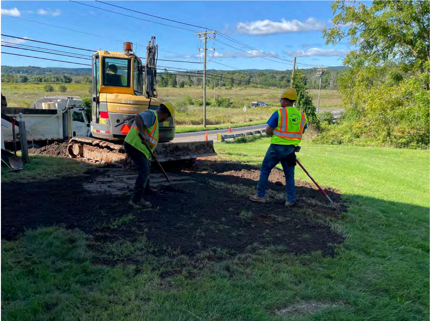
Picture 4: Ludlow raking out loam that they placed on areas of the lawn disturbed during the installation of a 1" copper water service line at 47 Wallingford Road. View to the west.
