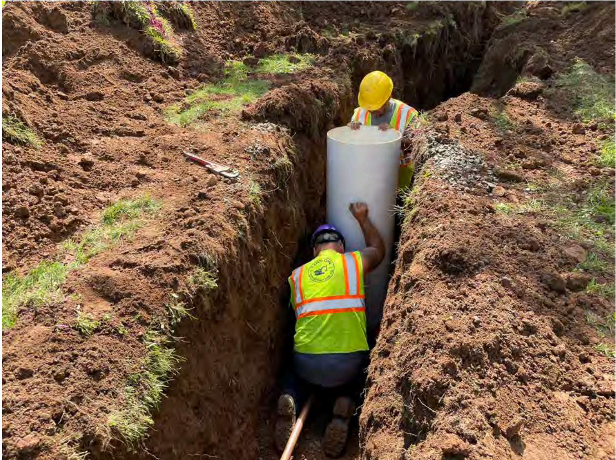
Picture 7: Ludlow installing a meter pit at the 22 Wallingford Road property as part of the installation of a 1.5” copper water service line. View to the south.
