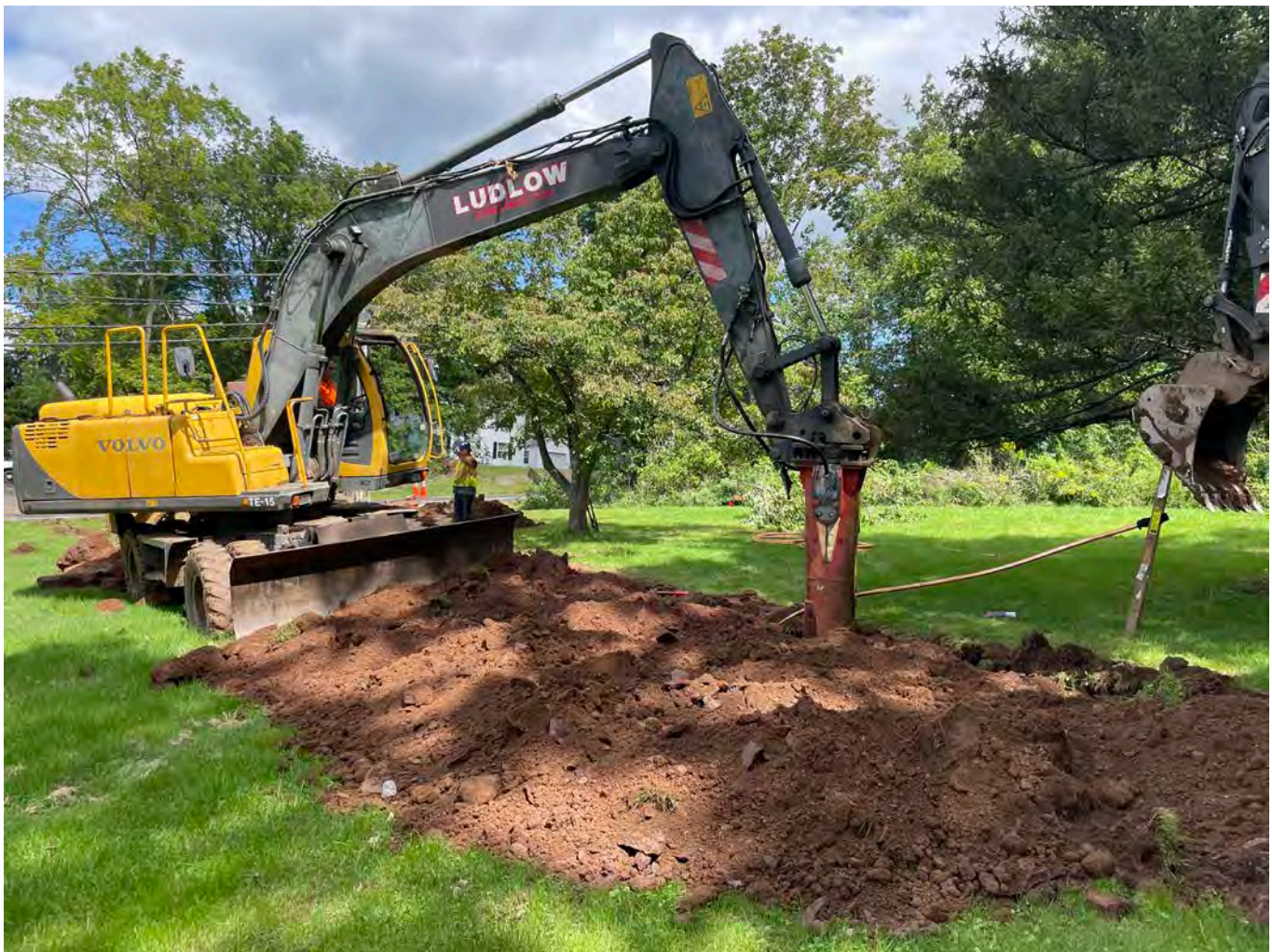
Picture 10: Ludlow hammering rock at the 22 Wallingford Road property for the installation of a 1.5” copper water service line. View to the northeast.
