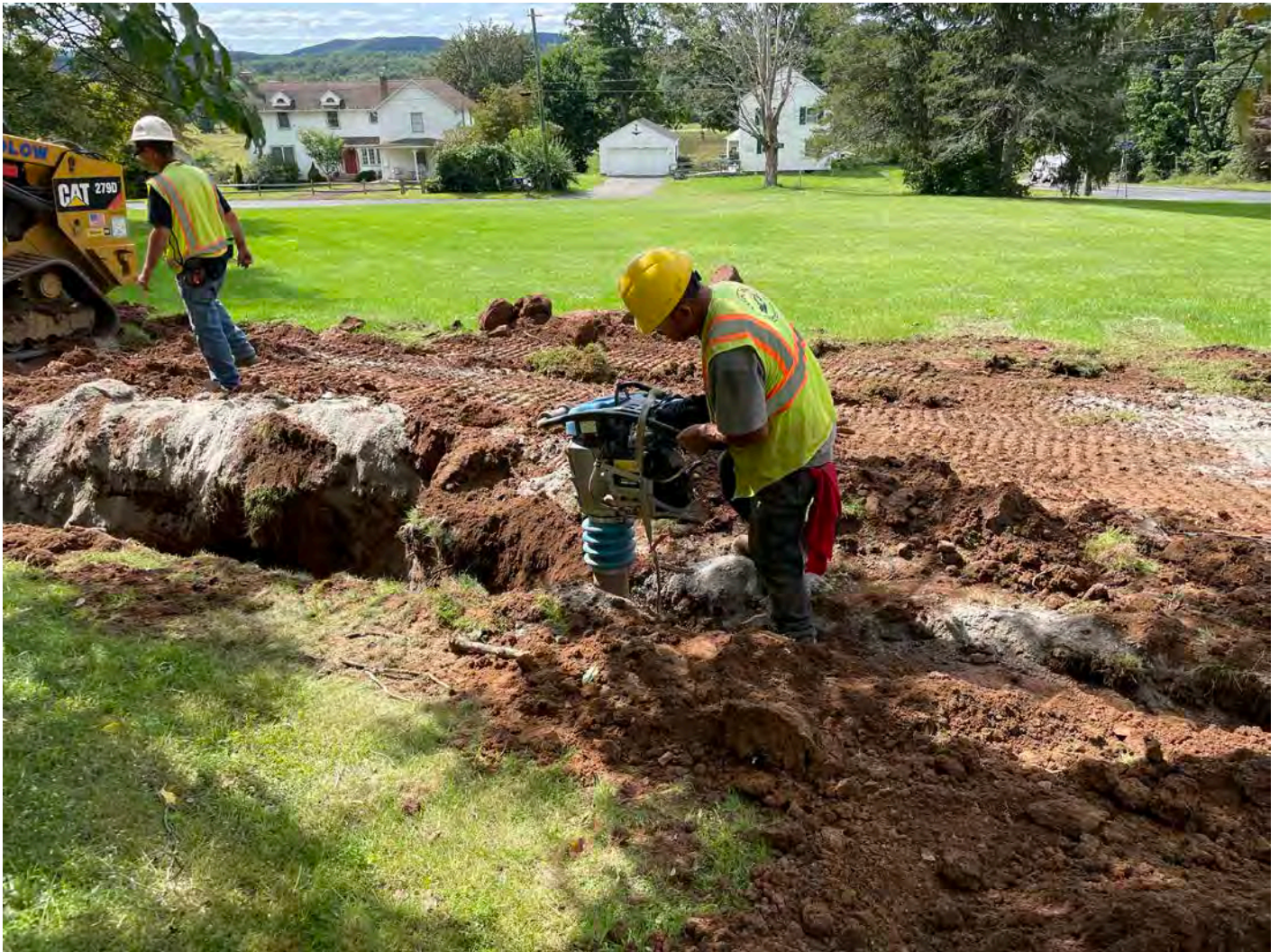
Picture 11: Ludlow compacting backfill with a jumping jack as part of the water service installation activities at the 22 Wallingford Road residence. View to the southwest.
