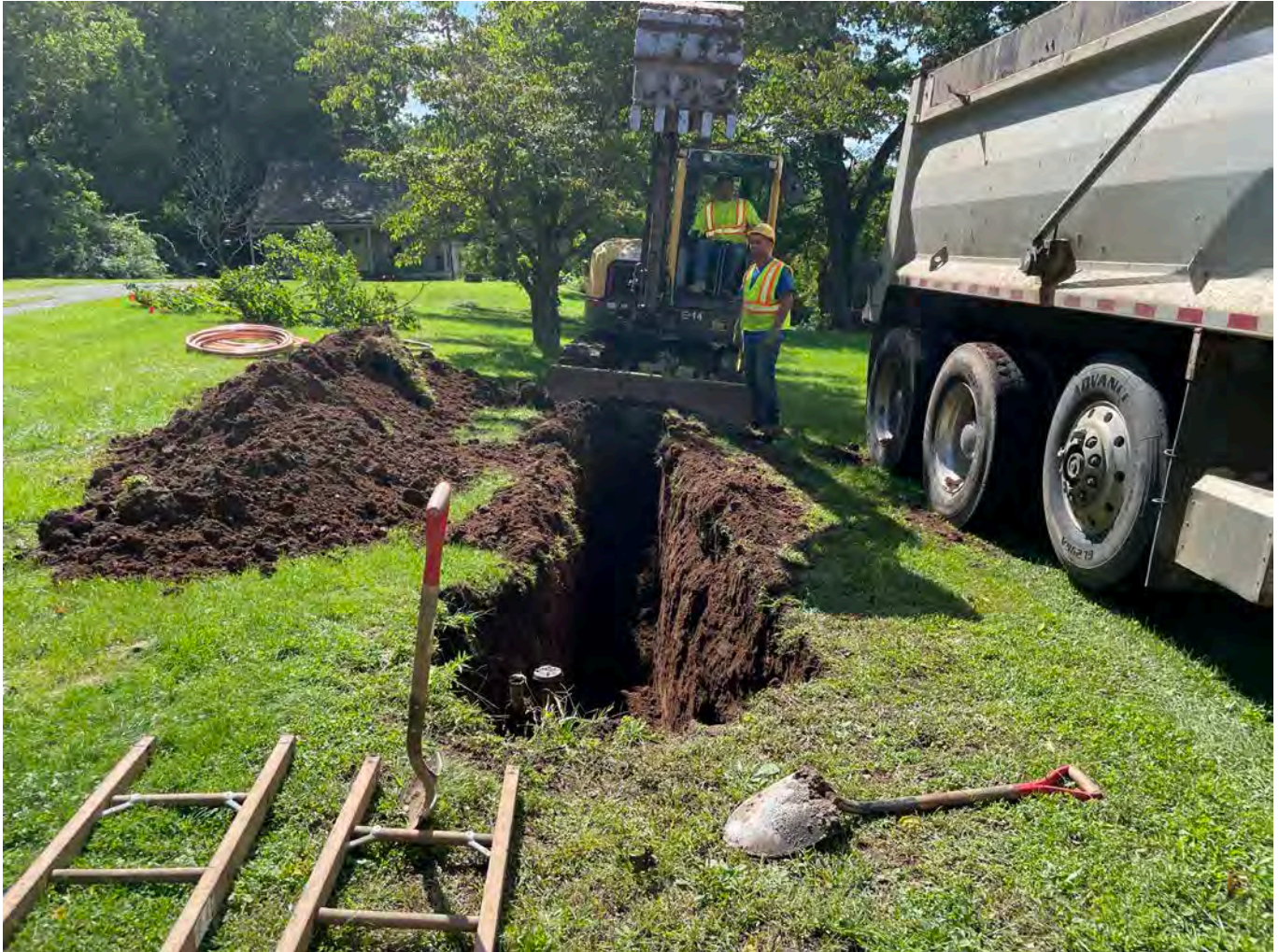
Picture 5: Ludlow excavating south of the curb stop for the installation of a 1.5" copper water service line at the 22 Wallingford Road property in Durham. View to the south.
