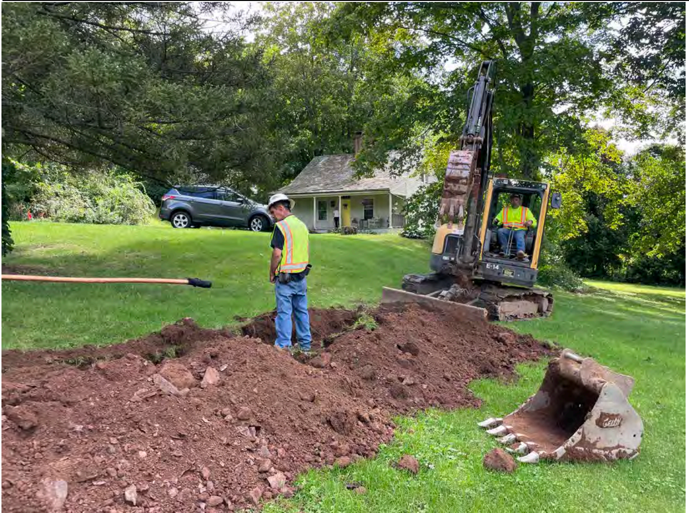
Picture 8: Ludlow excavating at the 22 Wallingford Road property in Durham for the installation of a 1.5" copper water service line. View to the south.
