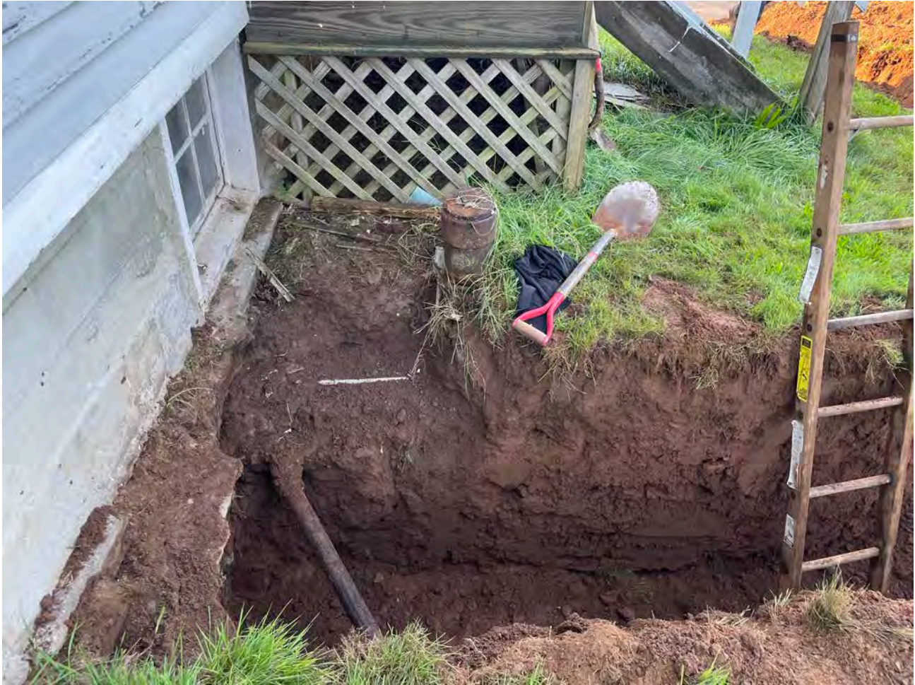
Picture 2: The western side of the foundation for 47 Wallingford Road after Ludlow daylighted it. View to the south.
