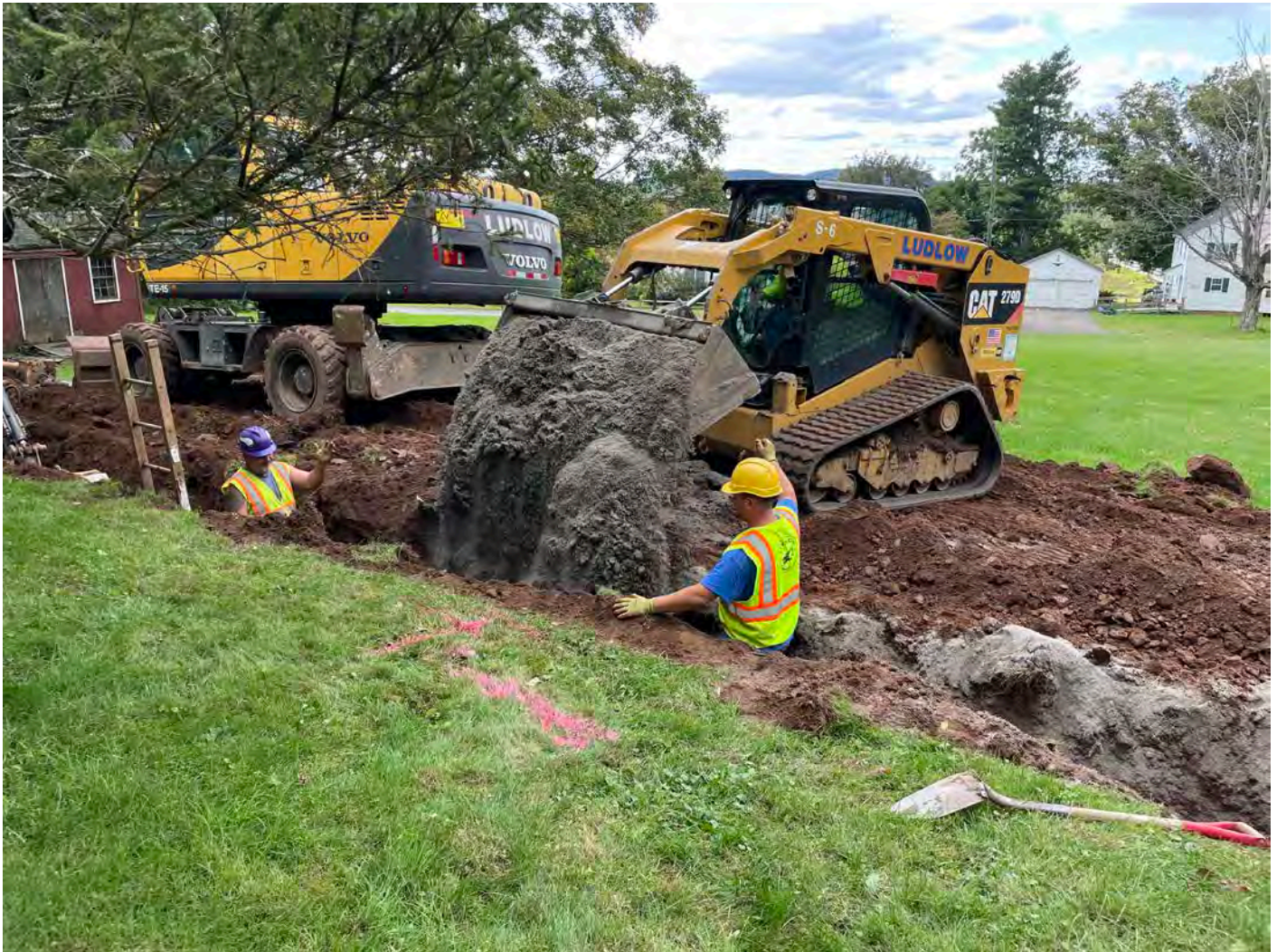
Picture 12: Ludlow placing sand over the 1.5" copper water service pipe they are installing at the 22 Wallingford Road property. View to the southwest.
