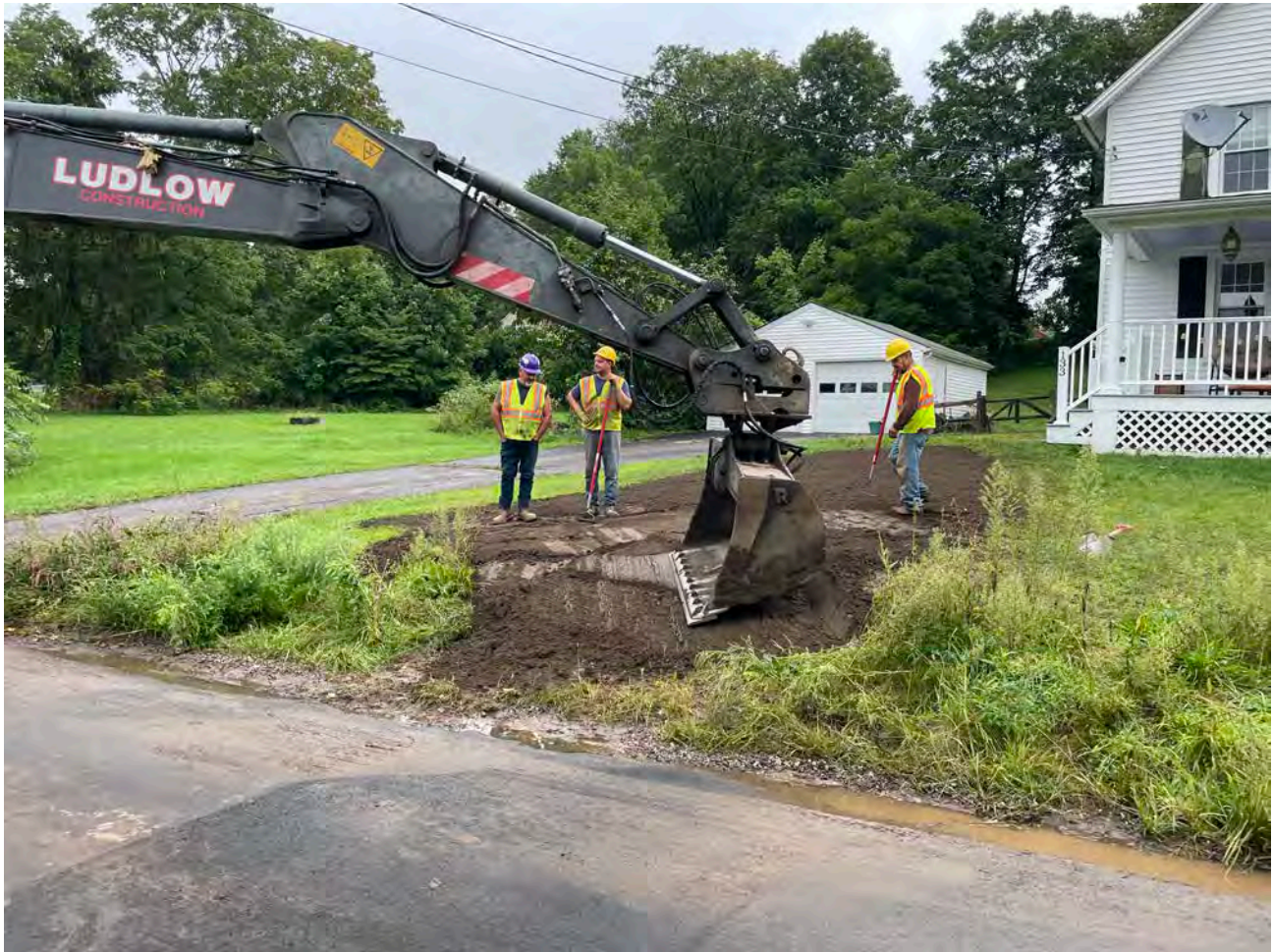
Picture 2: Ludlow finishing lawn restoration at the 133 Maple Avenue after the installation of a 1" copper water service line. View to the northeast.
