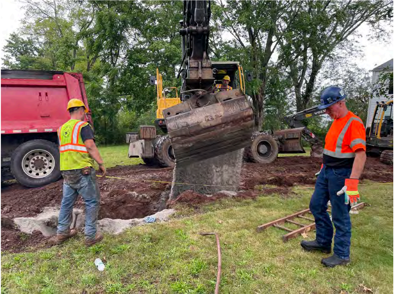
Picture 5: Ludlow placing sand over the 1" copper water service line they installed at the 17 Wallingford Road residence in Durham. View to the northwest.
