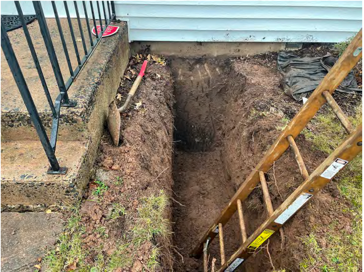
Picture 4: Concrete foundation of the 17 Wallingford Road residence that Ludlow has daylighted on the south side of the home for the installation of a 1” copper water service line. View to the north.
