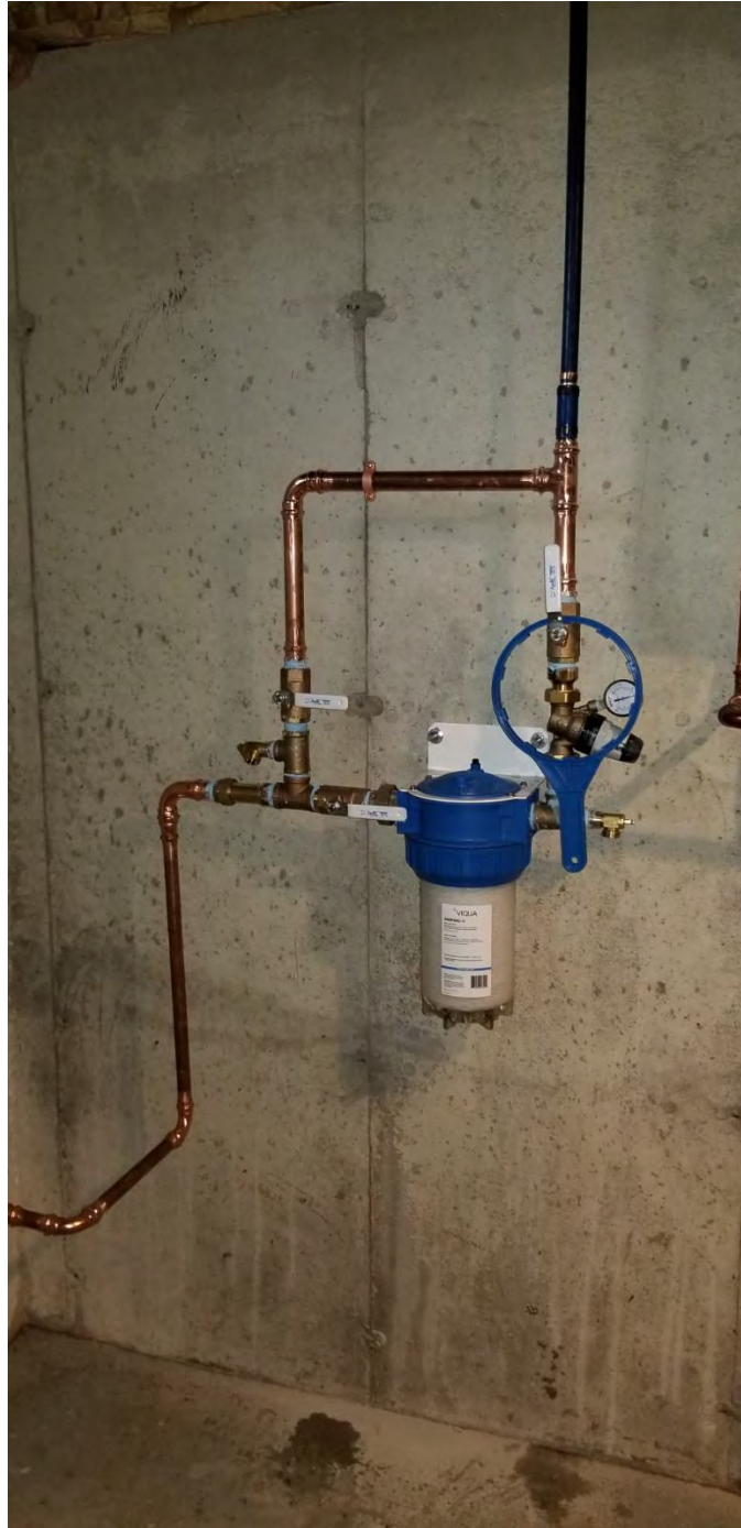
Picture 9: Final water service components that Fazzino installed at the 109 Maple Avenue residence.
