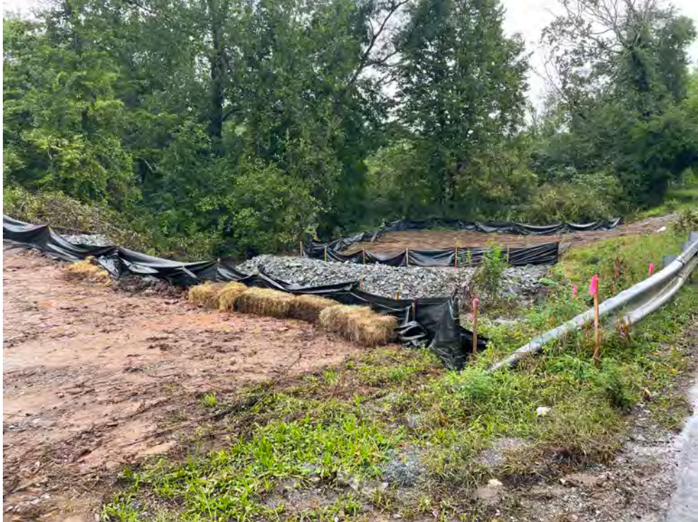
Picture 7: Ludlow placed new silt fence on both sides of Ball Brook at the Maiden Lane stream crossing work zone. View to the northeast.
