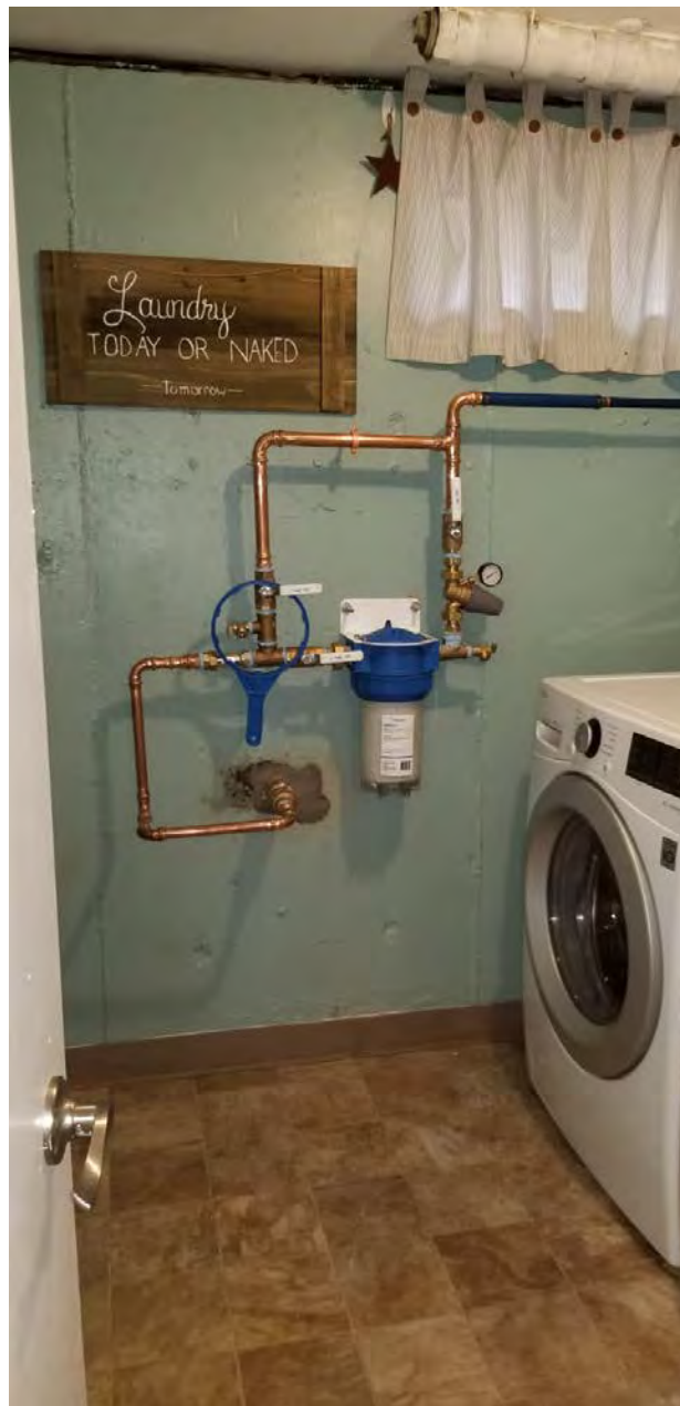
Picture 11: Final water service components that Fazzino installed at the 129 Maple Avenue residence.
