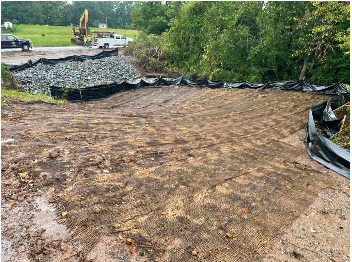
Picture 8: Ludlow placed new silt fence on both sides of Ball Brook at the Maiden Lane stream crossing work zone. View to the northwest.
