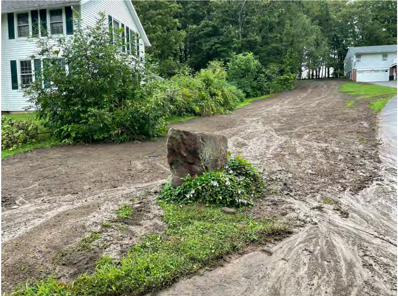
Picture 1: Portion of the lawn at 129 Maple Avenue that saw minor erosion from the previous night's rain event. Ludlow cleaned the road and driveway apron with a Broce Broom. View to the east.
