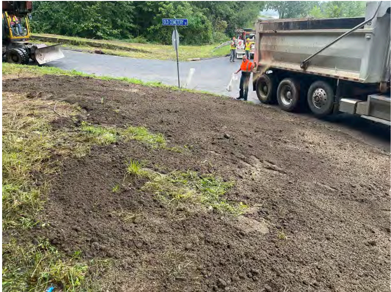
Picture 3: Ludlow placing grass seed on top of loam they just placed on the northeast corner of the intersection of Old Cemetery Road and Maple Avenue, Durham. View to the southeast.
