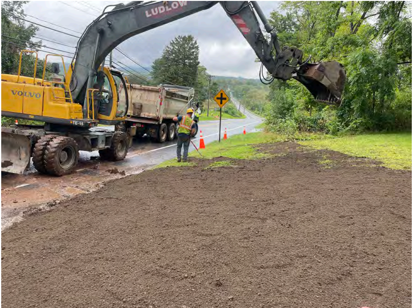
Picture 6: Ludlow raking out loam as part of restoration activities on the sections of the lawn at the 17 Wallingford Road residence that were disturbed during the installation of a 1" copper water service line. View to the west.
