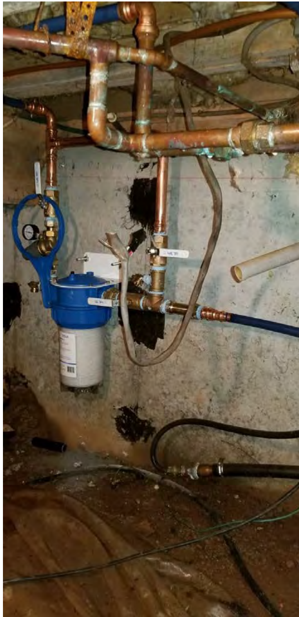
Picture 10: Final water service components that Fazzino installed at the 119 Maple Avenue residence.
