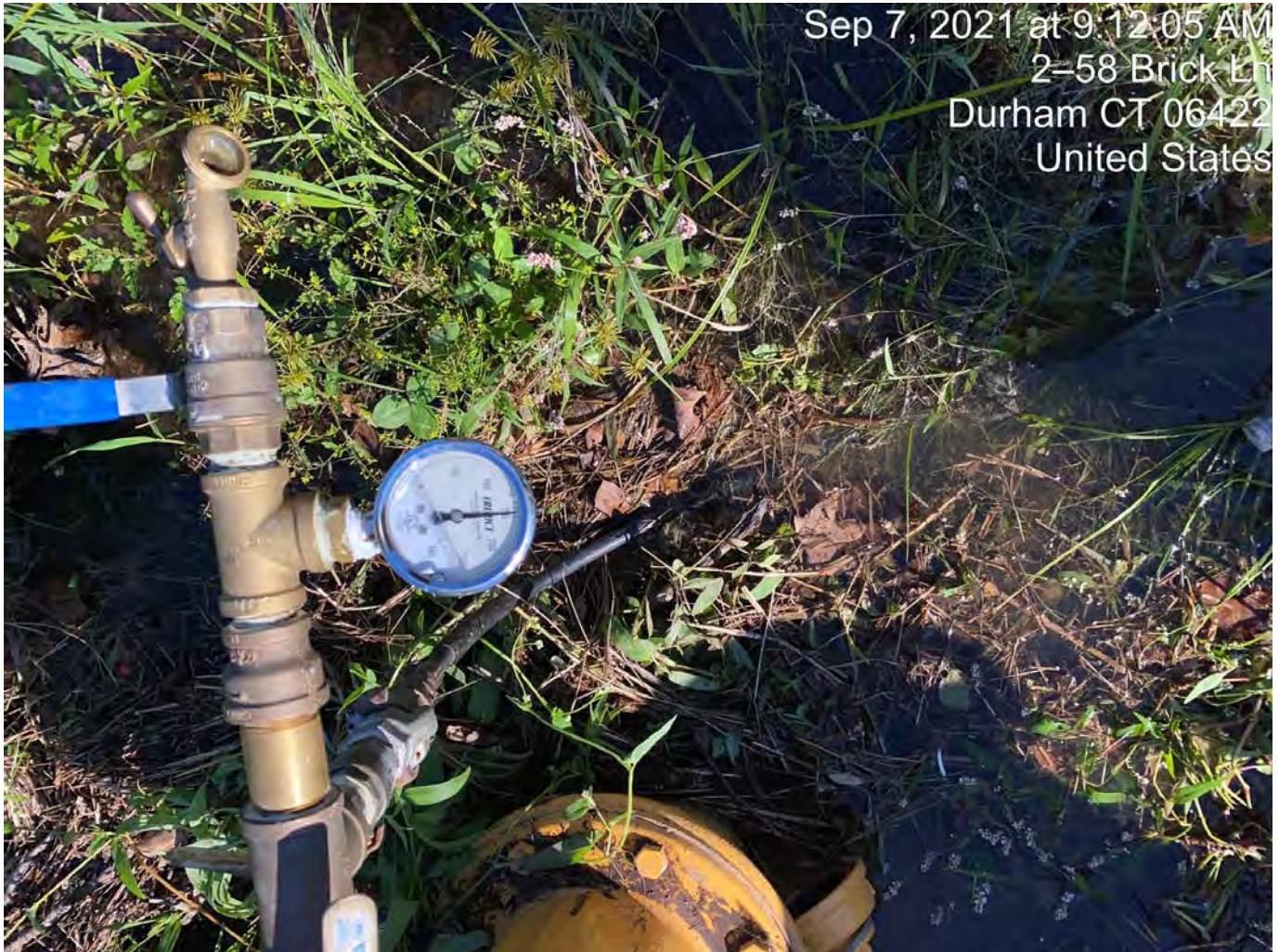
Picture 6: Starting pressure for the pressure test that Ludlow conducted on September 7, 2012, on the 12" DIP they installed as part of the Maiden Lane stream crossing.
