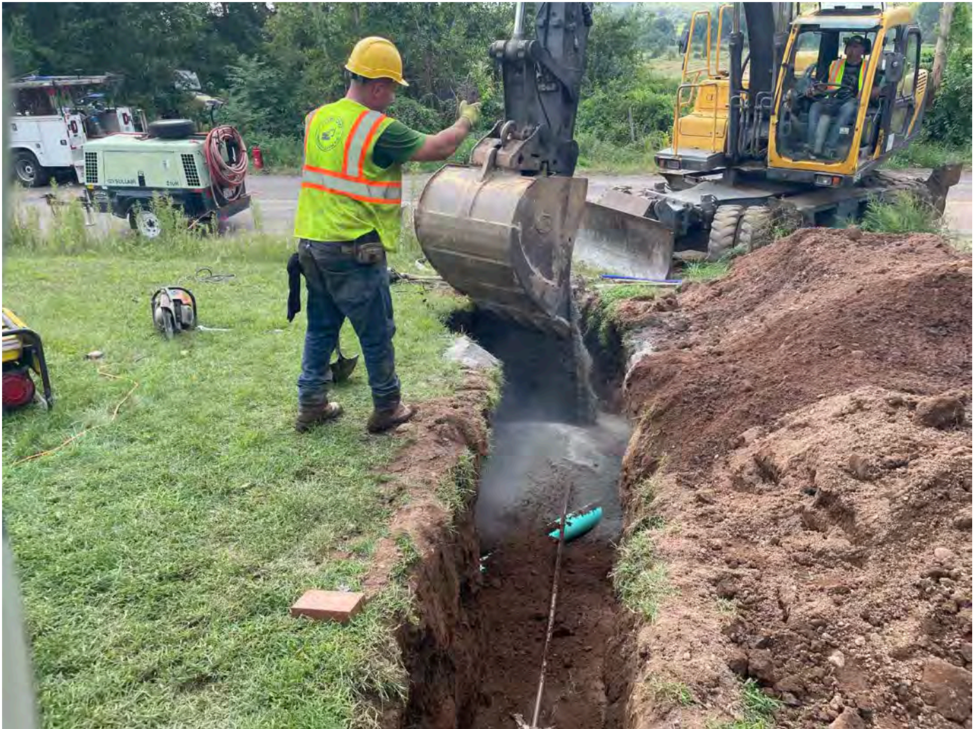
Picture 13: Ludlow placing sand over the 1" copper water service line they installed at the 133 Maple Avenue property. View to the west.
