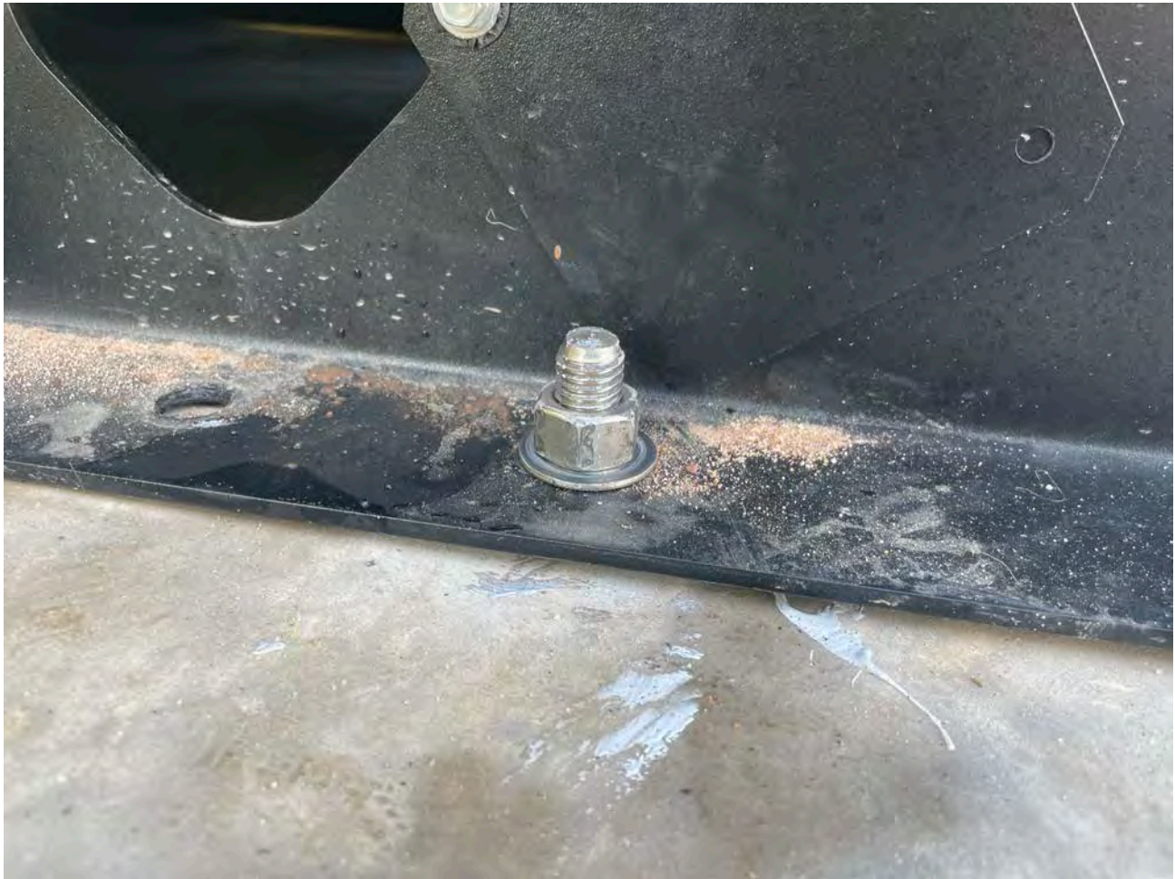
Picture 2: Closeup of one of the bolts used to anchor the booster station generator to its concrete pad. View to the southwest.
