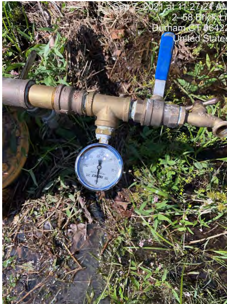
Picture 7: End pressure for the pressure test that Ludlow conducted on September 7, 2012, on the 12" DIP they installed as part of the Maiden Lane stream crossing.
