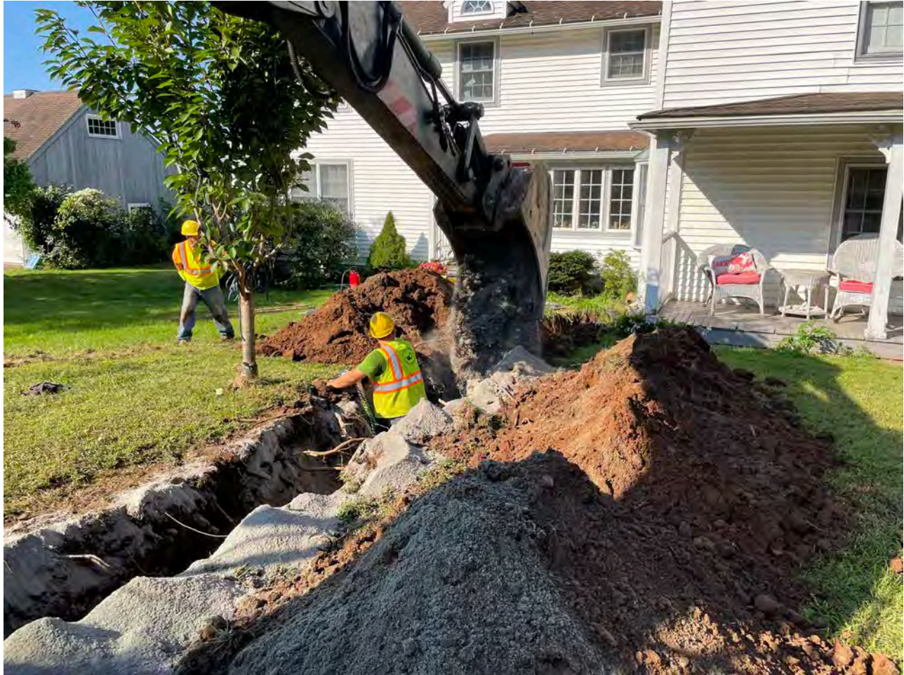
Picture 3: Ludlow placing sand followed by caution tape over the 1” copper water service line they have placed in the trench they excavated at the 146 Maple Avenue residence.
