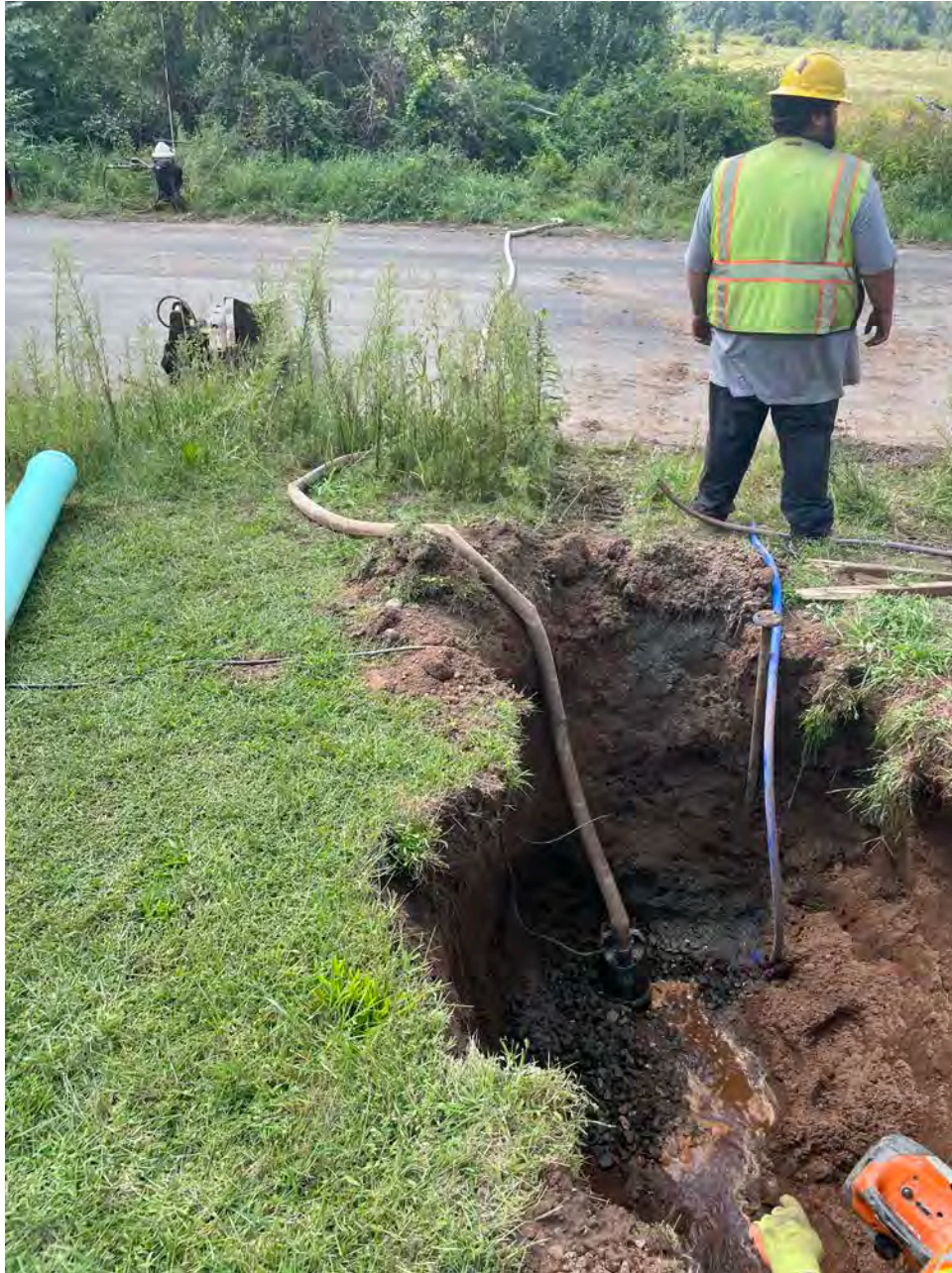
Picture 10: Ludlow pumping water from the excavation at the 133 Maple Avenue property as they install a 1" copper water service line. Water is being pumped into the empty lot located across the street to the west of the 133 Maple Avenue property. View to the west.
