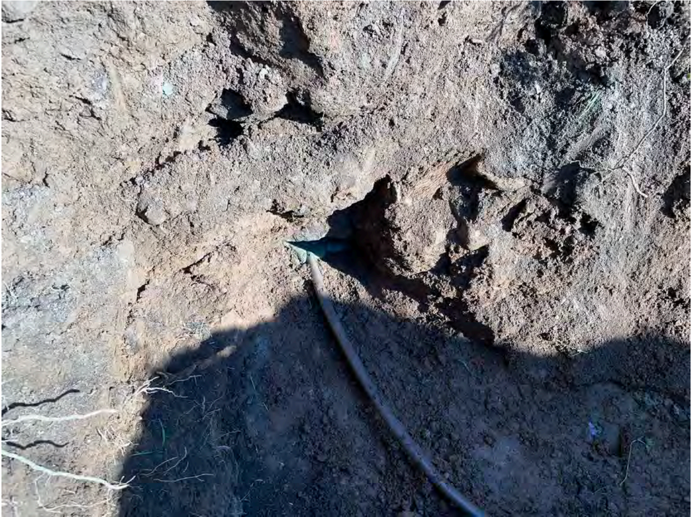
Picture 4: 1" copper water service line penetrating into the south side of the foundation for 146 Maple Avenue, on the most eastern portion of the house that juts out to the east towards Maple Avenue.
