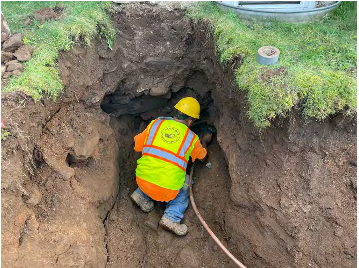
Picture 12: Ludlow securing 1" copper water service line with non-shrink grout on the north side of the 133 Maple Avenue residence. View to the south.
