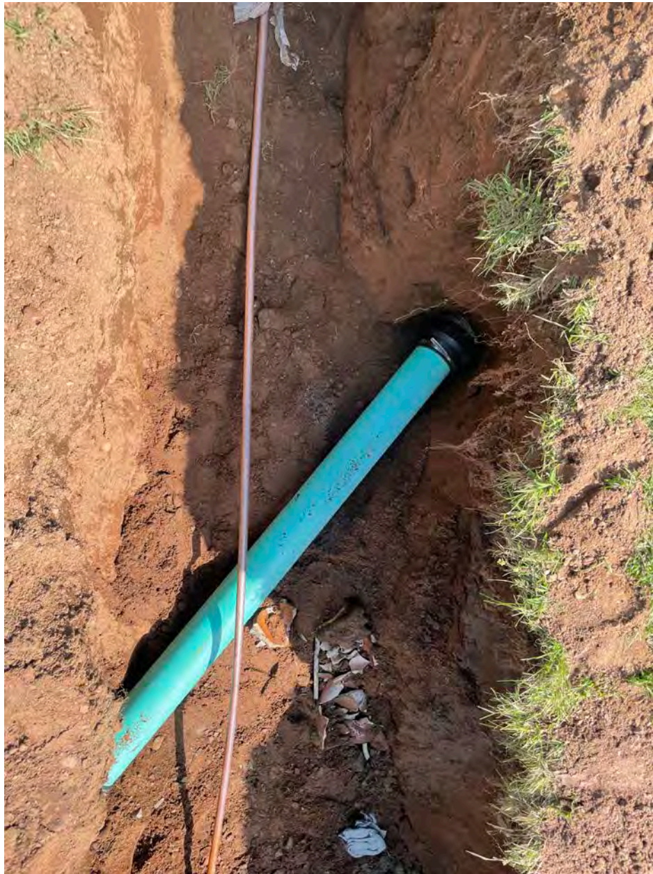
Picture 11: Repair that Ludlow made to a 6" clay drainage line at the 133 Maple Avenue property.
