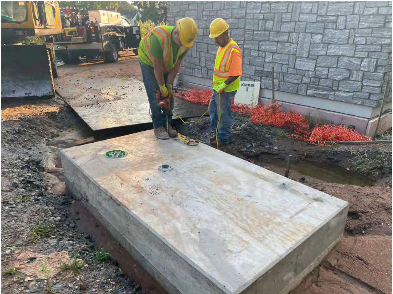
Picture 1: Ludlow drilling into the concrete pad for the generator located on the west side of the booster station at Station 750+63. View to the northeast.
