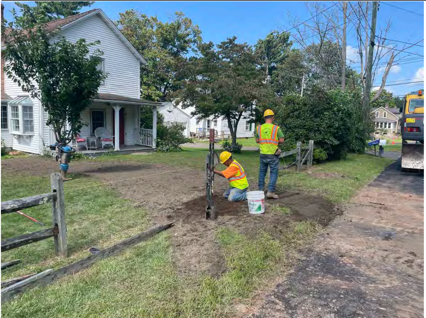
Picture 8: Ludlow working on reassembling a portion of the fence they temporarily took down at the 146 Maple Avenue residence after installing a 1" copper water service line. View to the northwest.
