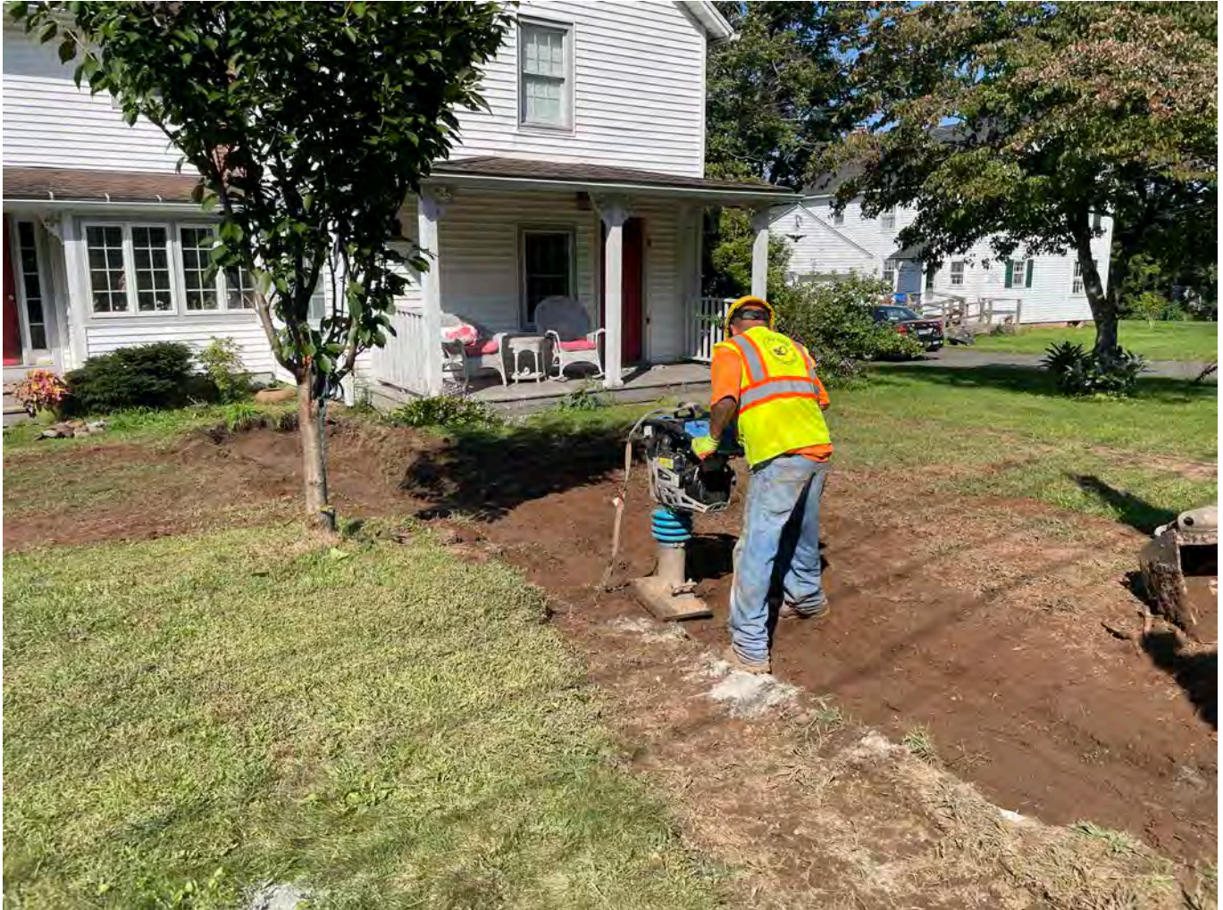
Picture 5: Ludlow compacting fill that was backfilled over the 1" copper water service line they installed at the 146 Maple Avenue residence. View to the northwest.
