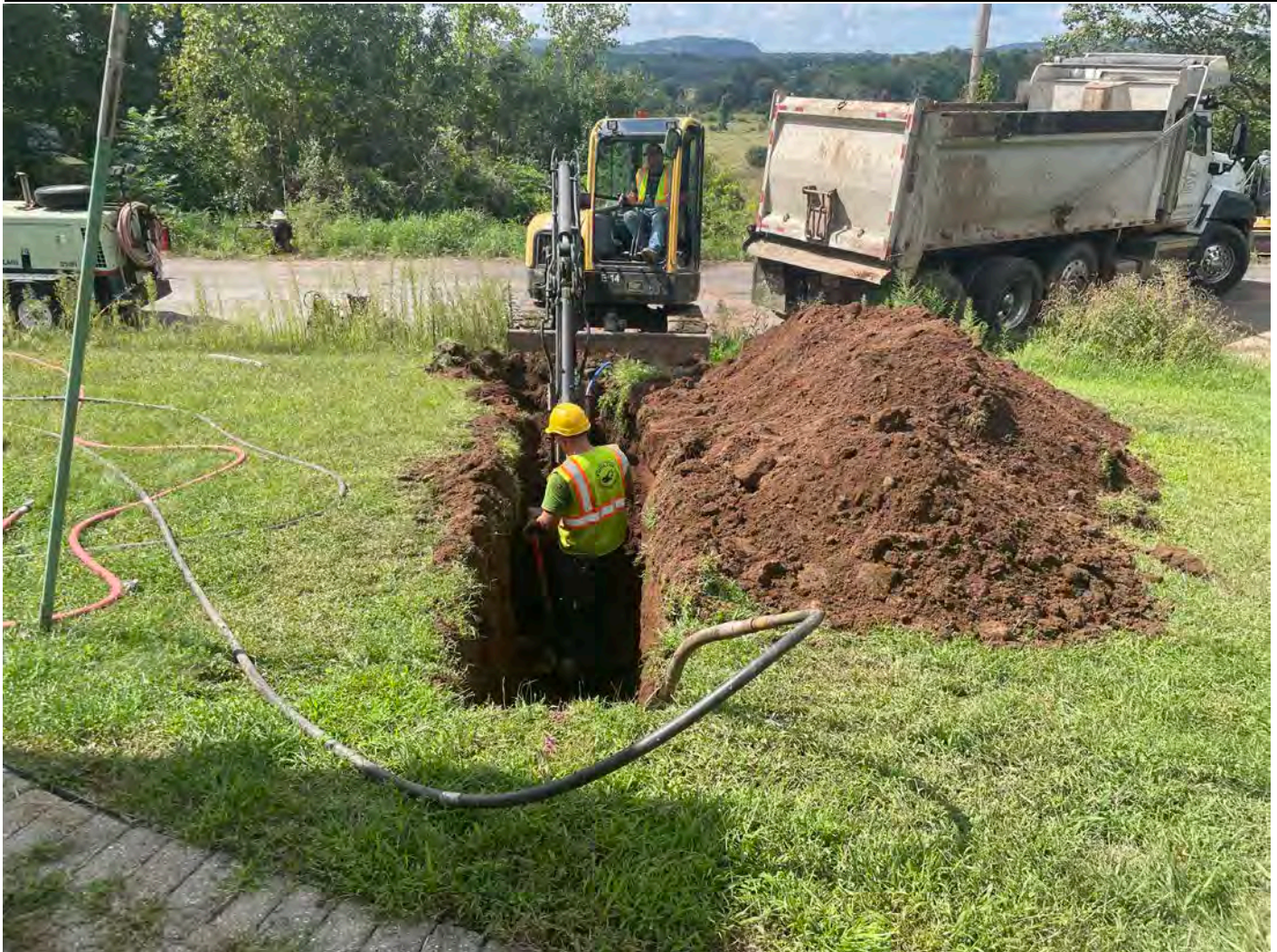
Picture 9: Ludlow excavating at the 133 Maple Avenue property to install a 1" copper water service line. View to the west.
