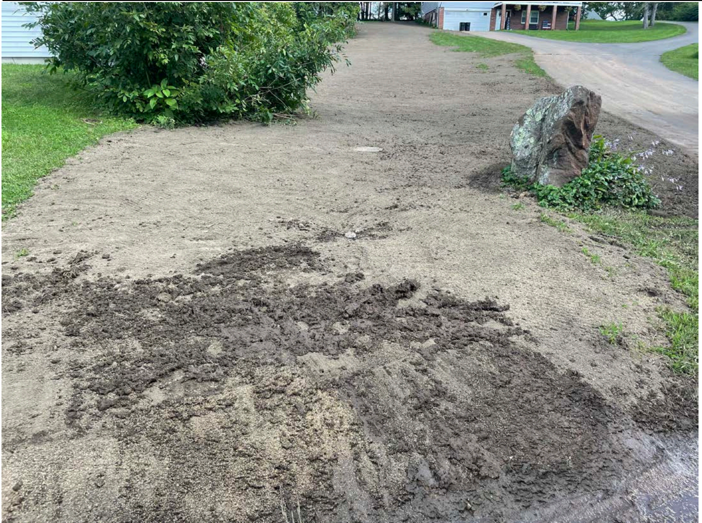
Picture 8: The 129 Maple Avenue, Durham, property after Ludlow restored those sections of the lawn that were disturbed during the installation of a 1.5" copper water service line. View to the east.
