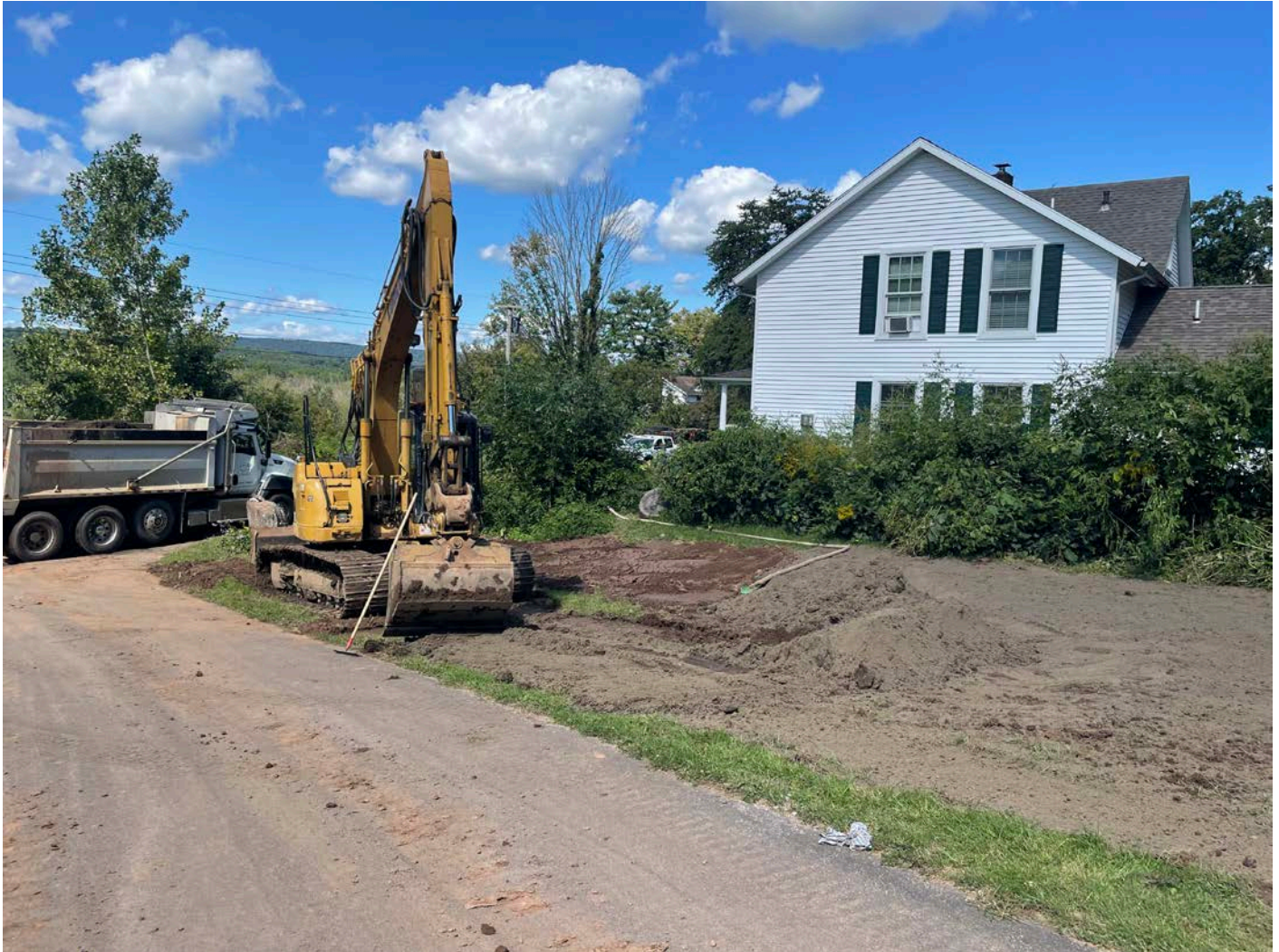
Picture 4: Ludlow restoring those areas on the 129 Maple Avenue, Durham, property that were disturbed during the installation of a 1.5" copper water service line. View to the northwest.
