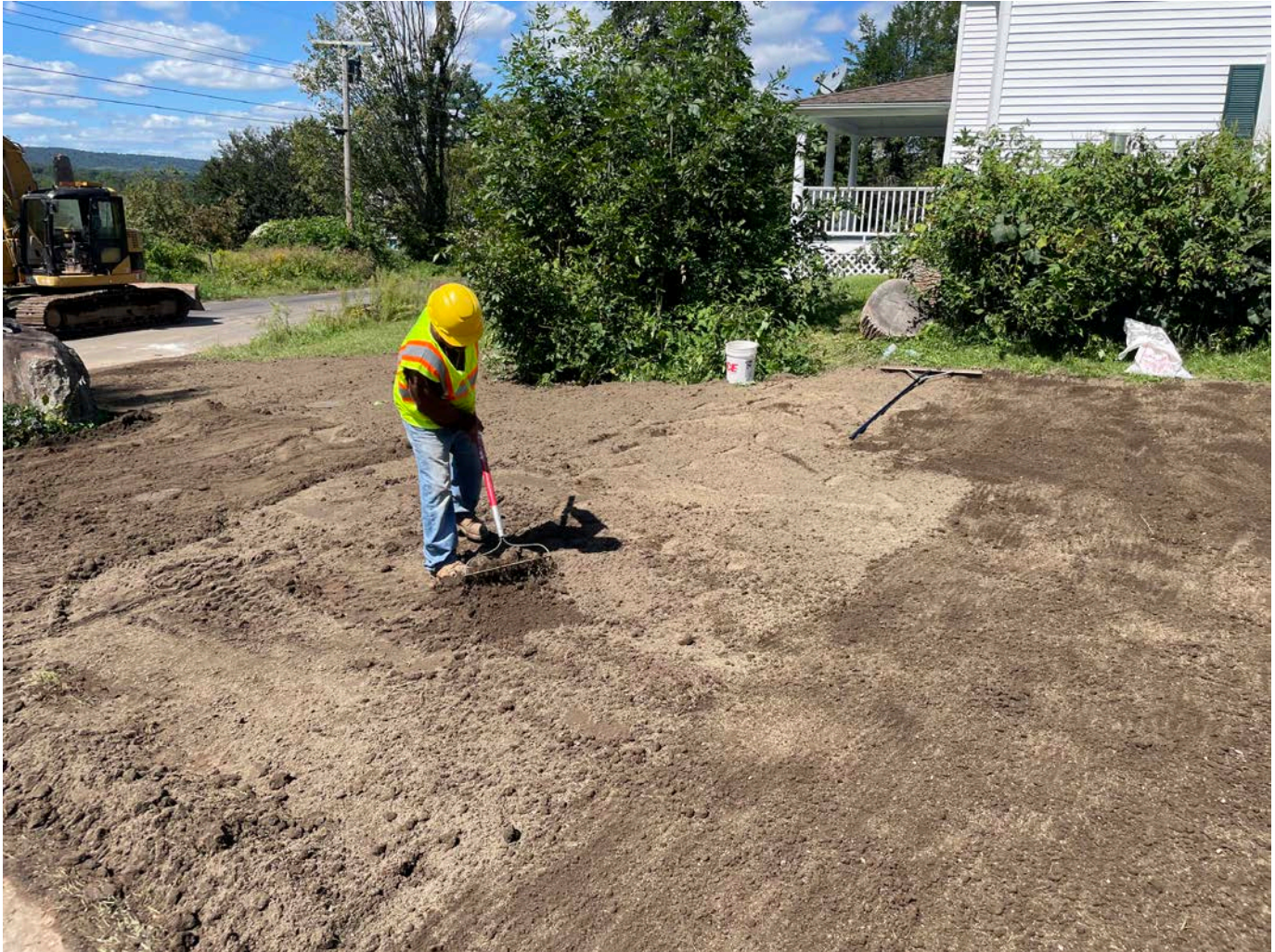
Picture 6: Ludlow raking loam on one of the areas on the 129 Maple Avenue, Durham, property that were disturbed during the installation of a 1.5" copper water service line. View to the northwest.
