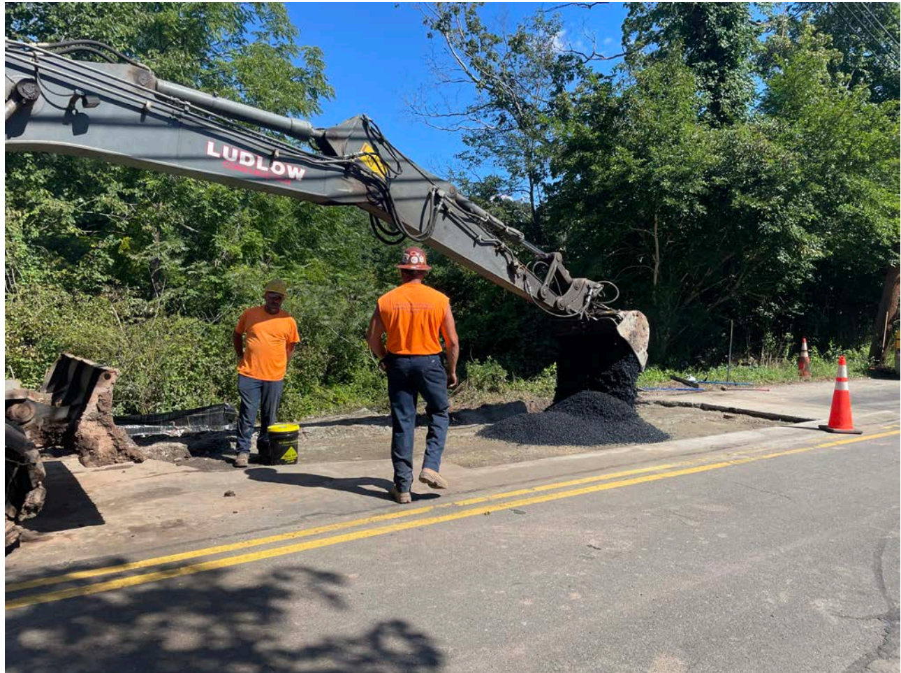
Picture 3: Ludlow placing asphalt over the backfilled excavation at Station 412+20 on Maiden Lane, Durham. View to the northeast.
