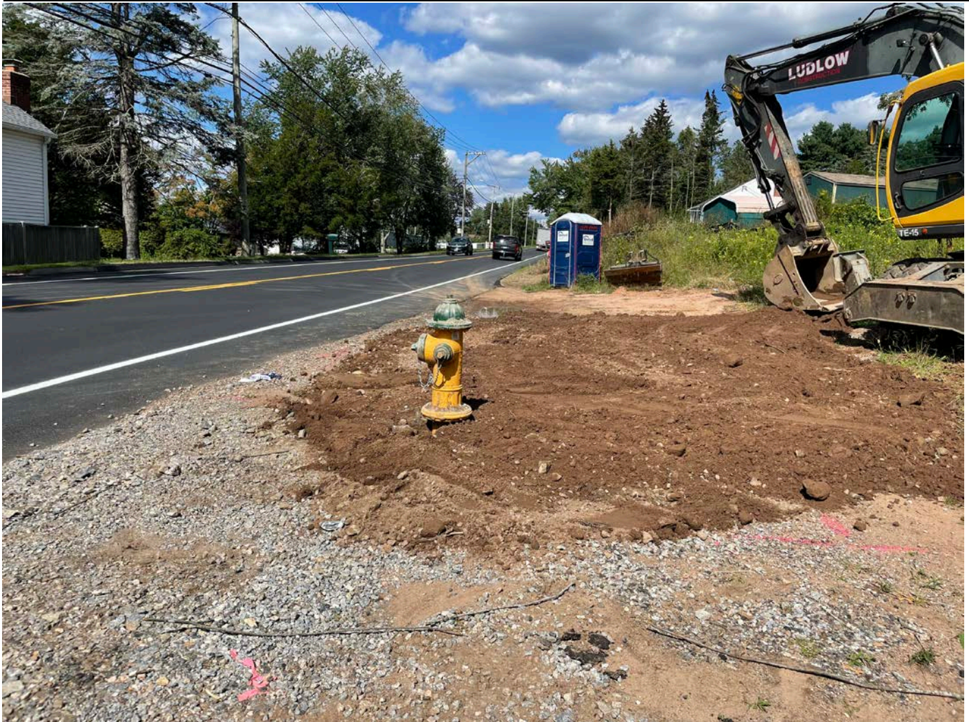
Picture 10: Hydrant that Ludlow reinstalled at Station 124+65 next to the water meter building located at Station ~124+80. View to the north.
