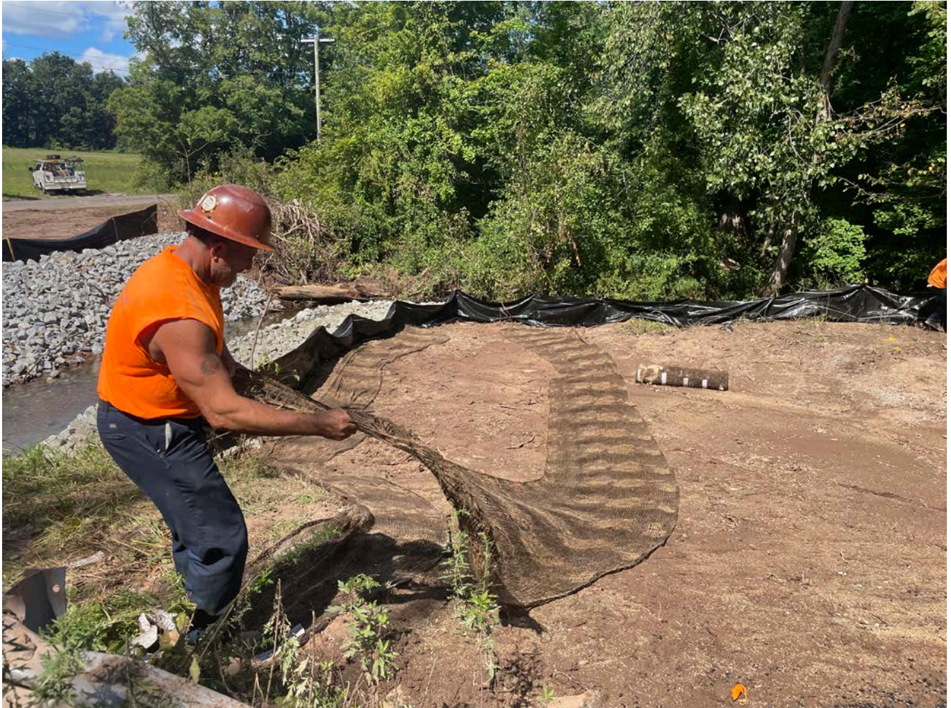
Picture 5: Ludlow placing erosion control netting over the soils located on the east side of Ball Brook at the Maiden Lane stream crossing. View to the north.
