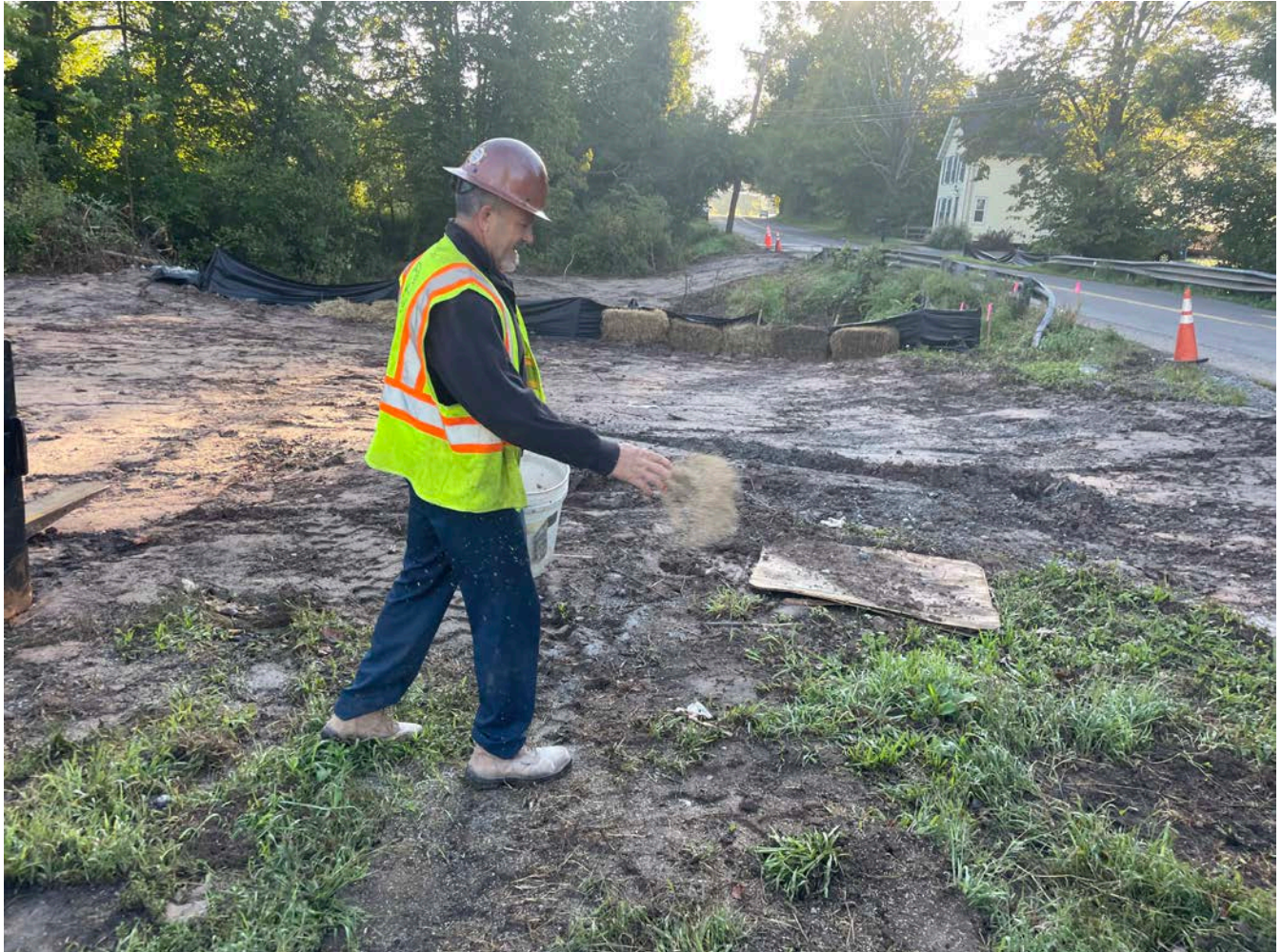
Picture 1: Ludlow spreading grass seed on the west side of Ball Brook at the Maiden Lane stream crossing in Durham. View to the southeast.
