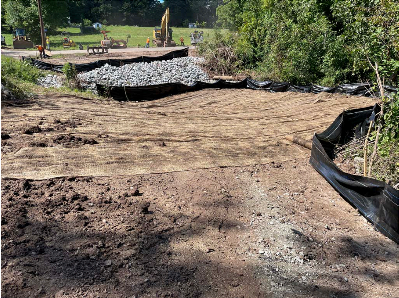
Picture 7: Erosion control mats that Ludlow placed on the east side of Ball Brook at the Maiden Lane stream crossing. View to the northwest.
