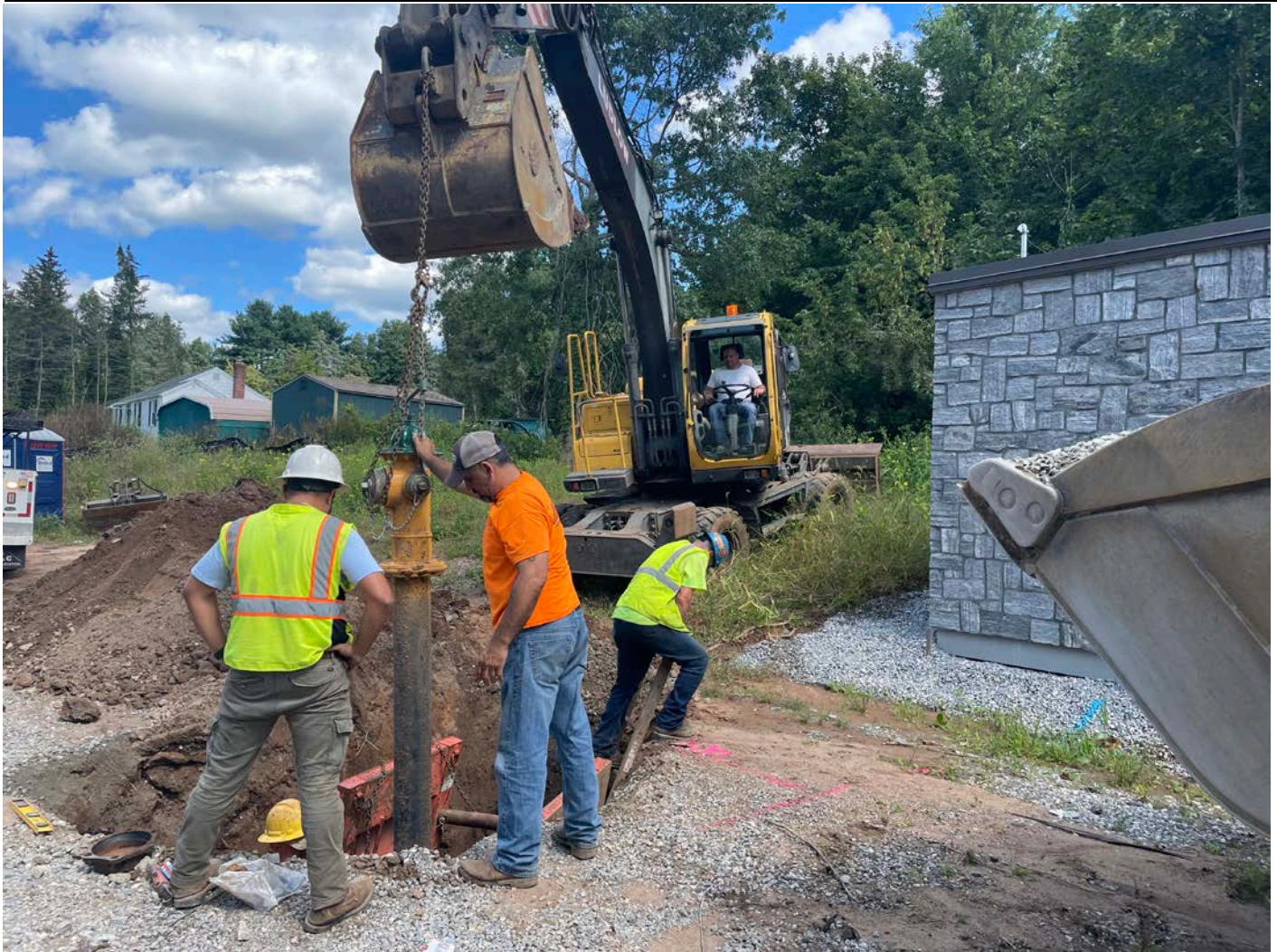
Picture 9: Ludlow maneuvering a hydrant into place for reinstallation at Station 124+65 on S. Main Street in Middletown. View to the northeast.
