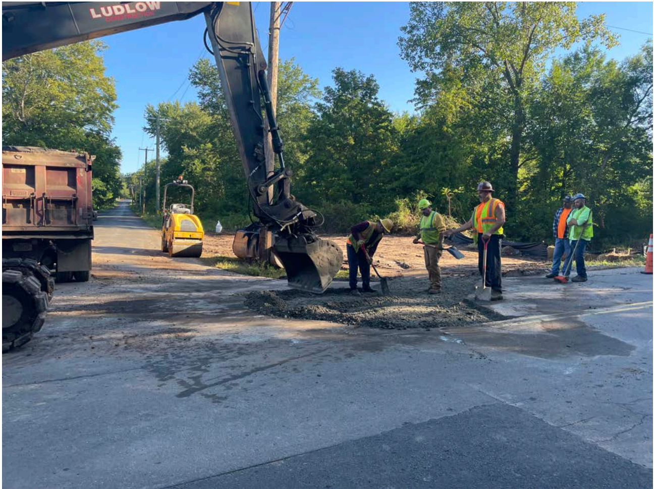
Picture 2: Ludlow placing processed stone over the backfilled excavation at Station 410+47 on Maiden Lane, Durham. View to the northeast.
