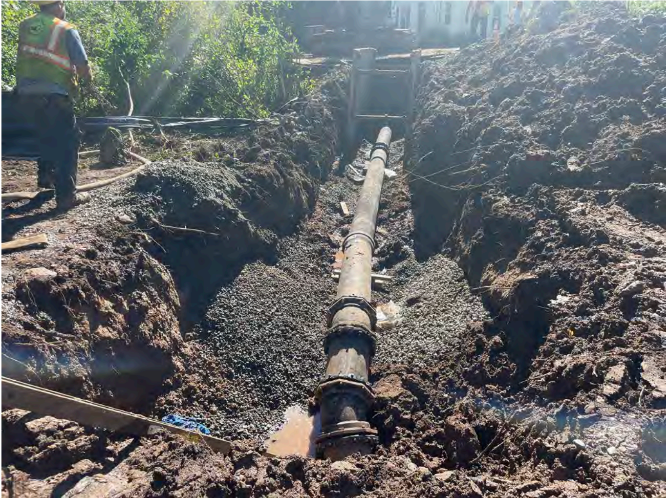
Picture 5: 12" DIP connecting the 12" DIP coming off Station 412+20 to the 12" DIP coming off the east side of the Maiden Lane stream crossing. View to the southeast.
