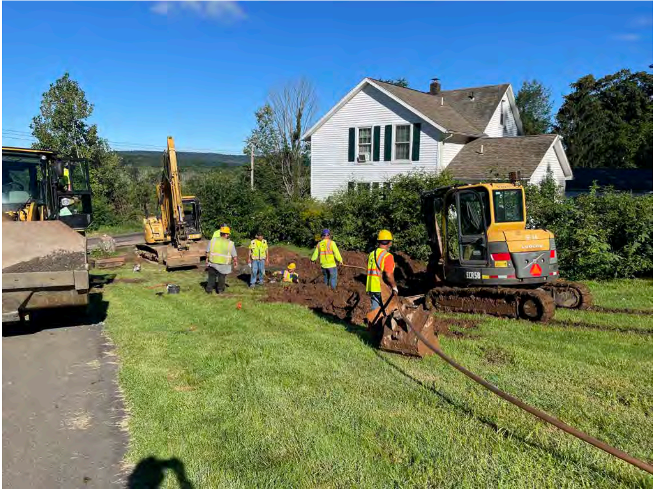
Picture 2: Ludlow installing 1.5" copper water service pipe at the 129 Maple Avenue property. View to the north.
