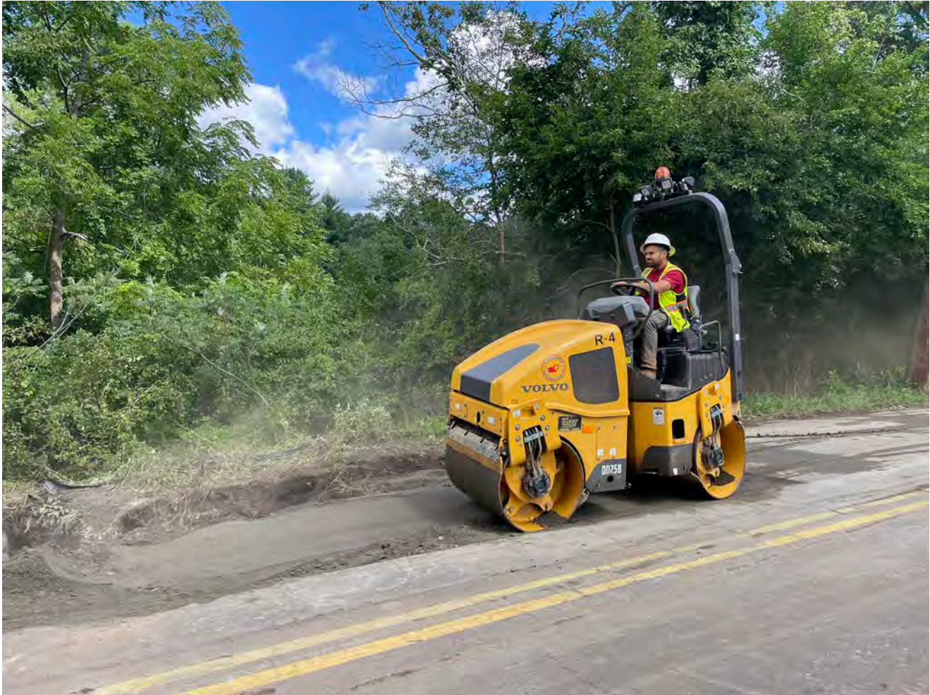
Picture 7: Ludlow using a rolling compactor on the backfilled excavation at Station 412+20. View to the northeast.
