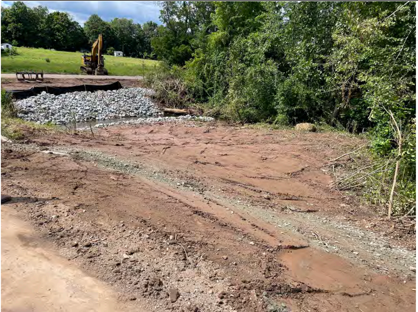
Picture 11: Maiden Lane stream crossing, looking to the northeast from Station 412+20.
