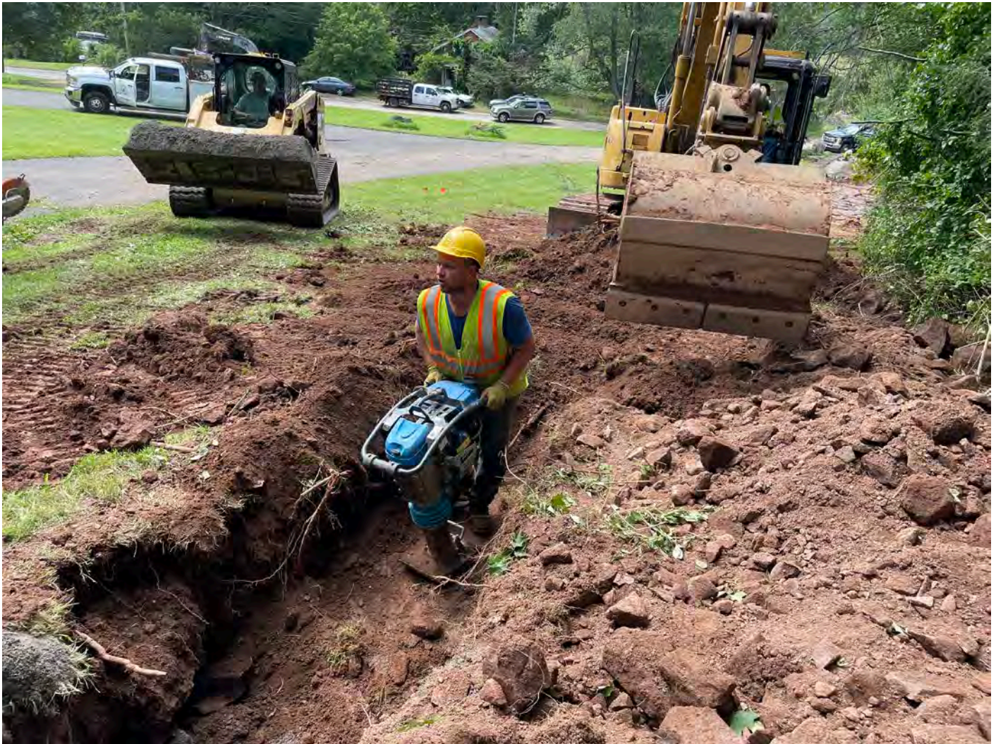
Picture 10: Ludlow compacting native fill that has been placed over the 1.5" copper water service line they installed at the 129 Maple Avenue property. View to the west.
