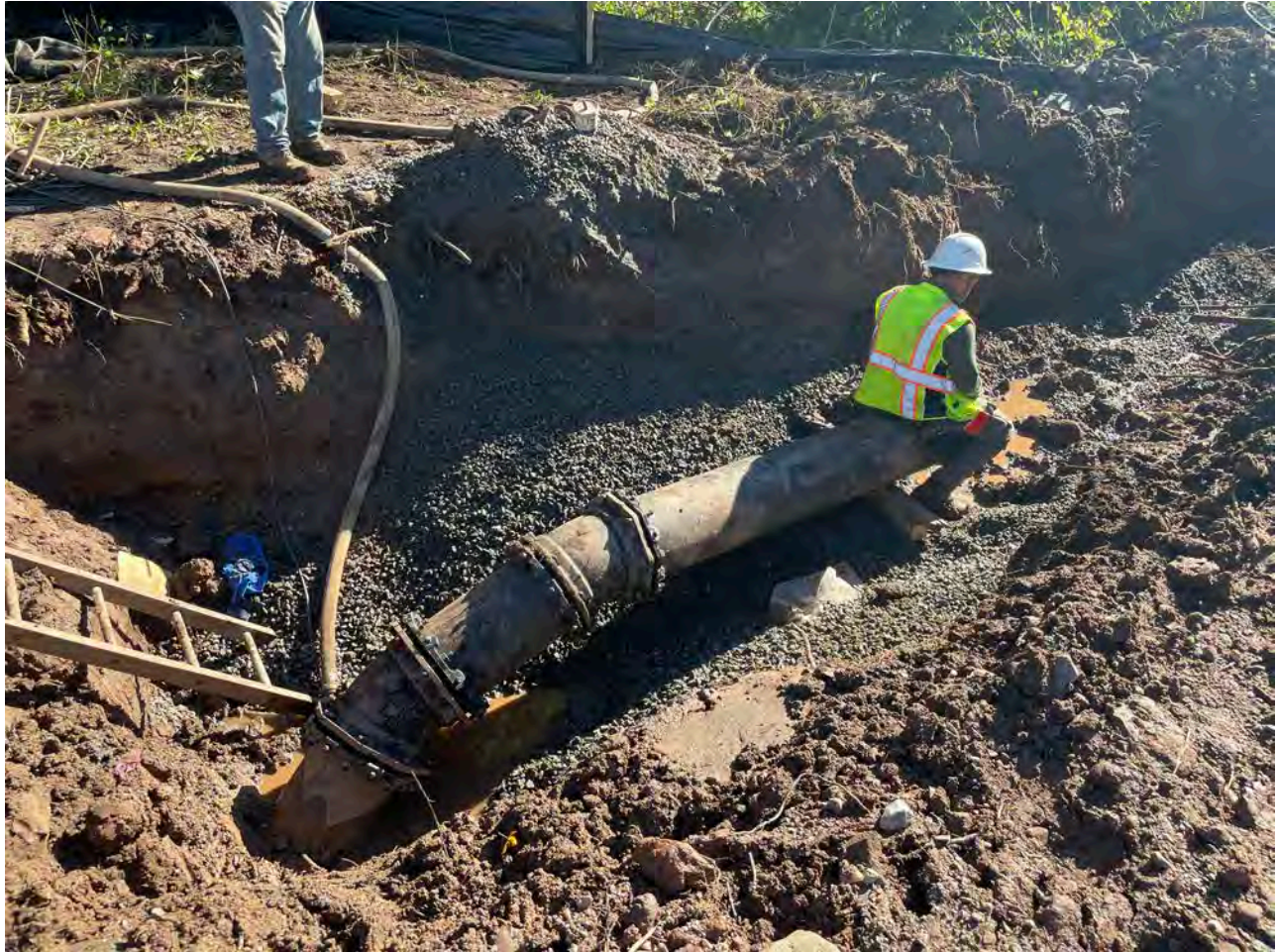
Picture 3: Section of 12" DIP that Ludlow connected to the 12" DIP coming off the east side of the Maiden Lane Stream crossing. View to the southeast.
