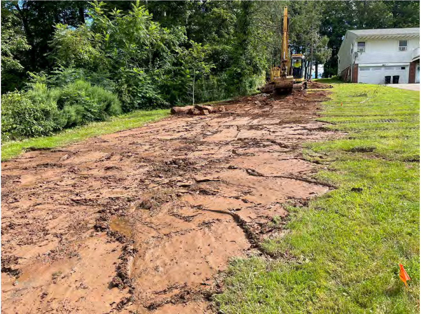
Picture 6: Portion of the lawn at 129 Maple Avenue that was disturbed during the installation of 1.5" copper water service line. View to the east.
