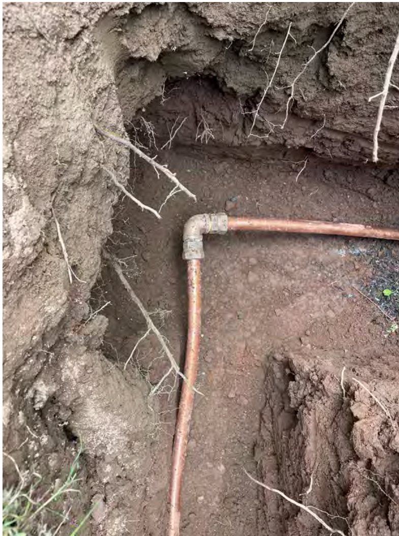
Picture 9: Union between two sections of 1.5" copper water service line that Ludlow installed at the 129 Maple Avenue residence.
