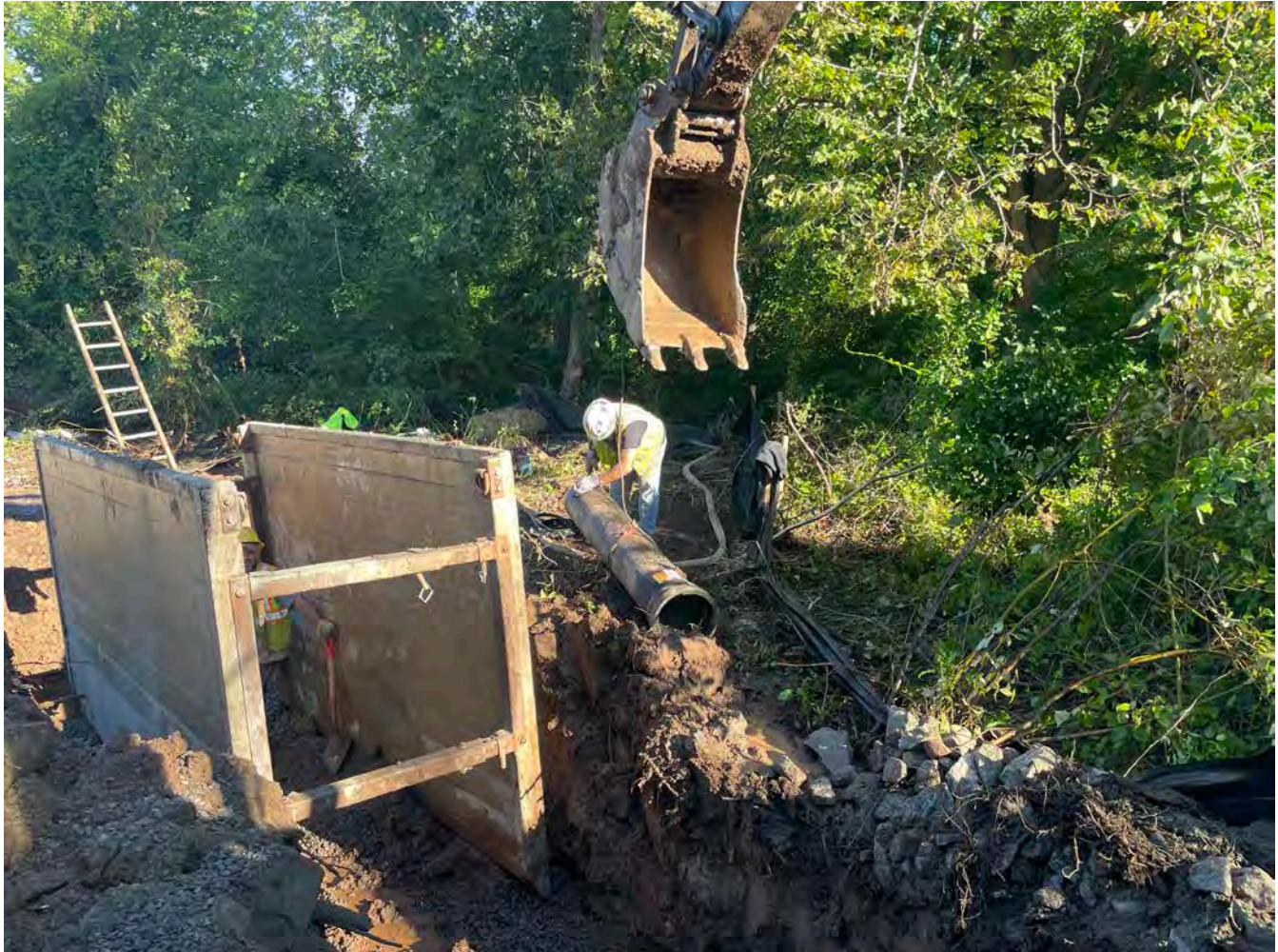
Picture 1: Ludlow installing 12" DIP to the northwest of Station 412+20. View to the north.
