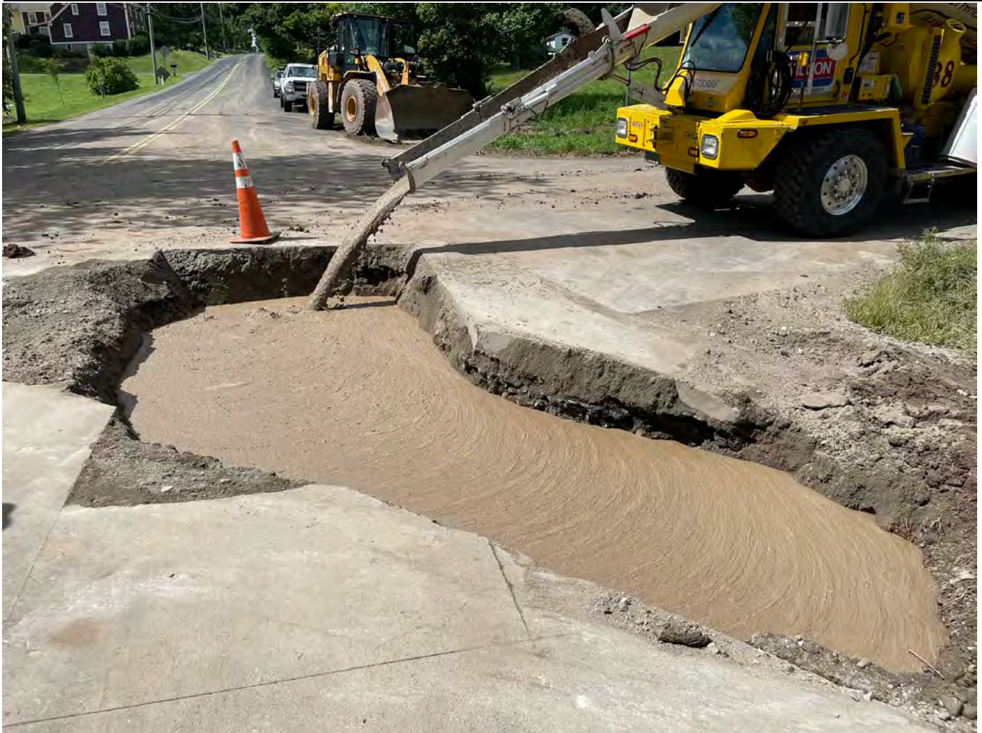
Picture 8: Tilcon placing flowable fill into the excavation at Station 410+47 under the direction of Ludlow. View to the west.
