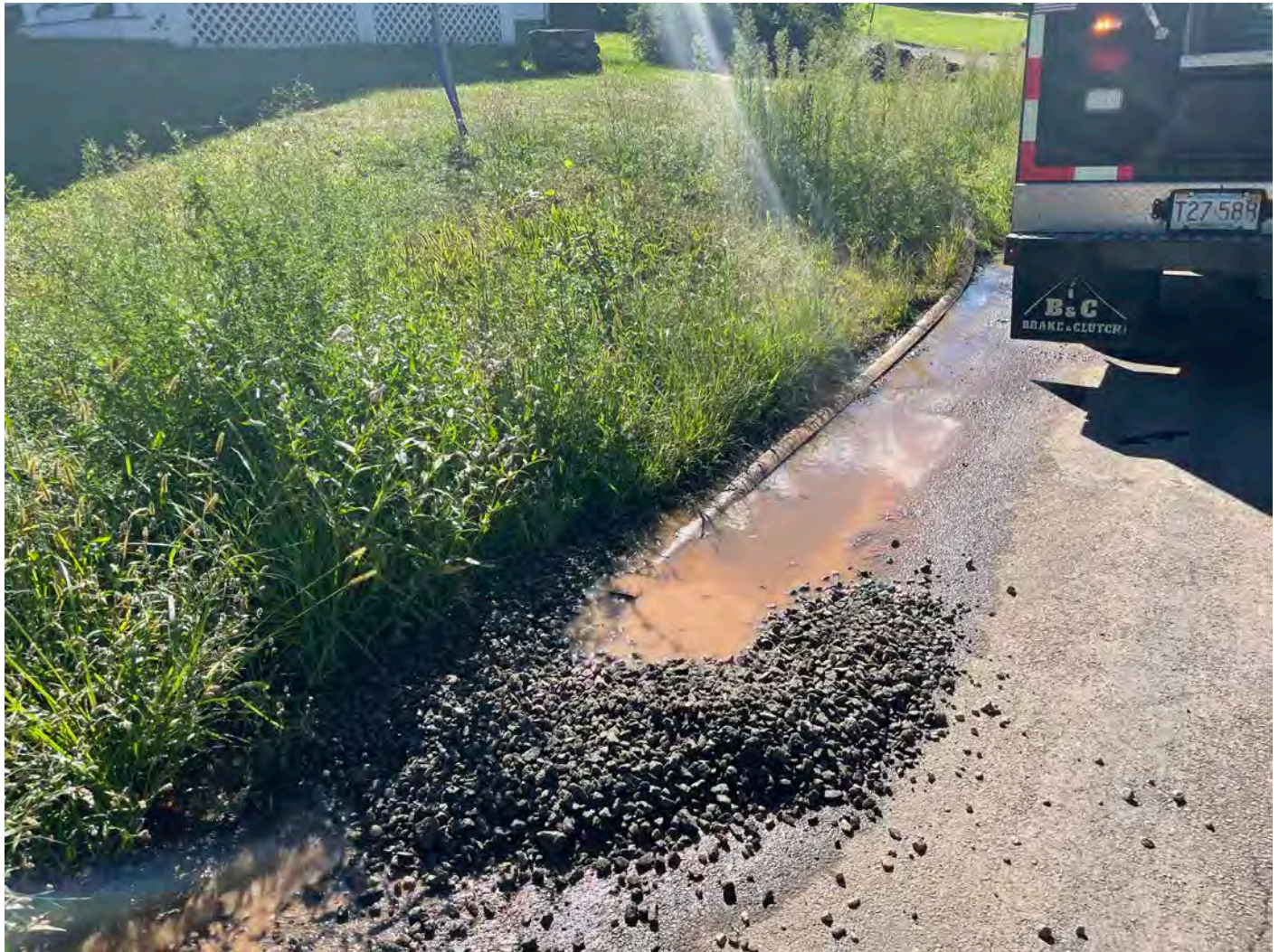
Picture 4: Water being discharged to the east side of Maple Avenue that is being pumped from the excavation at the 129 Maple Avenue, Durham, property. The water was later redirected into a silt bag. View to the southeast.
