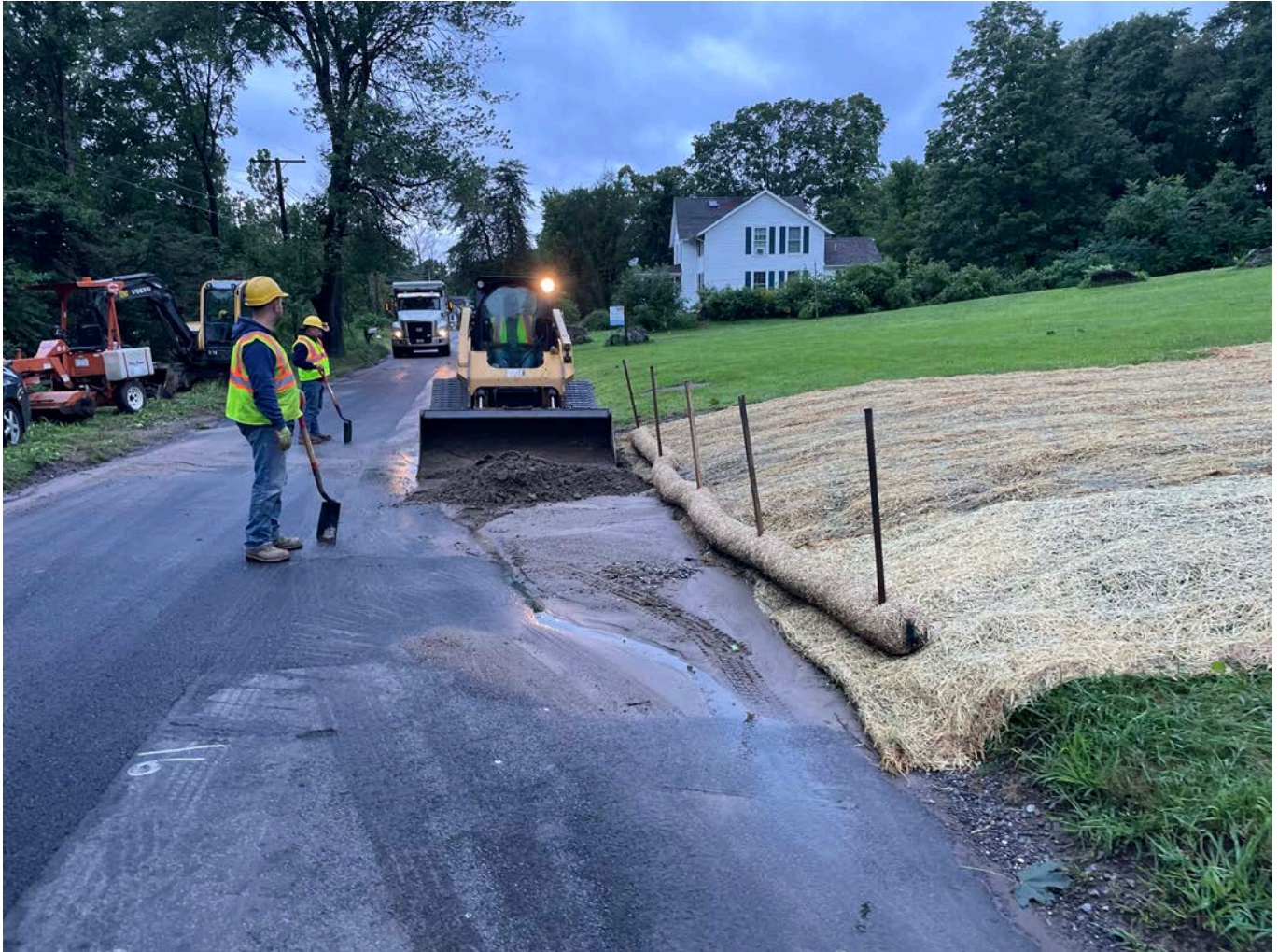
Picture 5: Ludlow cleaning up a small amount of silt/fines that washed off the 119 Maple Avenue property during last night's storm event. View to the north.
