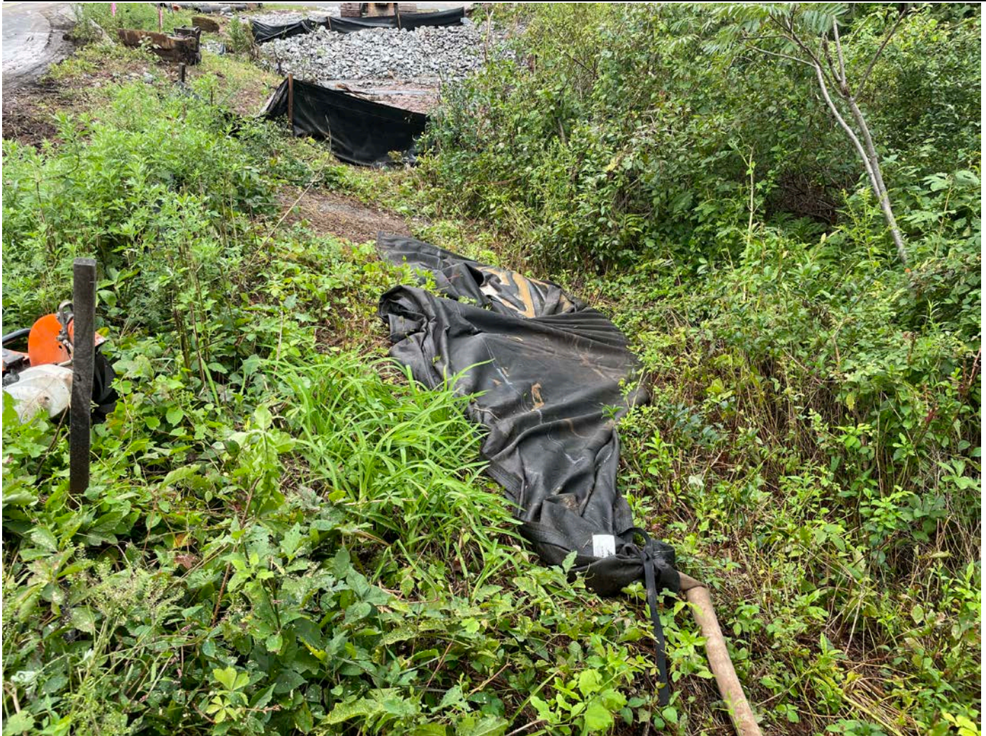
Picture 12: Silt bag Ludlow used to discharge water pumped from the excavation located at Station 412+20 Maiden Lane. View to the northwest.
