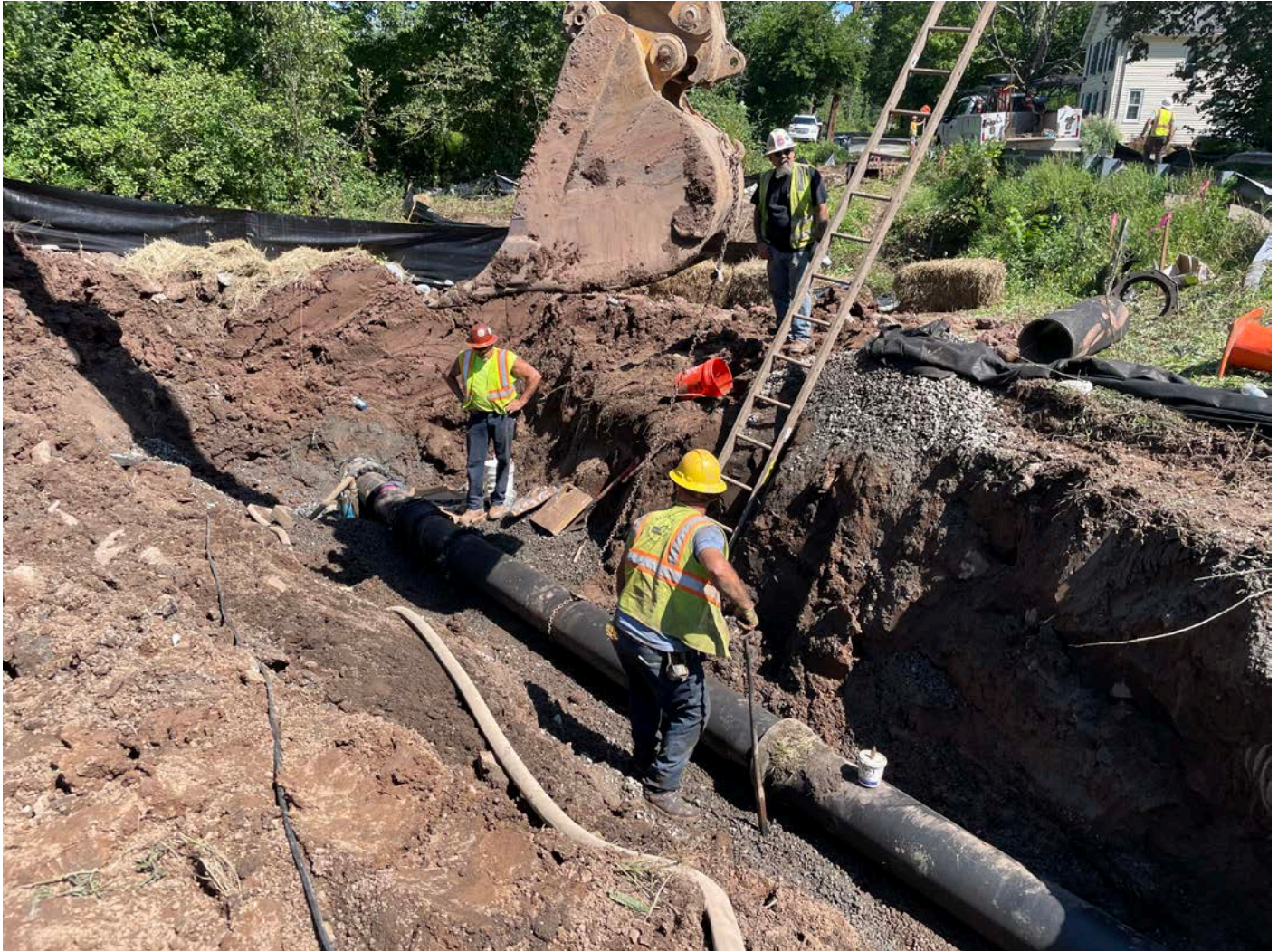
Picture 14: Ludlow placing the final section of 12" DIP on the west side of the Ball Brook stream crossing to complete the connection to 12" DIP that Ludlow installed in Maiden Lane last year. View to the east.
