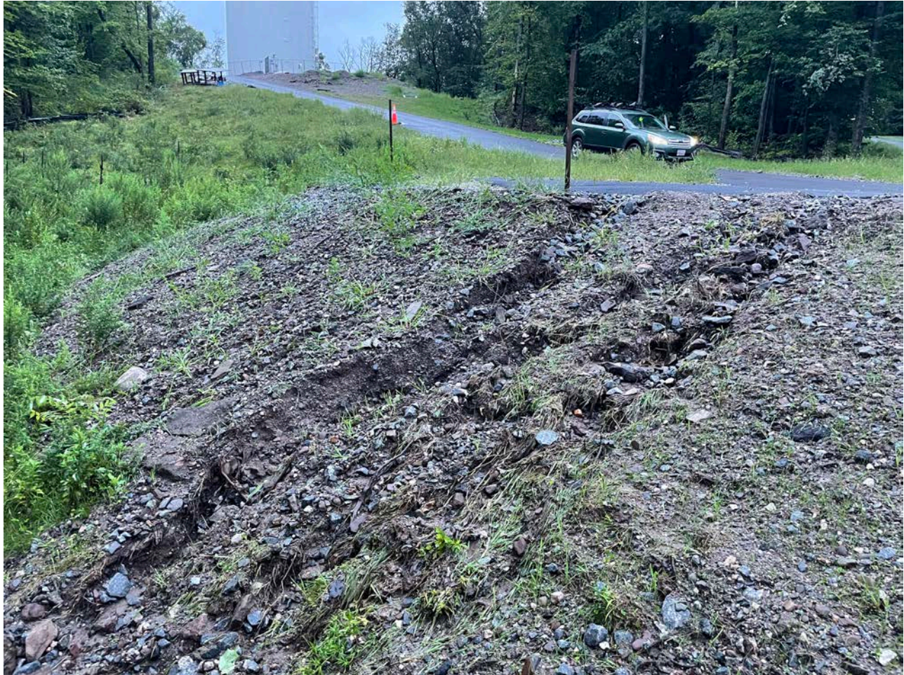
Picture 3: Rills located on the north side of the turnout on the Shared Access Driveway at Station 14+00 that were made deeper by last night's storm event. View to the southeast.
