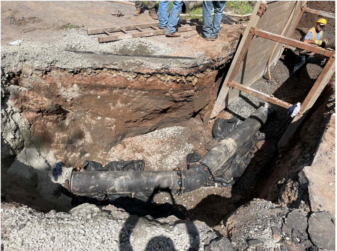
Picture 10: 12" DIP that Ludlow has placed between Stations 410+47 and ~411+30 west of Ball Brook as part of the Maiden Lane stream crossing. View to the north.
