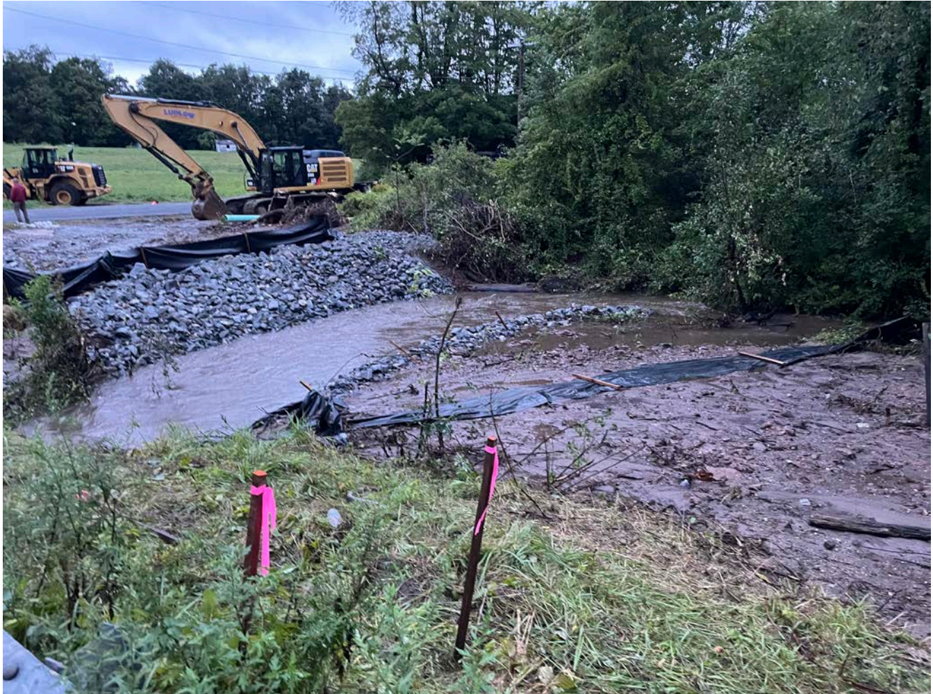
Picture 1: The Maiden Lane stream crossing, looking to the northwest. Heavy stream flow from last night's storm event has washed the hay bales that Ludlow placed on the east bank of Ball Brook downstream and flattened the silt fence.
