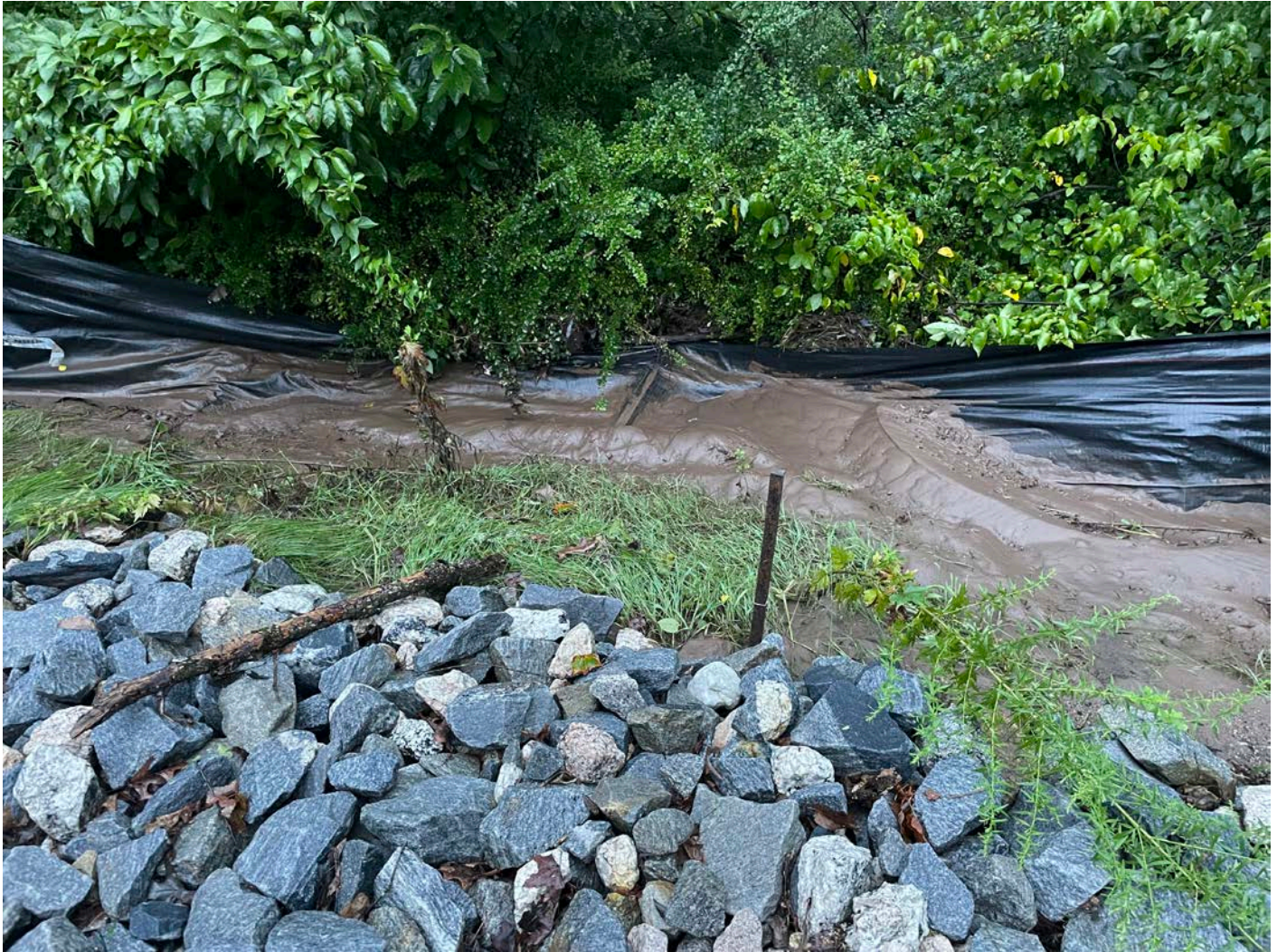
Picture 4: Sediment that has stacked up against the silt fence located on the north side of the Shared Access Driveway at Station 14+00. View to the north.
