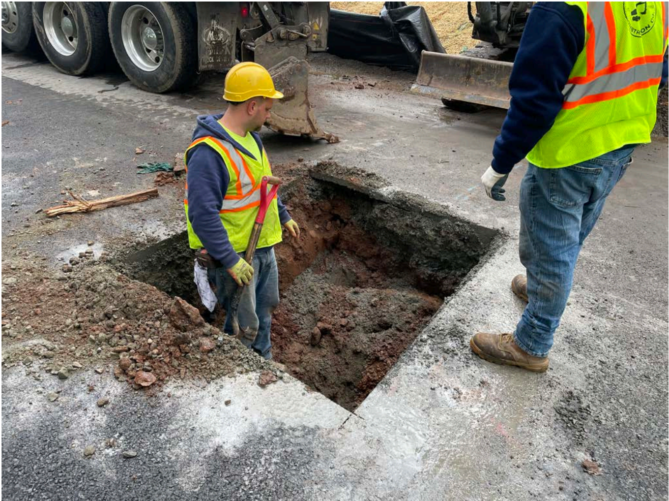
Picture 6: Ludlow daylighting the southbound lane of Maple Avenue to inspect corporation stop for the 109 Maple Avenue residence. View to the southeast.
