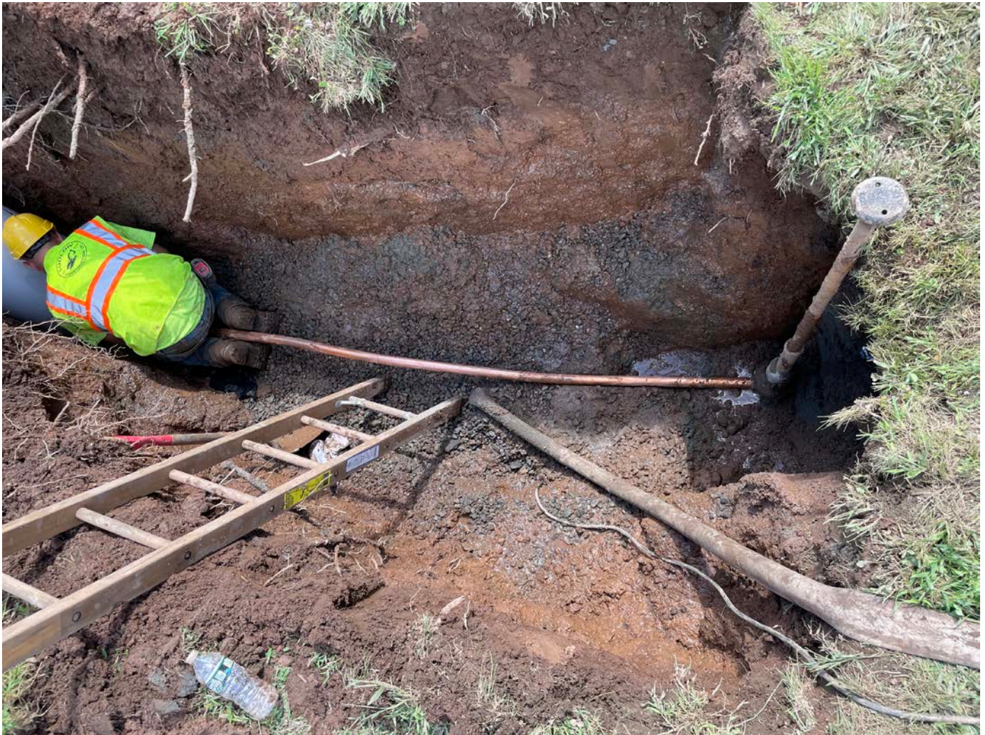
Picture 11: Ludlow placing 1.5" copper water service line between the curb stop and the meter pit for 129 Maple Avenue. View to the south.
