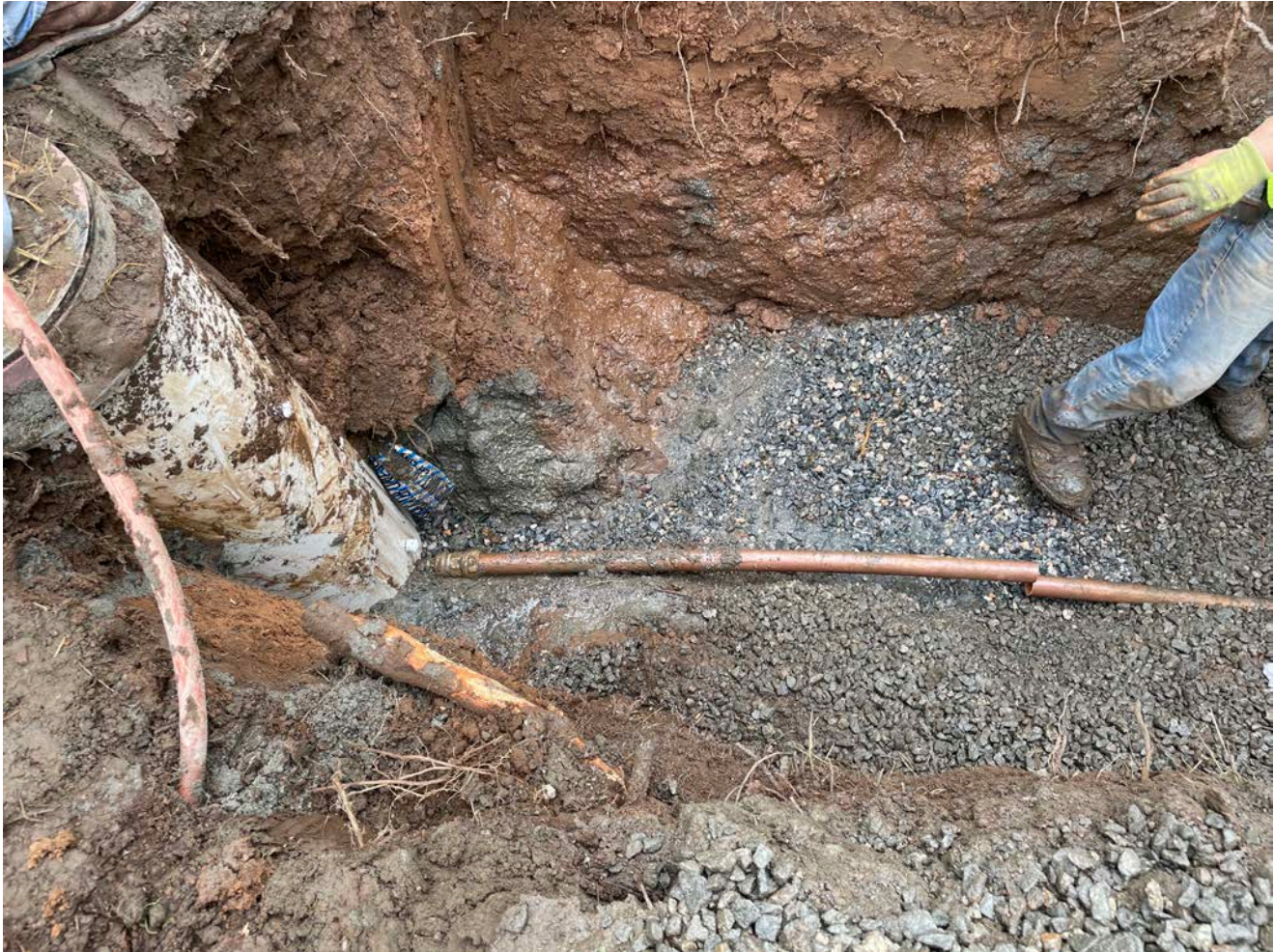
Picture 8: Ludlow located and cleared a clogged fitting where the copper water line connects to the west side of the meter pit at 109 Maple Avenue. View to the south.
