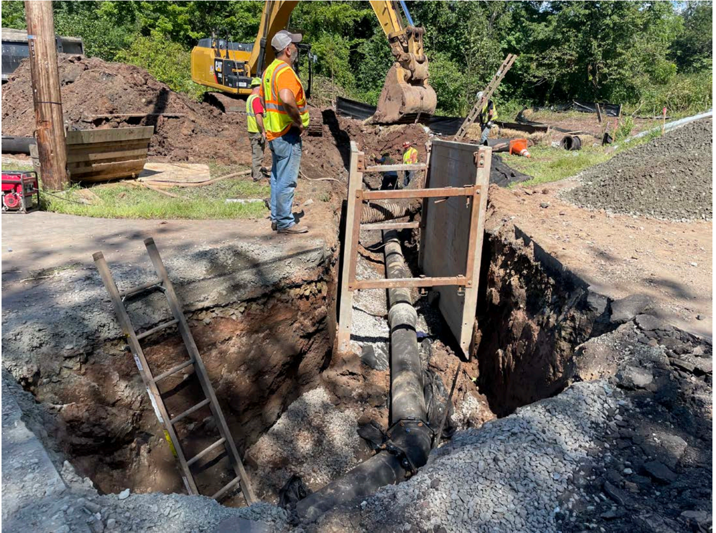
Picture 13: 12" DIP that Ludlow has placed from Stations 410+47 and 411+30 as part of the Maiden Lane stream crossing. View to the northeast.
