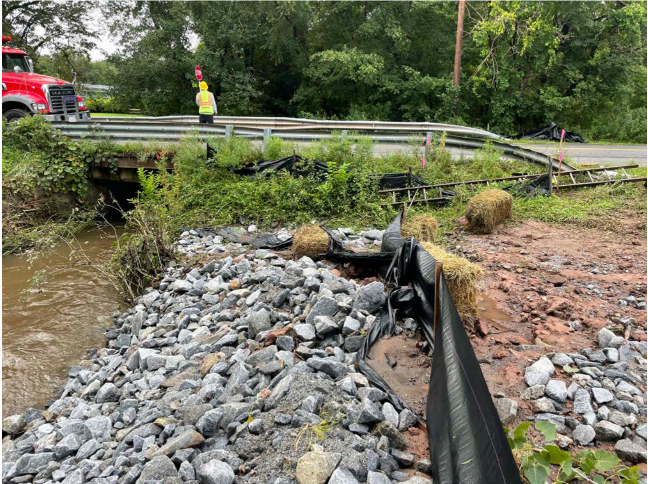
Picture 2: Silt fence and hay bales that Ludlow placed yesterday on the west bank of Ball Brook at the Maiden Lane stream crossing that were moved or damaged by last night's storm event. View to the south.
