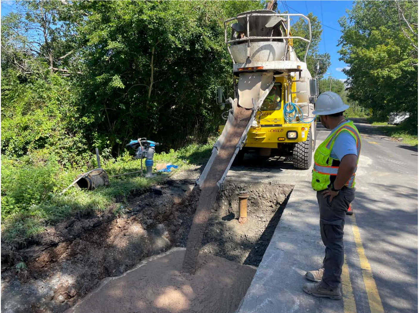
Picture 15: Ludlow overseeing a Tilcon truck placing flowable fill into the excavation at Station 412+20 Maiden Lane. View to the east.
