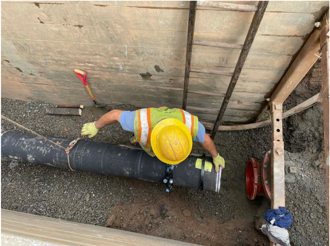
Picture 7: Ludlow inserting a section of 12" DIP into an existing gate valve located at Station 412+20 east of the Ball Brook stream crossing.
