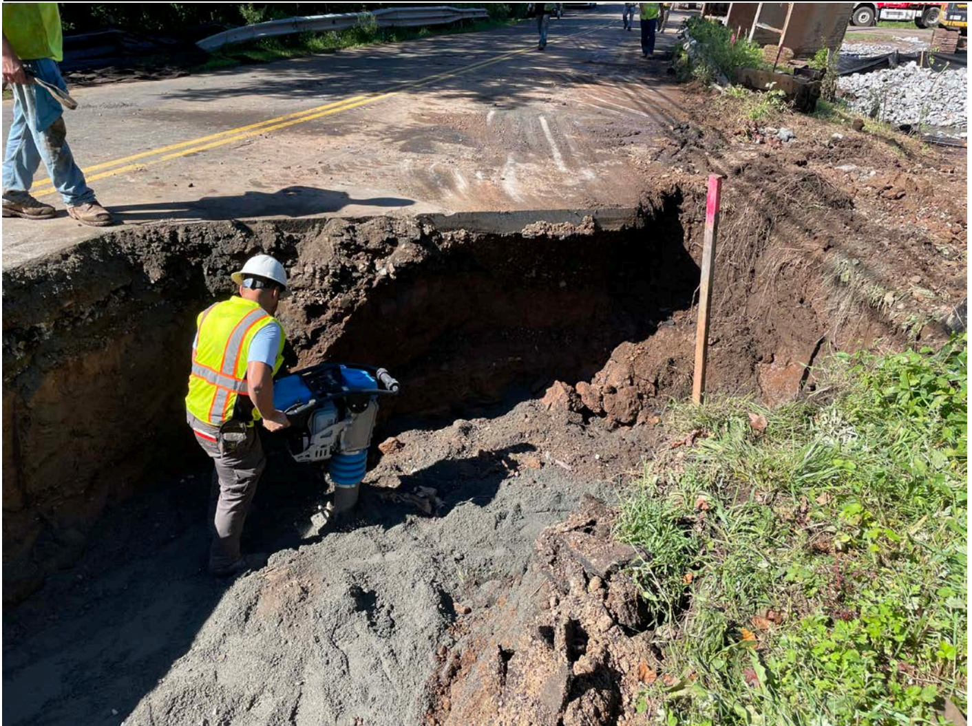
Picture 9: Ludlow compacting sand placed over 12" DIP they installed west of the gate valve at Station 412+20. View to the northwest.
