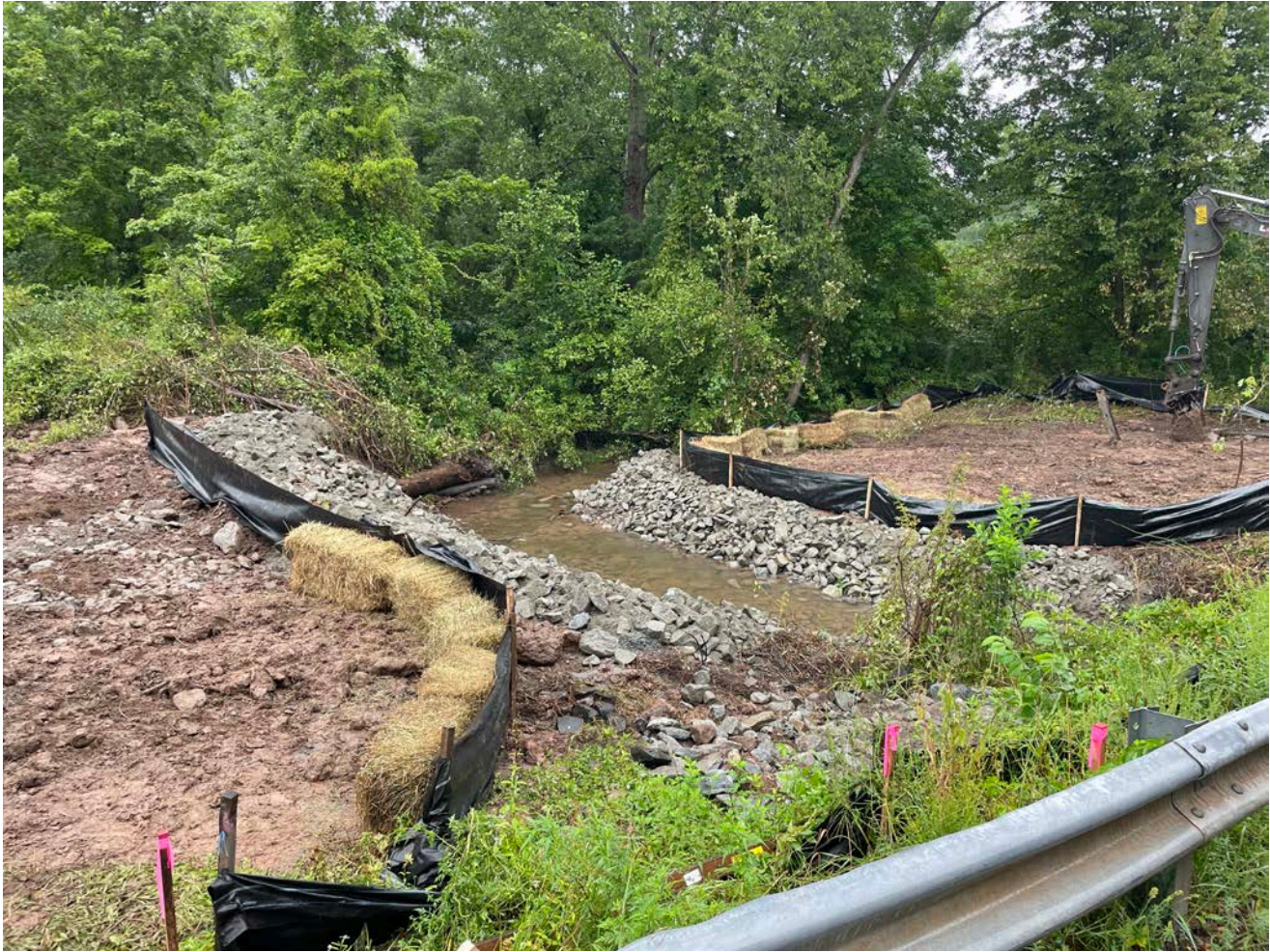
Picture 6: Overview of the Maiden Lane stream crossing after Ludlow has placed riprap on the stream bed and the banks of Ball Brook, and has placed silt fence and hay bales along each side of the stream bank. View to the northeast.
