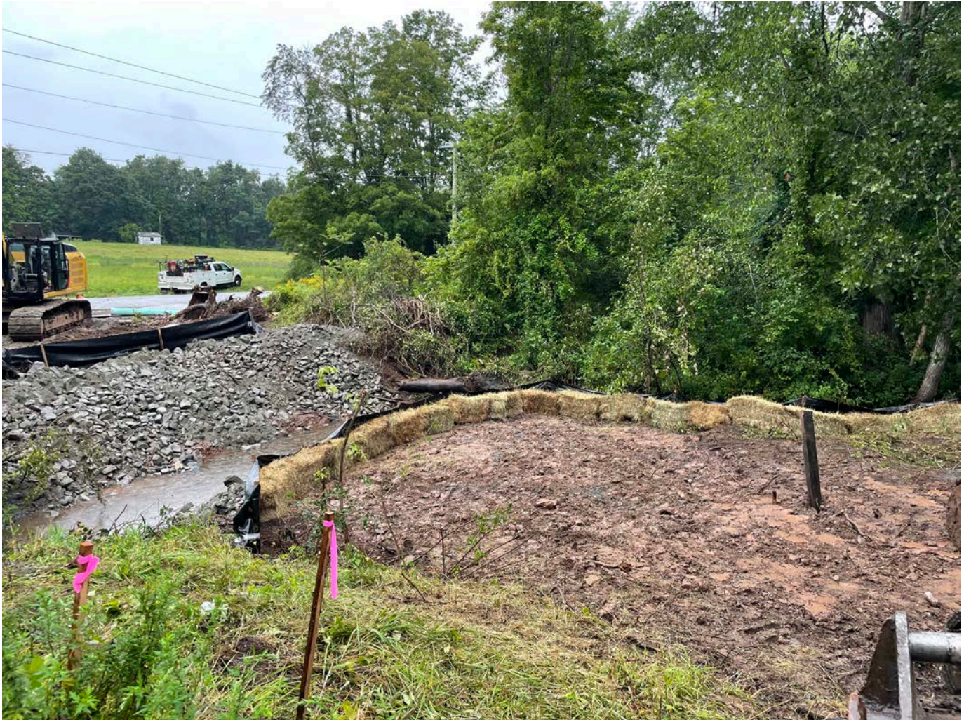
Picture 7: Overview of the Maiden Lane stream crossing after Ludlow has placed riprap on the stream bed and the banks of Ball Brook and has placed silt fence and hay bales along each side of the stream bank. View to the northwest.
