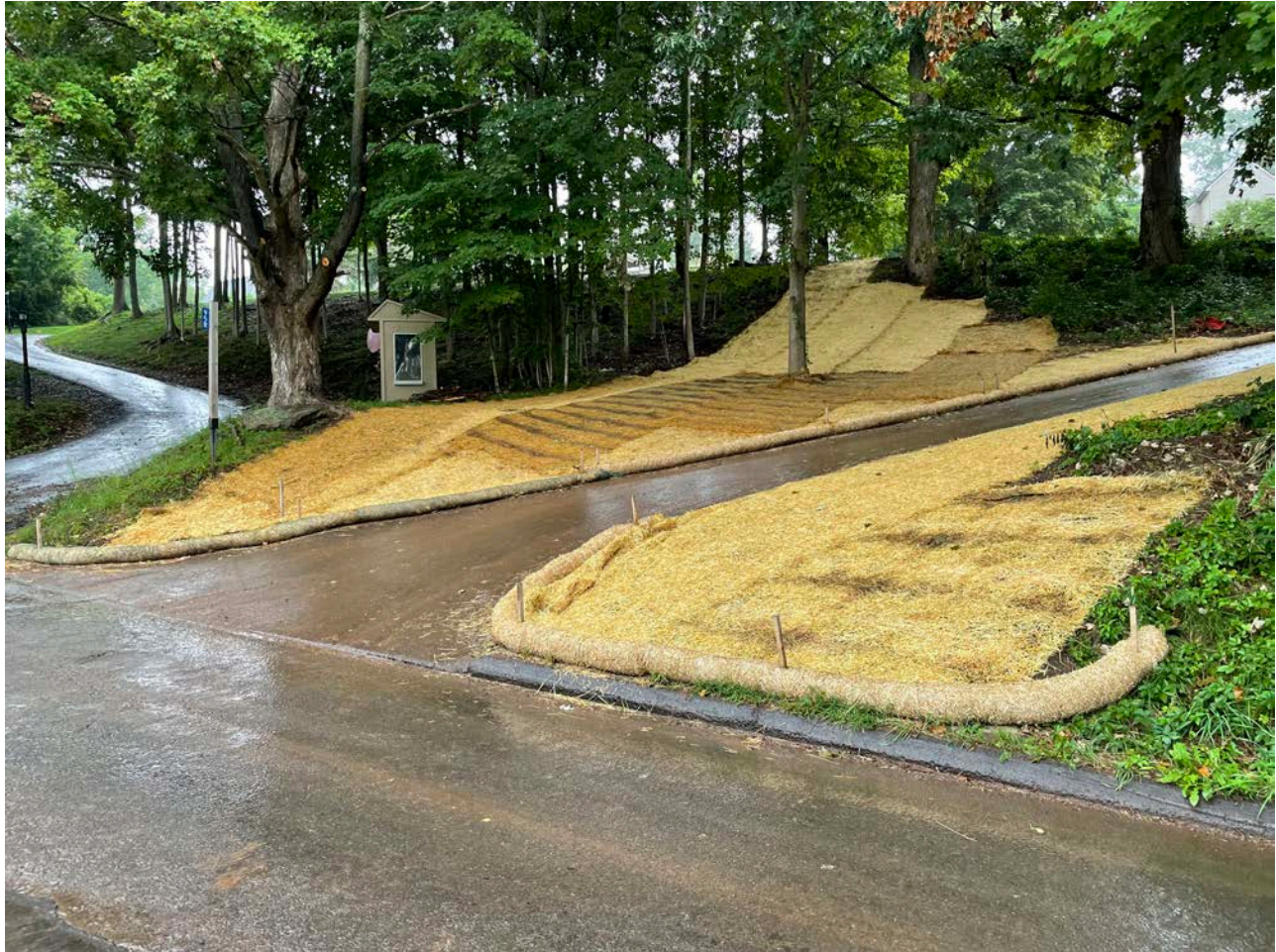
Picture 3: Erosion control that Ludlow has placed on either side of the driveway for the 95R Maple Avenue property. View to the northeast.
