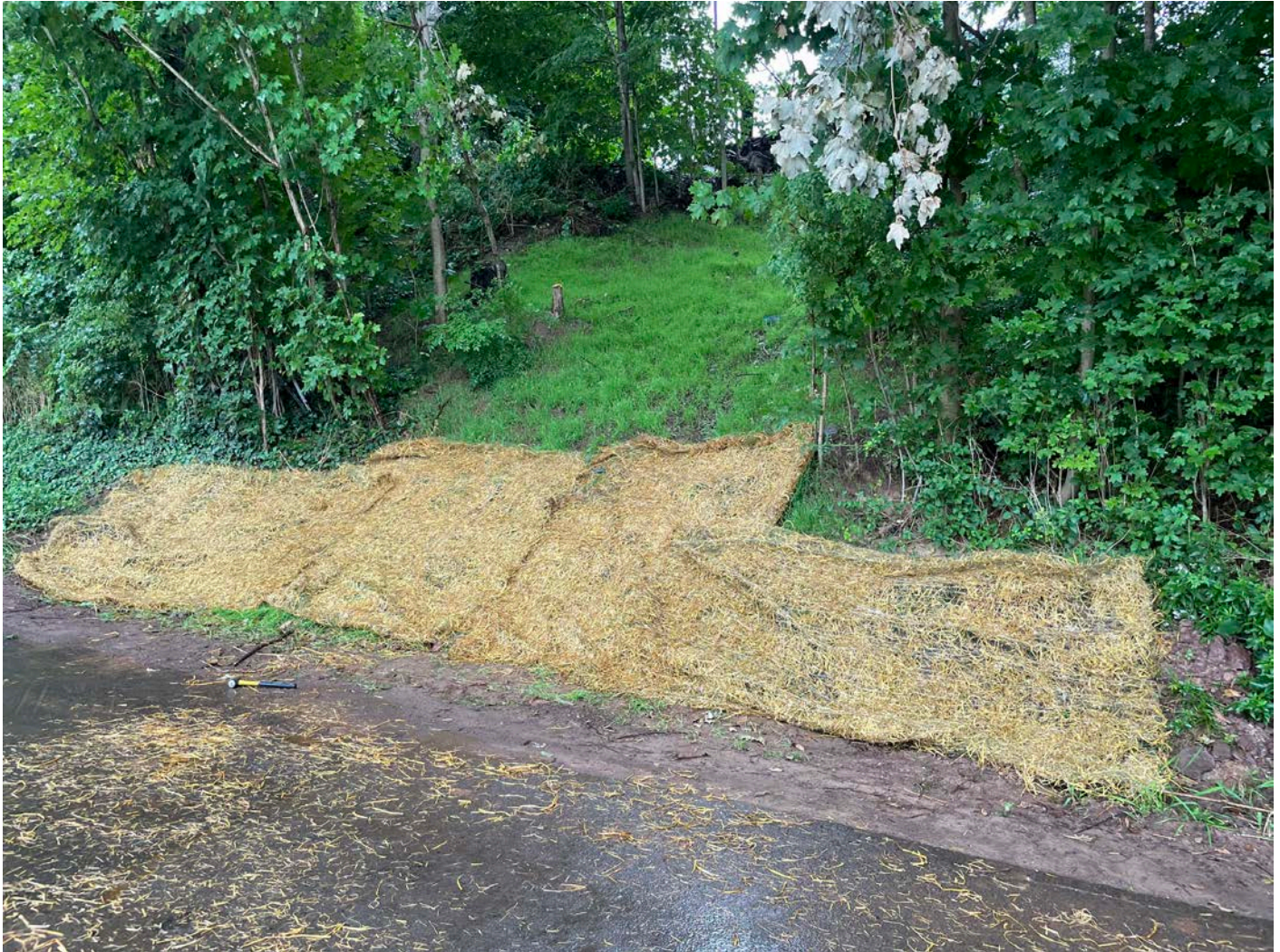
Picture 4: Erosion control that Ludlow has placed on either side of the driveway for the 95R Maple Avenue property. View to the east.
