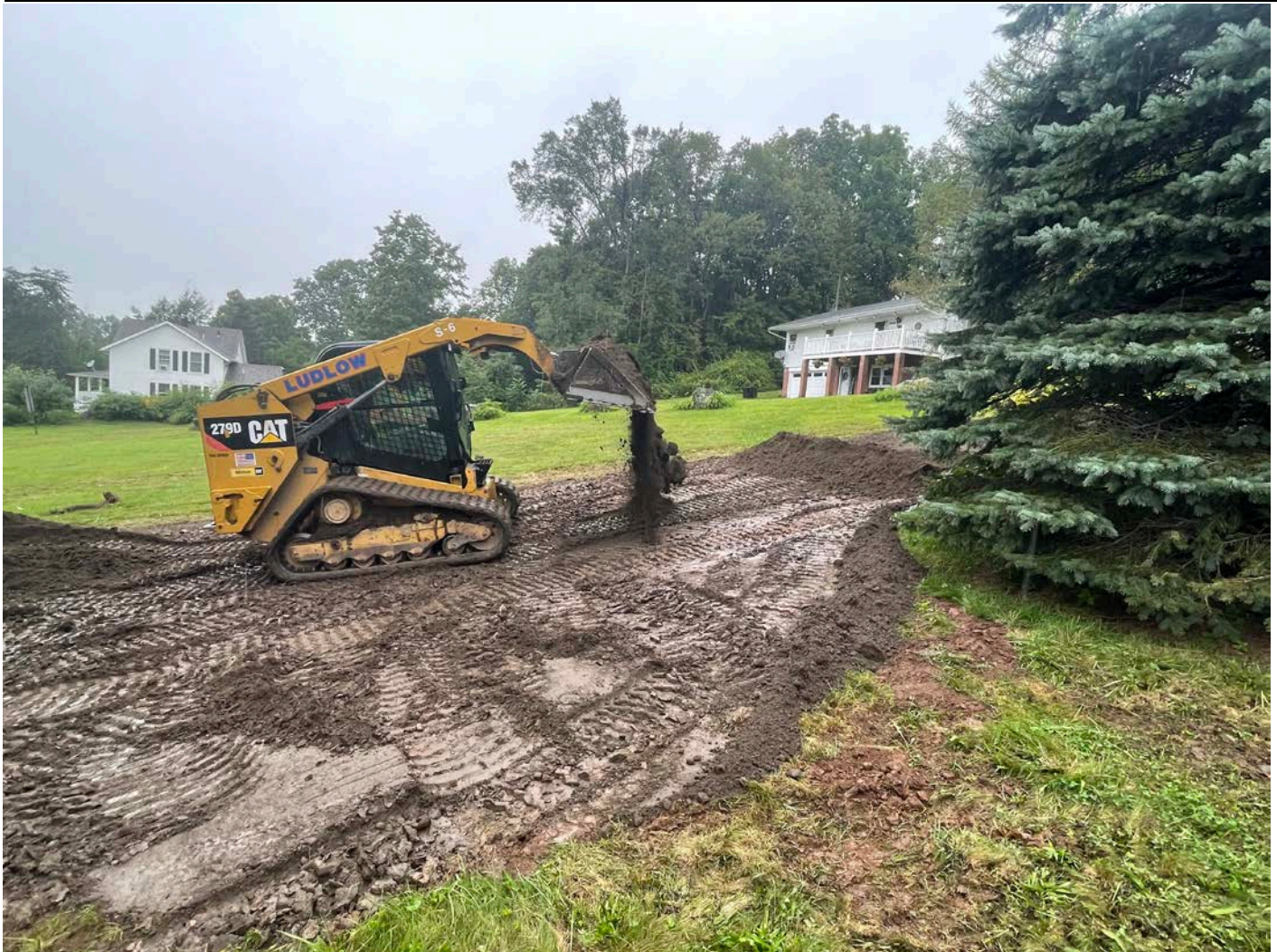
Picture 9: Ludlow placing loam at the 119 Maple Avenue residence to repair the portions of the lawn that were disturbed during the installation of a 1.5" copper water service. View to the northeast.
