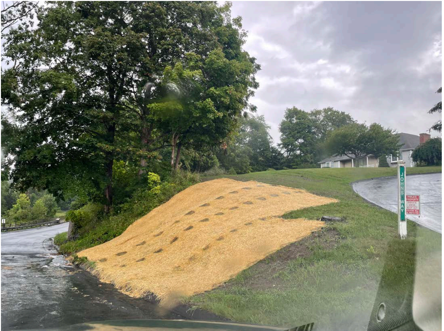
Picture 10: Erosion control that Ludlow has placed at the 10 Johns Way property. View to the northeast.
