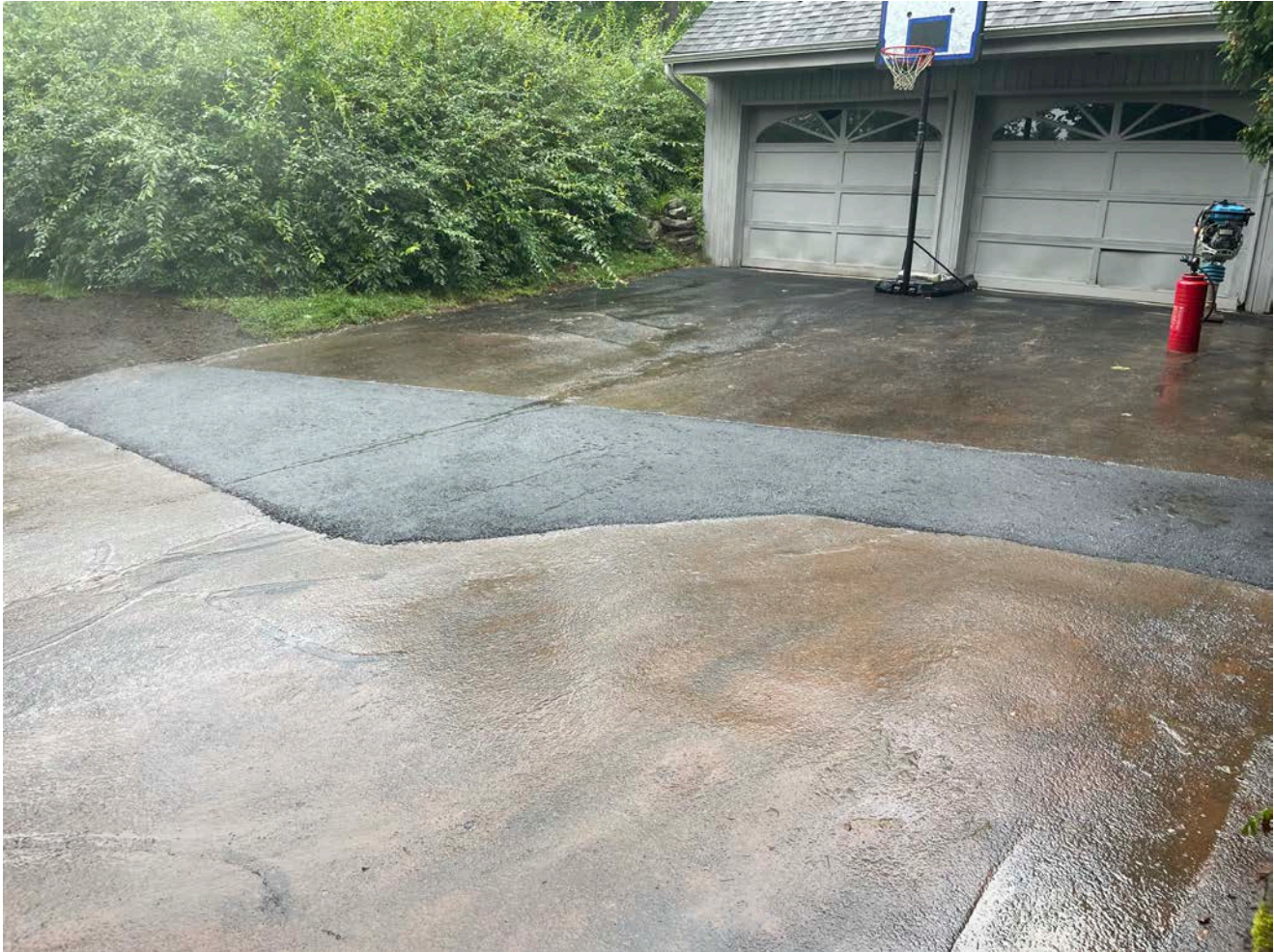
Picture 8: Asphalt patch that Ludlow placed to close he trench they cut across the driveway for 119 Maple Avenue property during the installation of a 1.5" copper water service line. View to the northeast.
