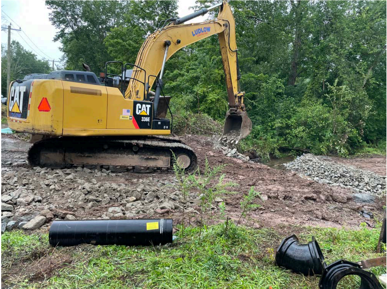
Picture 2: Ludlow placing riprap on the western bank of Ball Brook as part of restoration activities following the Maiden Lane stream crossing. View to the north.
