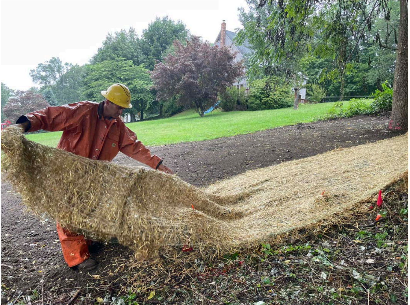
Picture 5: Ludlow placing straw mats at the 119 Maple Avenue. View to the north.
