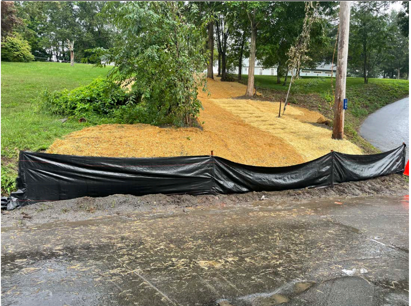
Picture 12: Erosion control that Ludlow has placed at the 109 Maple Avenue property. View to the east.
