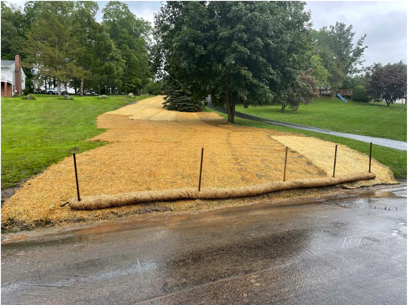
Picture 11: Erosion control that Ludlow has placed at the 119 Maple Avenue property. View to the east.
