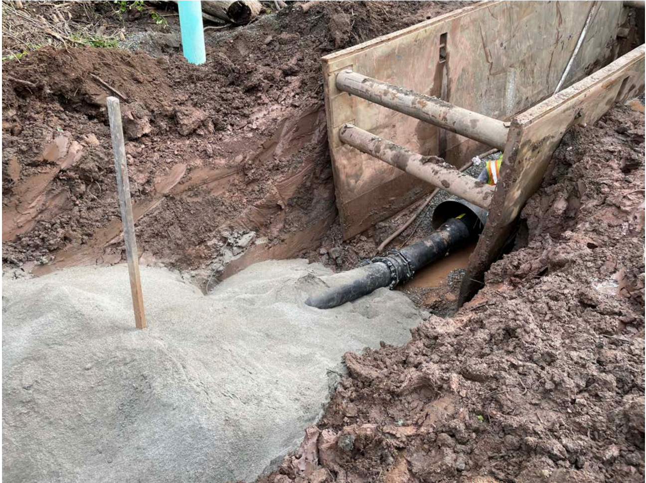
Picture 2: View of the western side of the trench box at the Maiden Lane stream crossing, looking northeast. Ludlow has connected ~12' section of 12" DIP to the 22.5° DIP bend they just installed and has begun to place sand over the DIP.
