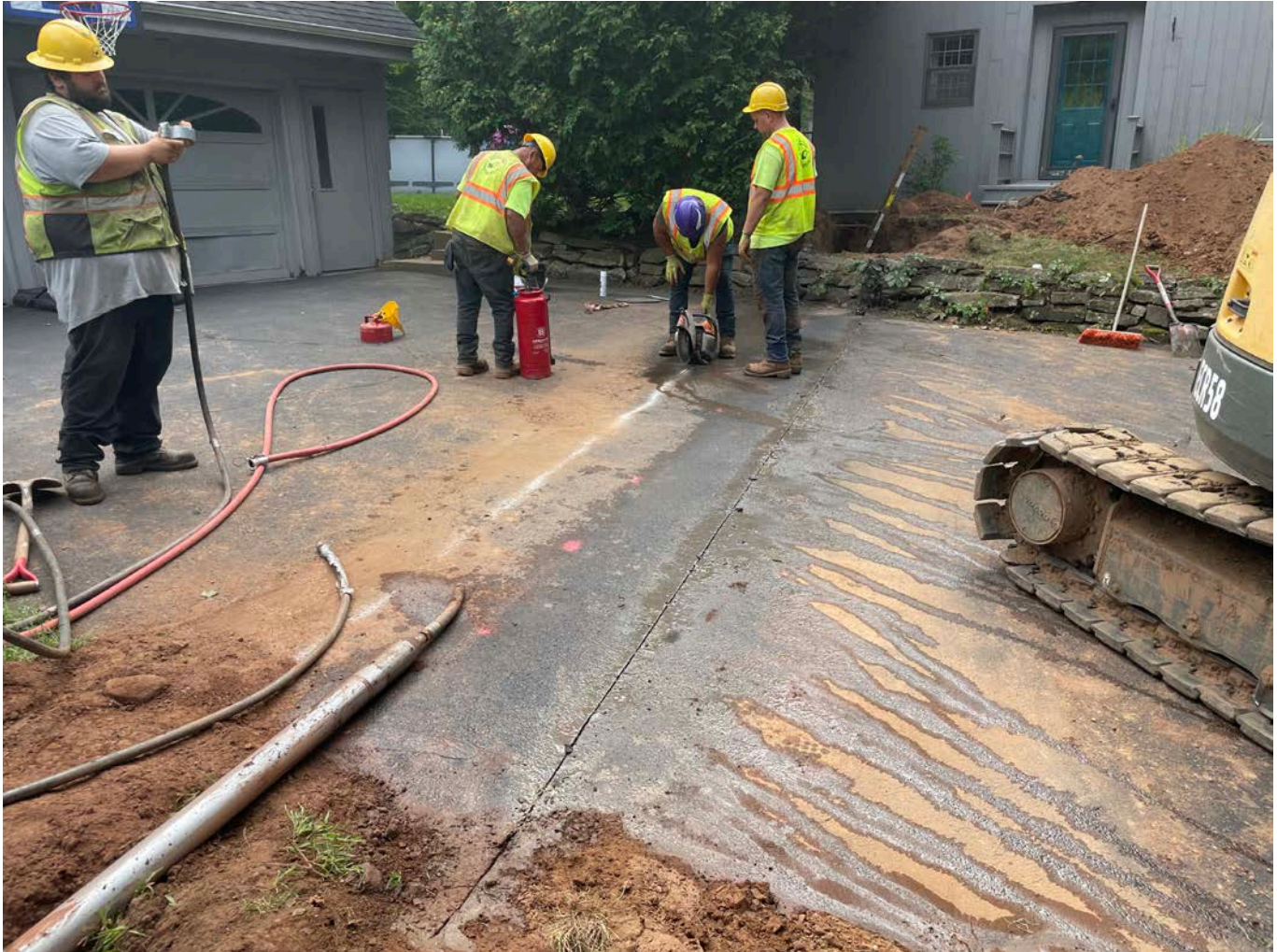
Picture 5: Ludlow saw cutting asphalt on the driveway for the 119 Maple Avenue property as part of the installation of a 1.5" copper water service line. View to the southeast.
