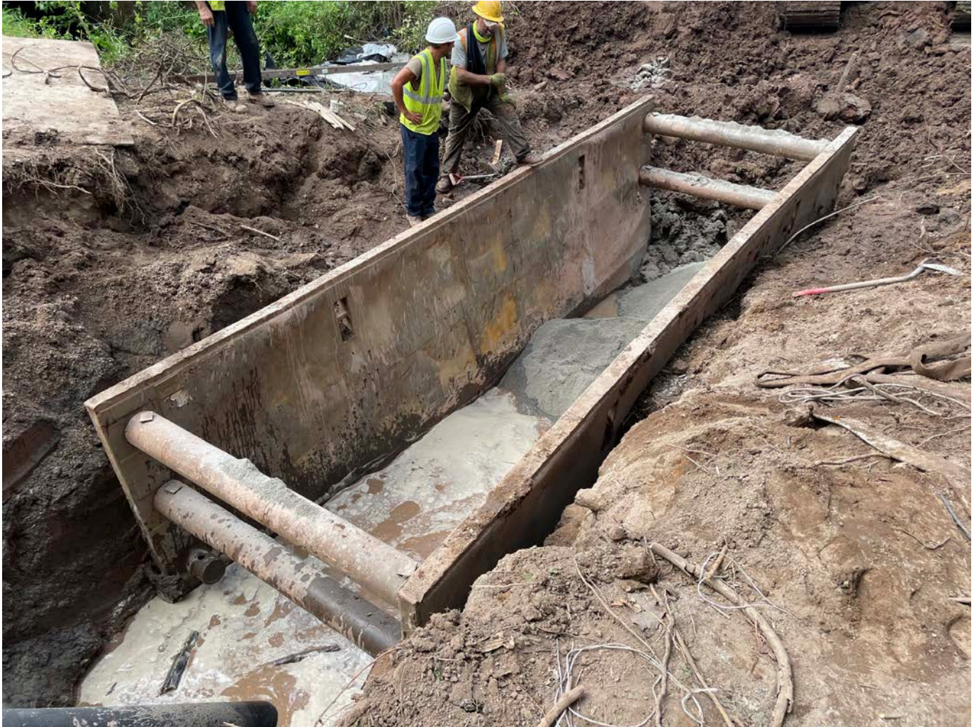
Picture 7: Sand that Ludlow has begun to place over the 36" steel casing that is located within the footprint of the trench box at the Maiden Lane stream crossing. View to southwest.
