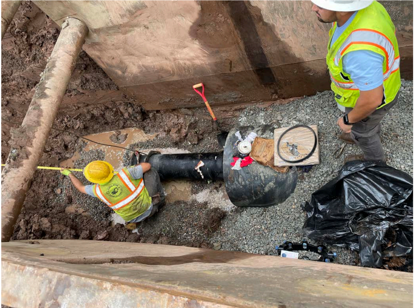
Picture 1: View of the western side of the trench box at the Maiden Lane stream crossing, looking north. Ludlow has connected a short piece of 12" DIP to the section of 12" DIP located inside of the 36" steel conduit and has added a 22.5° DIP bend.
