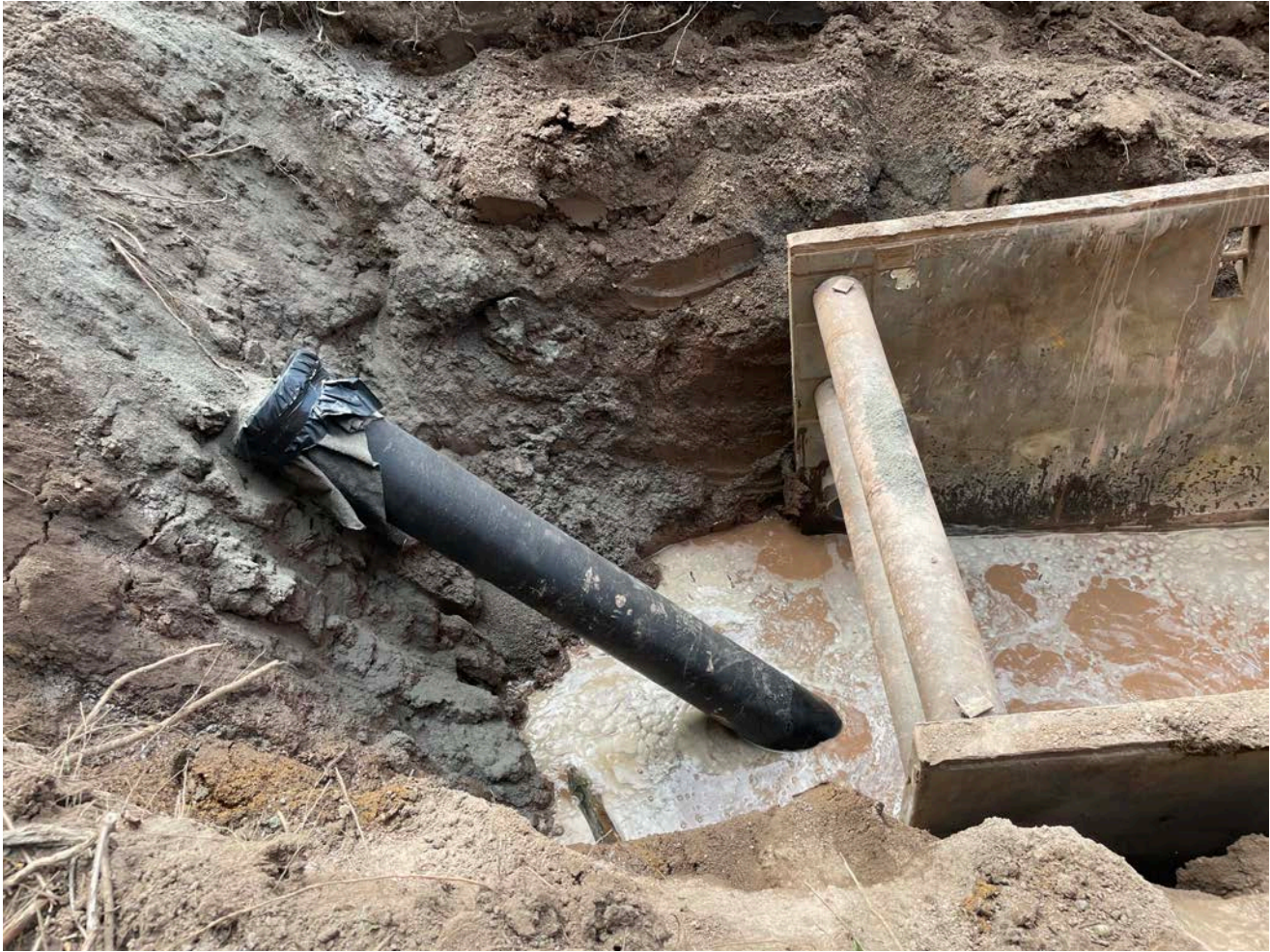
Picture 6: View of the eastern side of the trench box at the Maiden Lane stream crossing, looking south. Ludlow has connected a ~10 section of 12" DIP to a 45° DIP bend they just installed.
