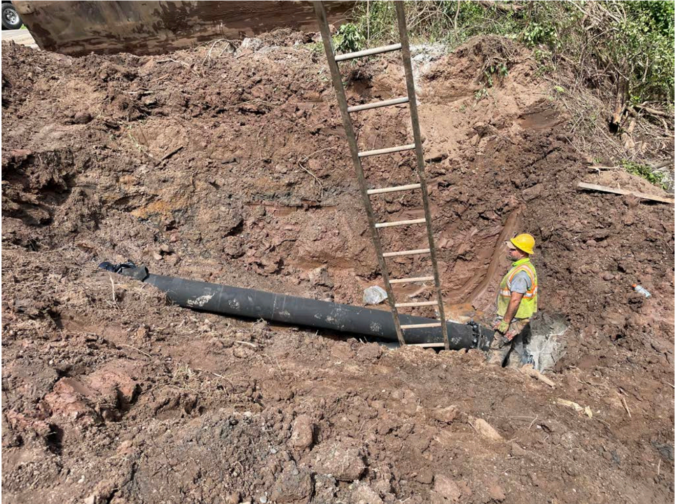
Picture 8: Additional 12" DIP that Ludlow has installed on the western bank of Ball Brook as part of the Maiden Lane stream crossing. View to the north.
