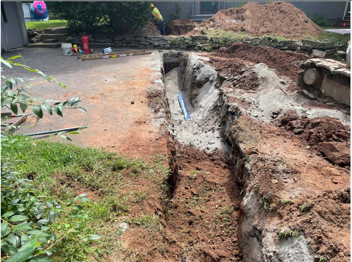
Picture 9: Driveway at the 119 Maple Avenue residence where Ludlow is placing sand followed by caution tape followed by native fill over the 1.5" copper water service line they just installed. View to the south.
