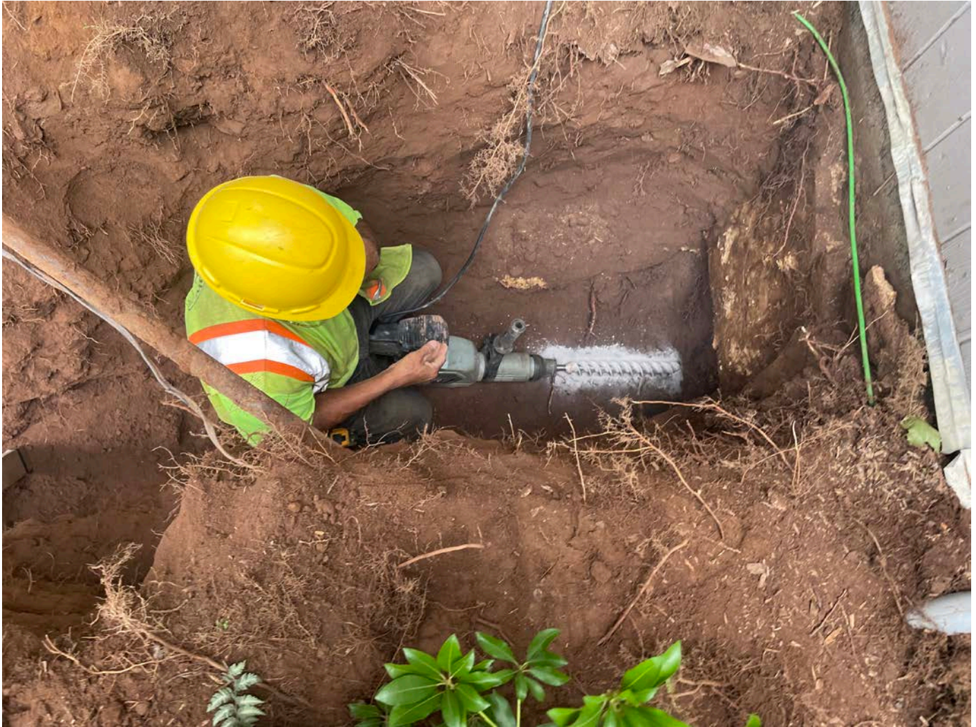
Picture 4: Ludlow using a rotary hammer to penetrate the concrete foundation of the 119 Maple Avenue property for the installation of a 1.5" copper water service line.
