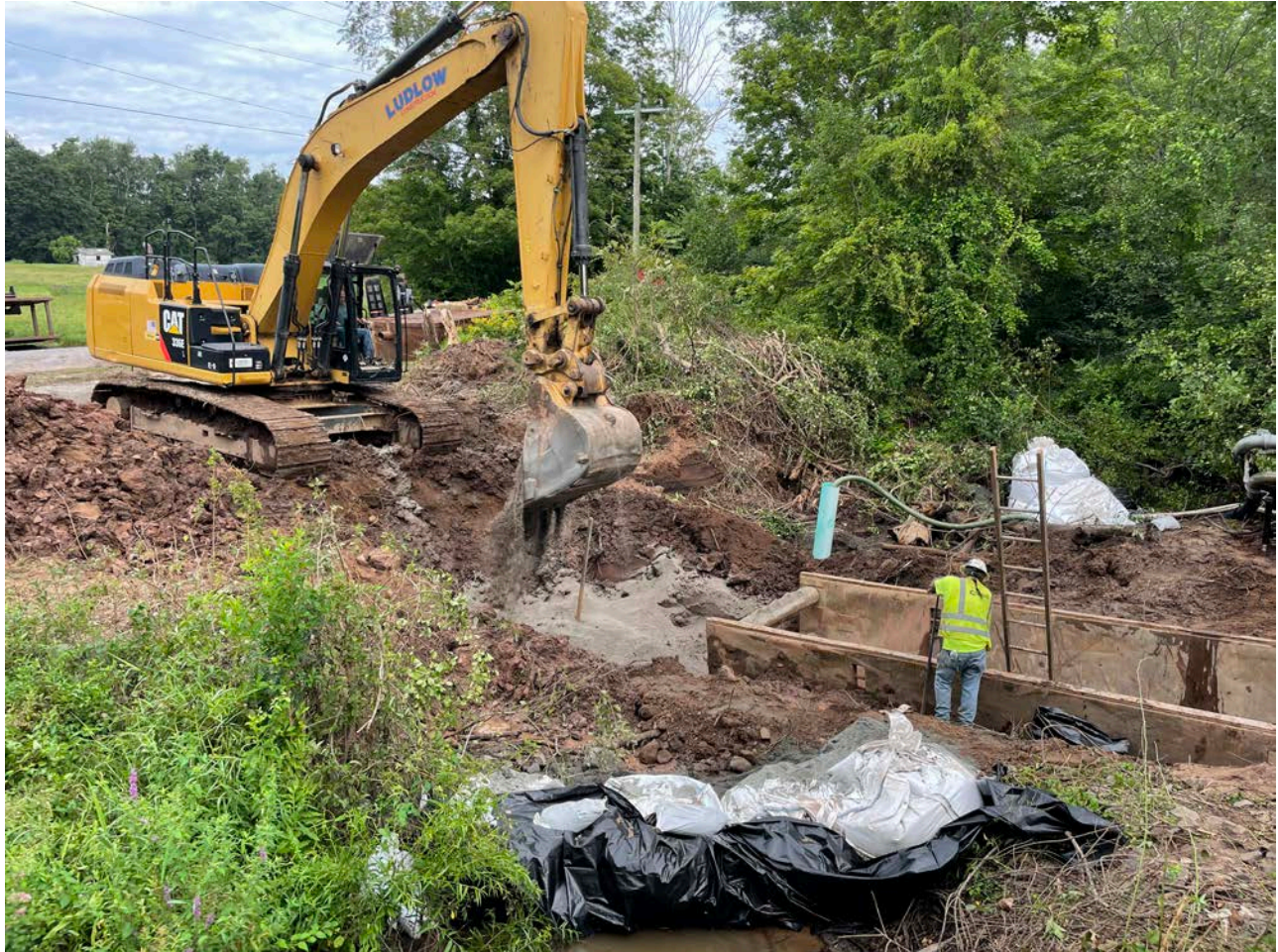
Picture 3: Ludlow placing sand over newly-installed 12" DIP on the west side of the trench box at the Maiden Lane stream crossing. View to the northwest.
