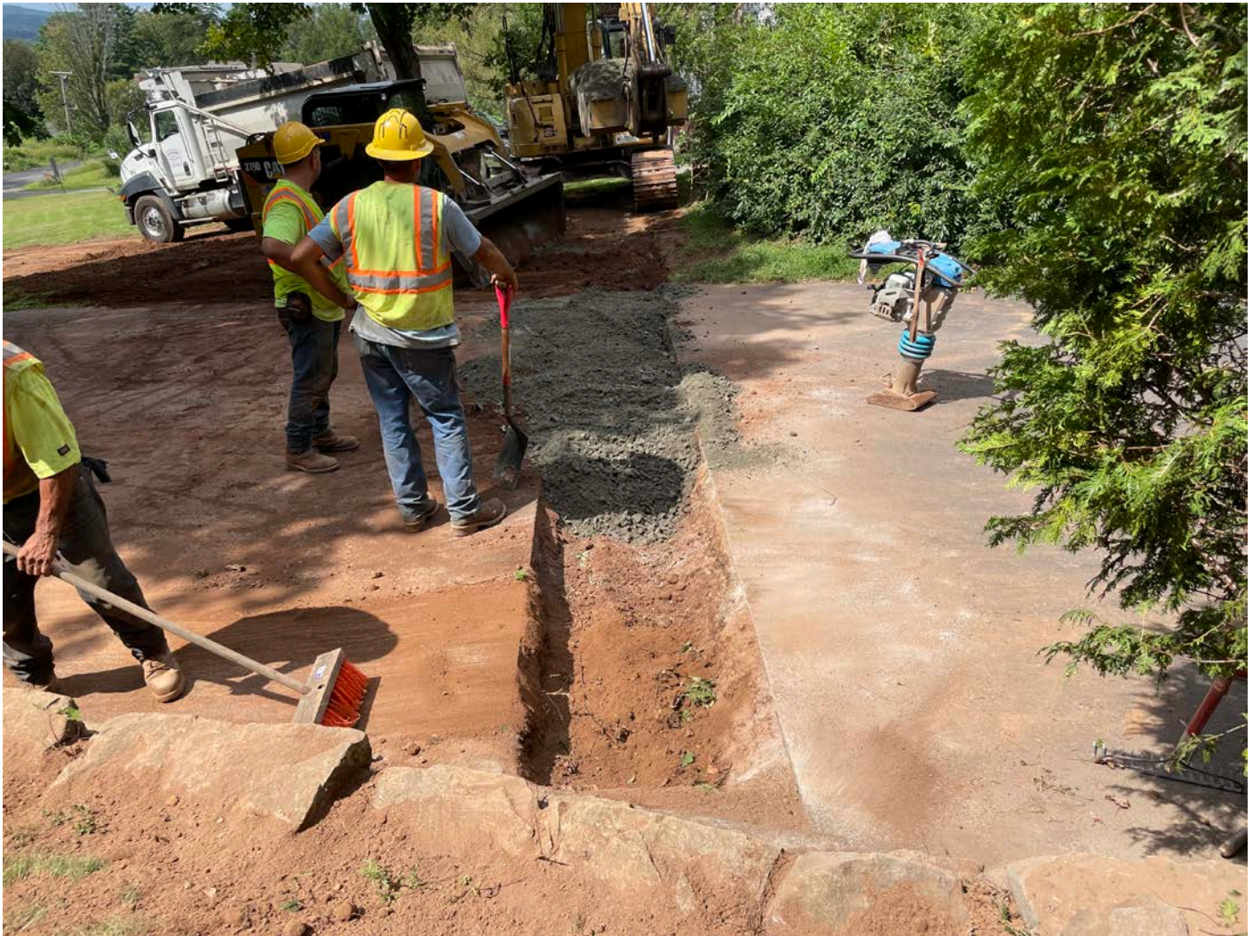
Picture 11: Driveway at the 119 Maple Avenue residence where Ludlow is placing 1'-1.5' of 1.5" gravel as the final backfill over the 1.5" copper water service line they just installed. View to the north.
