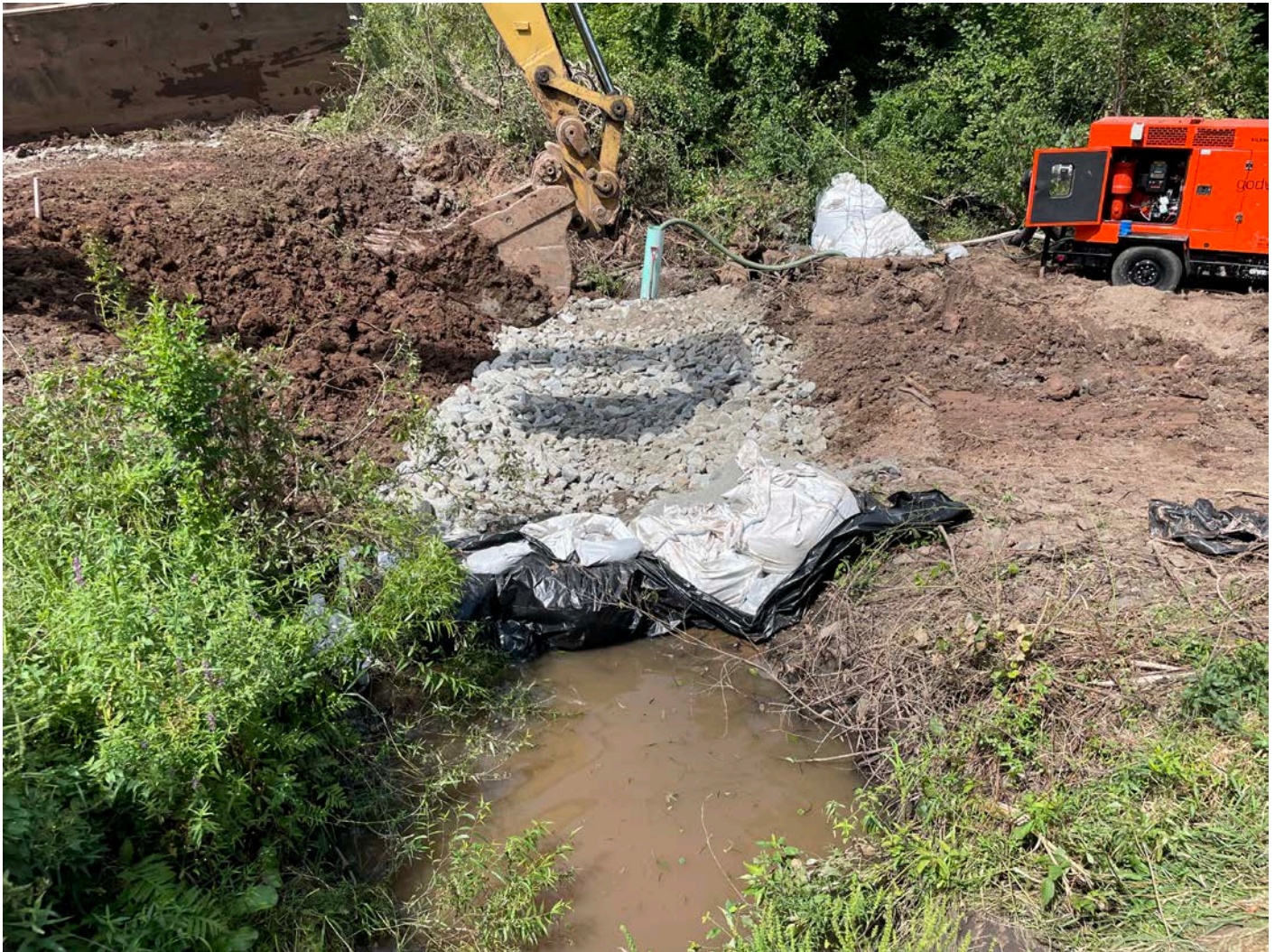
Picture 10: Overview of the Maiden Lane stream crossing. Ludlow has placed rip rap on the stream bed of Ball Brook and has begun to reconstruct the west bank of the brook. View to the north.
