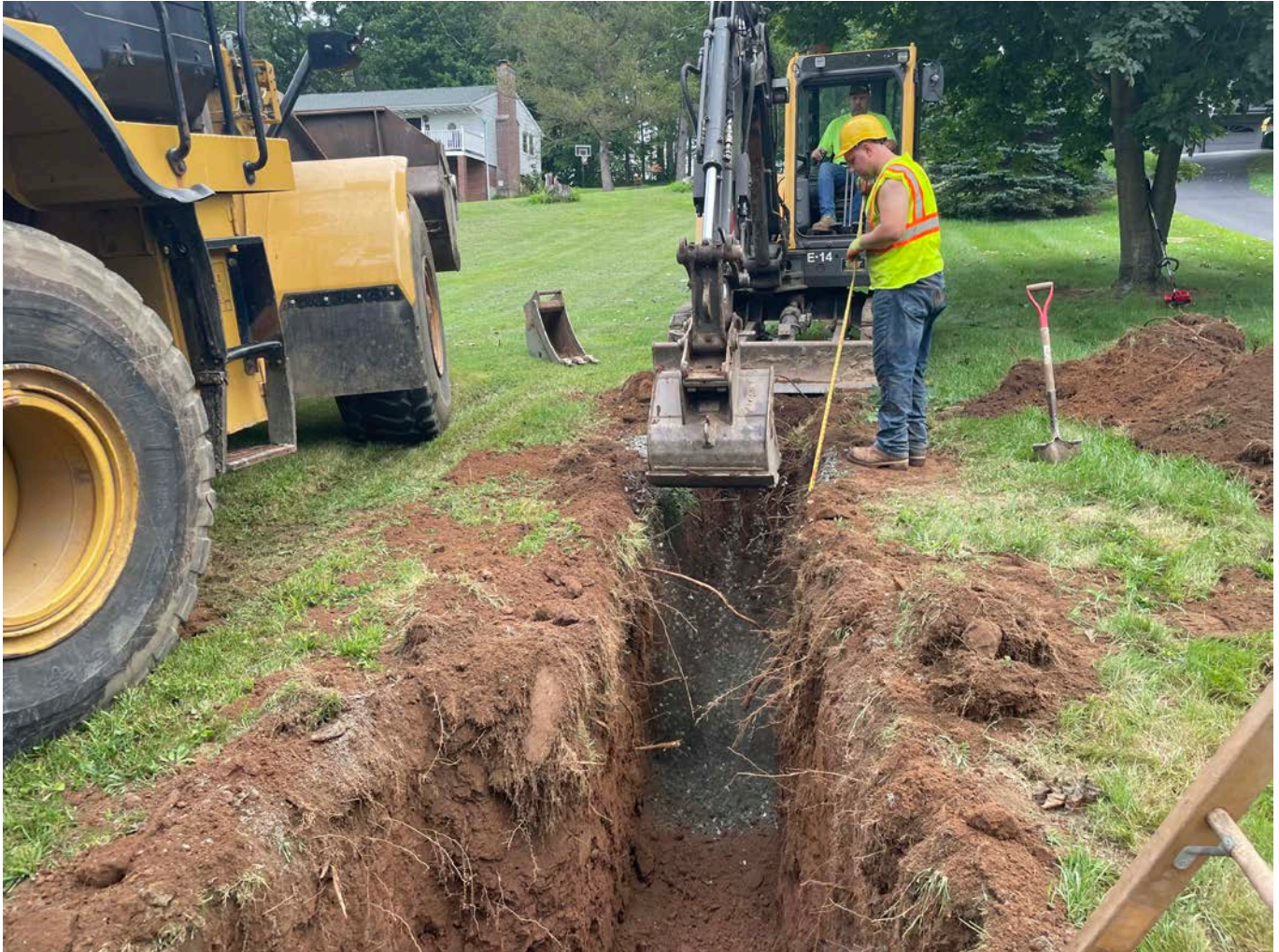
Picture 5: Ludlow placing a bed of ¾” stone that will underlie a meter pit they will be installed in the trench at 119 Maple Avenue as part of the installation of a 1.5” copper water service line. View to the east.
