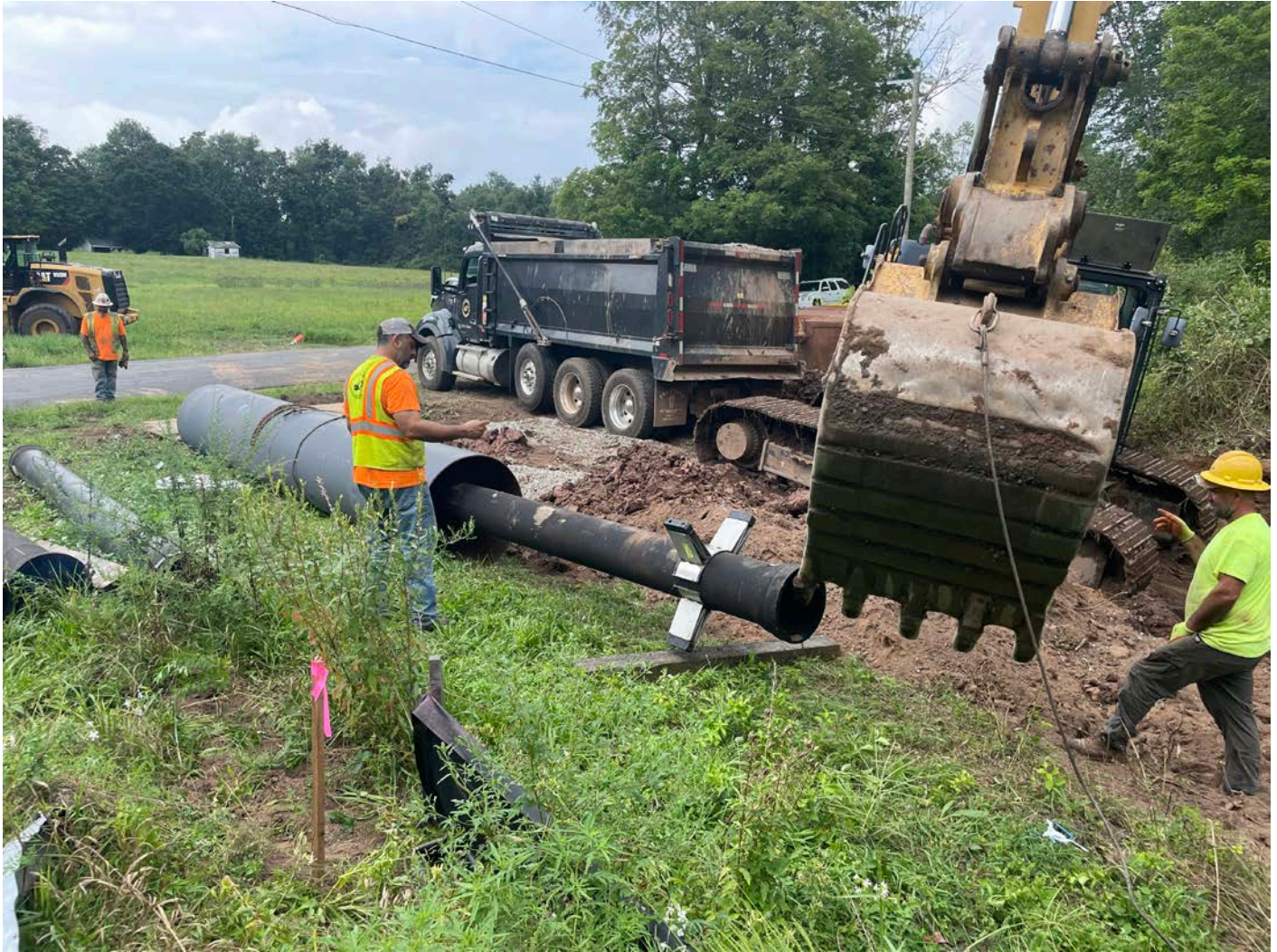
Picture 10: Ludlow inserting 12" DIP with spacers attached to it inside of 36" steel conduit for placement across the stream bed of Ball Brook as part of the Maiden Lane stream crossing. View to the northwest.
