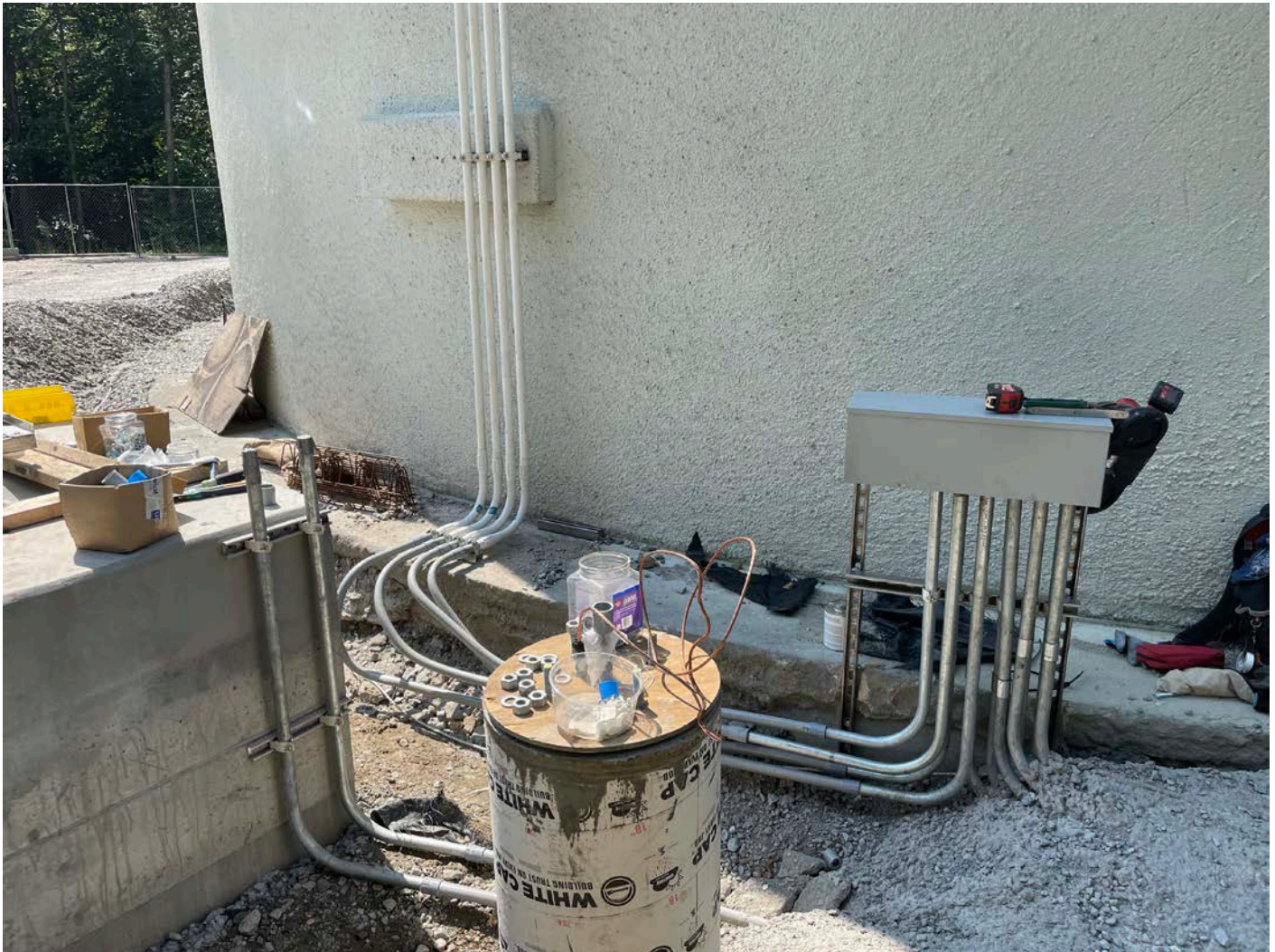
Picture 10: Conduits that A&R Electrical installed today on the pull box located on the northeast side of the water tank located east of the Shared Access Driveway in Middletown. View to the south.
