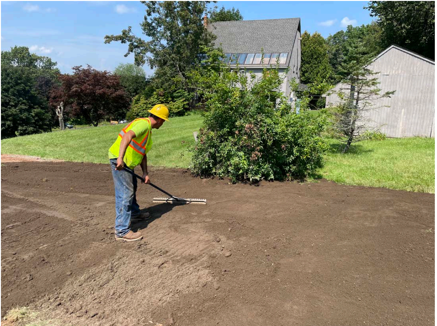
Picture 11: Ludlow raking out loam at the 109 Maple Avenue property, Durham, as part of restoration efforts following the installation of a 2" copper water service line. View to the northwest.
