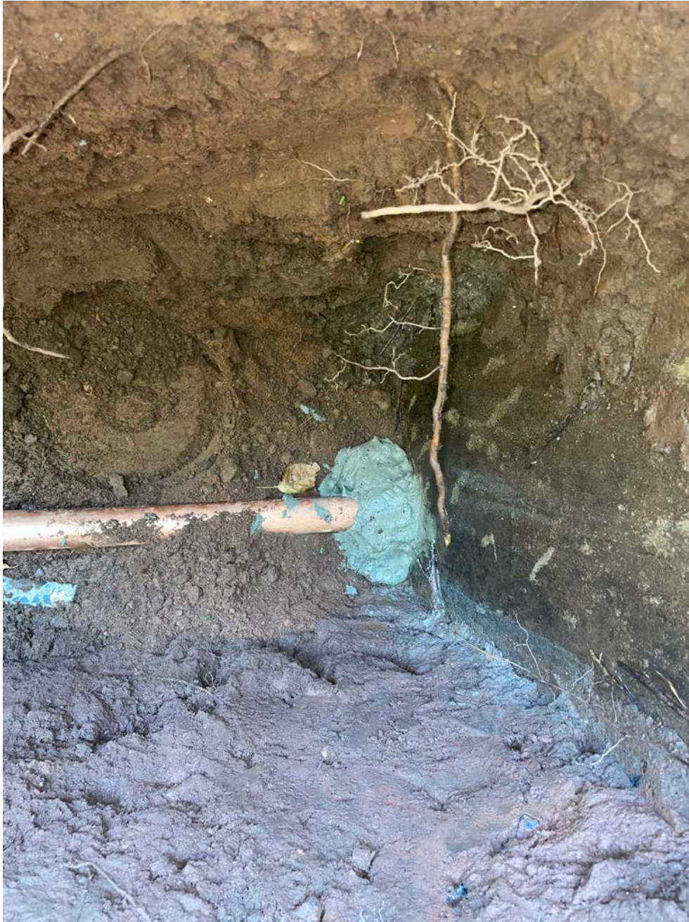
Picture 6: 2" copper water service pipe that has been cemented into place with non-shrink grout on the northern foundation of the 109 Maple Avenue residence. View to south.
