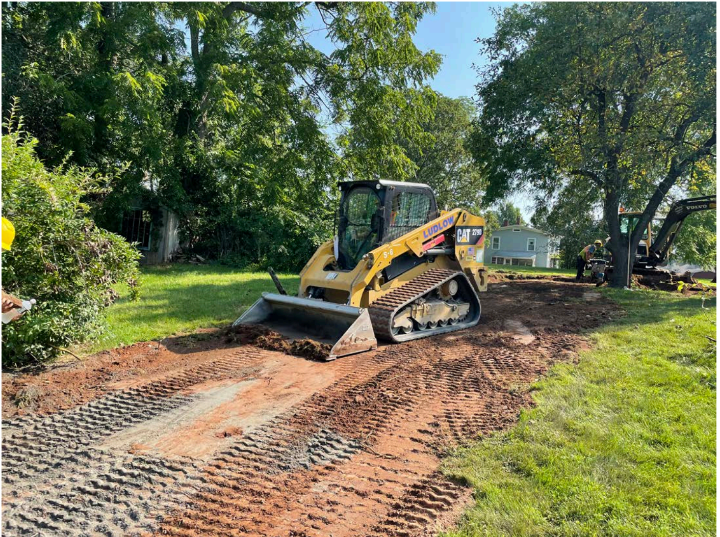
Picture 9: Ludlow grading loam as they restore the sections of the lawn at the 109 Maple Avenue residence that were disturbed during the Installation of a 2" copper water service line. View to the northeast.
