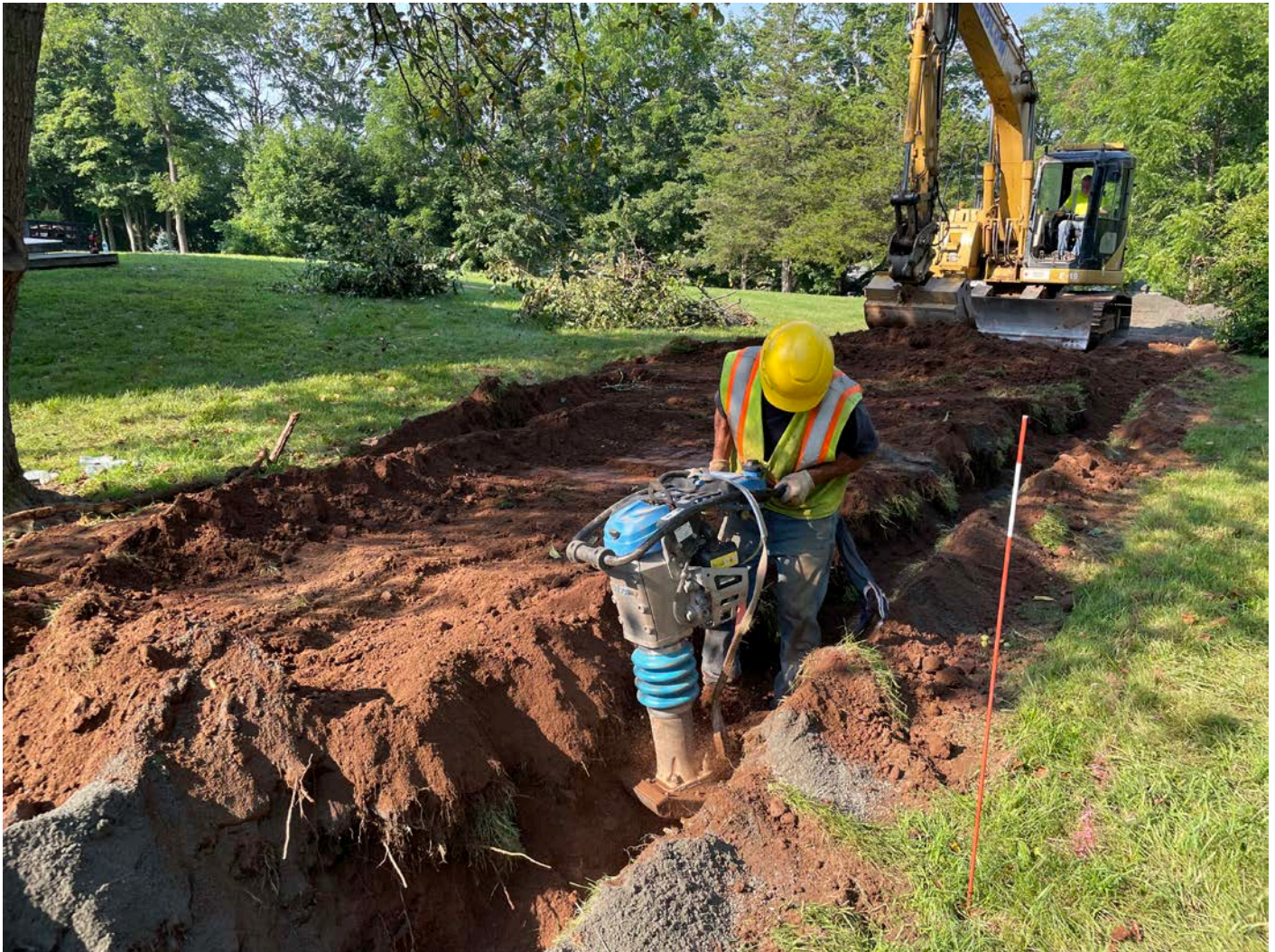
Picture 8: Ludlow using a jumping jack to compact native fill that was backfilled in 1' lifts at the 109 Maple Avenue residence in Durham. View to the southwest.
