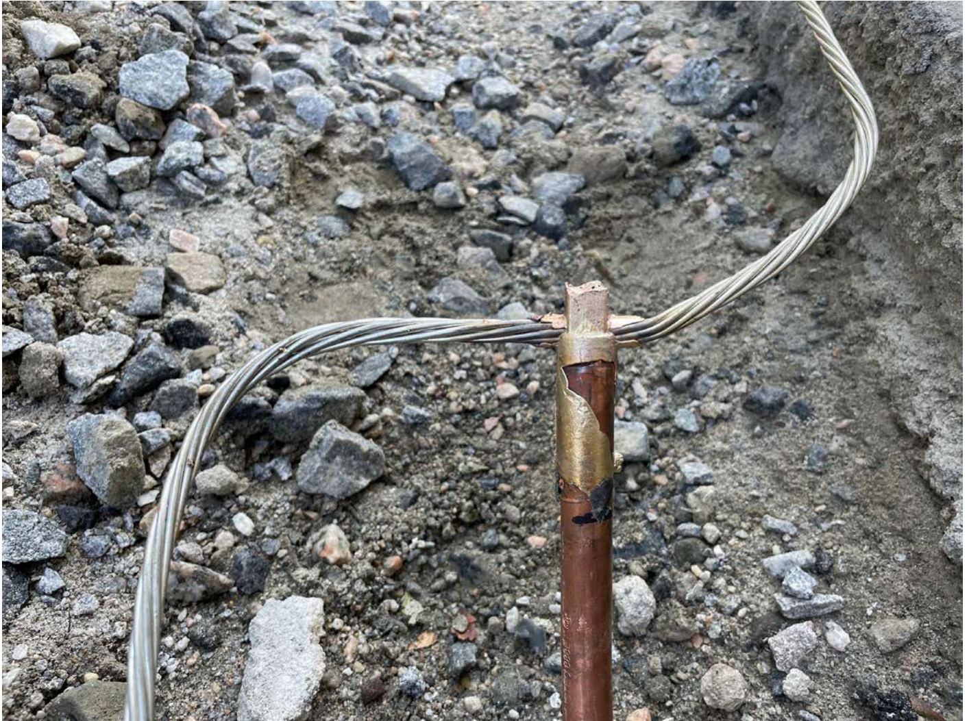
Picture 4: Grounding line that was cad welded to a grounding rod at the water tank work zone located east of the Shared Access Driveway in Middletown.
