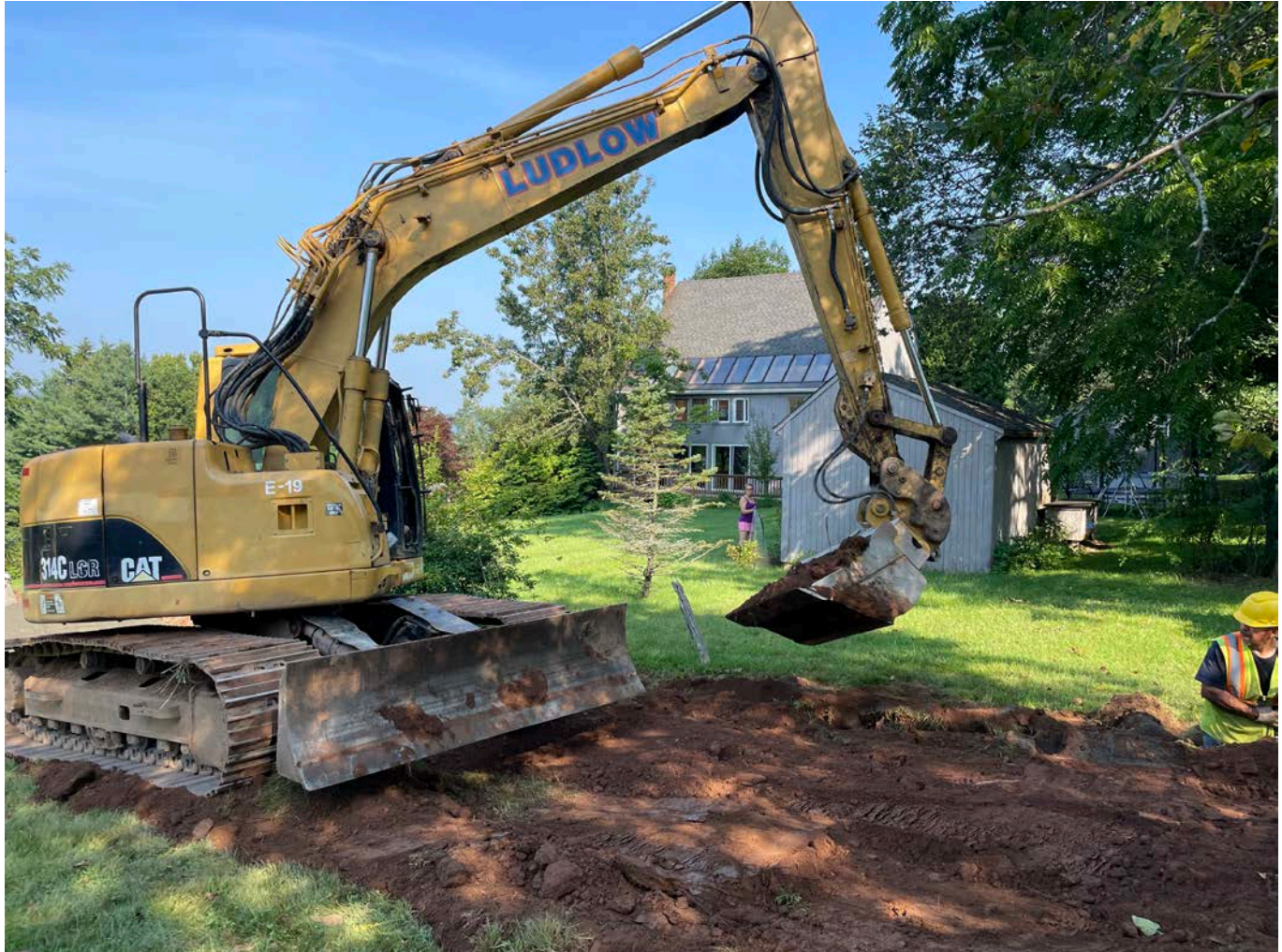
Picture 5: Ludlow backfilling the trench they excavated at the 109 Maple Avenue property for the installation of a 2" copper water service line. View to the north.
