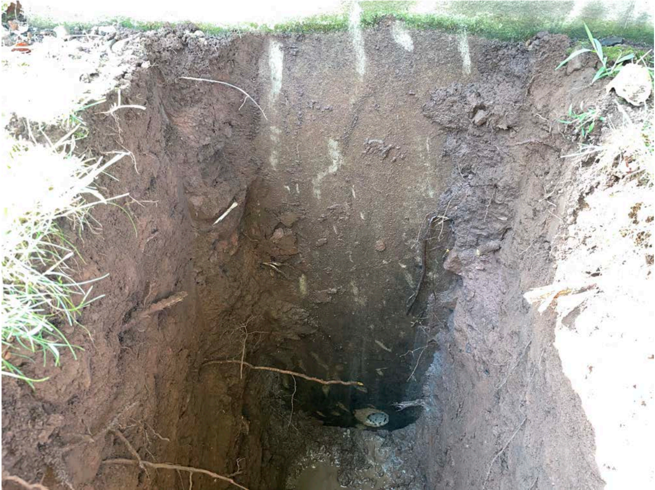
Picture 2: Hole that Ludlow cored through the northern foundation for the 109 Maple Avenue residence for the installation of a 2" copper water service line. View to the south.
