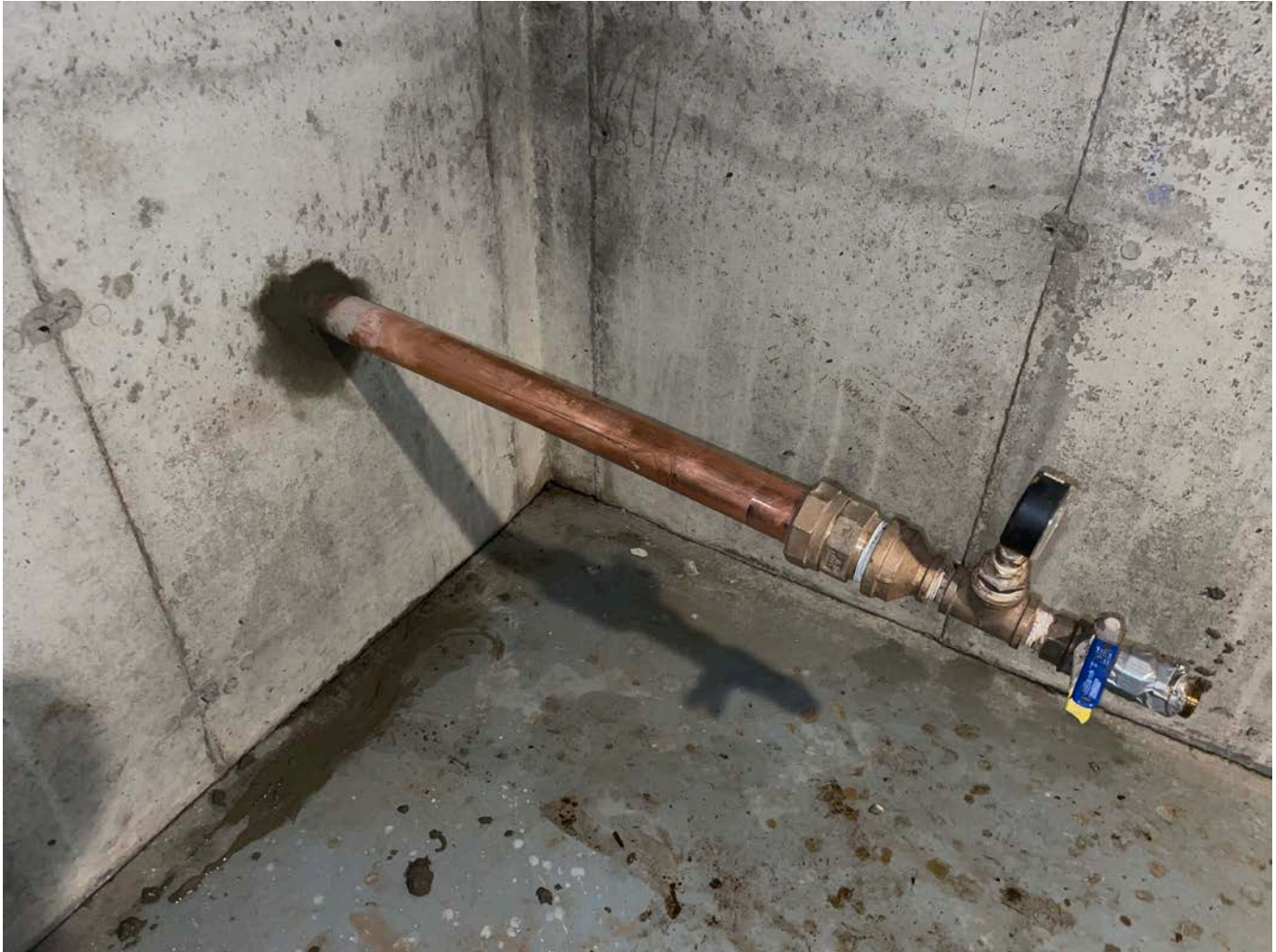
Picture 7: 2" copper water service pipe that has been cemented into place with non-shrink grout on the northern foundation of the 109 Maple Avenue residence. View to northeast.
