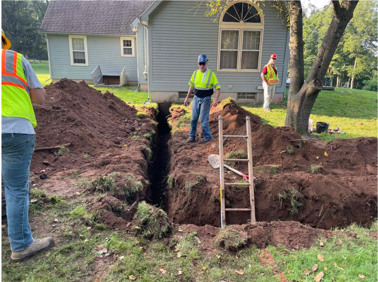
Picture 3: Trench that Ludlow has excavated for the installation of a 2" copper water service line at the 109 Maple Avenue property. View to the south.
