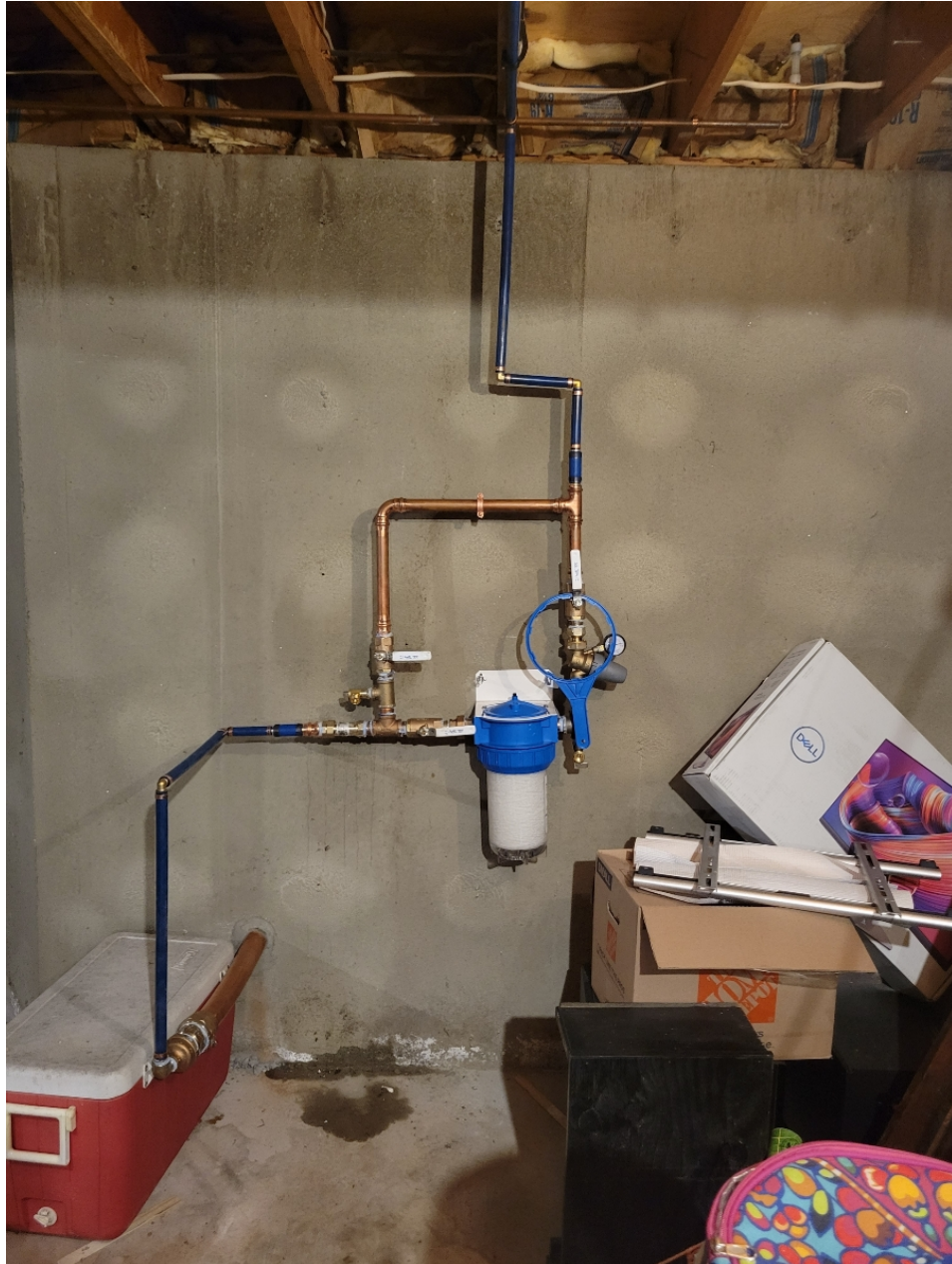
Picture 13: View of final water service components installed at the 95R Maple Avenue property by Fazzino Plumbing.
