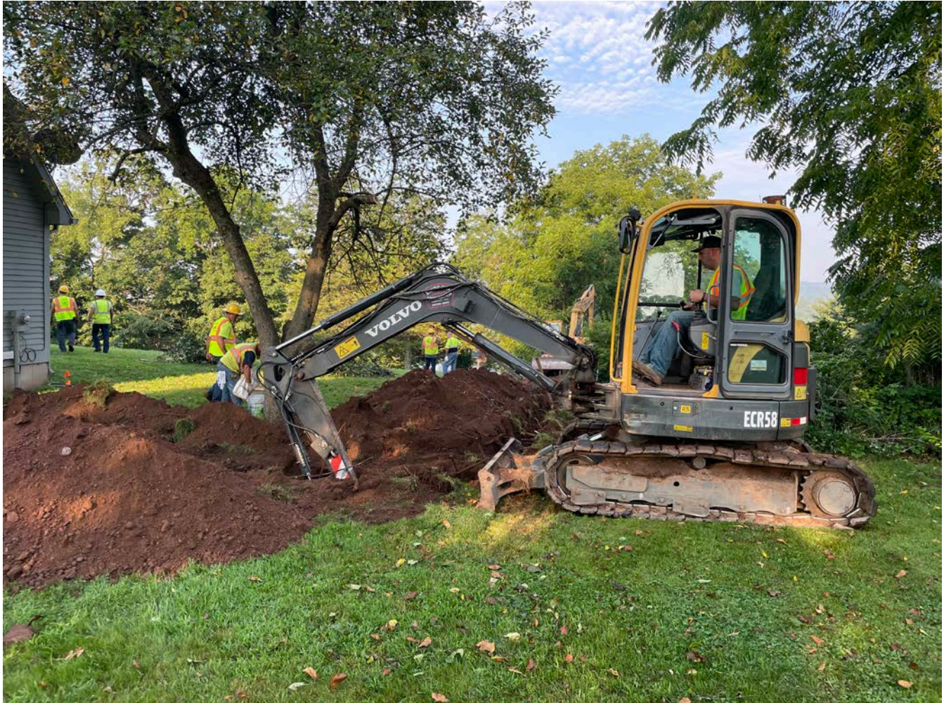
Picture 1: Ludlow excavating at the 109 Maple Avenue property as they install a 2" copper water service line. View to the southwest.
