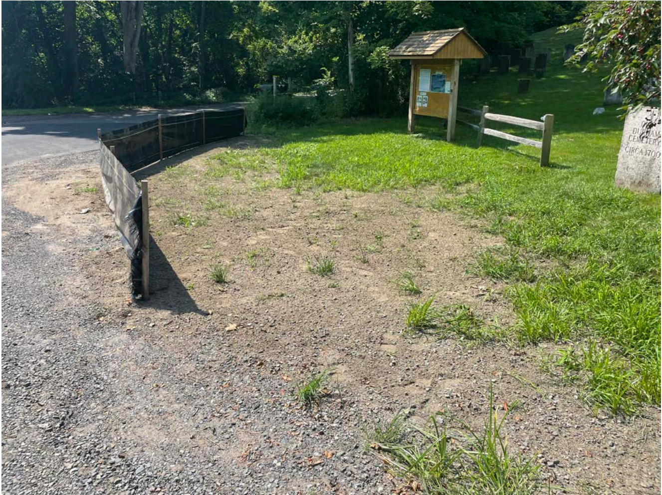
Picture 6: Loam, grass seed, and silt fence placed in front of the cemetery located on the corner of Main Street and Old Cemetery Road. View to southwest.
