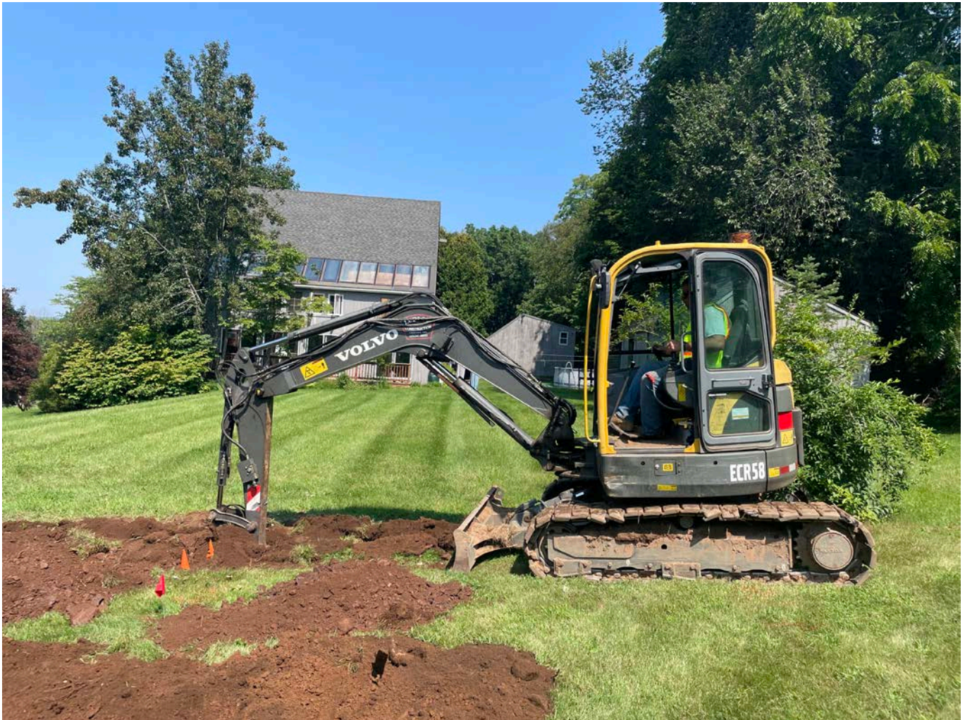
Picture 5: Ludlow excavating a trench ahead of the placement of 2" copper water service pipe at the 109 Maple Avenue property. View to the north.
