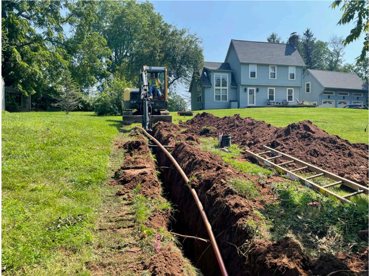
Picture 3: Ludlow excavating a trench ahead of the placement of 2" copper water service pipe at the 109 Maple Avenue property. View to the east.
