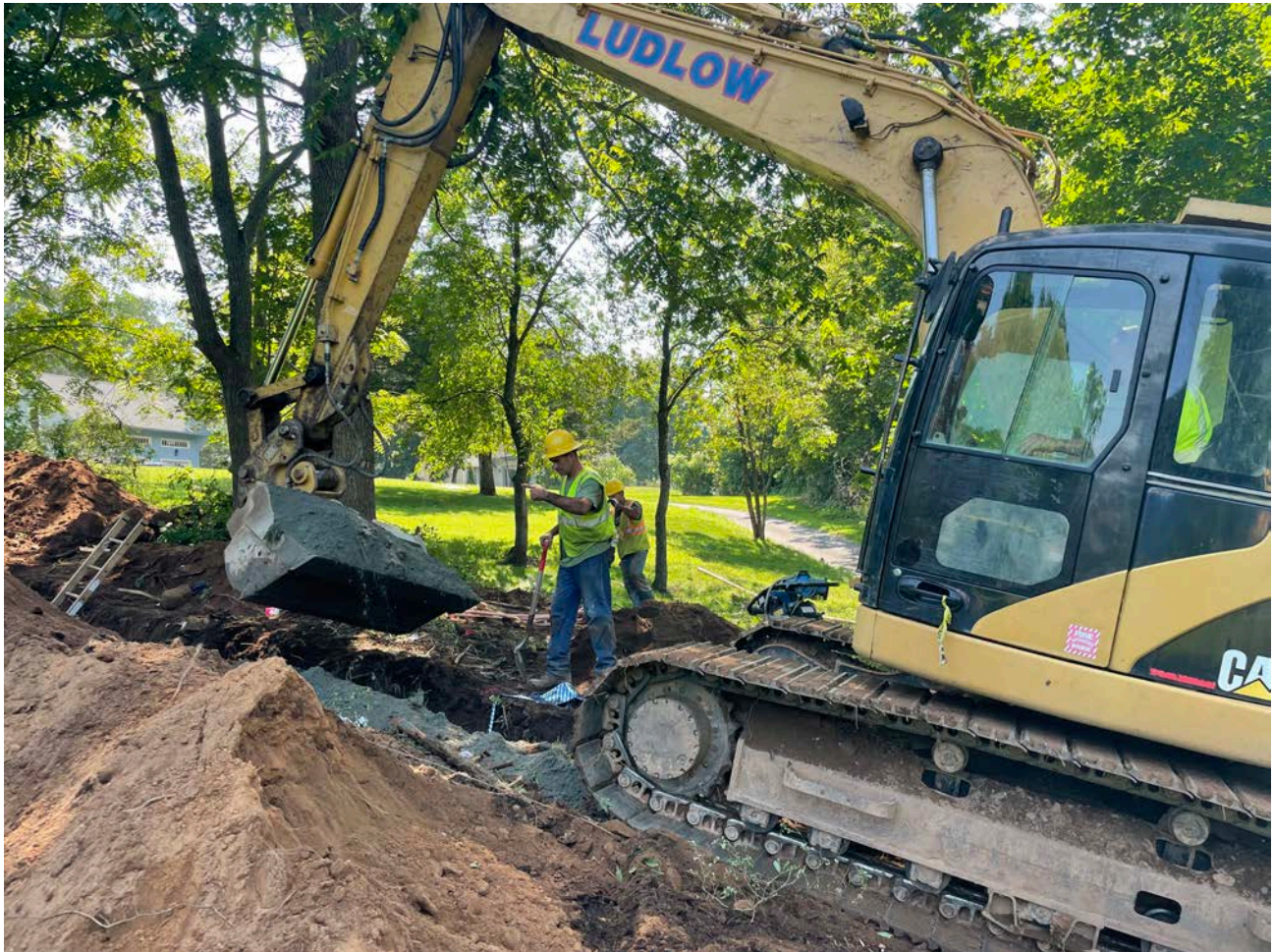
Picture 2: Ludlow placing sand over 2" copper water service line at the 109 Maple Avenue residence. View to the southeast.
