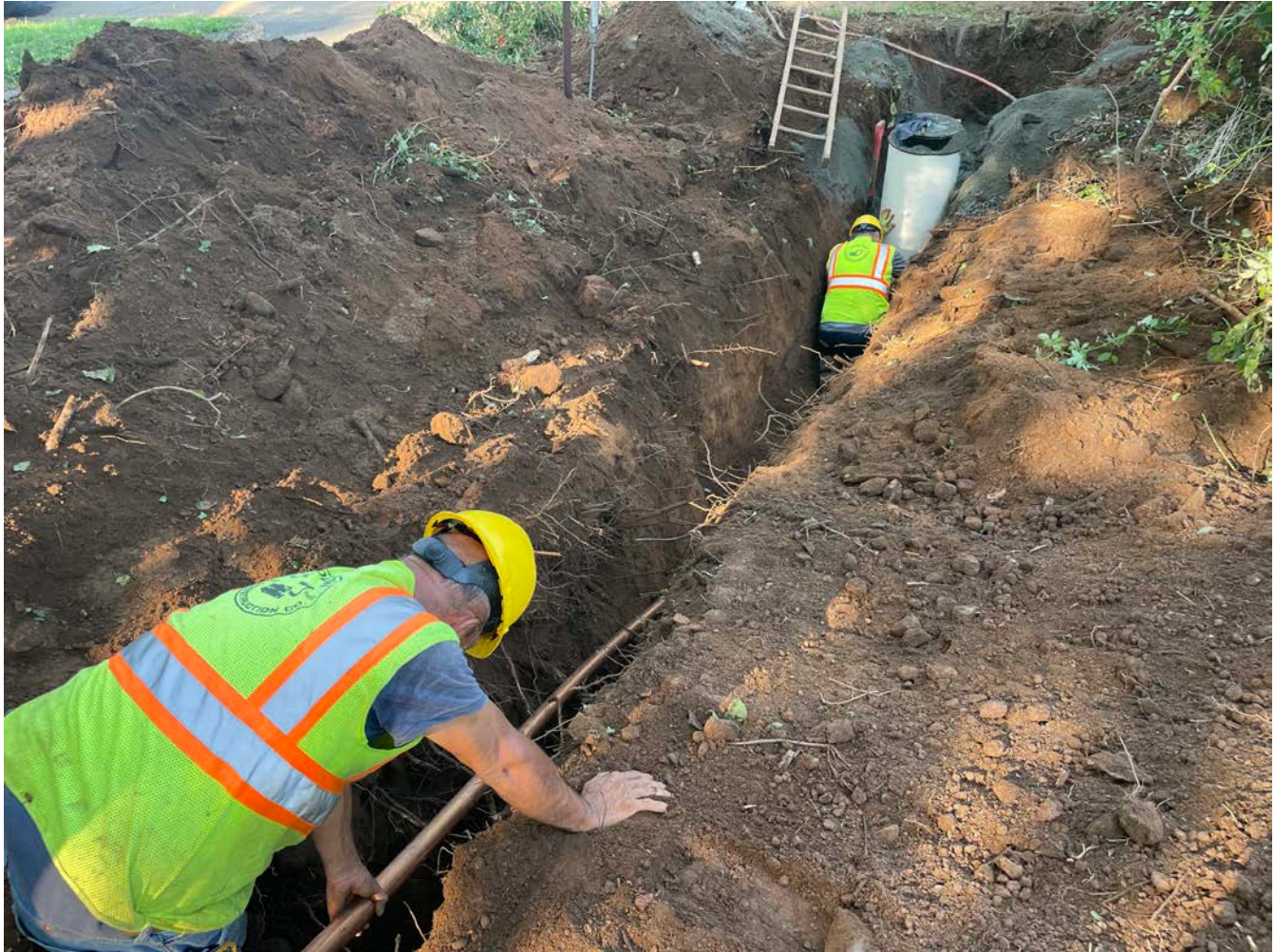
Picture 1: Ludlow placing 2" copper water service line at the 109 Maple Avenue residence. View to the southwest.
