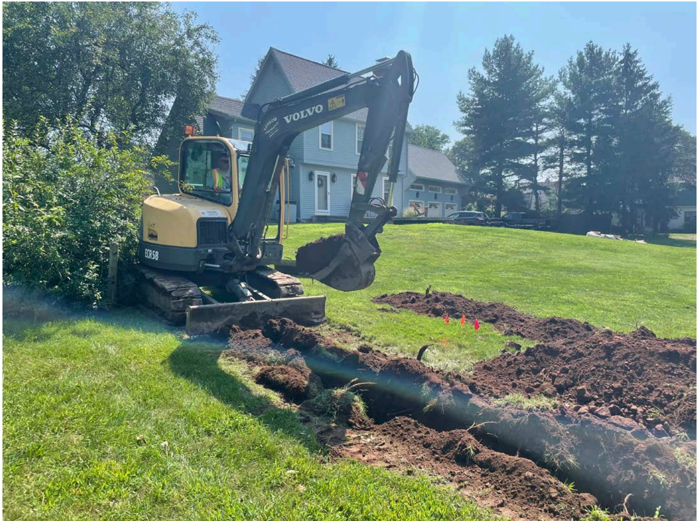
Picture 4: Ludlow excavating a trench ahead of the placement of 2" copper water service pipe at the 109 Maple Avenue property. View to the southeast.
