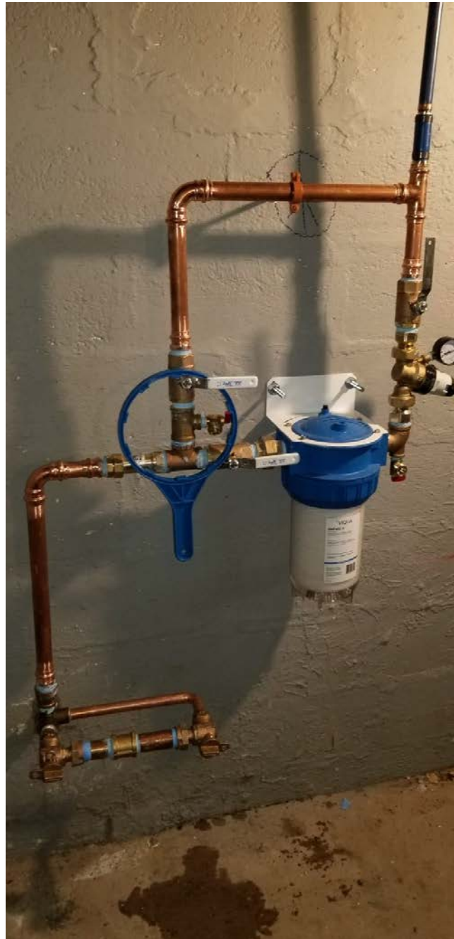
Picture 7: Installation of final water service components at 29 Maple Avenue, Durham.
